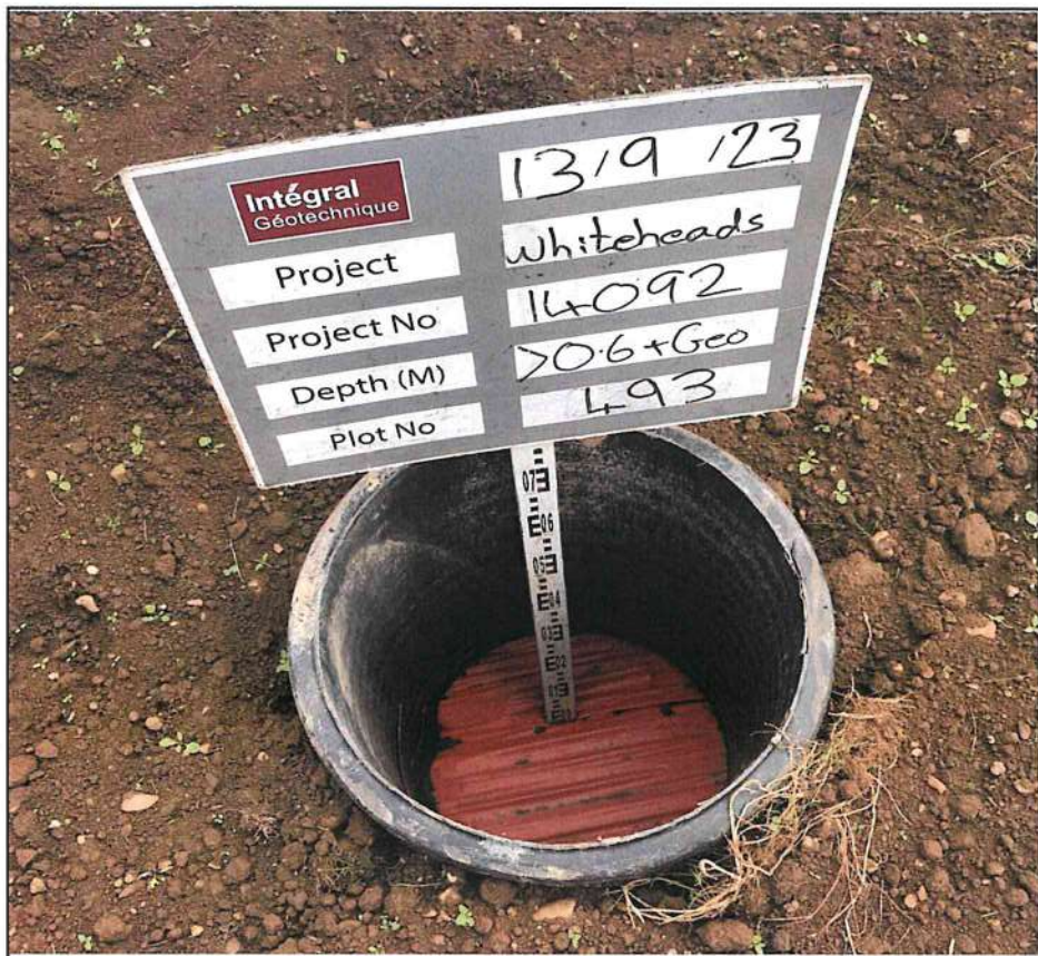
Plot 493 Membrane Placement
