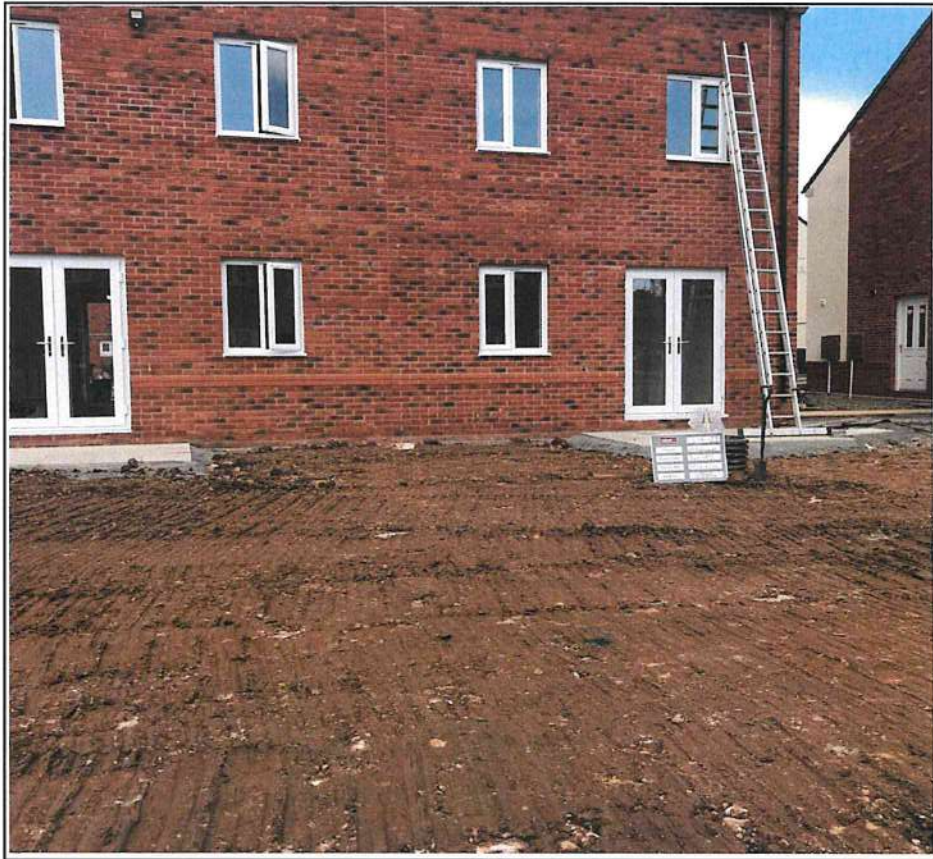
Plot 83 and 84 Capping Depth Check
