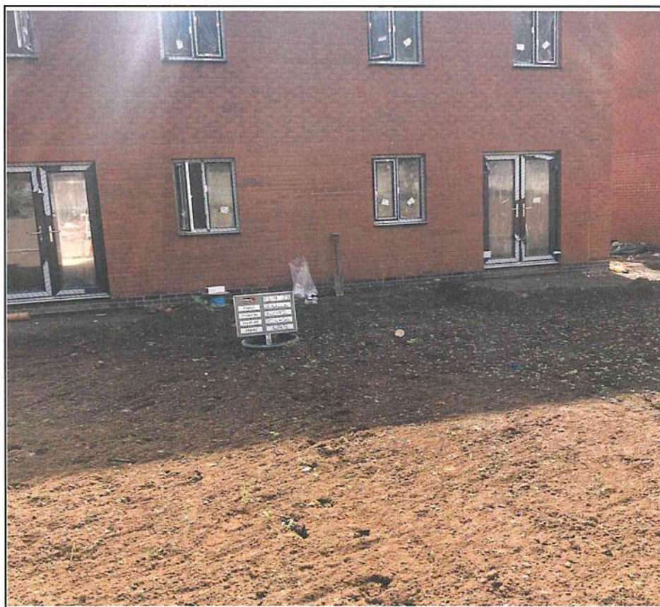
Plot 493 Capping Depth Check
