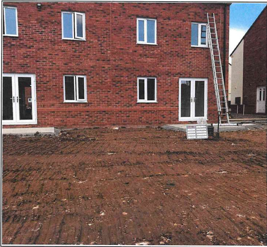
Plot 83 and 84 Capping Depth Check
