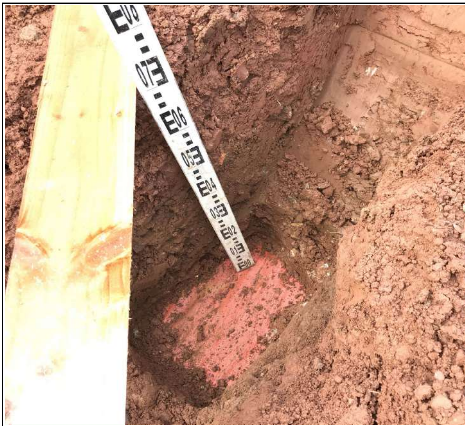
Plot 110 Membrane Placement
