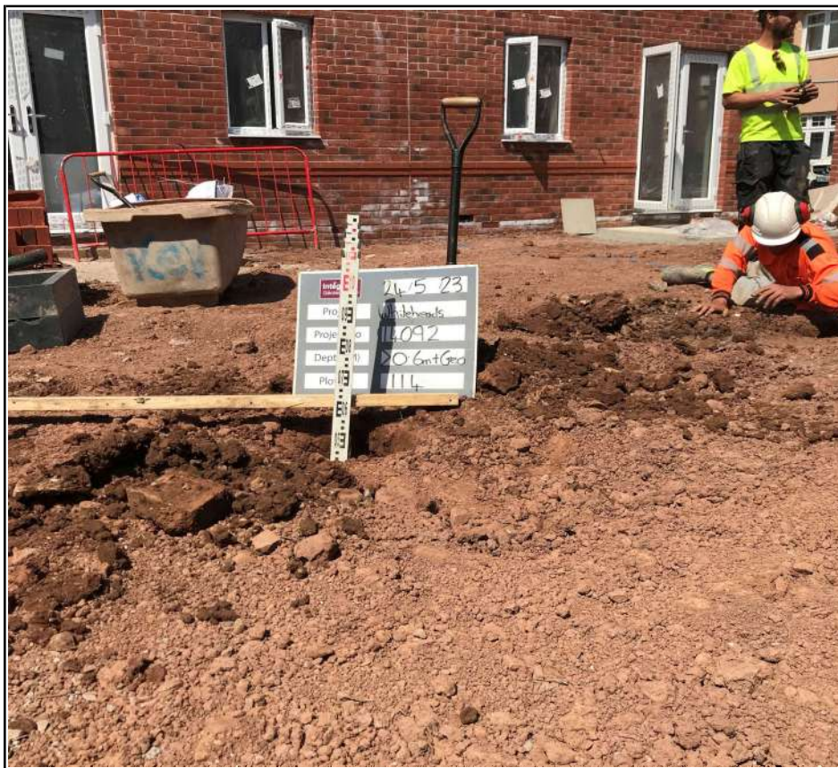
Plot 114 Capping Depth Check
