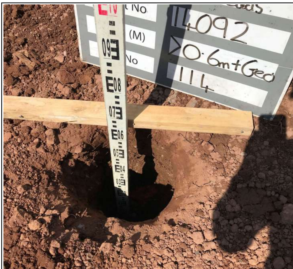
Plot 114 Excavation Trial Pit
