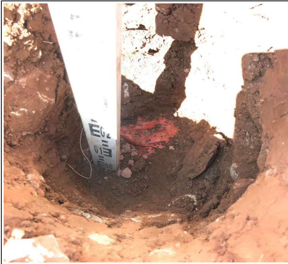
Plot 114 Membrane Placement
