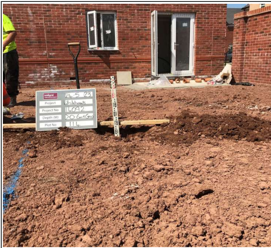
Plot 114 and 115 Capping Depth Check
