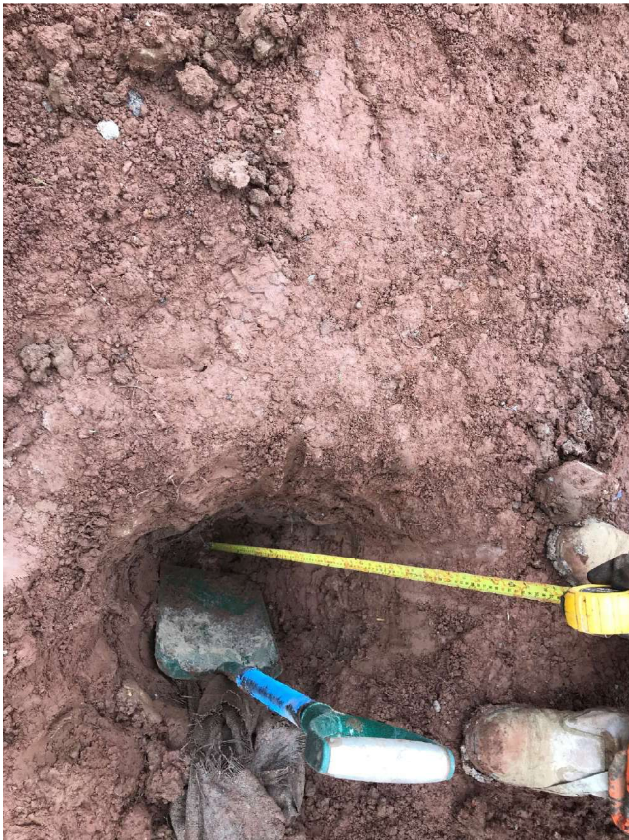
Second Hand dug trial pit dug in the landscape areas of Plots 122 to 130 of Block G confirm over 600mm of clean topsoil and subsoil over a separation membrane.
