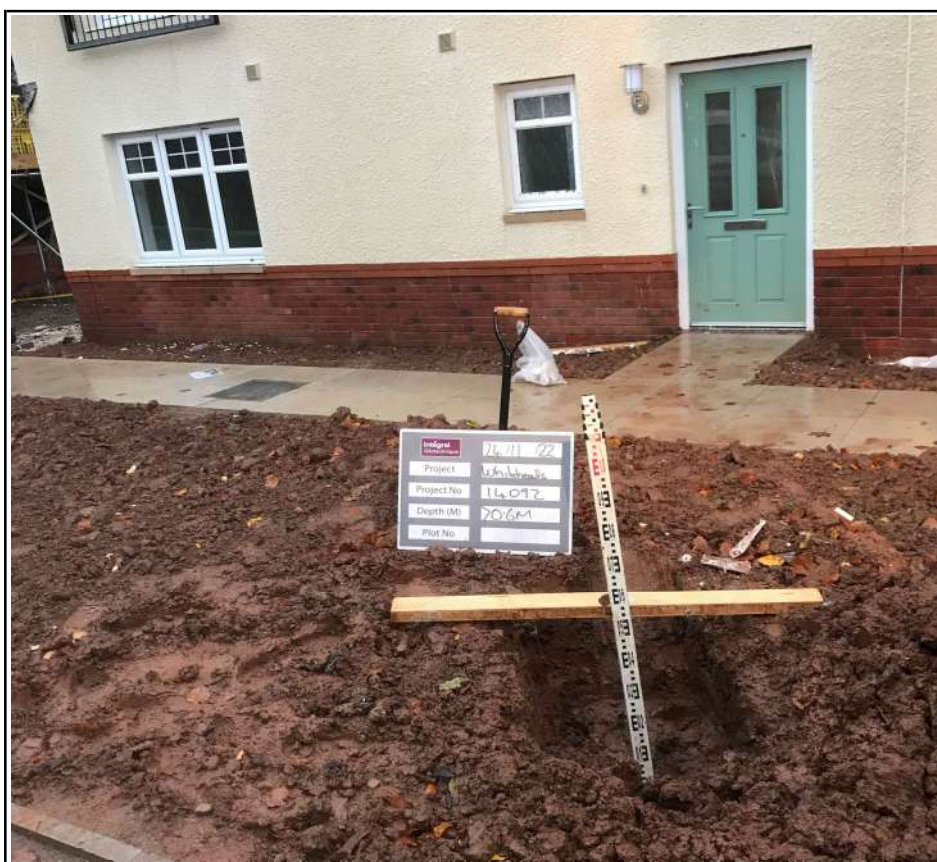
Block H Plots 131 to 139 Excavation Trial Pit
