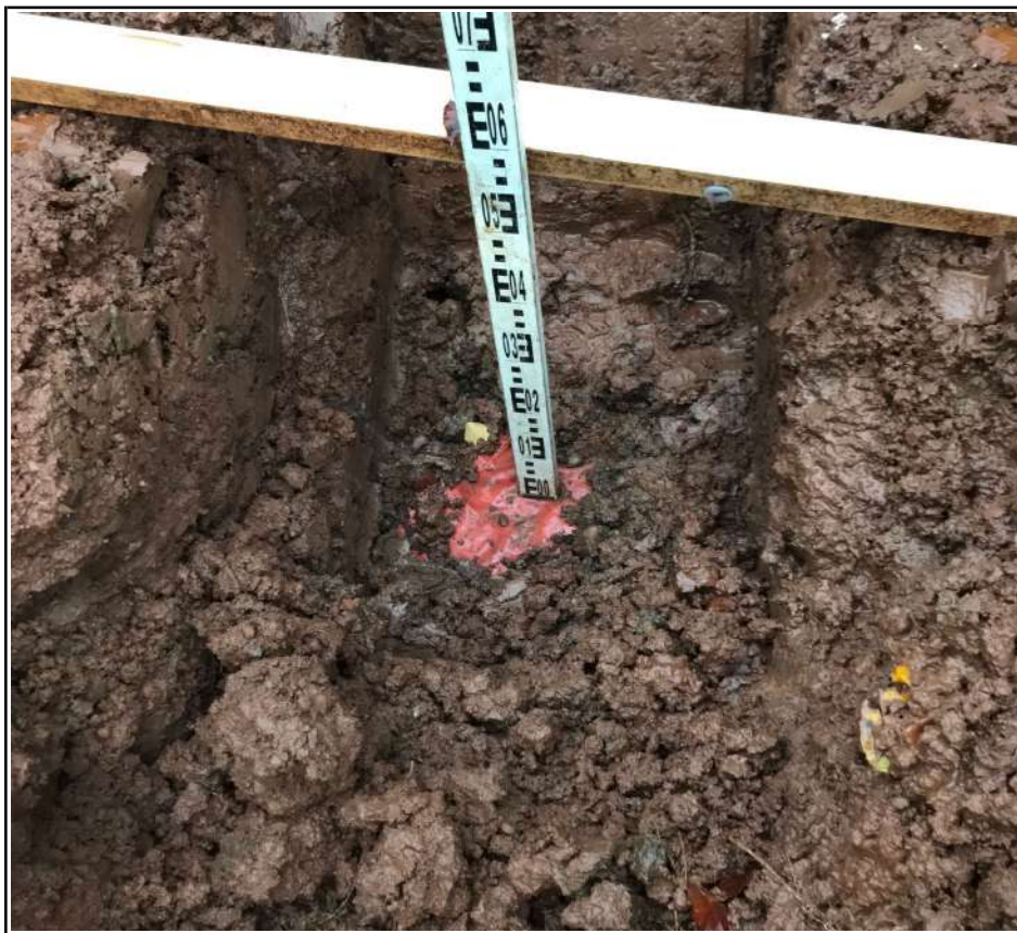
Block H Plots 131 to 139 Membrane Placement
