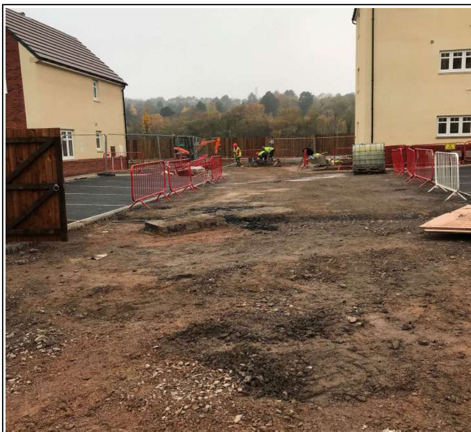
Block H Plots 131 to 139 Rear Carpark Area Prior to Tarmac Laying
