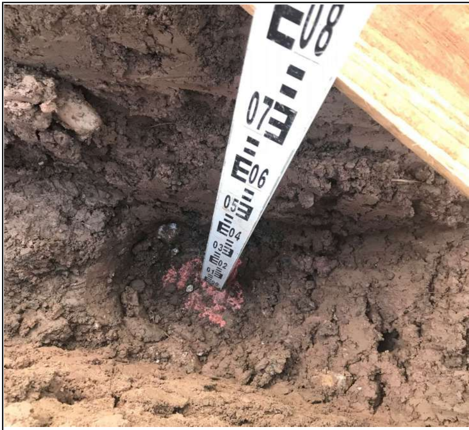
Plot 150 Membrane Placement
