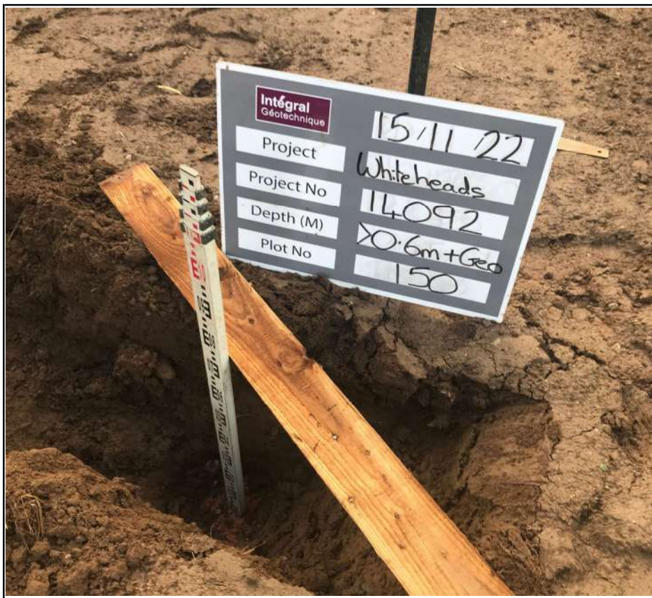
Plot 150 Excavation Trial Pit
