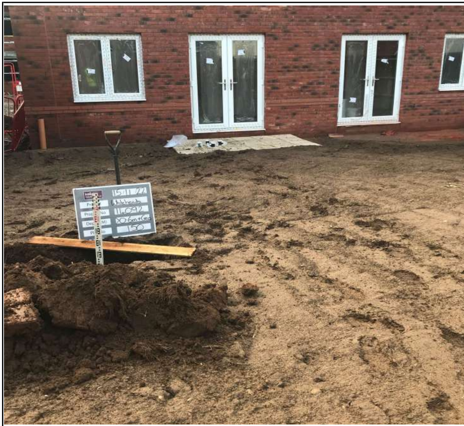
Plot 159 Capping Depth Check
