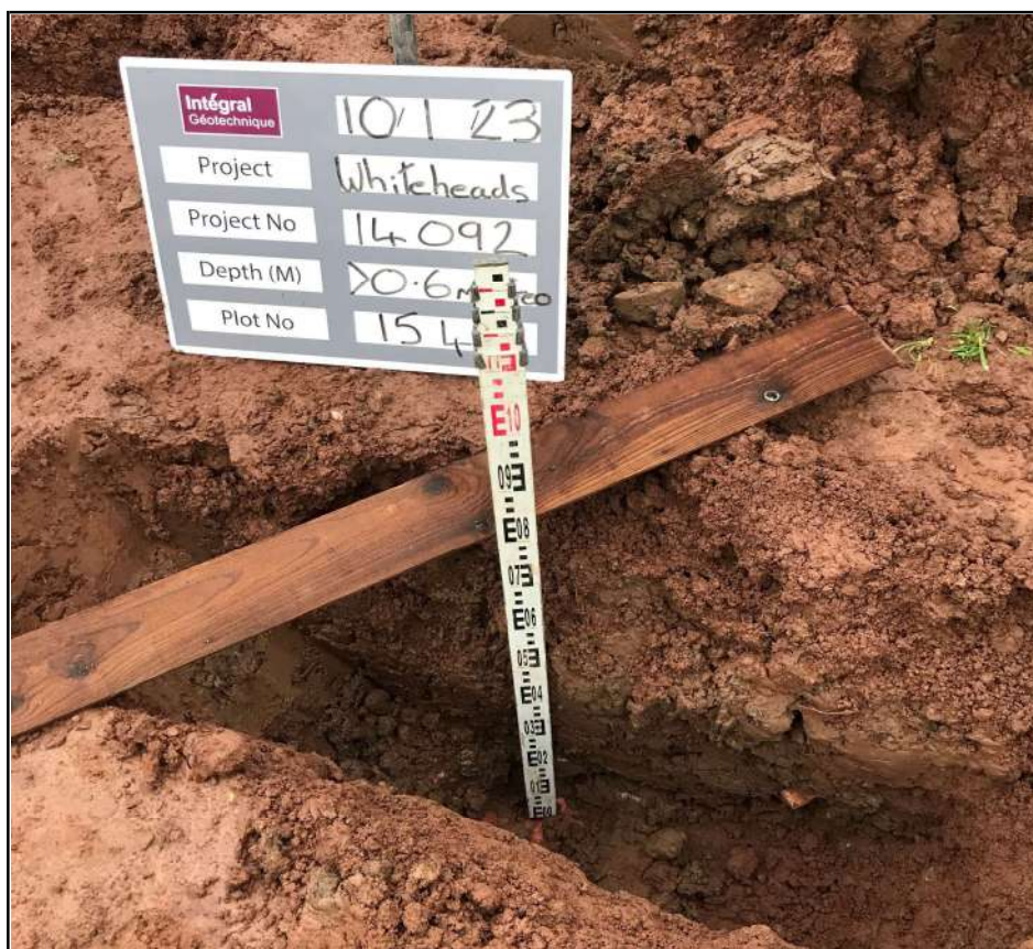
Plot 154 Excavation Trial Pit
