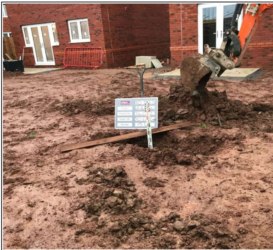
Plot 154 Capping Depth Check
