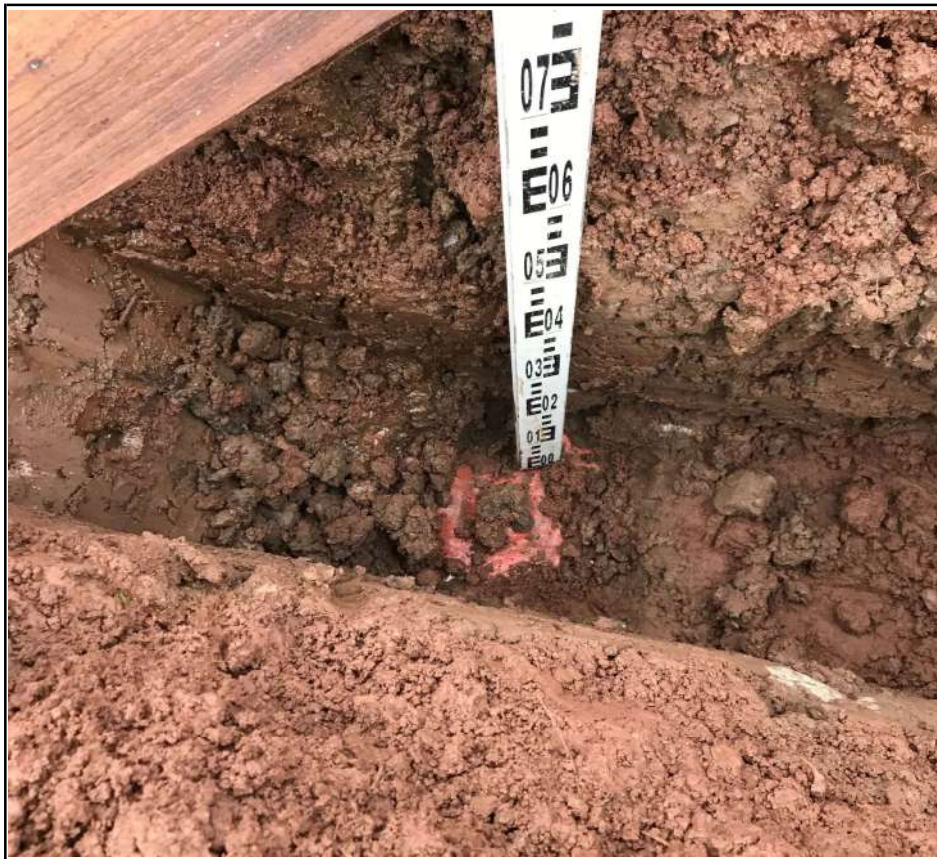
Plot 154 Membrane Placement
