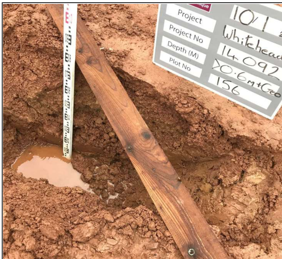
Plot 156 Excavation Trial Pit
