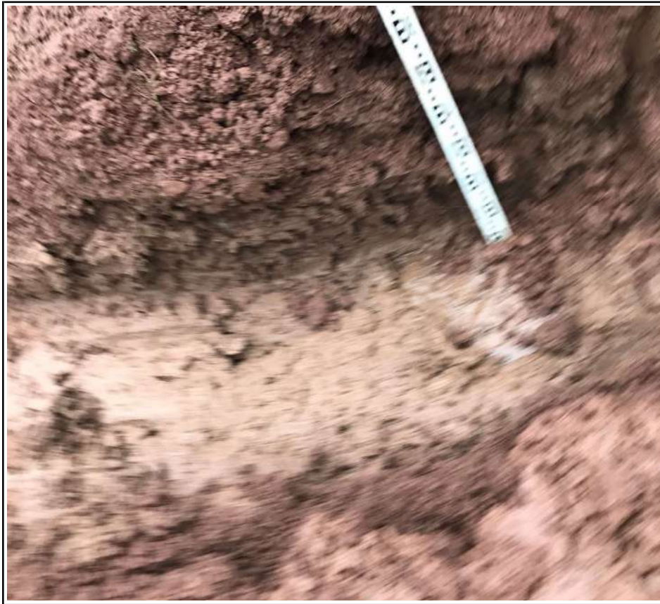
Plot 159 Membrane Placement
