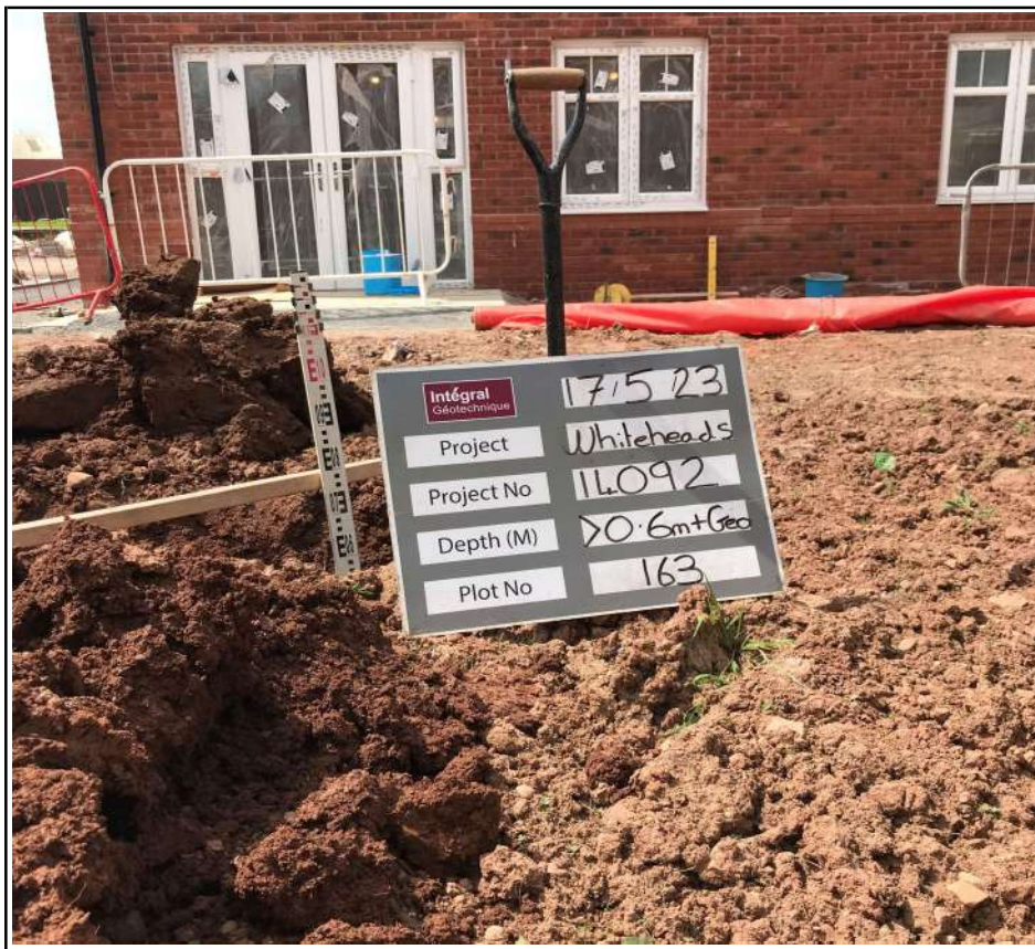
Plot 163 Membrane Placement
