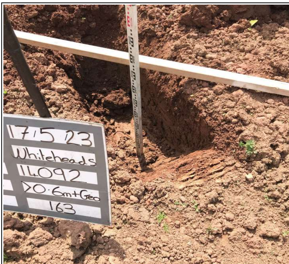
Plot 163 Membrane Placement
