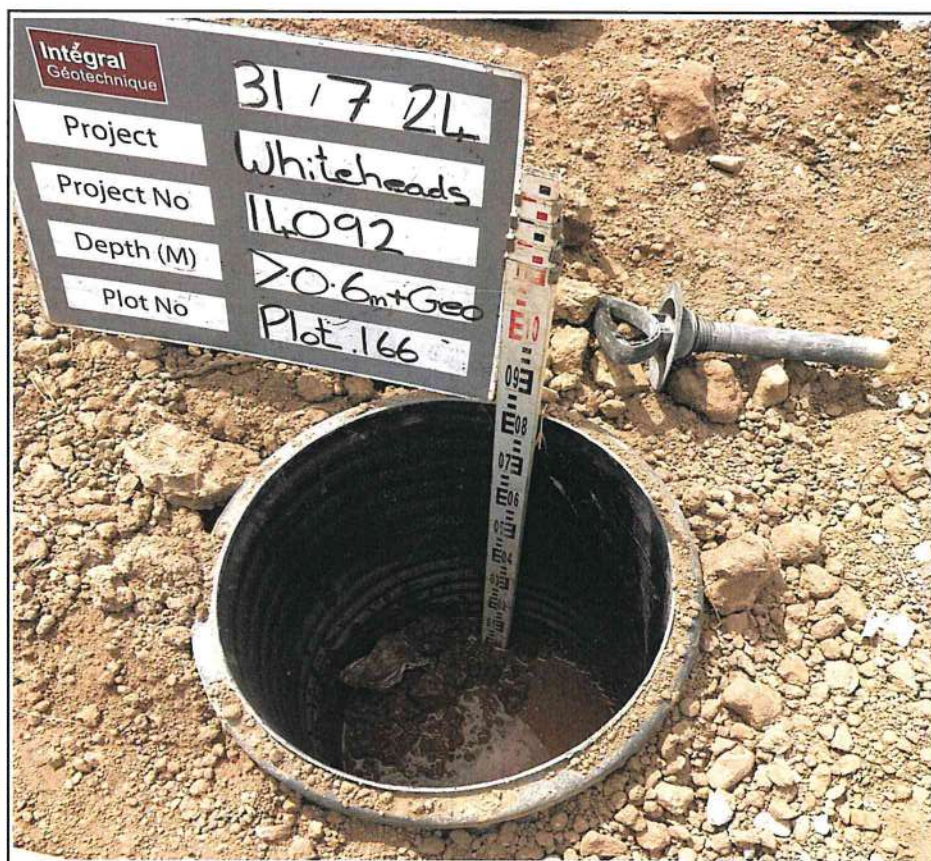
Plot 166 Excavation Trial Pit
