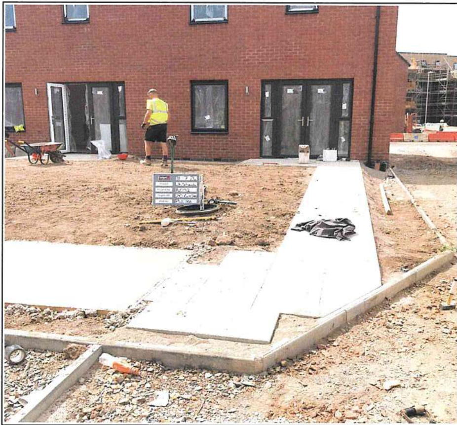
Plot 166 Capping Deph Check
