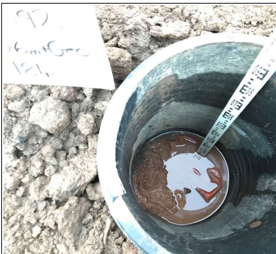
Plot 184 membrane Placement
