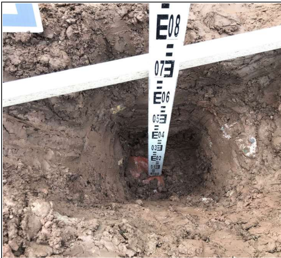
Plot 190 Membrane Placement
