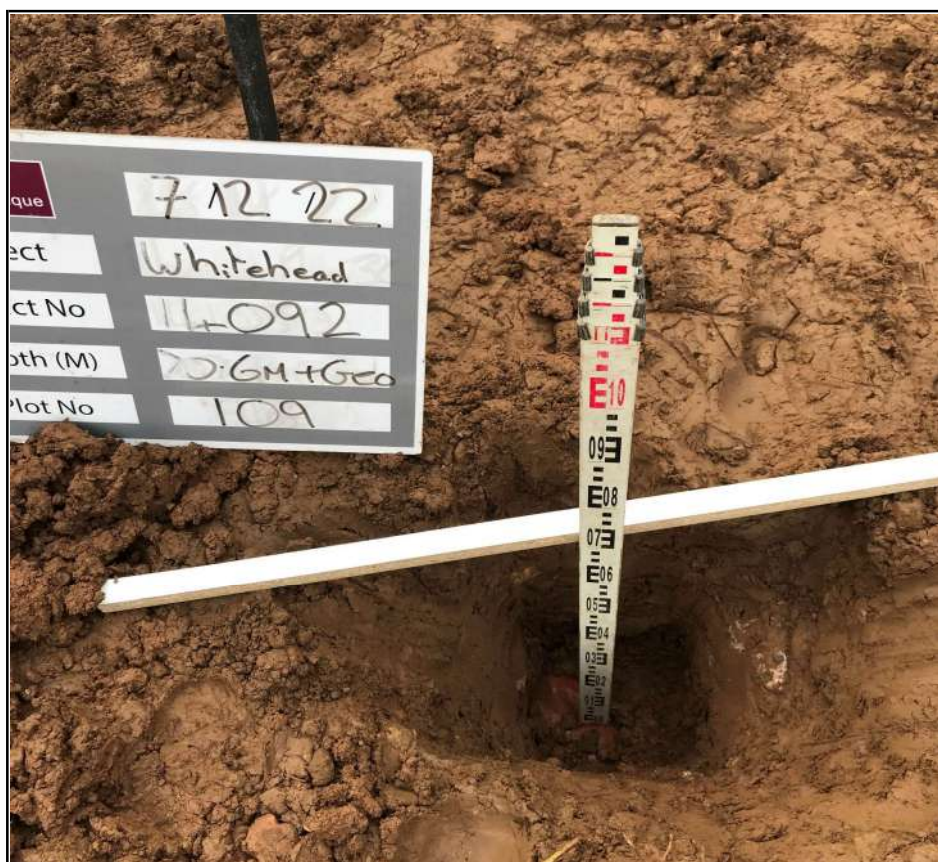
Plot 190 Excavated Trial Pit
