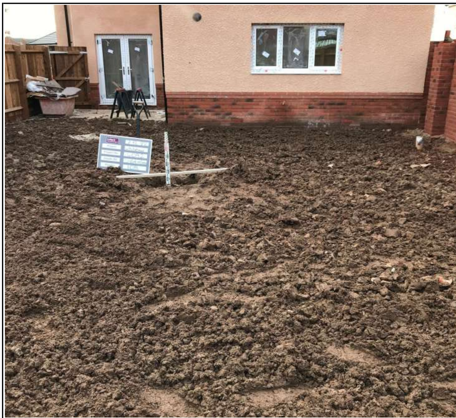
Plot 190 Capping Depth Check
