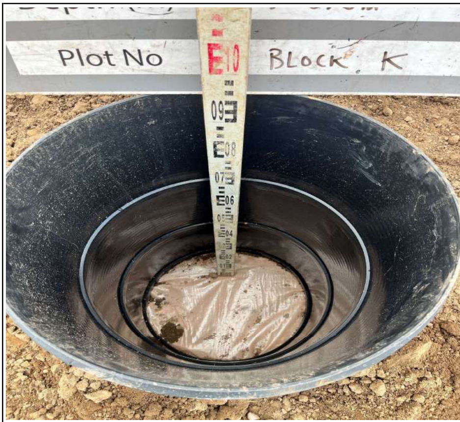
Block K Membrane Placement
