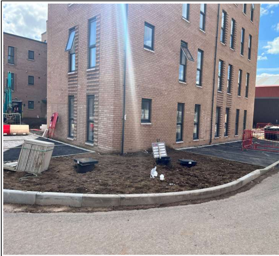
Block K Capping Depth Check
