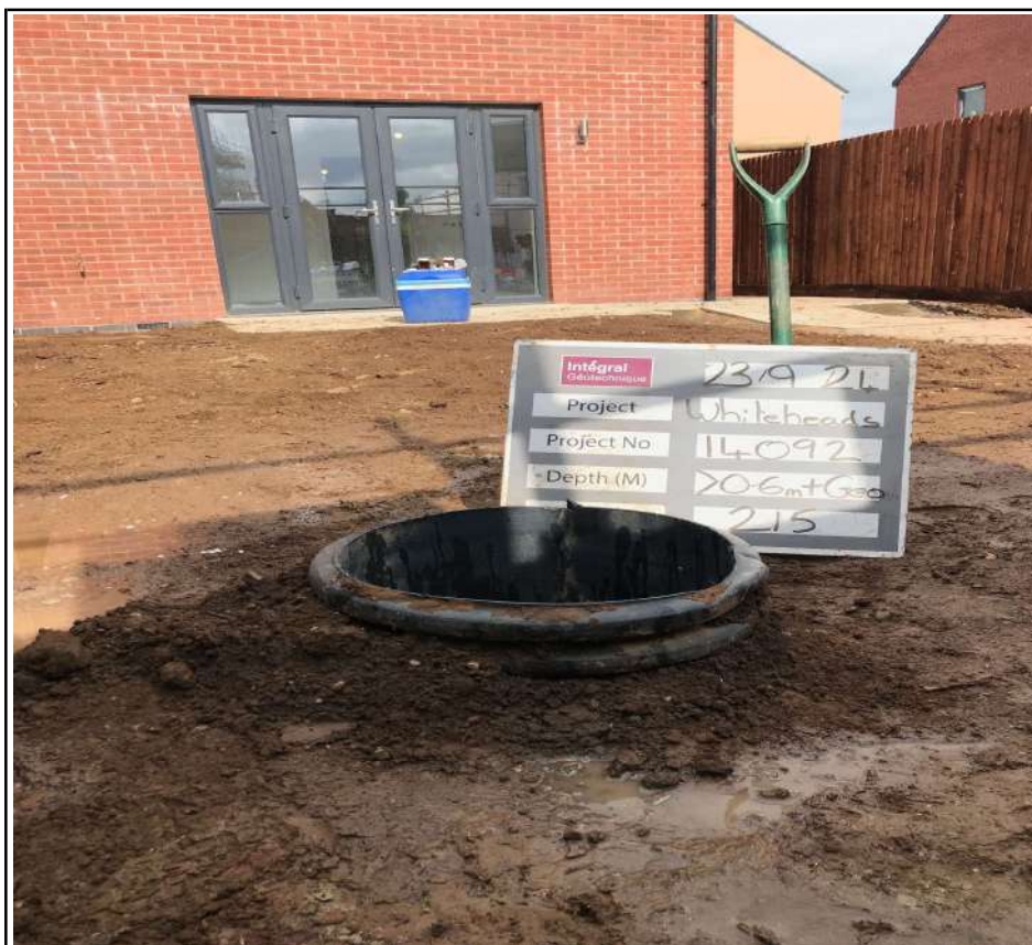
Plot 215 Capping Depth Check
