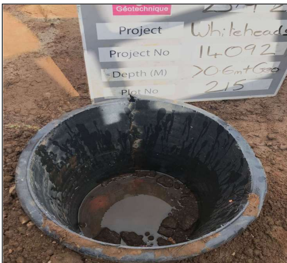
Plot 215 Membrane Placement
