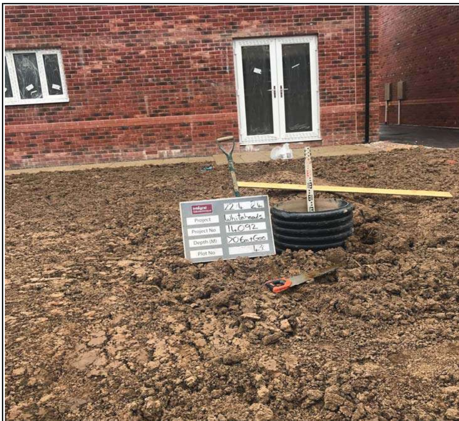
Plot 430 Capping Deph Check
