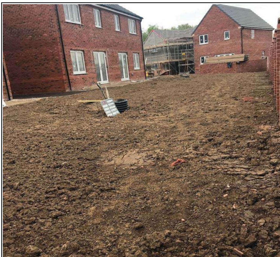
Plot 430 to 432 In-Filled Rear Gardens
