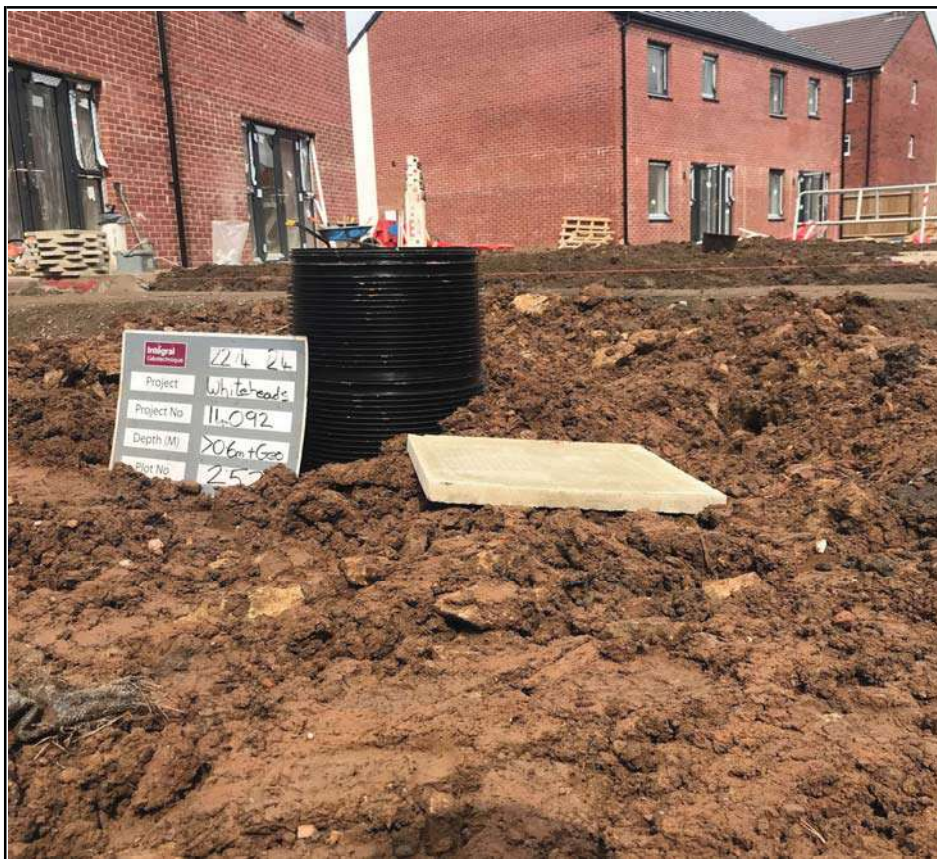
Plot 252 Capping Deph Check
