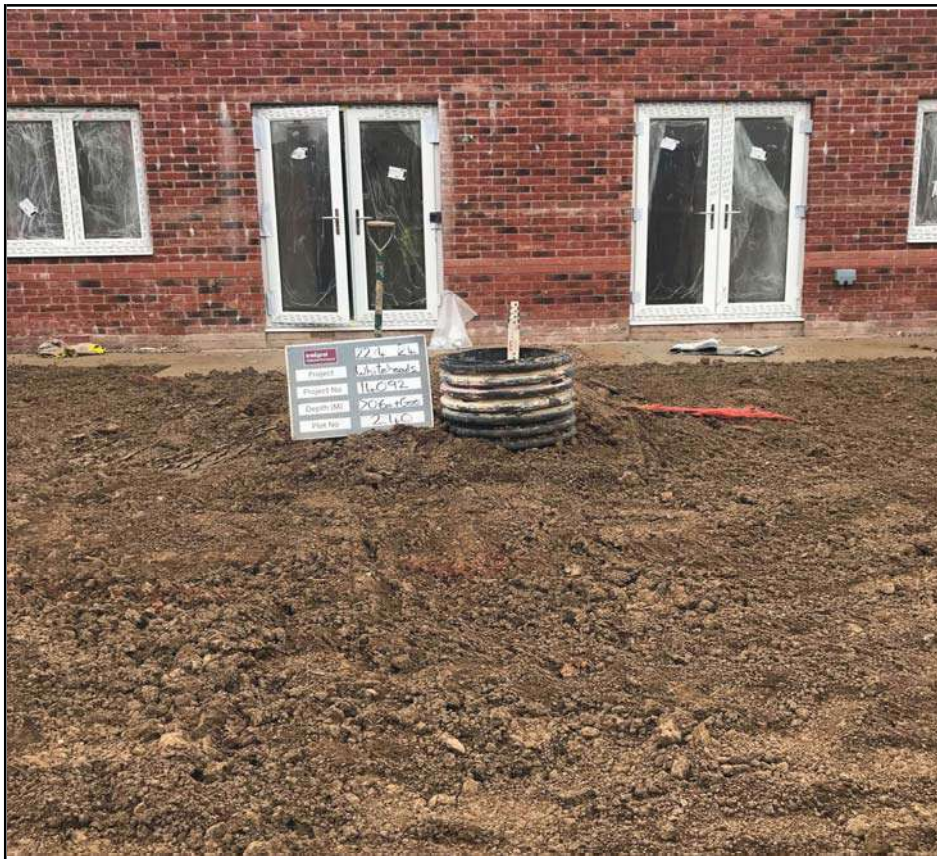
Plot 240 Capping Deph Check
