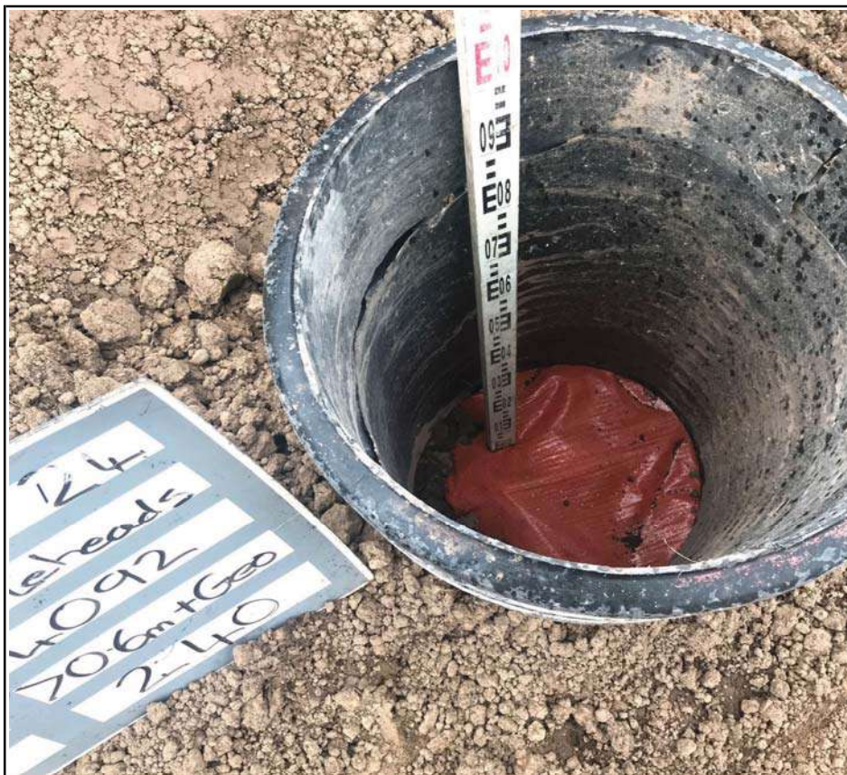
Plot 240 Membrane Placement
