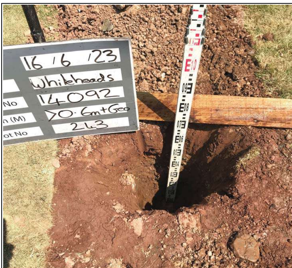
Plot 243 Trial Pit Excavation
