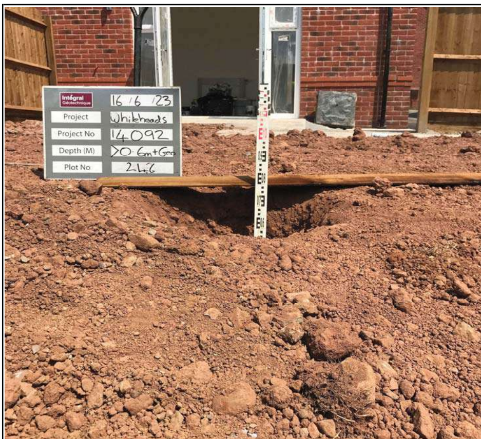
Plot 246 Capping Depth Check
