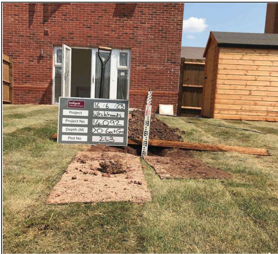
Plot 243 Capping Depth Check
