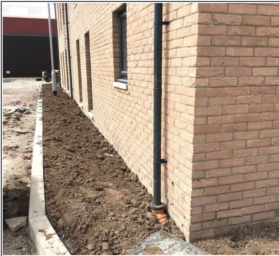
Apartment Block L South/West Flank
