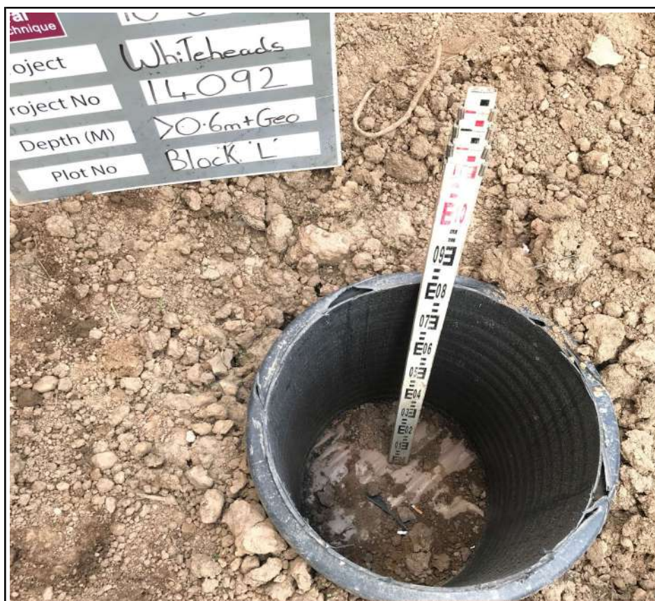
Apartment Block L Membrane Placement
