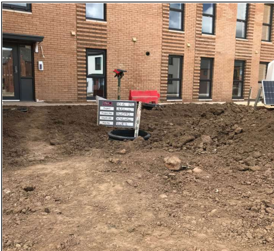
Apartment Block L Capping Deph Check
