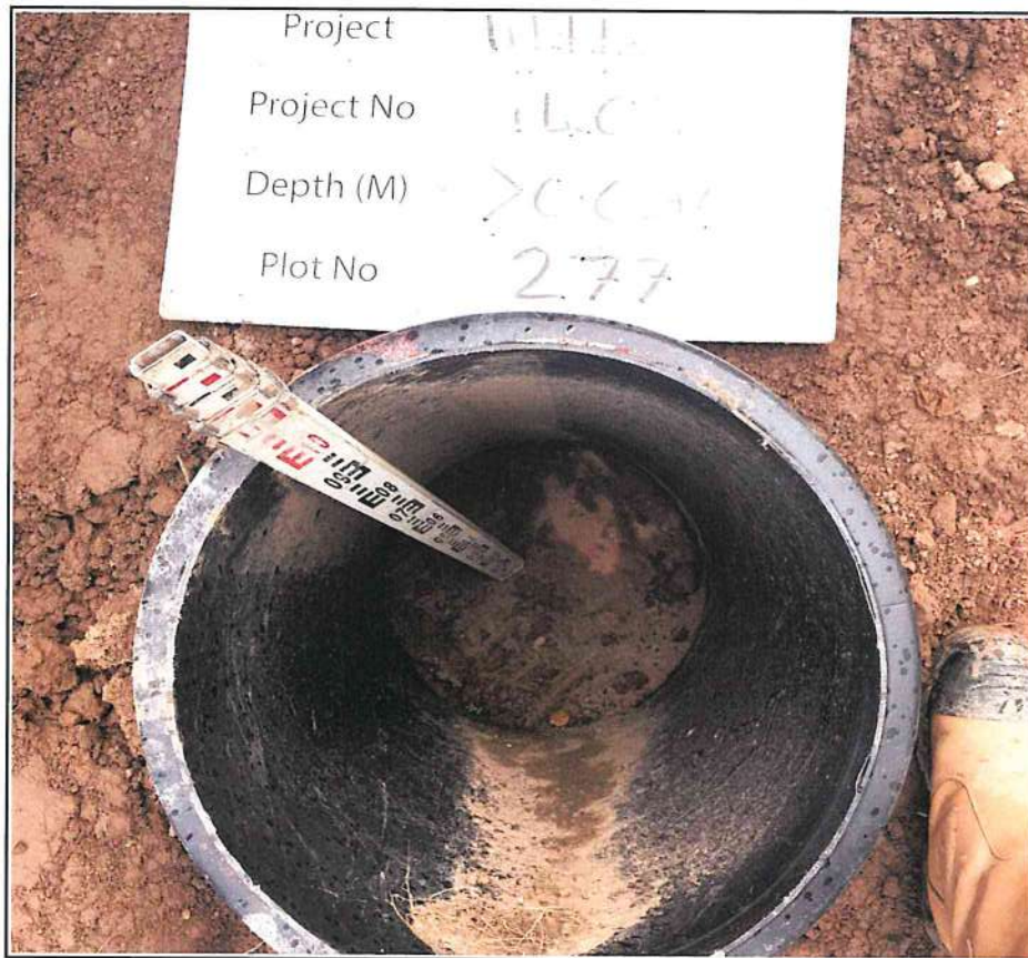
Plot 277 Membrane Placement
