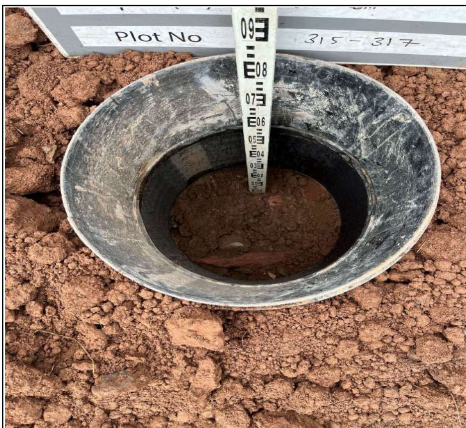
Plot 317 to 317 Membrane Placement
