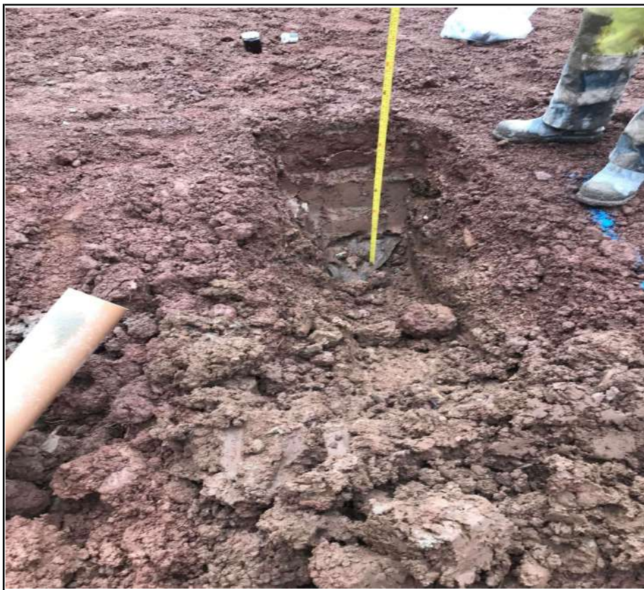
Plot 290 Capping Depth Check and Membrane Placement
