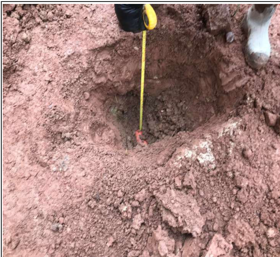
Plot 296 Capping Depth Check and Membrane Placement
