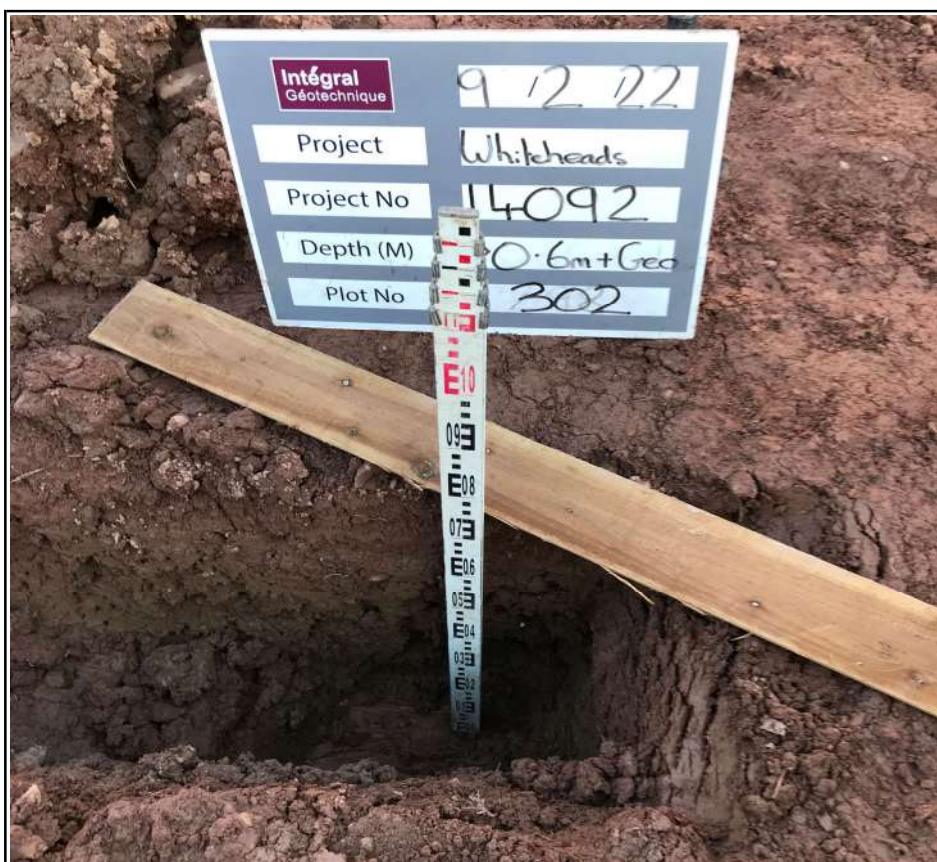
Plot 302 Trail Pit Excavation
