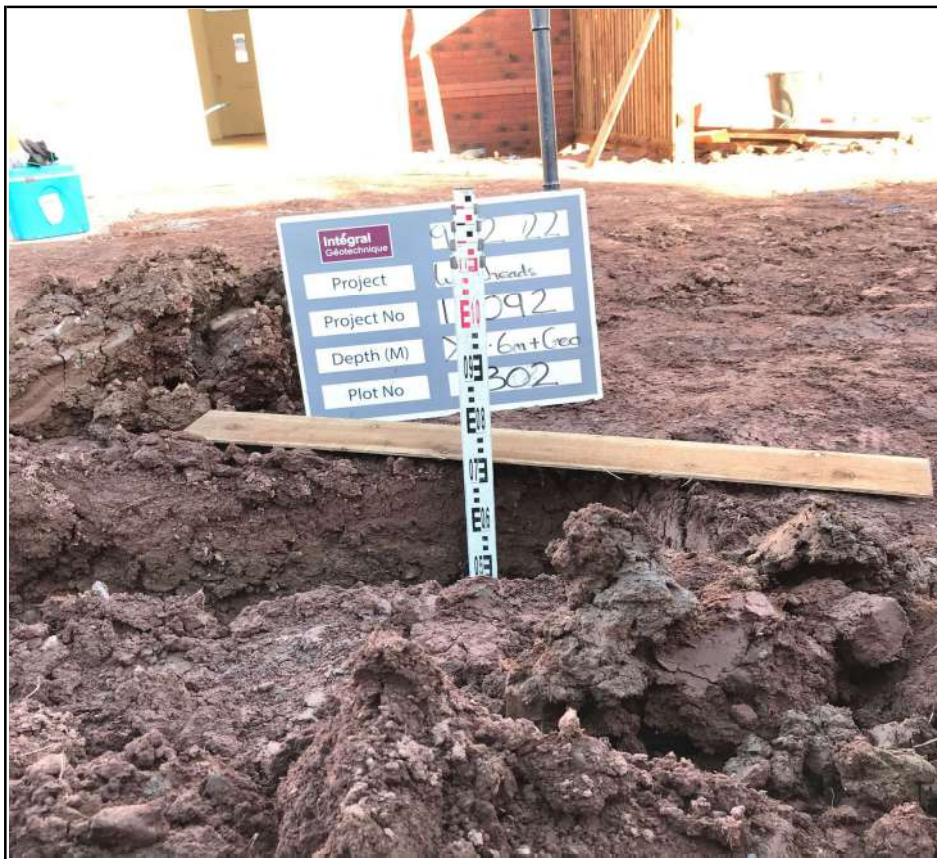
Plot 302 Capping Depth Check
