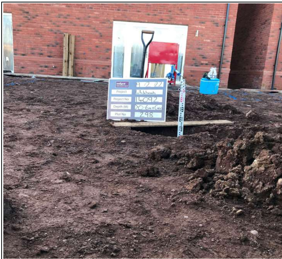
Plot 298 Capping Depth Check
