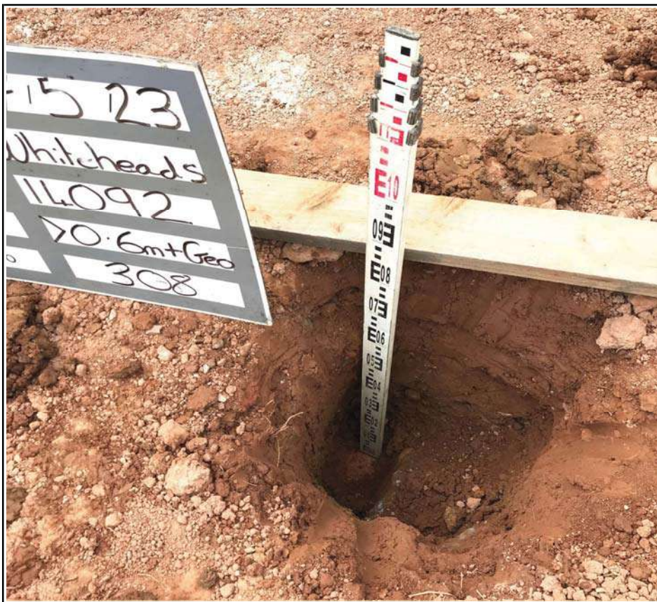
Plot 308 Excavation Trial Pit Showing Membrane Placement
