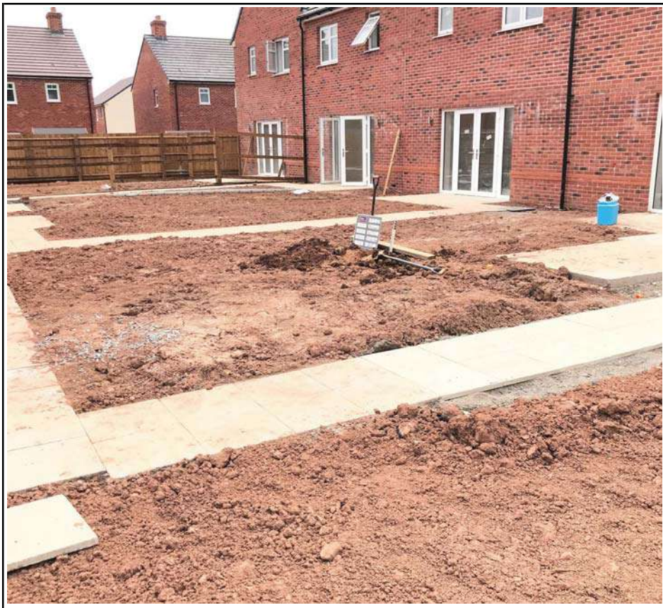
Plots 305 to 308 Showing Infilled Rear Garden
