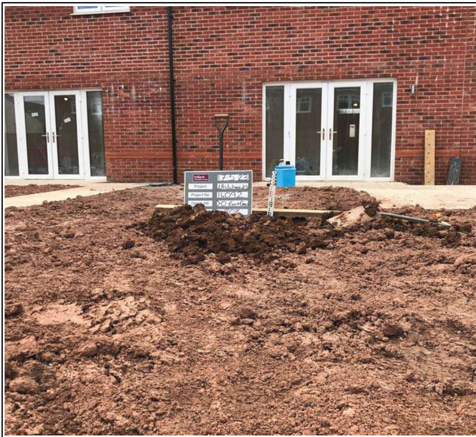
Plot 308 Capping Depth Check
