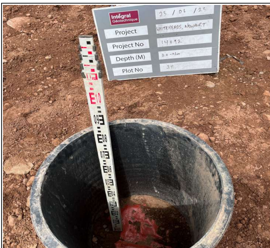
Plot 311 Trial Pit Excavation and Membrane Check
