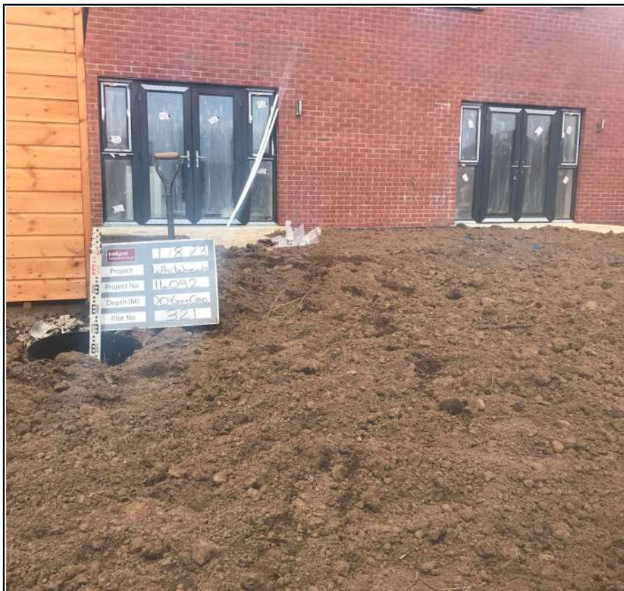
Plot 321 Capping Depth Check
