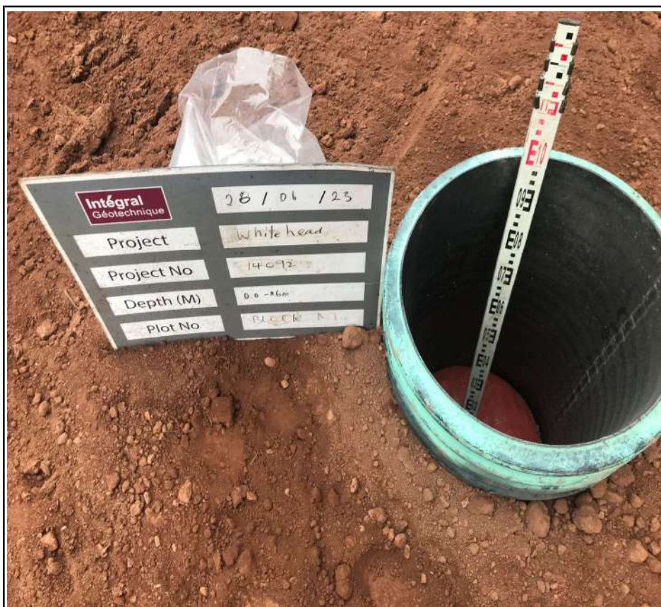
Block M Plots 324 to 347 Trial Pit Excavation
