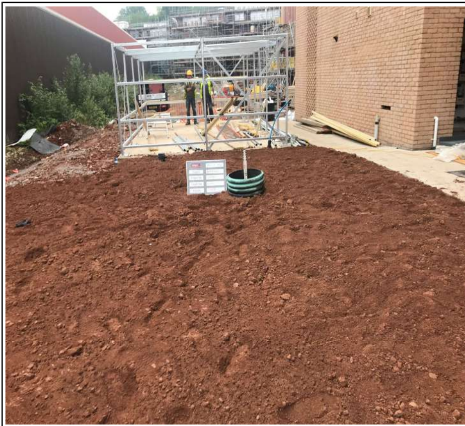
Block M Plots 324 to 347 Capping Depth Check
