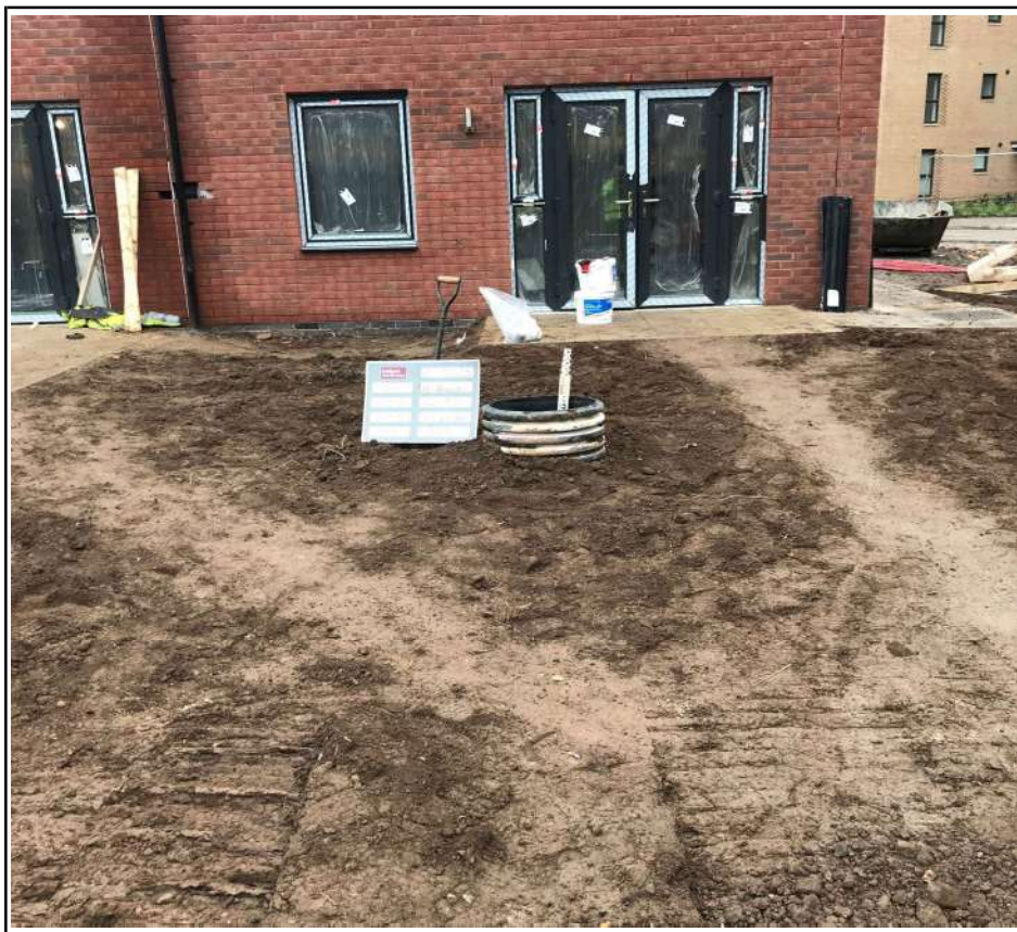
Plot 349 Capping Depth Check
