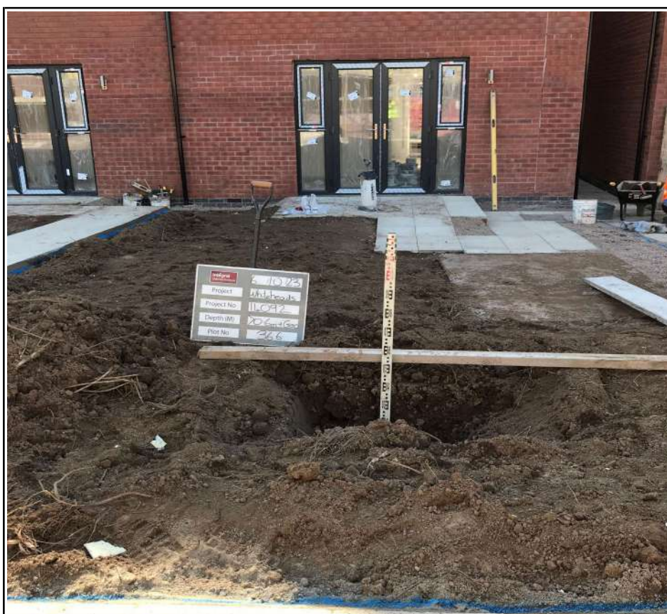
Plot 366 Capping Depth Check
