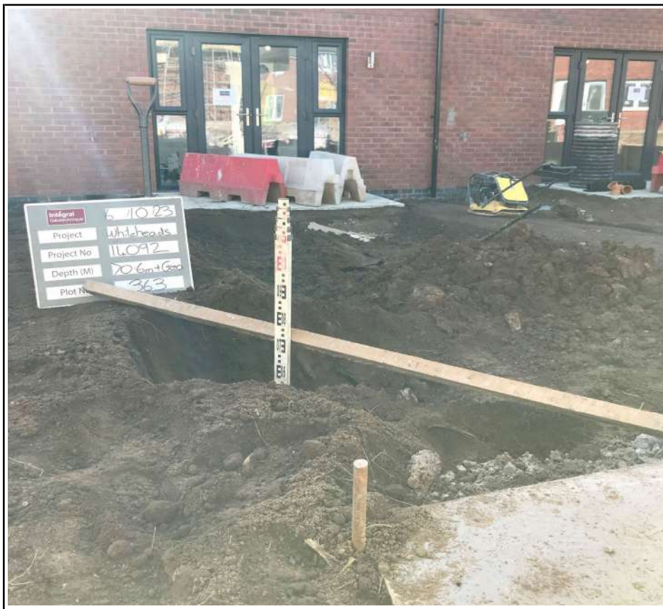
Plot 363 Capping Depth Check
