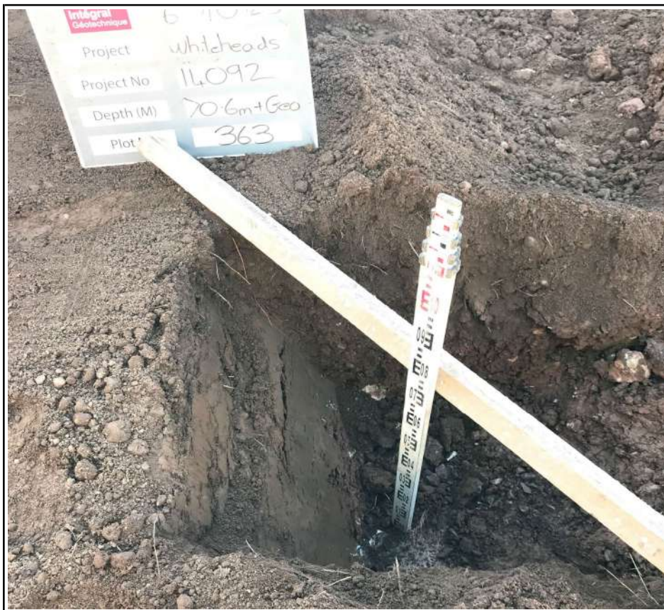
Plot 363 Trial Pit Excavation
