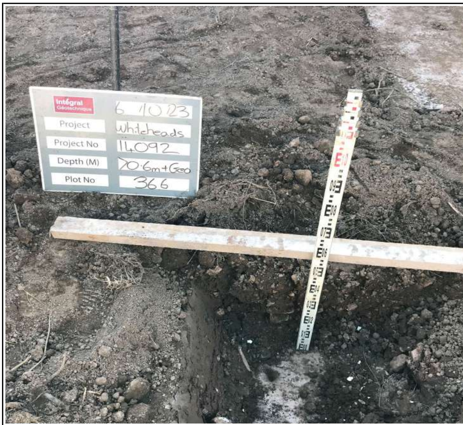
Plot 366 Trial Pit Excavation
