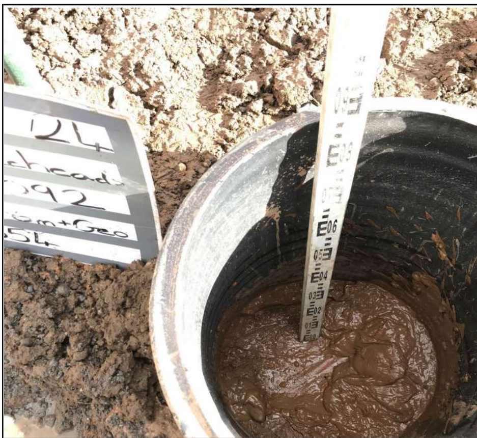
Plot 154 Membrane Placement
