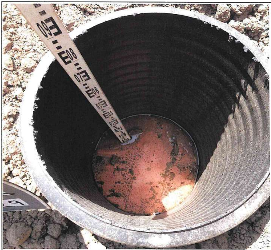
Plot 422 to 429 Membrane Placement
