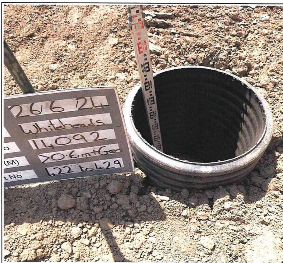
Plot 422 to 429 Excavation Trial Pit
