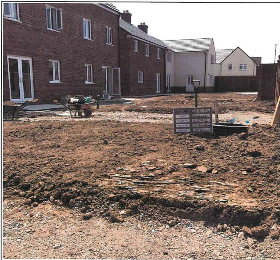
Plot 422 to 429 Capping Deph Check
