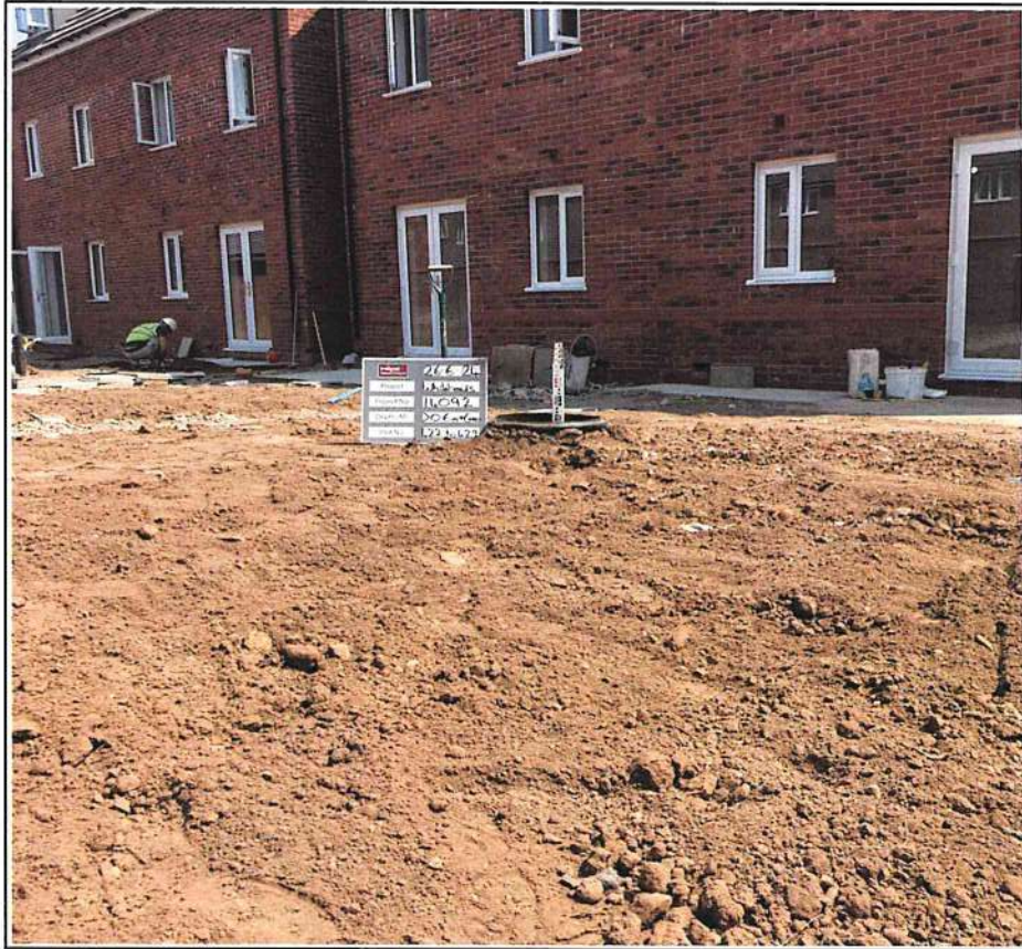
Plot 422 to 429 Capping Deph Check
