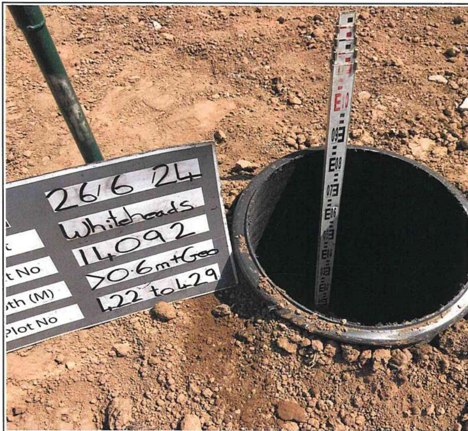
Plot 422 to 429 Excavation Trial Pit
