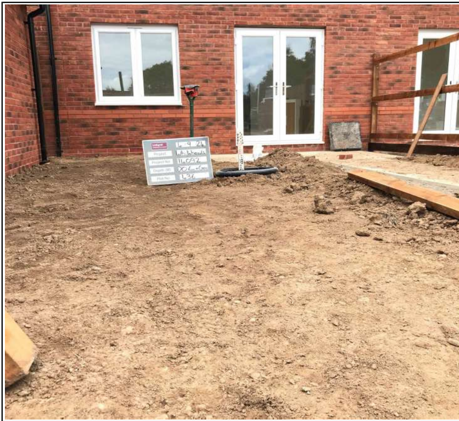
Plot 436 Capping Depth Check
