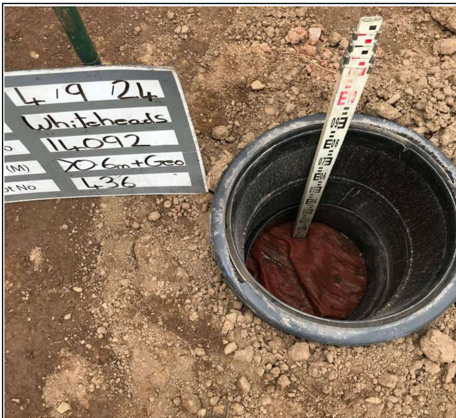
Plot 436 Membrane Placement
