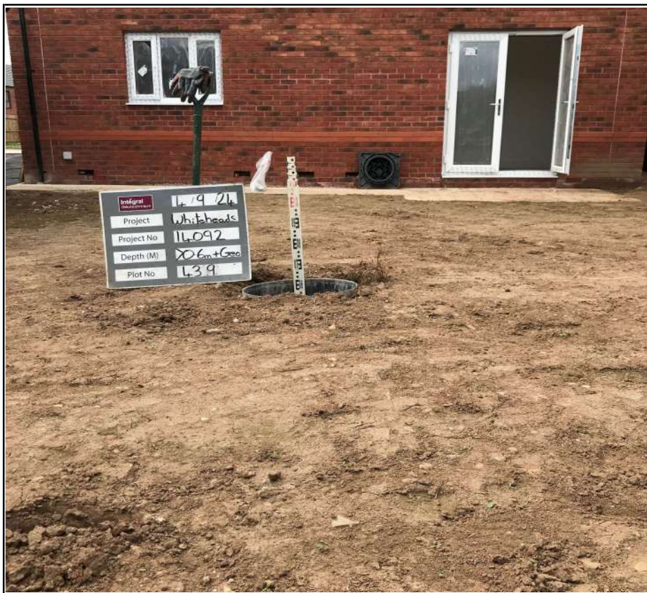
Plot 439 Capping Depth Check
