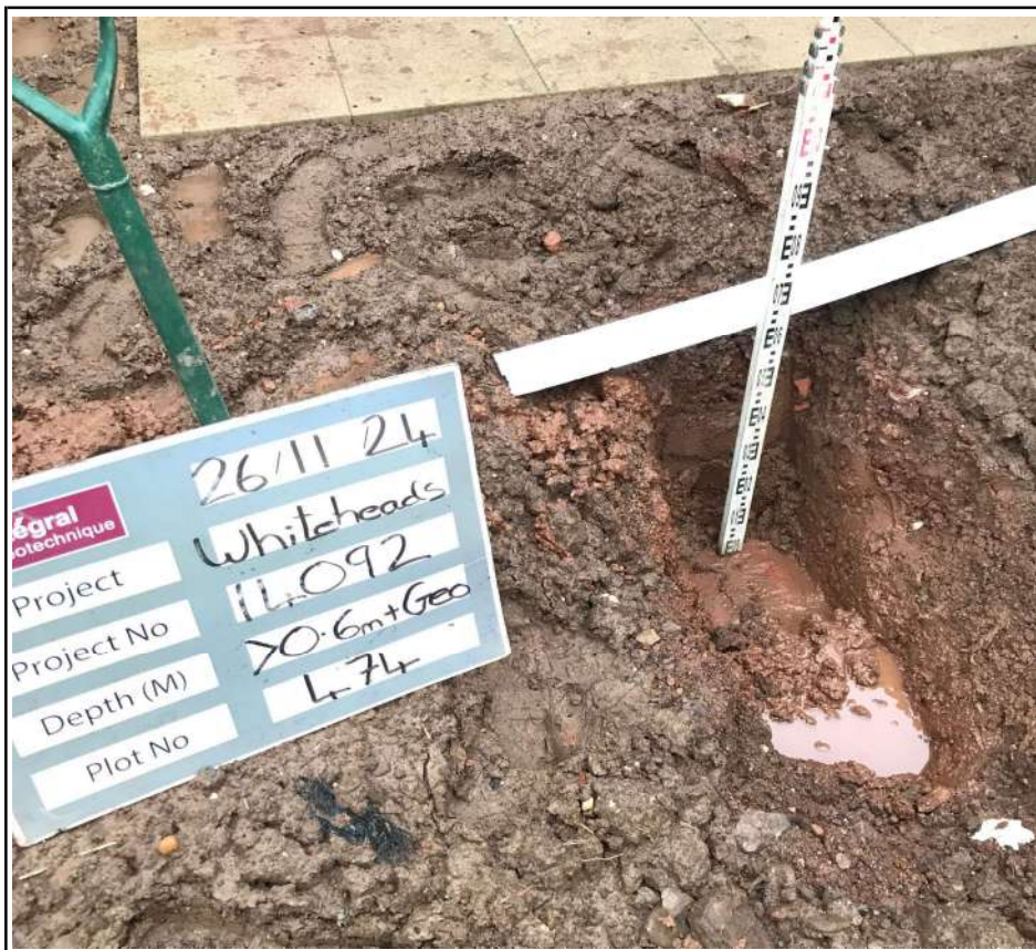
Plot 474 Capping Depth Check
