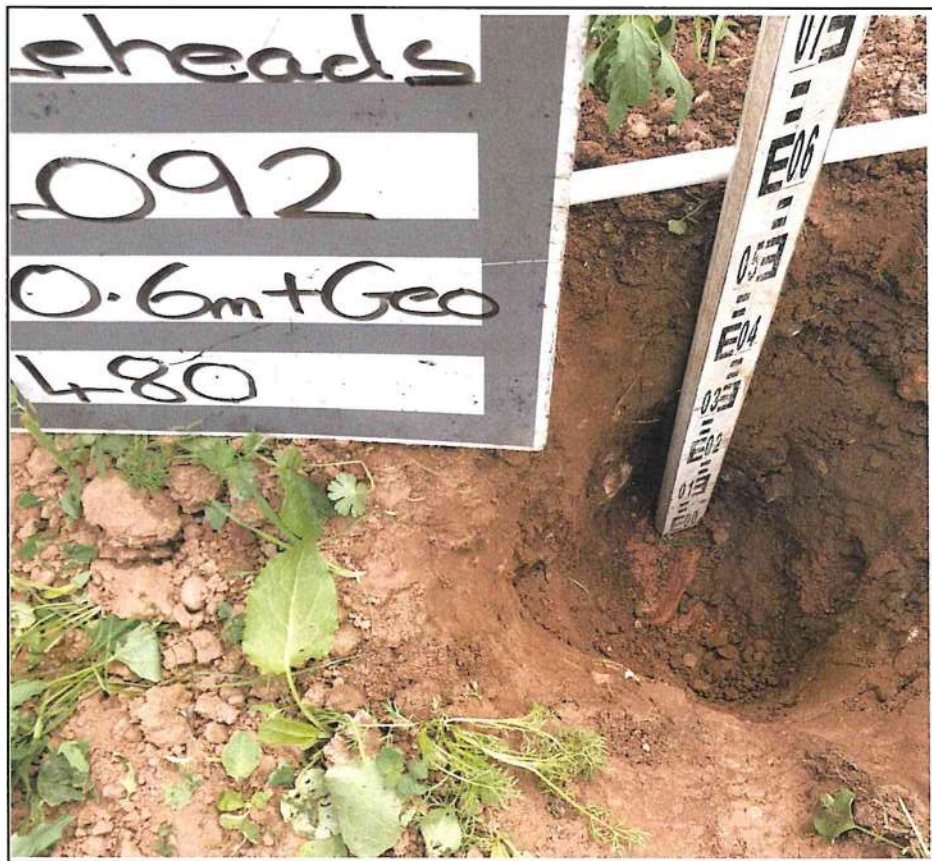
Plot 480 Membrane at Base of Capping Soils
