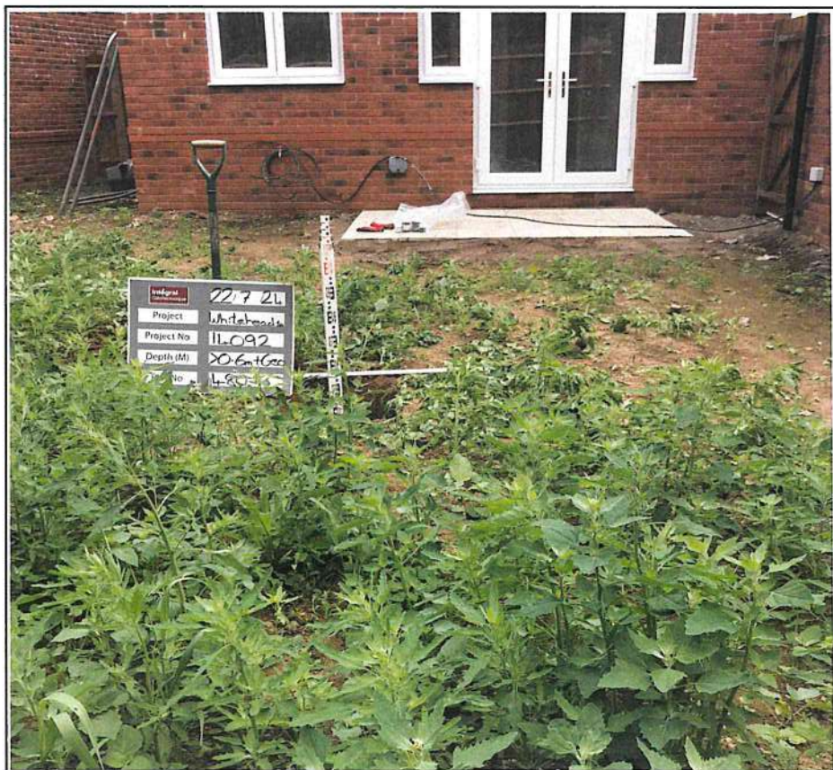
Plot 480 Capping Deph Check
