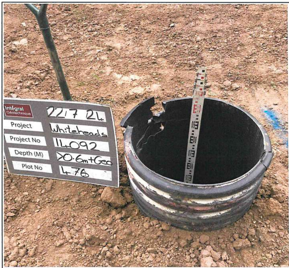
Plot 476 Capping Deph Check
