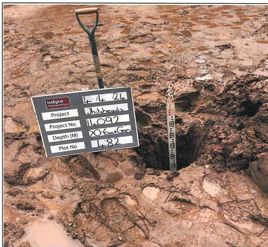
Plot 482 Trial Pit Excavation
