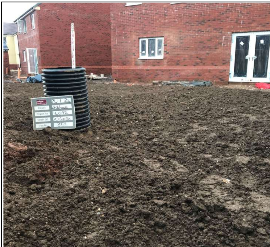
Plot 359 Capping Depth Check
