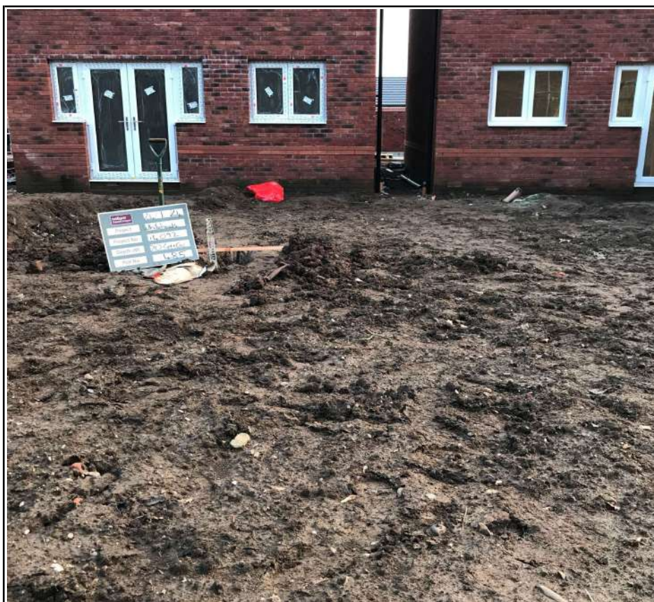
Plot 485 Capping depth check
