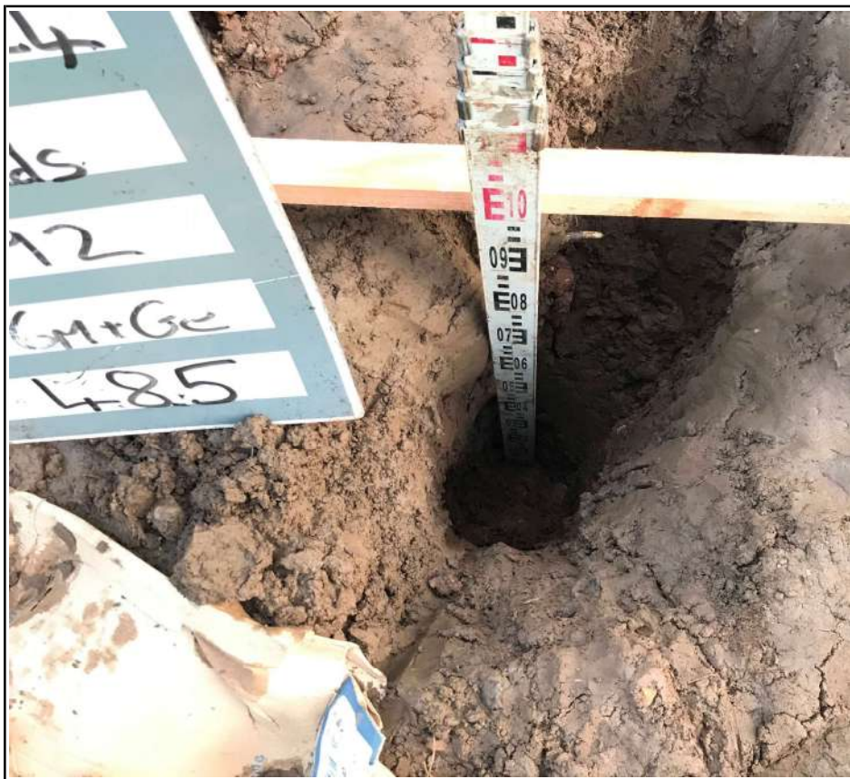
Plot 485 Excavation Trial Pit
