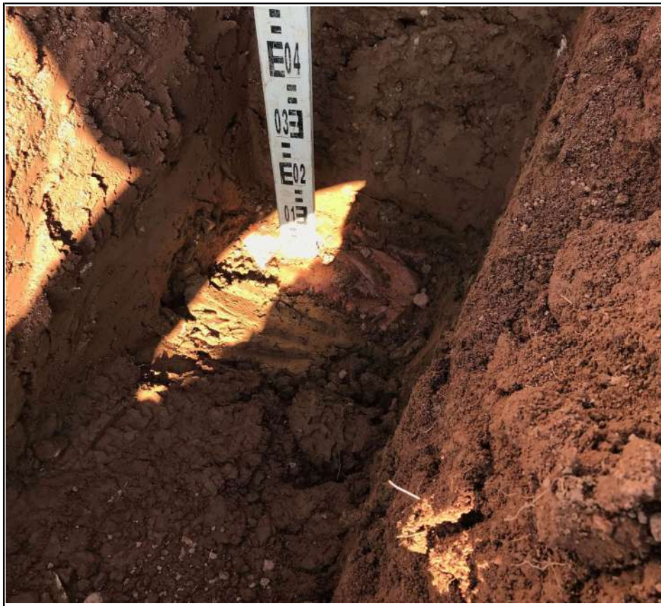
Block F (Plots 87 to 95) Membrane Placement
