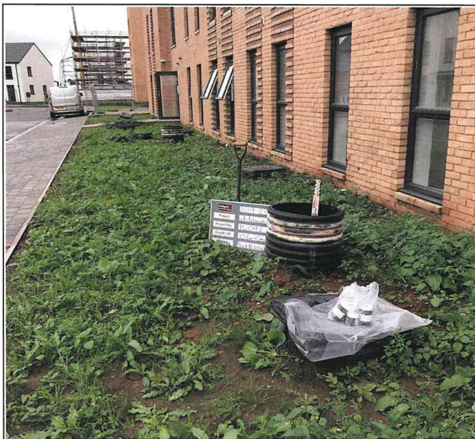
Block N Capping Layer Depth Check Point A
