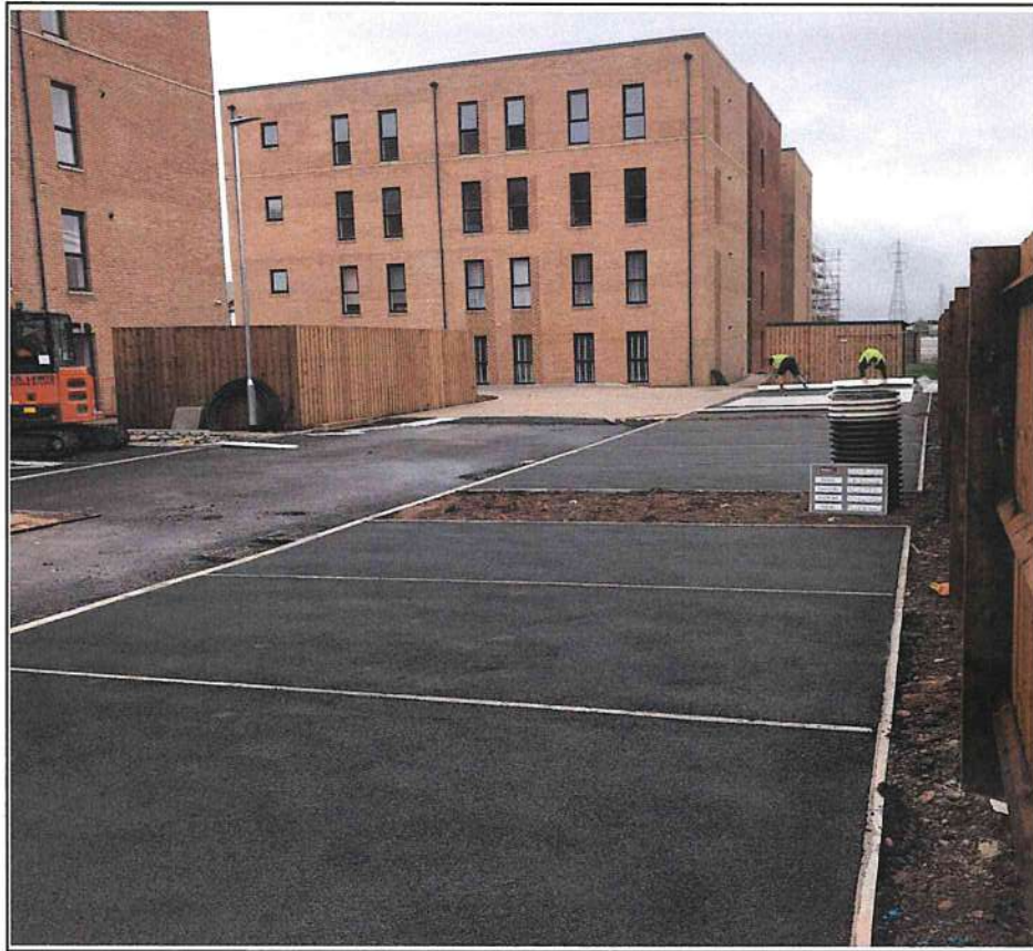
Block N Rear Carpark Area
