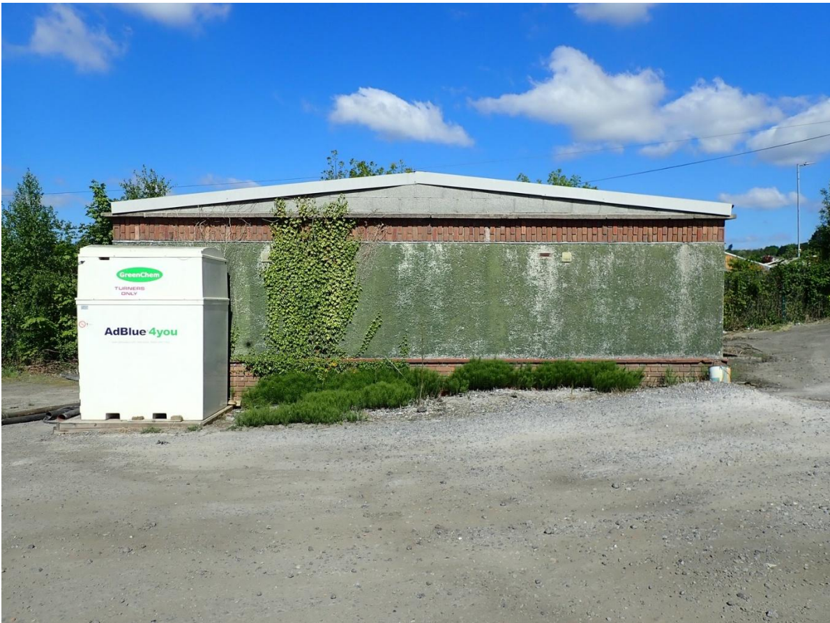
Building proposed to be demolished.
