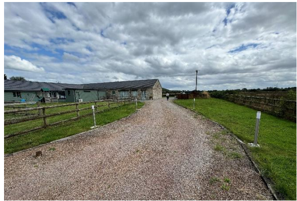
Figure 2 – Private drive leading up to the property from Bishton rd.
