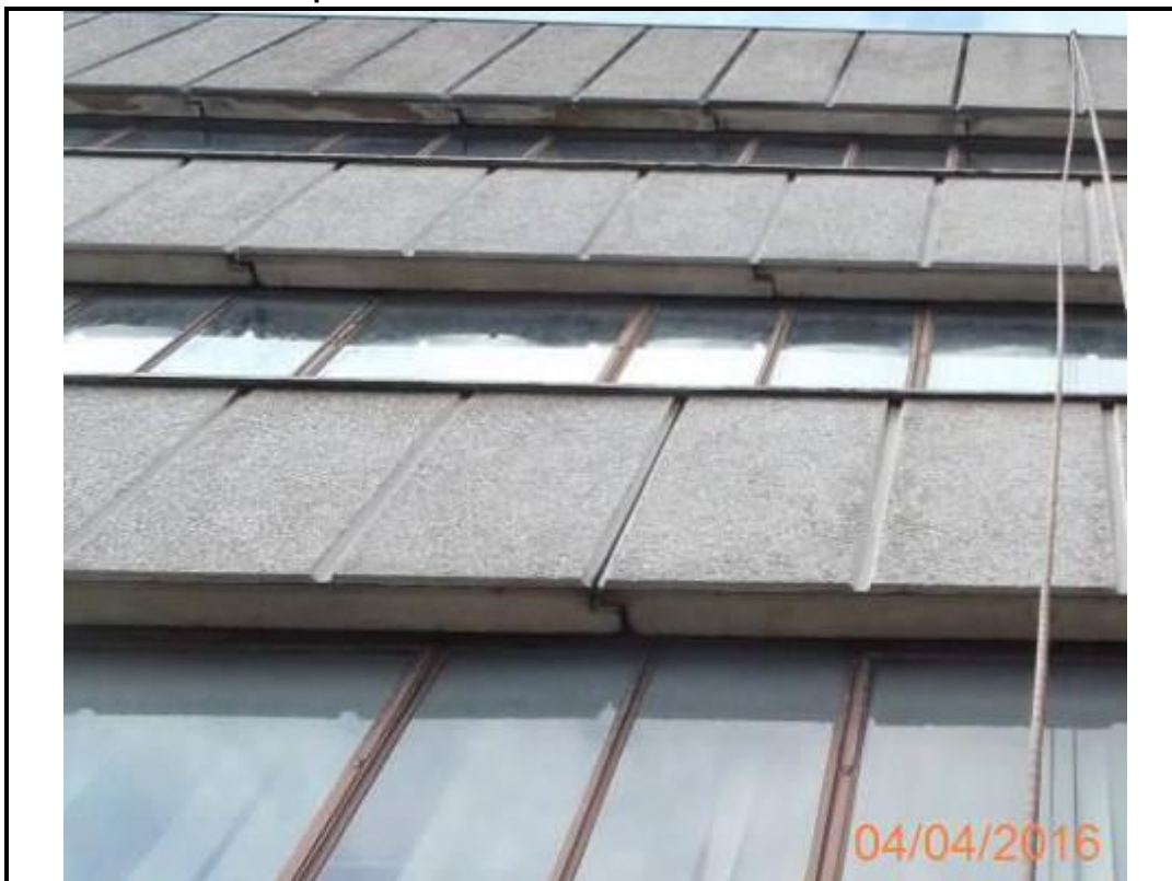
Photo 76. Drop 4 – South Elevation
