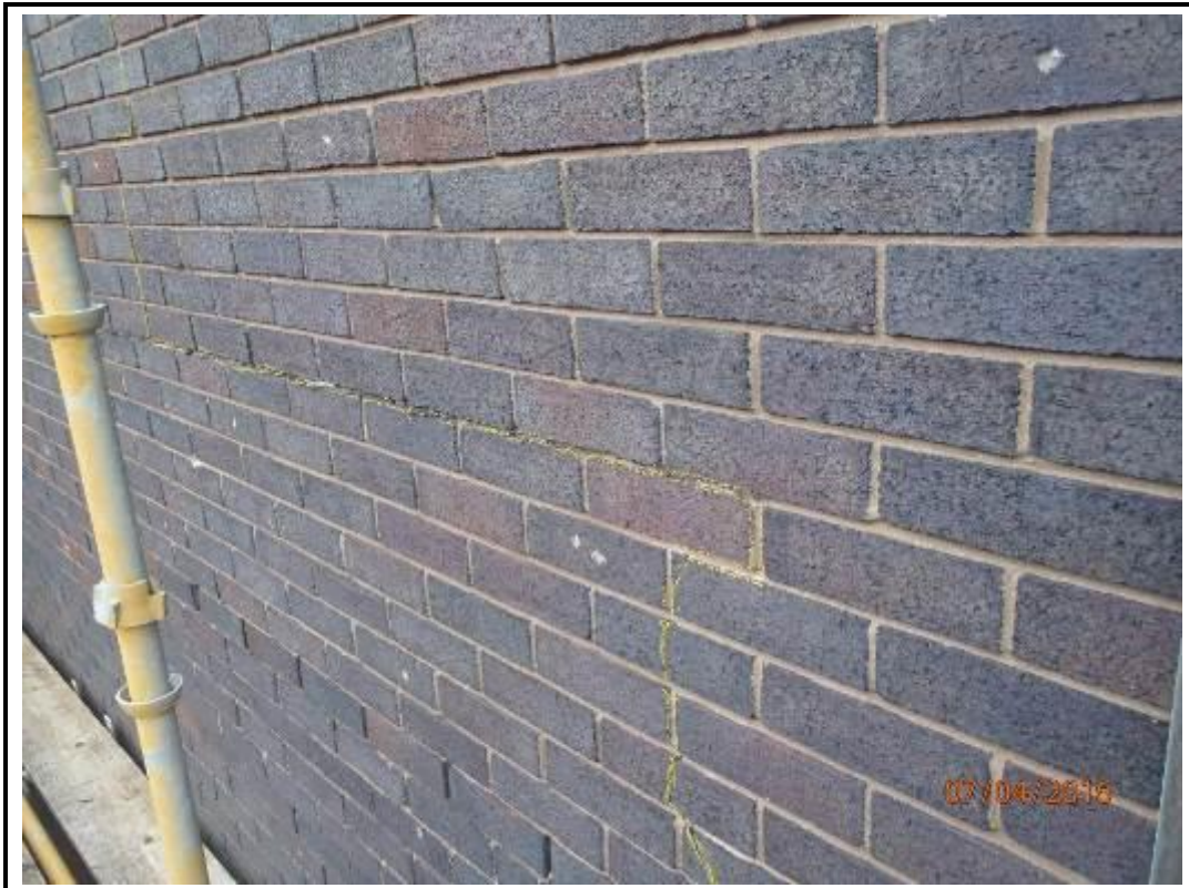
Photo 214. Drop 11 – West Elevation
