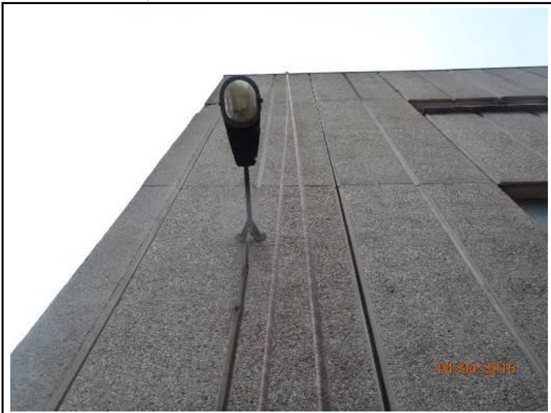
Photo 46. Drop 13 – East Elevation
