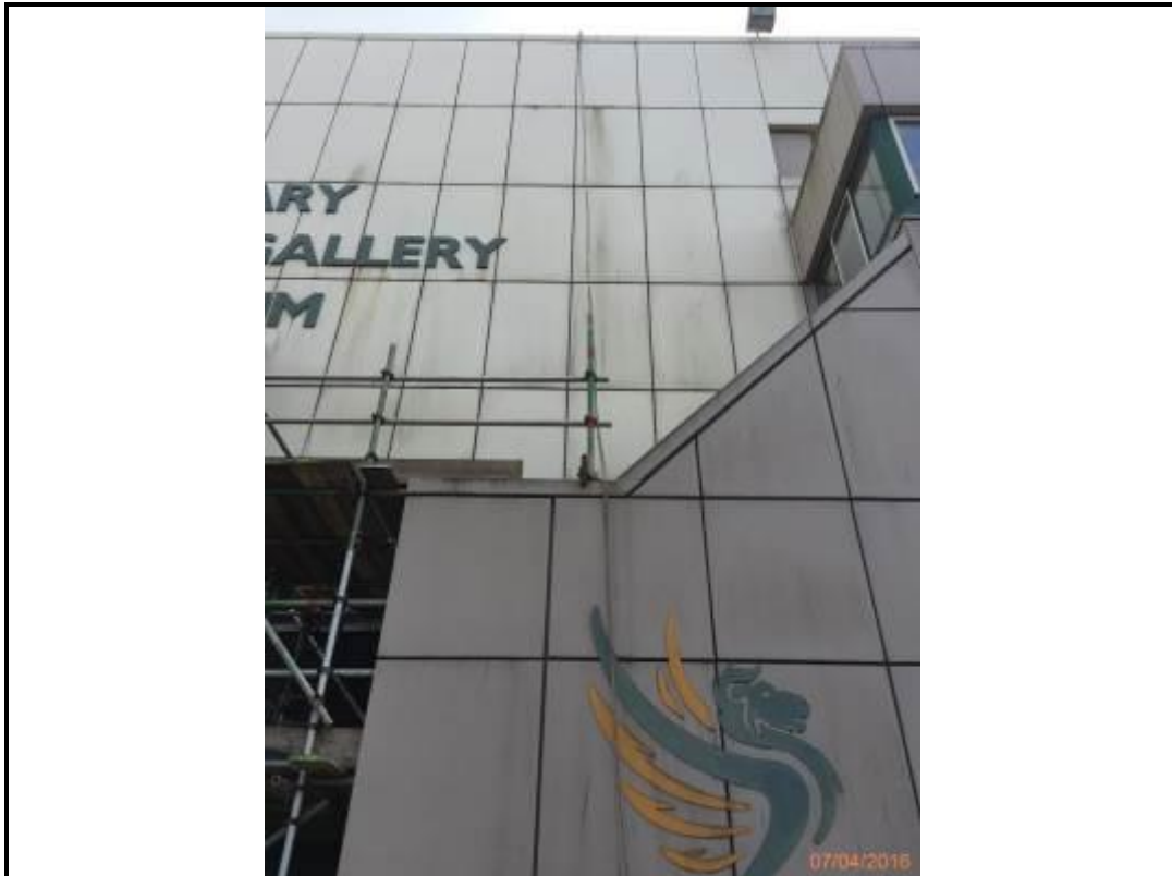
Photo 259. Drop 11 – North Elevation
