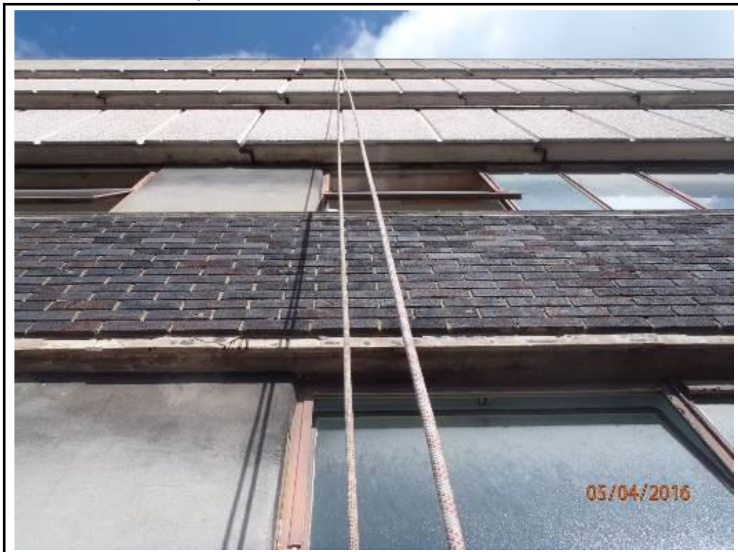
Photo 88. Drop 7 – South Elevation
