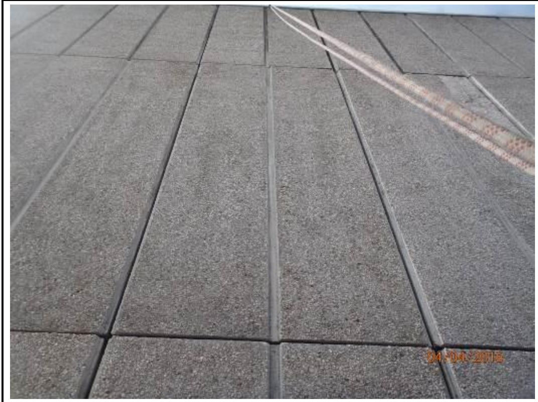
Photo 15. Drop 3 – East Elevation
