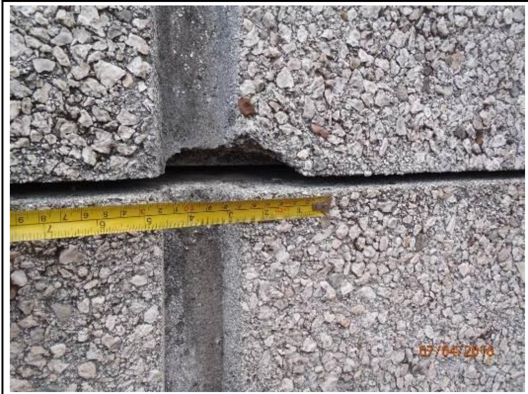
Photo 217. Drop 12 – West Elevation
