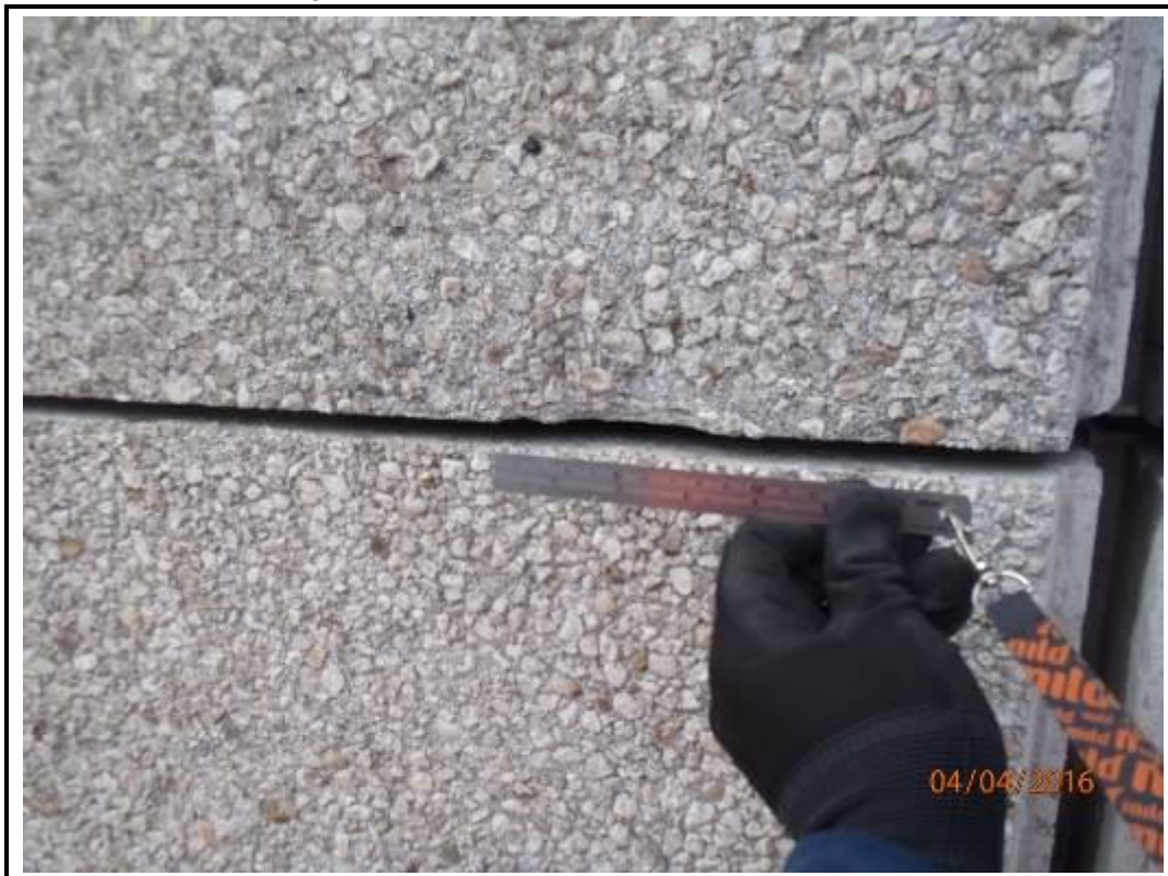
Photo 14. Drop 3 – East Elevation
