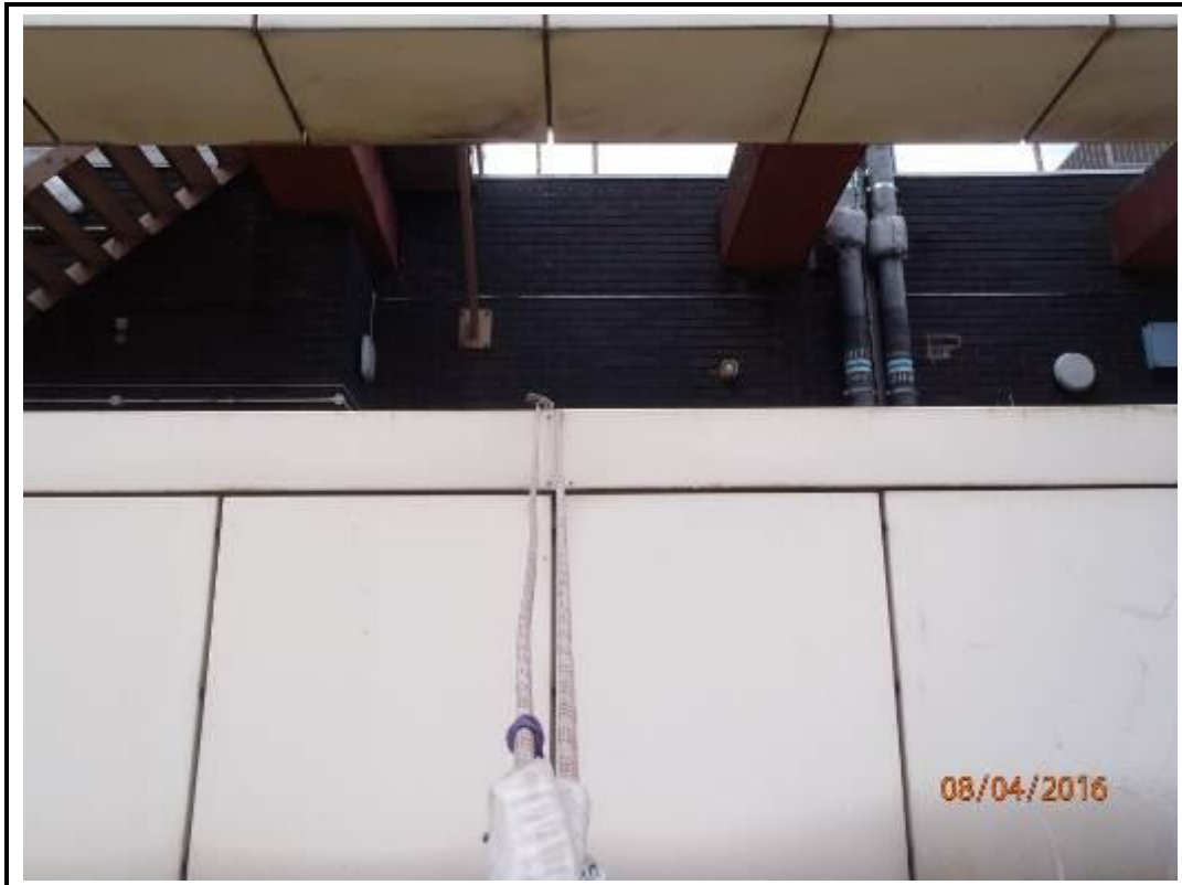
Photo 249. Drop 7 – North Elevation
