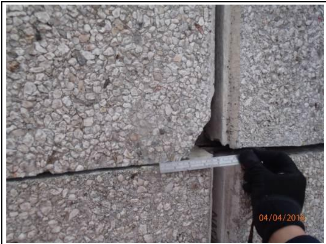
Photo 38. Drop 12 – East Elevation
