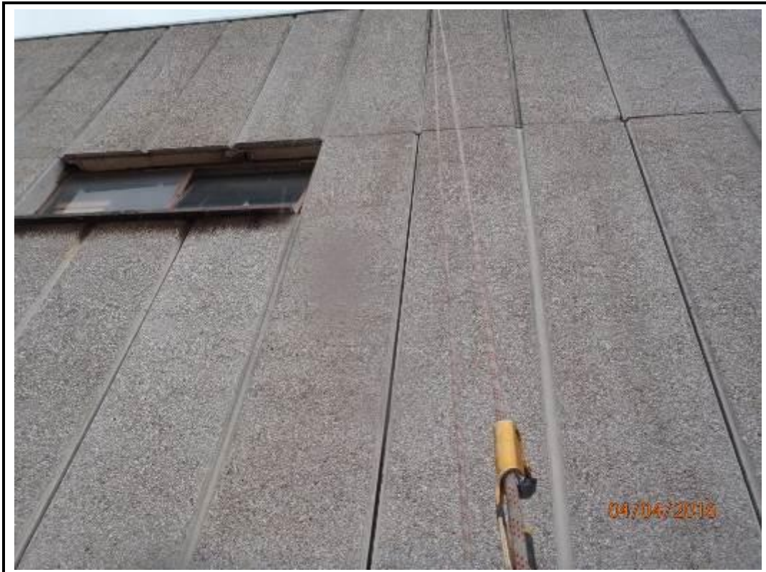
Photo 36. Drop 11 – East Elevation
