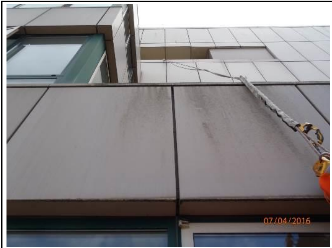
Photo 237. Drop 4 – North Elevation
