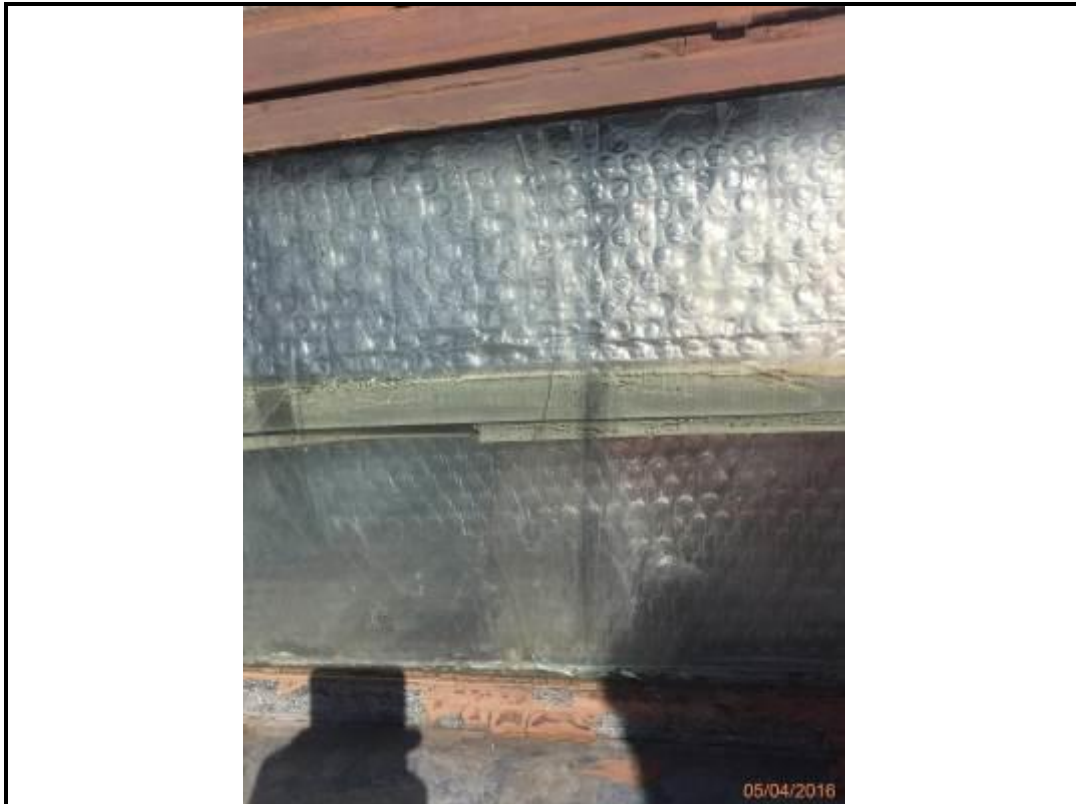
Photo 61. Drop 2 – South Elevation
