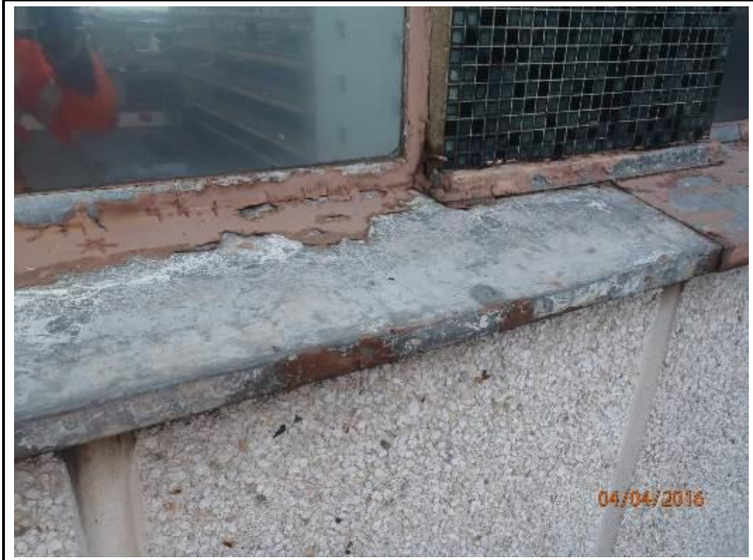
Photo 71. Drop 3 – South Elevation
