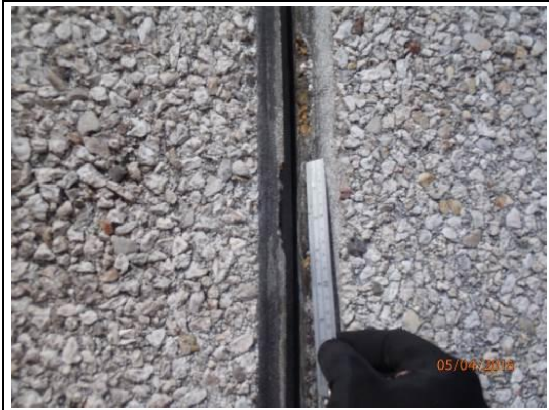
Photo 99. Drop 10 – South Elevation
