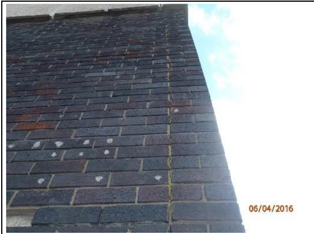
Photo 169. Drop 1 – West Elevation
