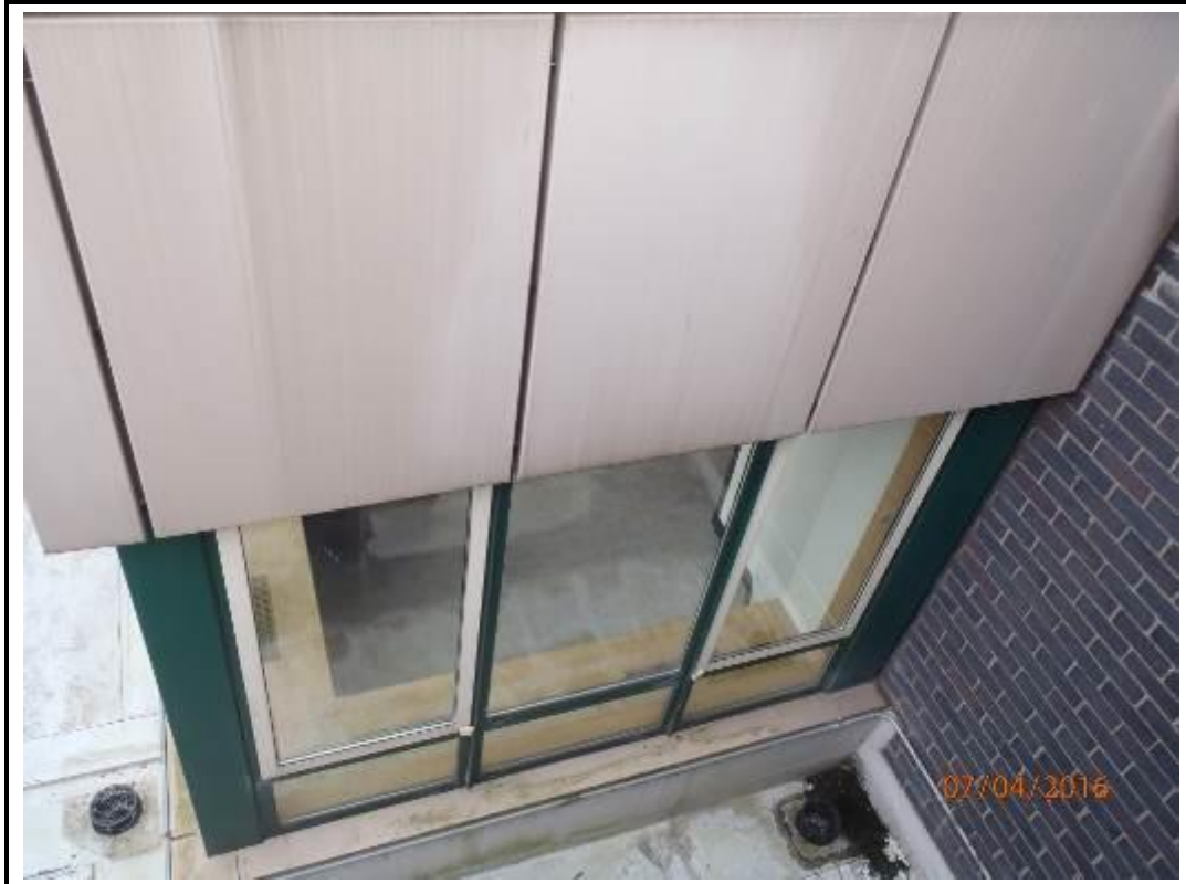
Photo 231. Drop 1 – North Elevation
