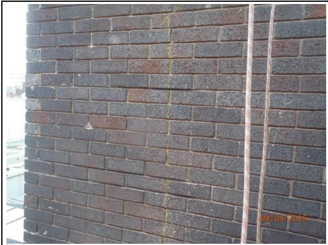
Photo 47. Drop 13 – East Elevation
