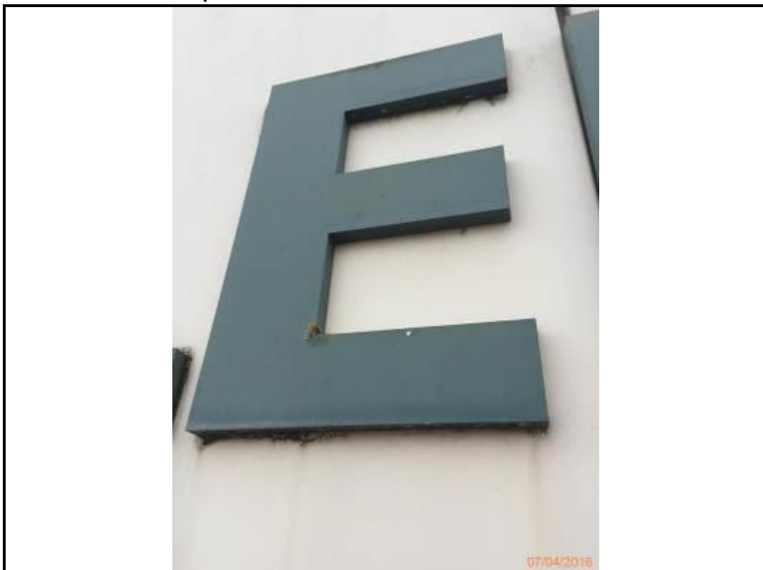
Photo 262. Drop 12 – North Elevation
