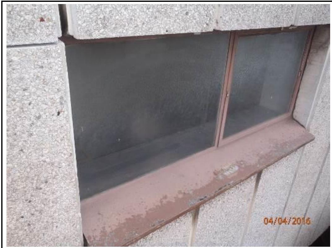
Photo 39. Drop 12 – East Elevation
