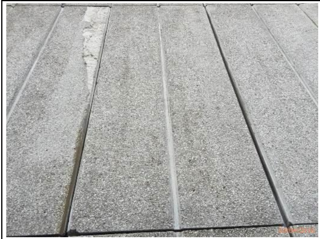
Photo 11. Drop 2 – East Elevation
