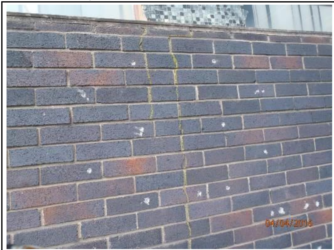
Photo 74. Drop 3 – South Elevation
