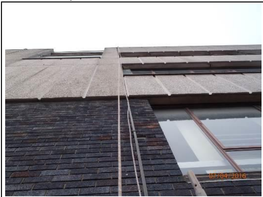
Photo 216. Drop 11 – West Elevation
