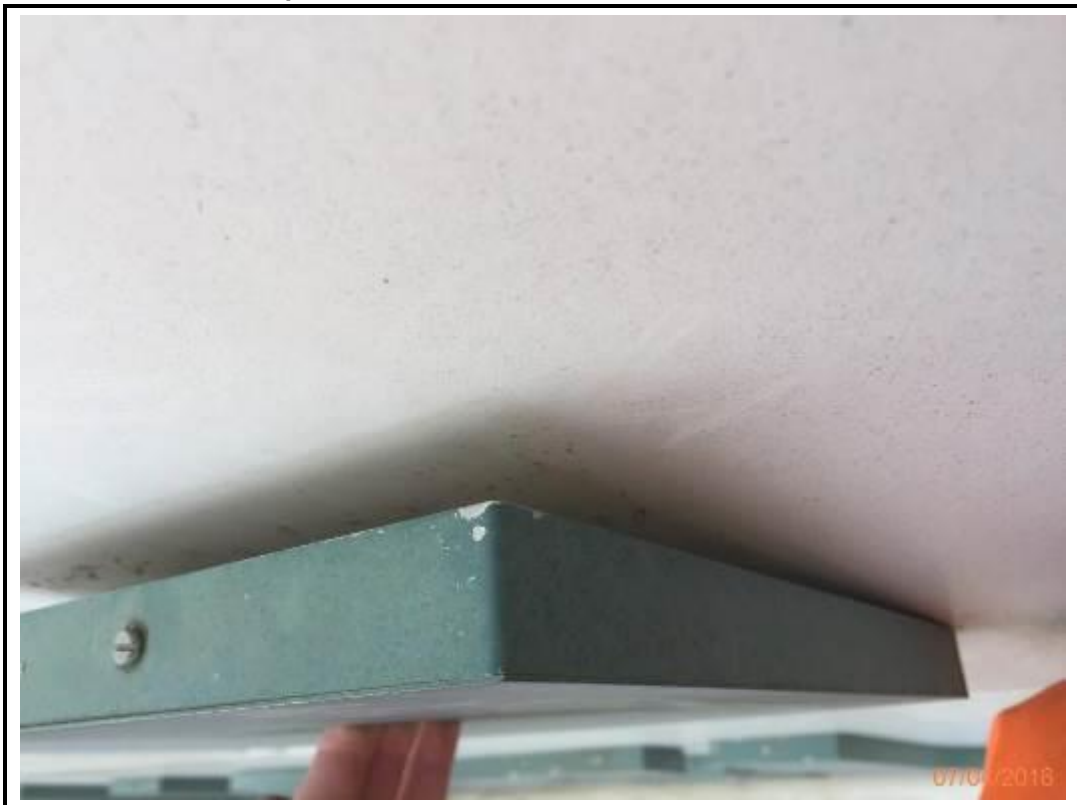
Photo 266. Drop 13 – North Elevation
