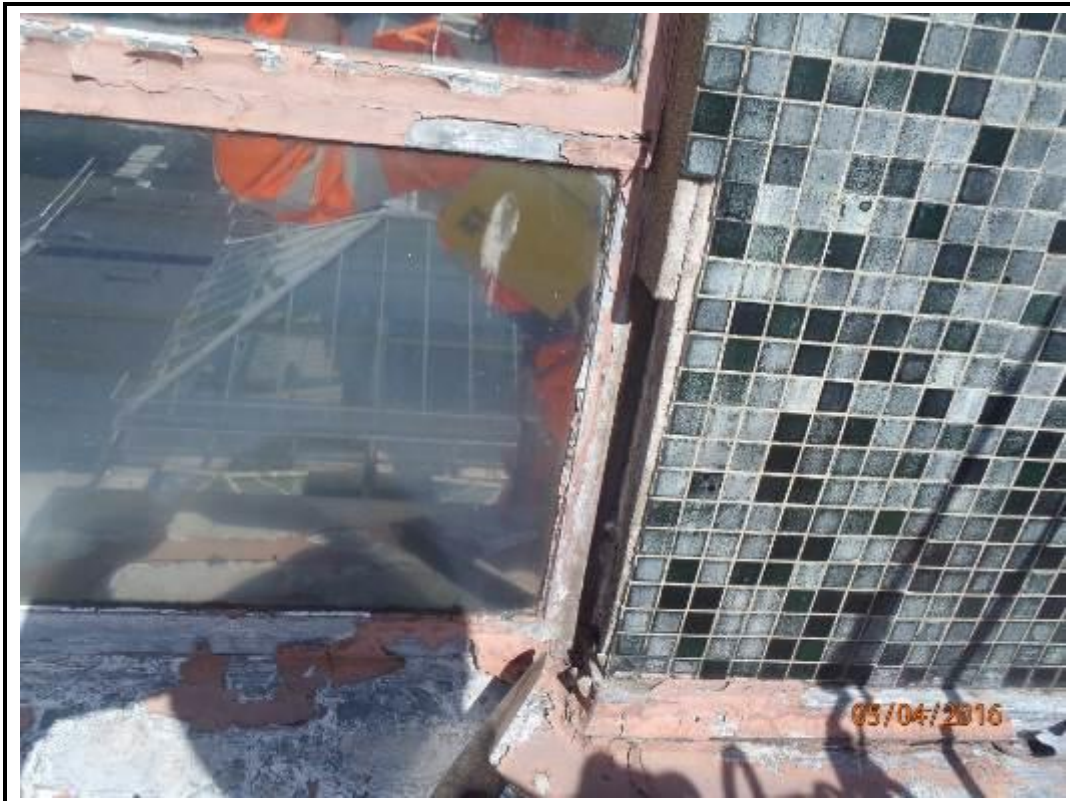
Photo 84. Drop 7 – South Elevation
