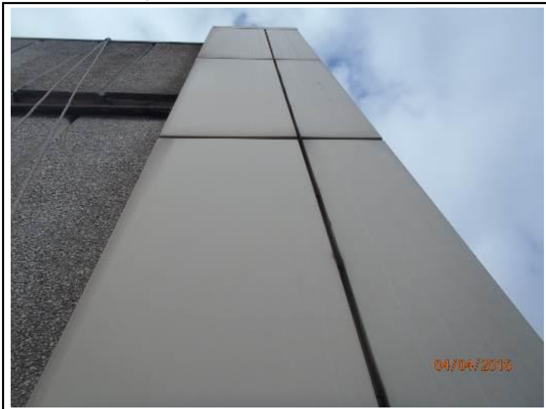
Photo 6. Drop 1 – East Elevation
