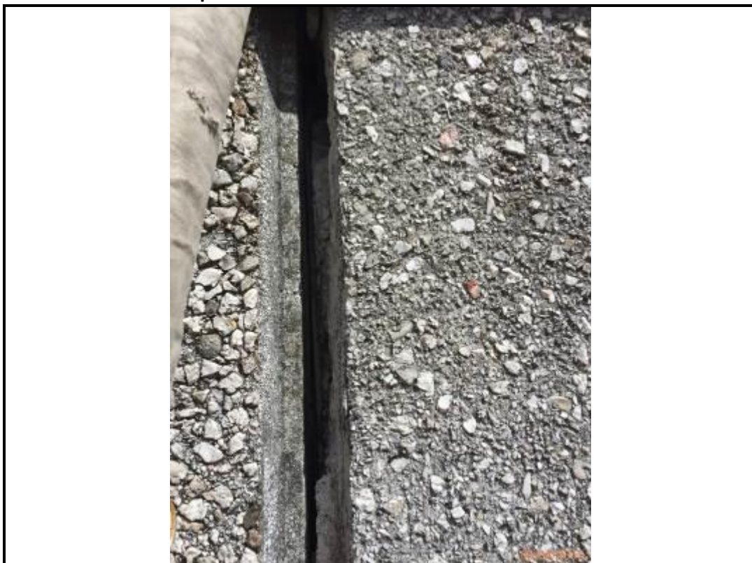
Photo 200. Drop 8 – West Elevation
