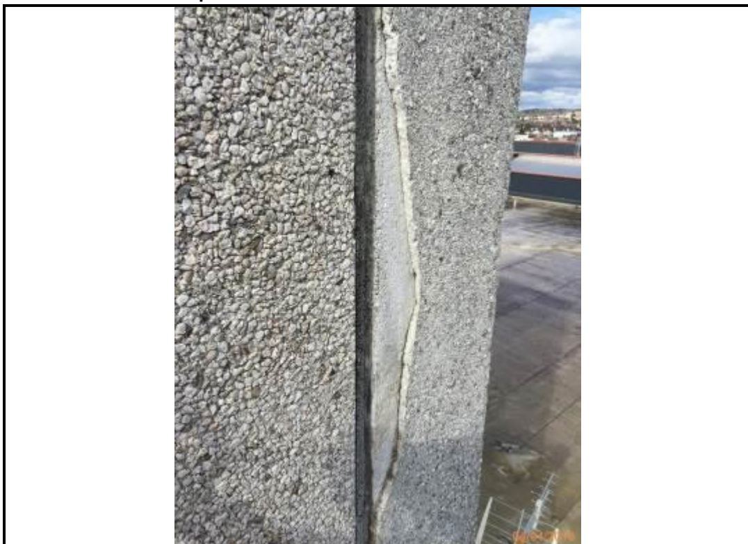
Photo 50. Drop 1 – South Elevation
