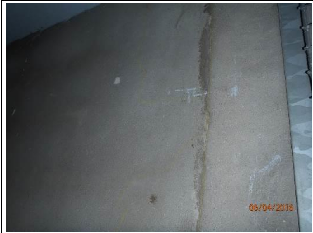
Photo 161. East Elevation – Brickwork Cladding Beneath Overhang
