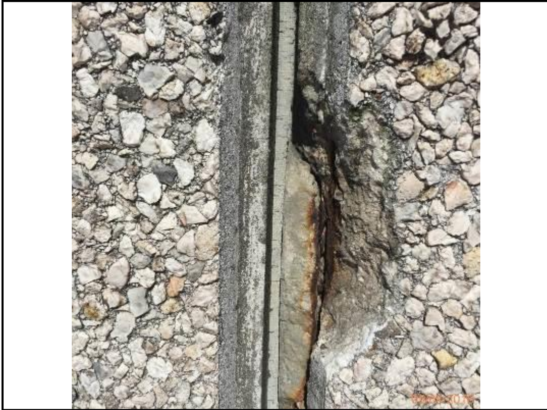
Photo 77. Drop 5 – South Elevation
