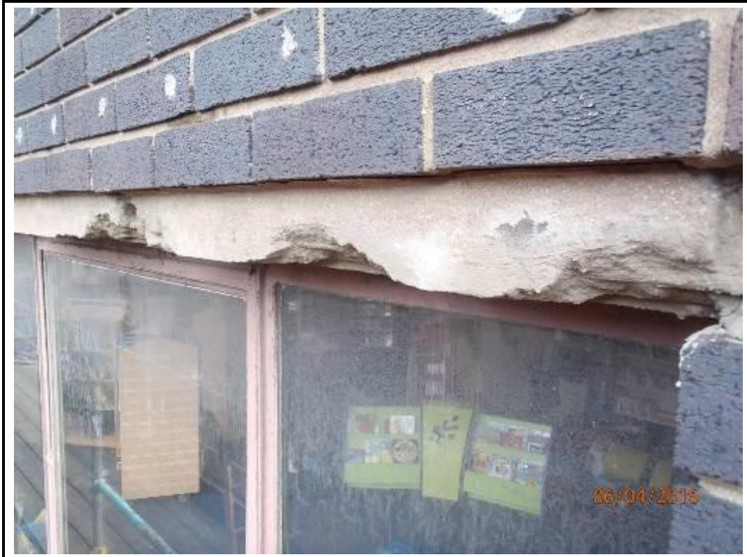
Photo 181. Drop 3 – West Elevation
