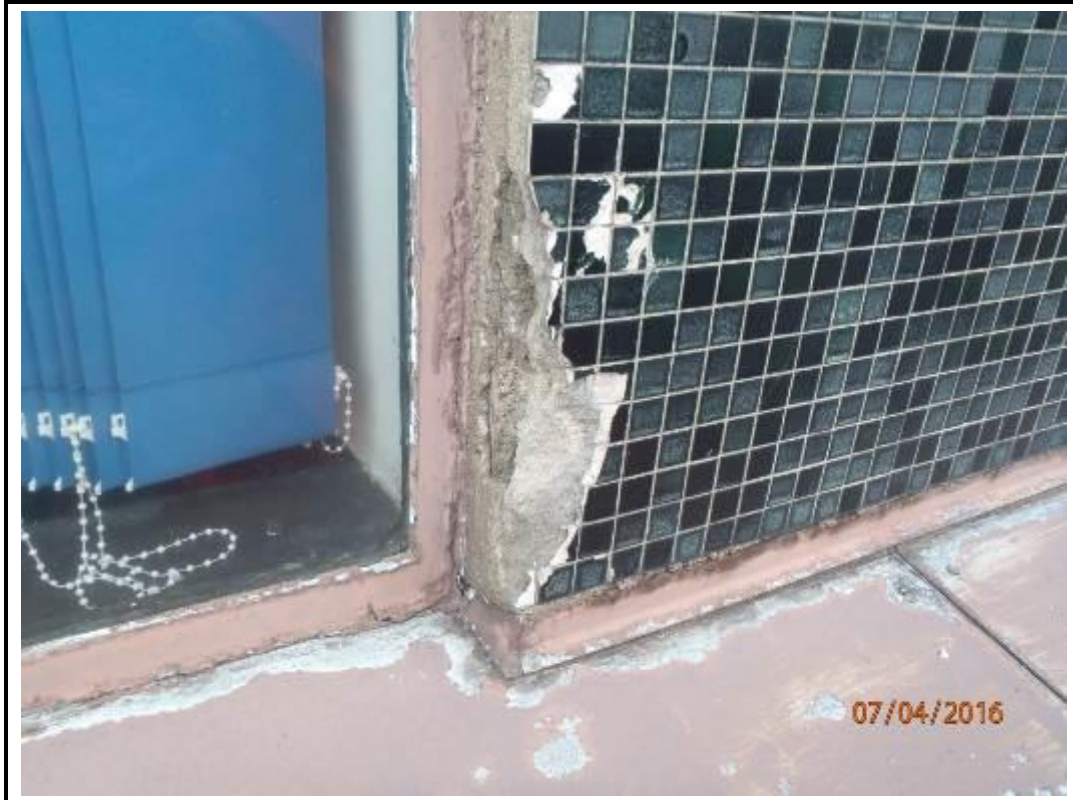
Photo 203. Drop 9 – West Elevation
