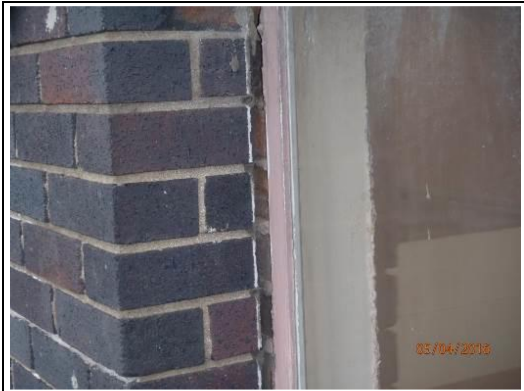
Photo 132. Drop 14 – South Elevation
