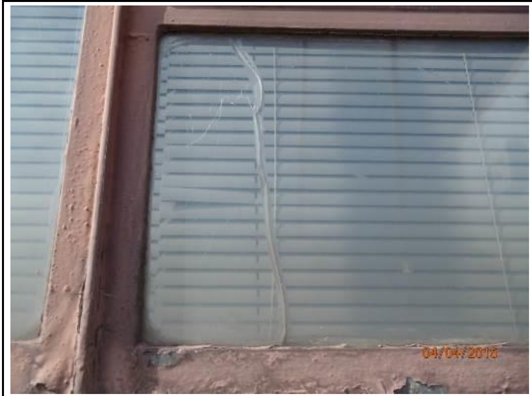
Photo 73. Drop 3 – South Elevation
