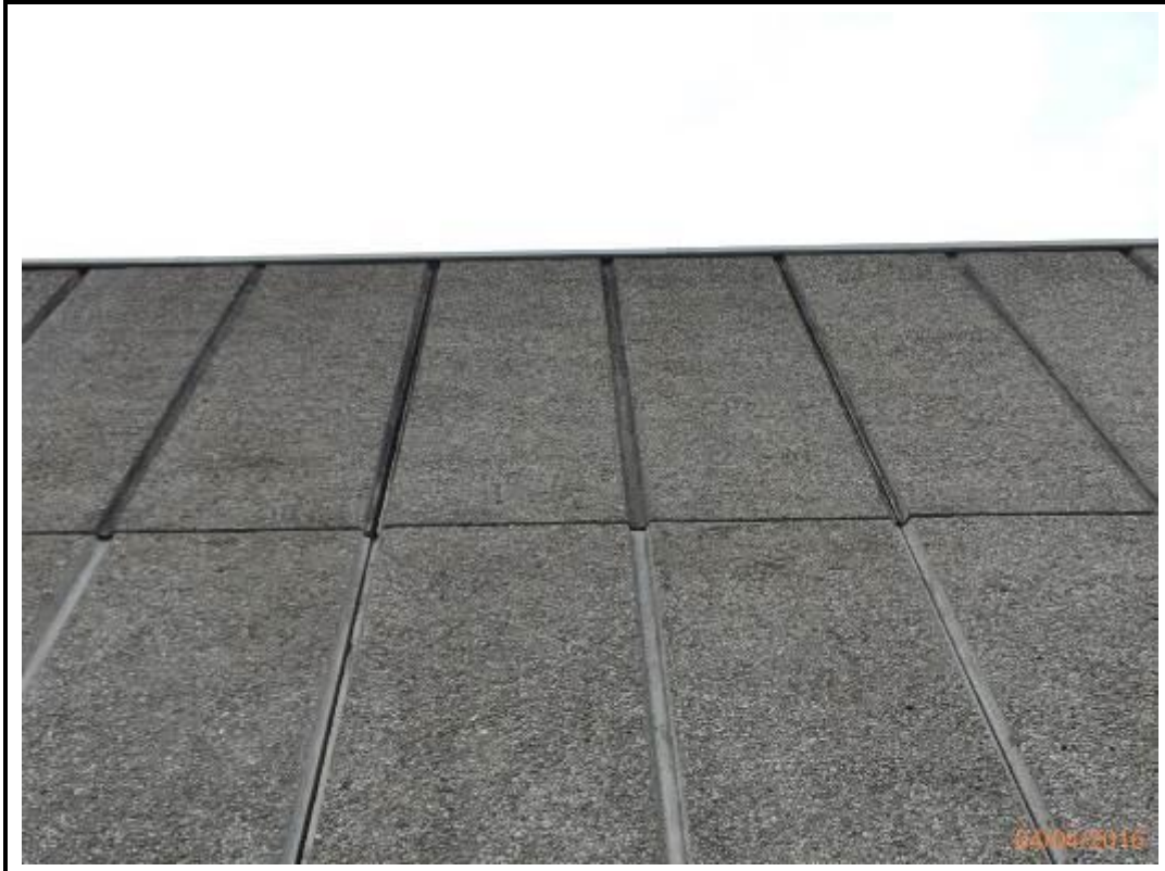
Photo 17. Drop 4 – East Elevation
