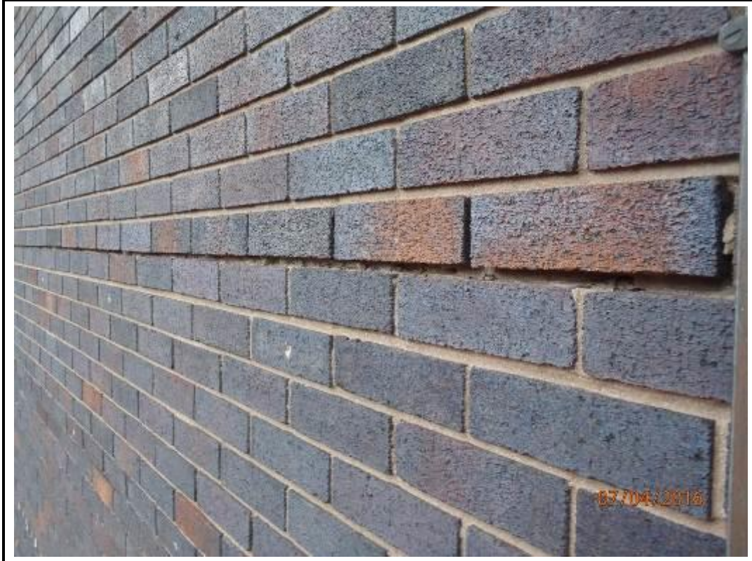
Photo 209. Drop 11 – West Elevation
