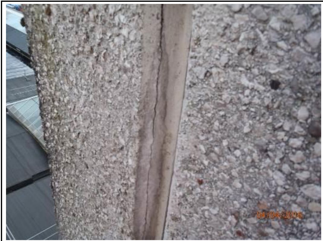
Photo 44. Drop 13 – East Elevation
