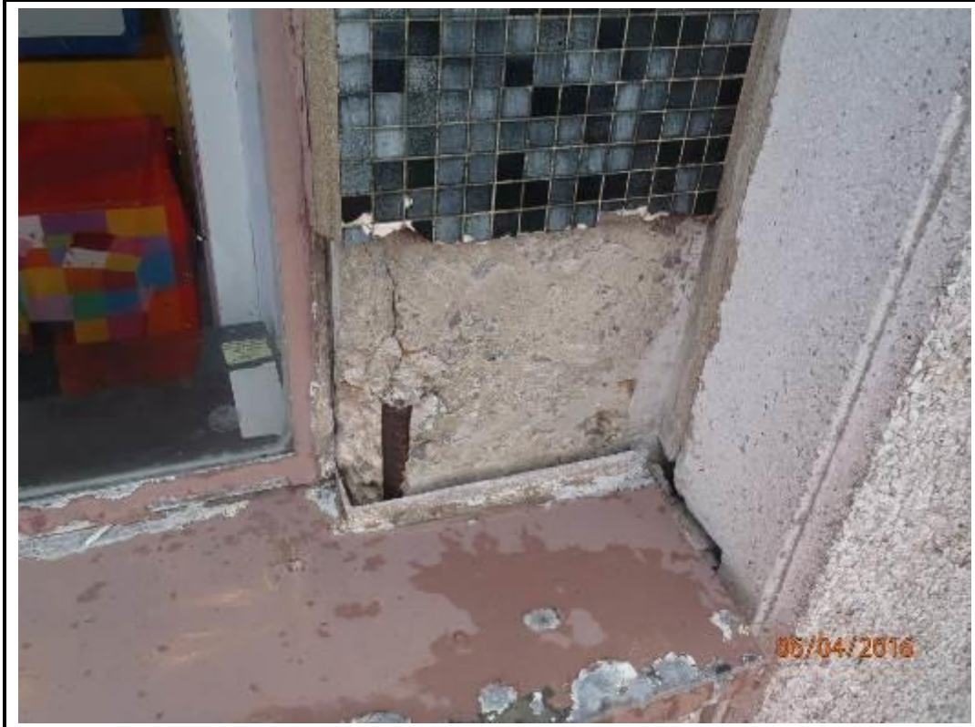
Photo 179. Drop 3 – West Elevation
