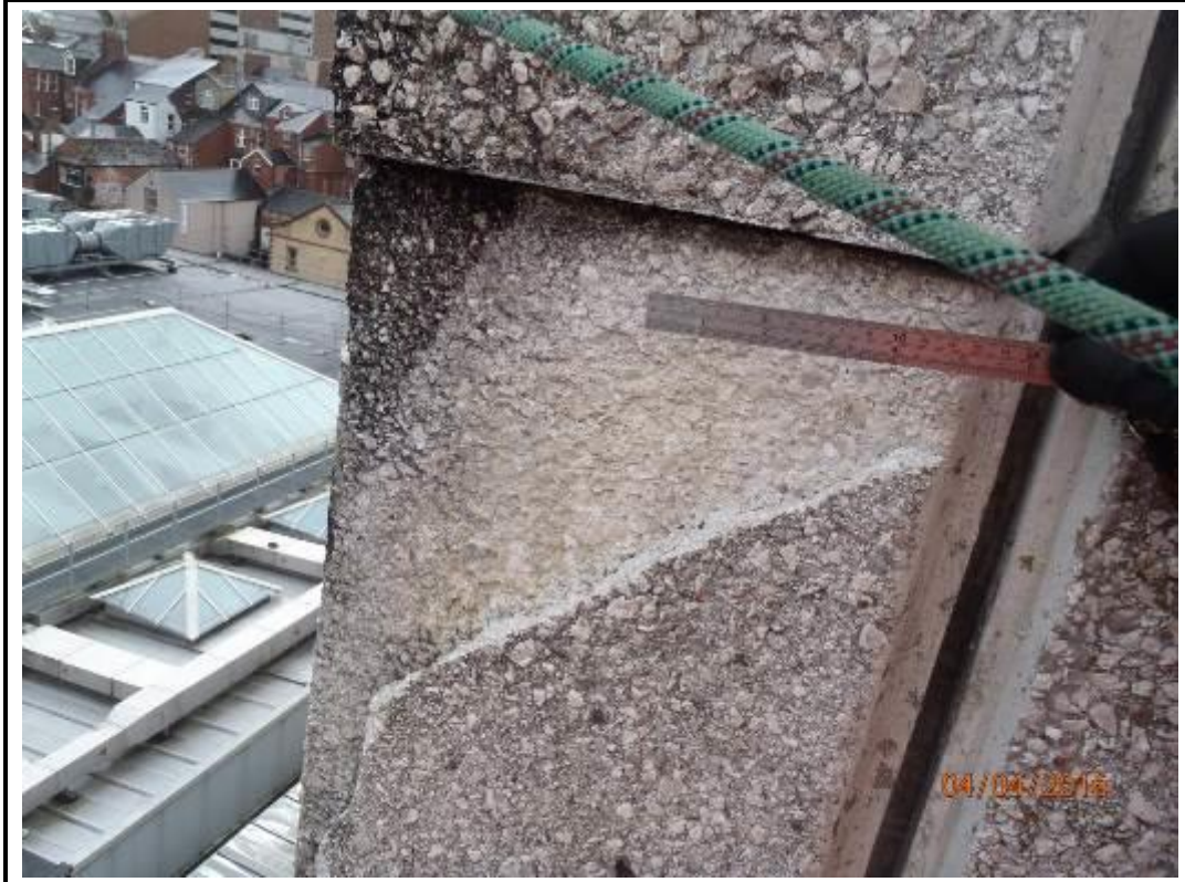
Photo 43. Drop 13 – East Elevation
