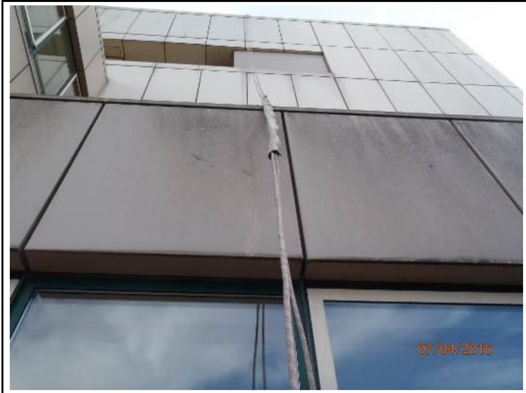
Photo 235. Drop 3 – North Elevation
