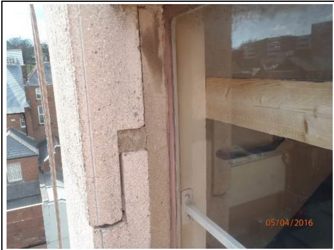
Photo 125. Drop 14 – South Elevation
