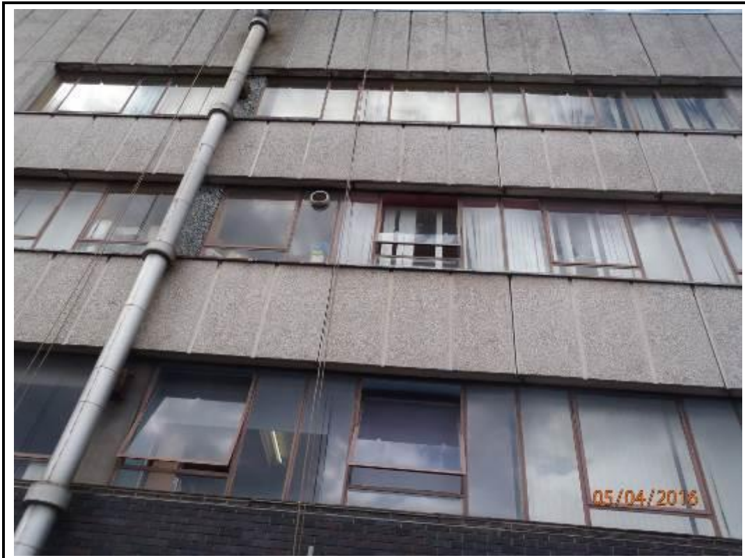
Photo 104. Drop 11 – South Elevation
