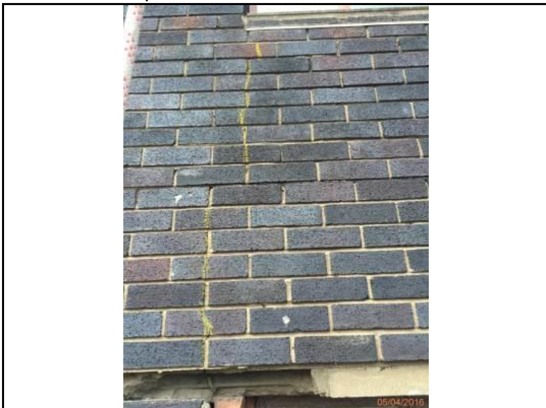
Photo 116. Drop 13 – South Elevation
