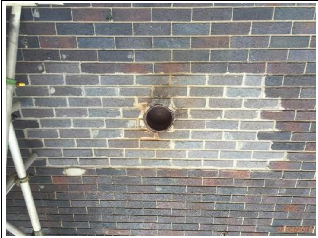
Photo 267. Drop 13 – North Elevation
