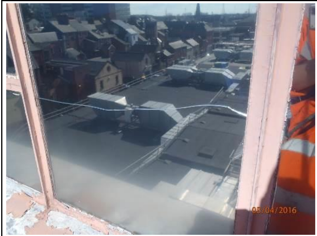
Photo 91. Drop 8 – South Elevation
