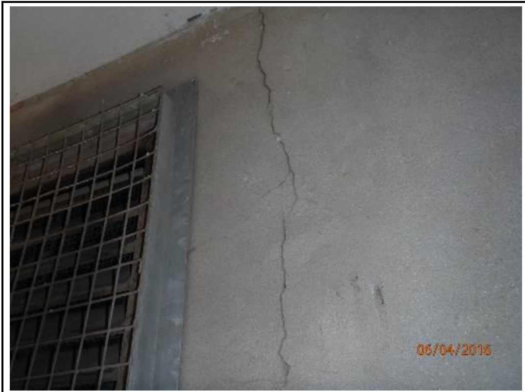
Photo 158. East Elevation – Brickwork Cladding Beneath Overhang
