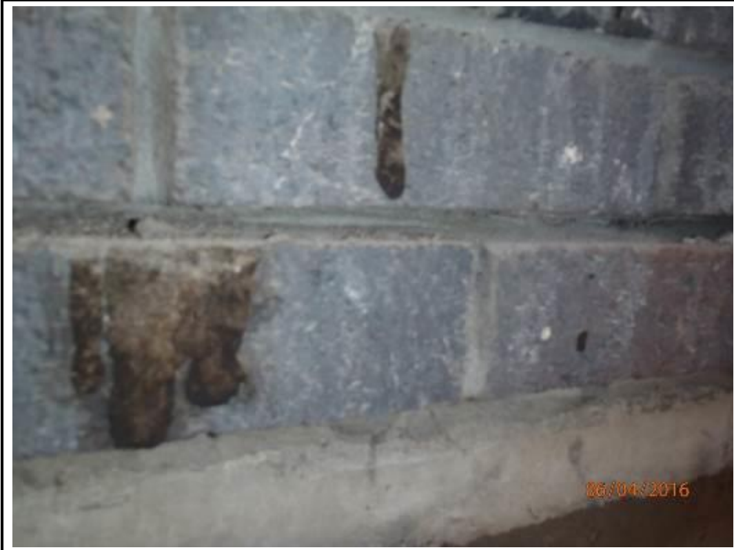
Photo 153. East Elevation – Brickwork Cladding Beneath Overhang
