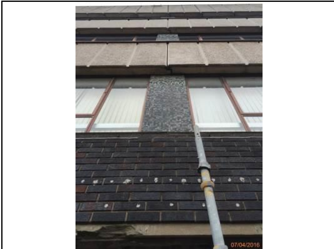
Photo 199. Drop 7 – West Elevation
