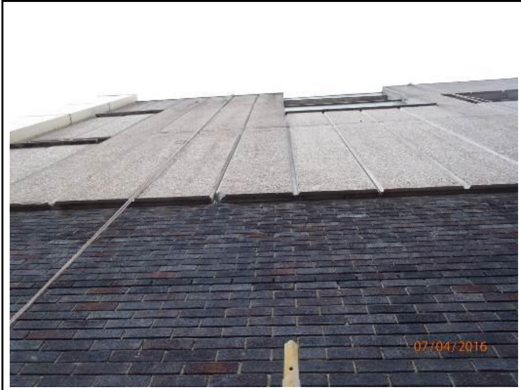
Photo 221. Drop 12 – West Elevation
