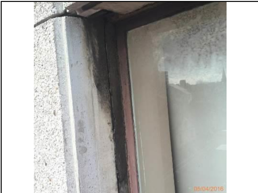
Photo 114. Drop 13 – South Elevation
