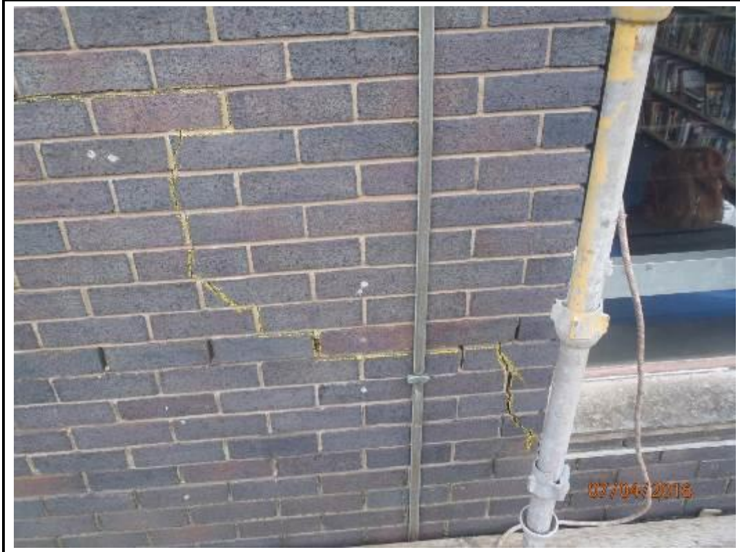
Photo 213. Drop 11 – West Elevation
