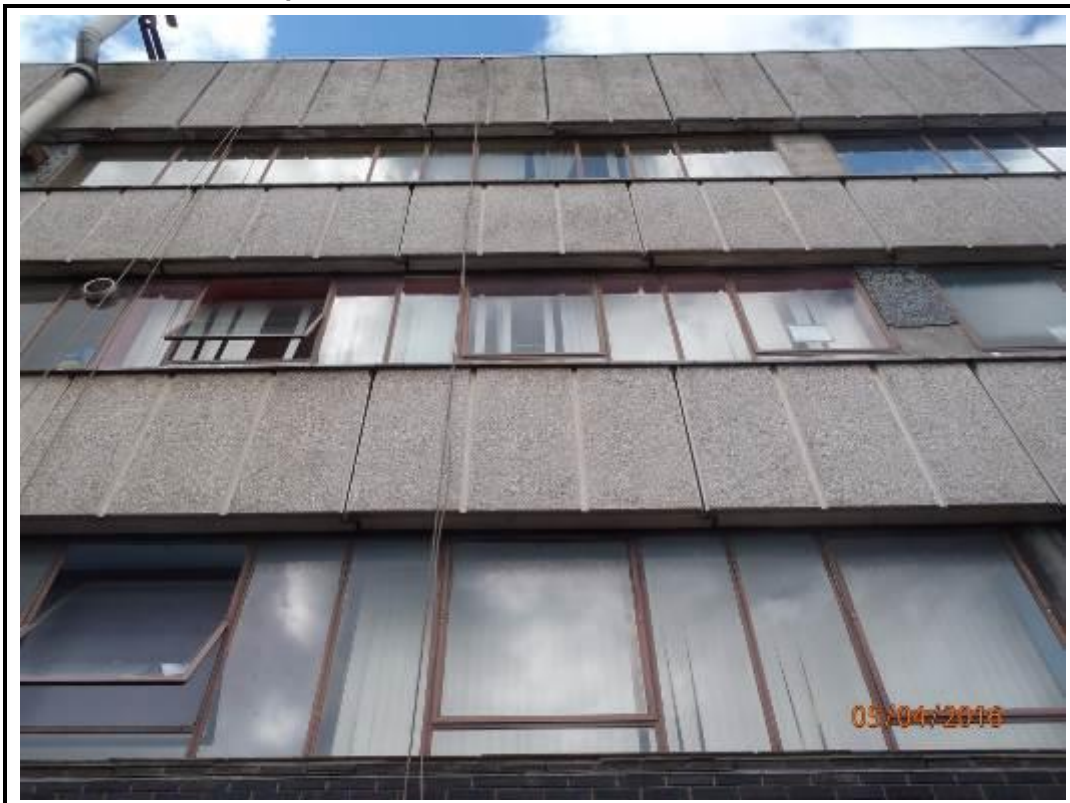
Photo 102. Drop 10 – South Elevation
