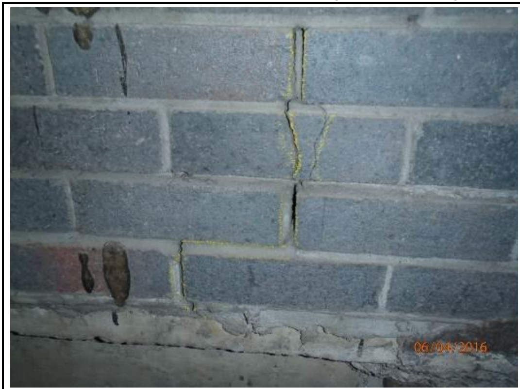
Photo 162. East Elevation – Brickwork Cladding Beneath Overhang
