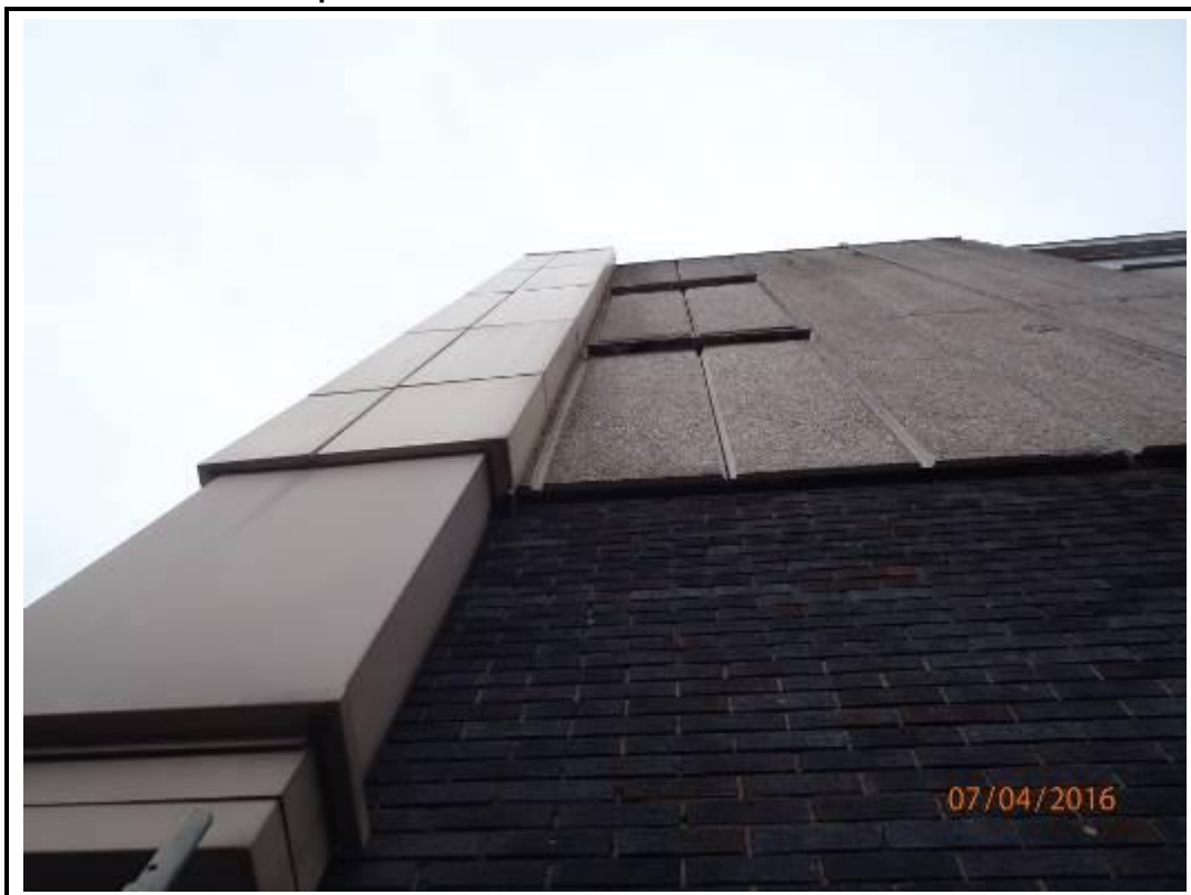
Photo 228. Drop 13 – West Elevation
