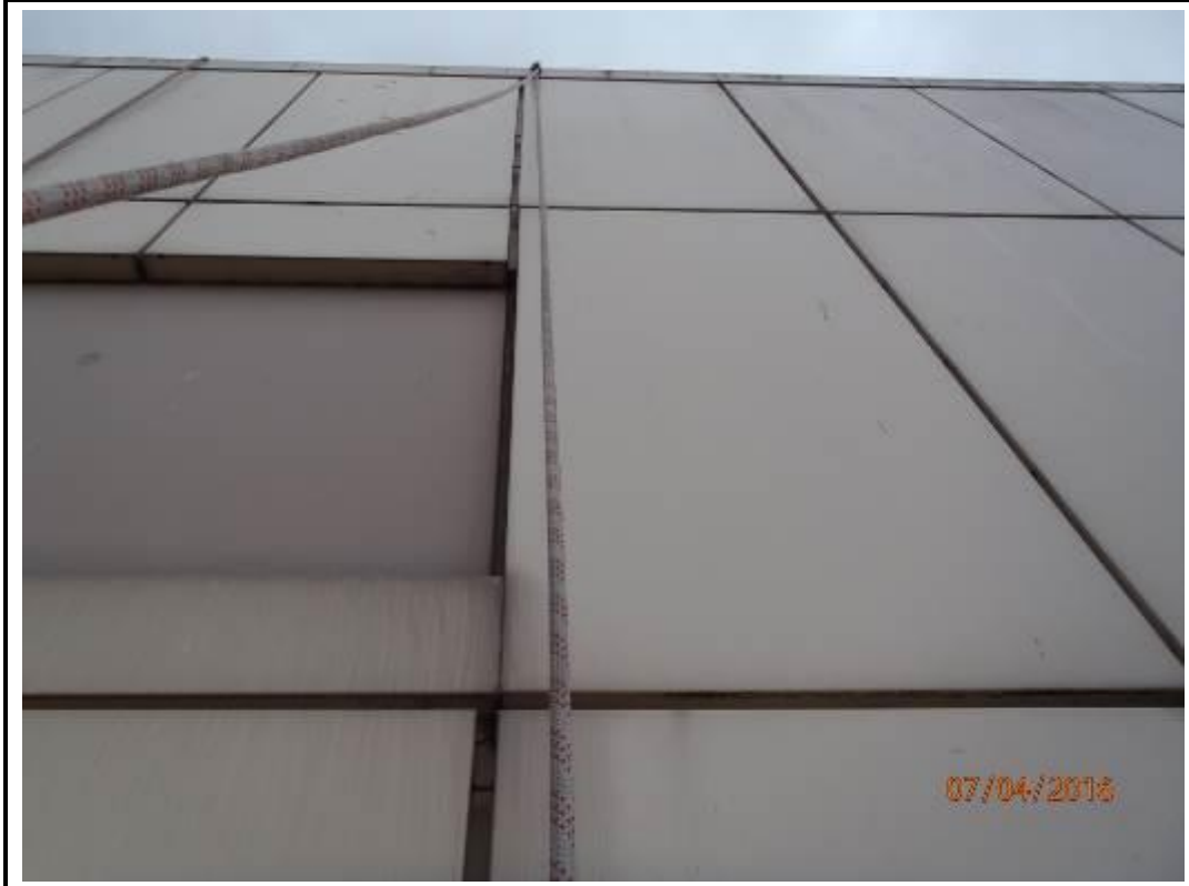
Photo 233. Drop 2 – North Elevation
