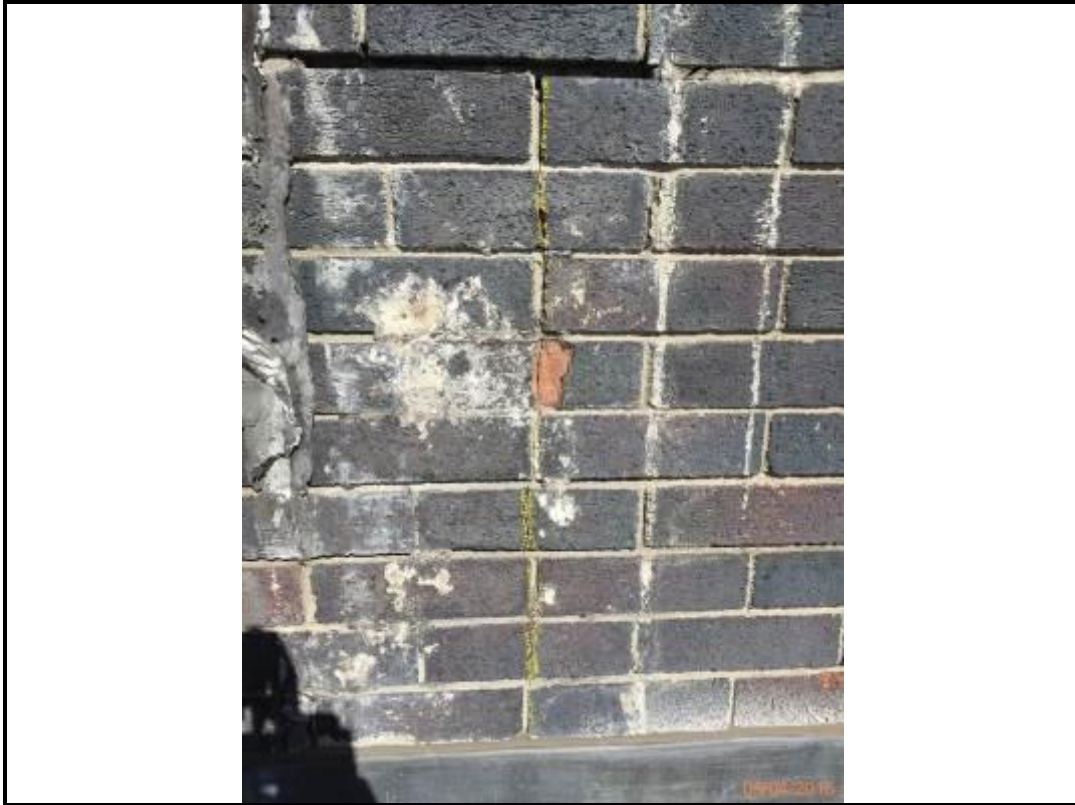
Photo 57. Drop 1 – South Elevation
