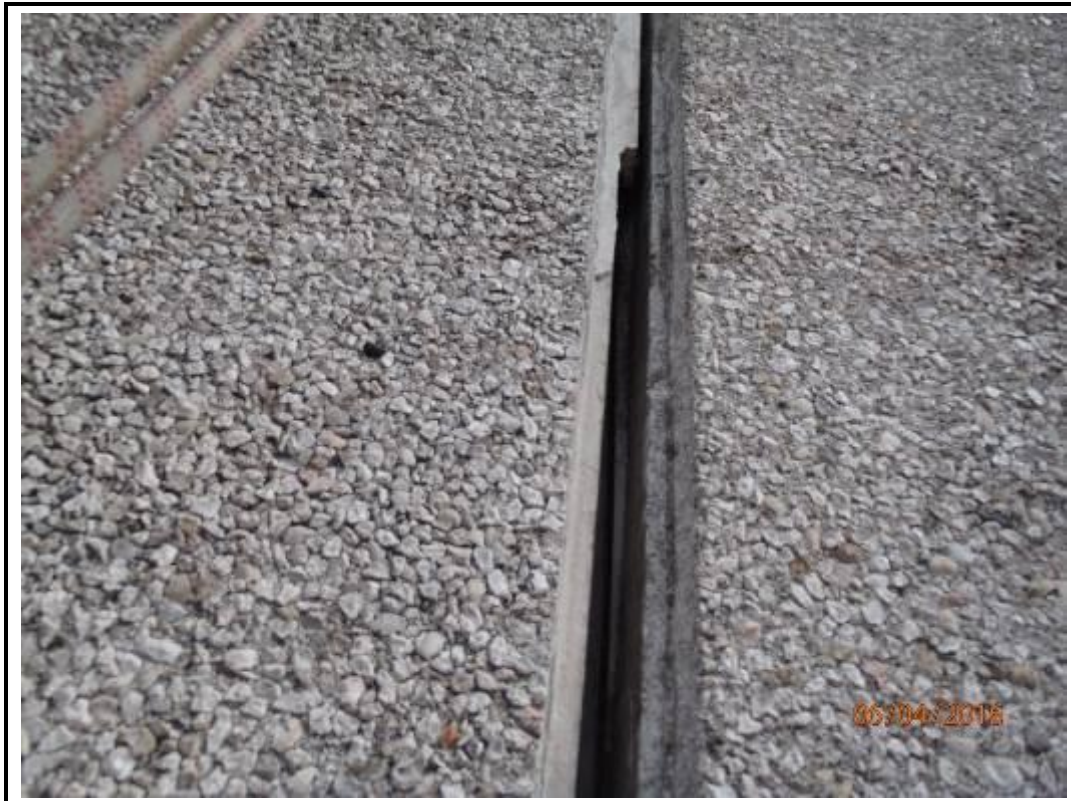
Photo 178. Drop 3 – West Elevation
