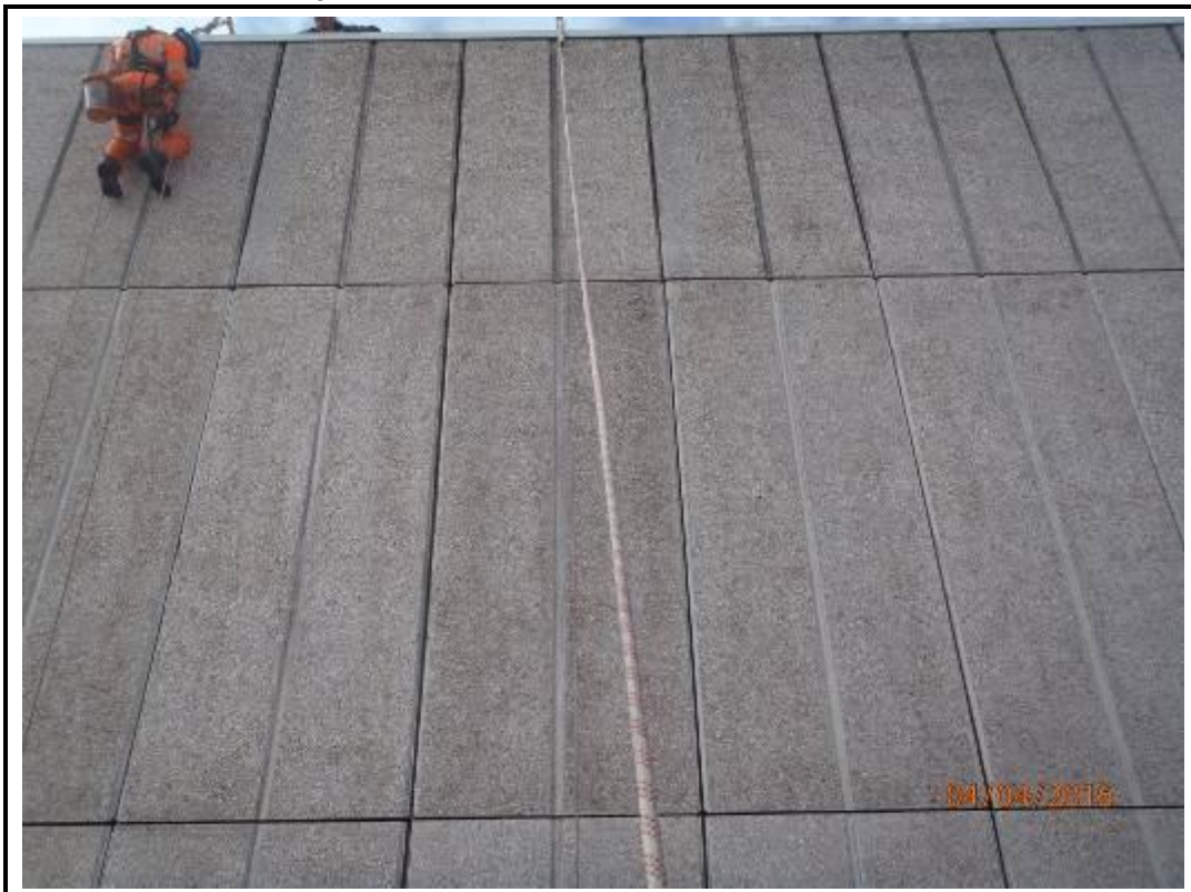
Photo 18. Drop 5 – East Elevation
