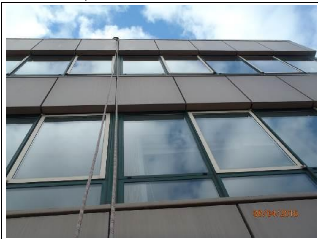
Photo 250. Drop 7 – North Elevation
