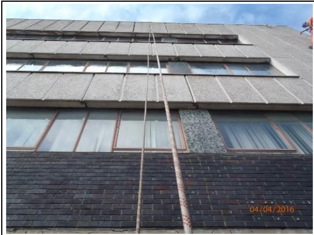
Photo 75. Drop 3 – South Elevation
