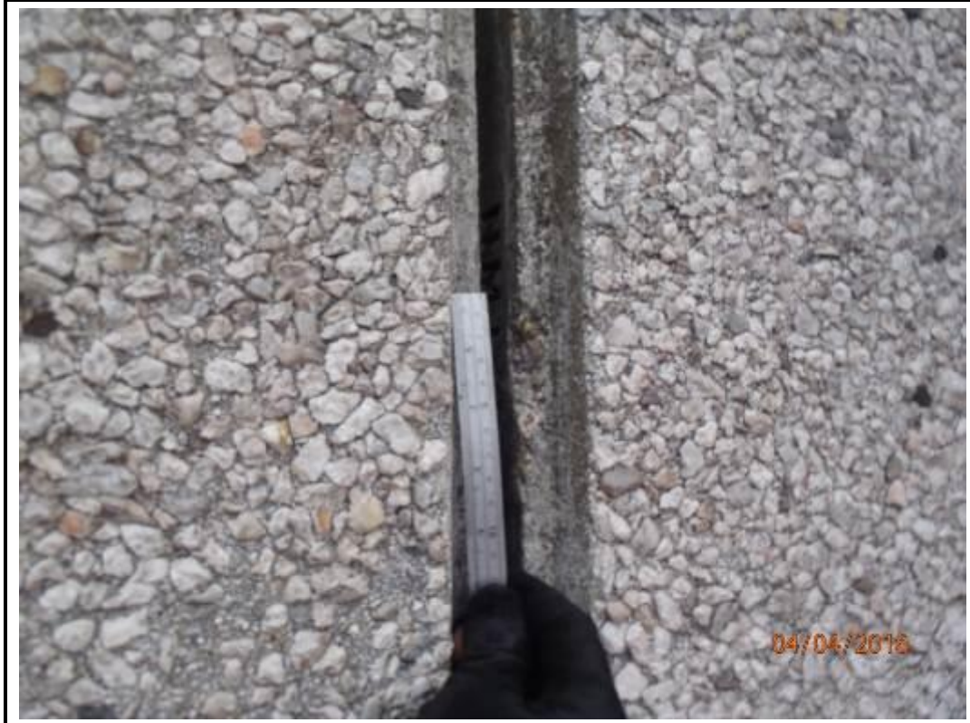
Photo 31. Drop 10 – East Elevation
