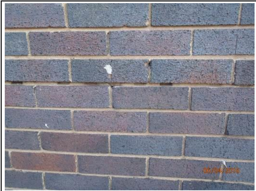
Photo 172. Drop 1 – West Elevation
