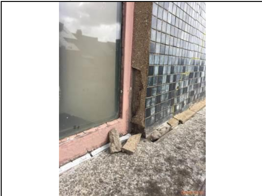
Photo 196. Drop 7 – West Elevation
