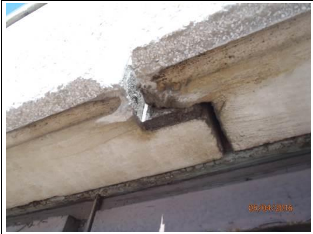
Photo 93. Drop 8 – South Elevation
