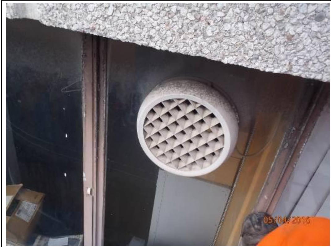
Photo 103. Drop 11 – South Elevation
