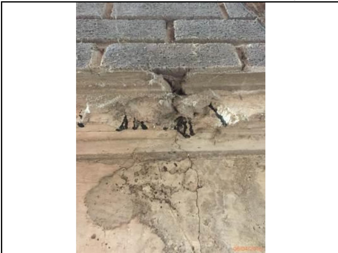
Photo 148. East Elevation – Brickwork Cladding Beneath Overhang
