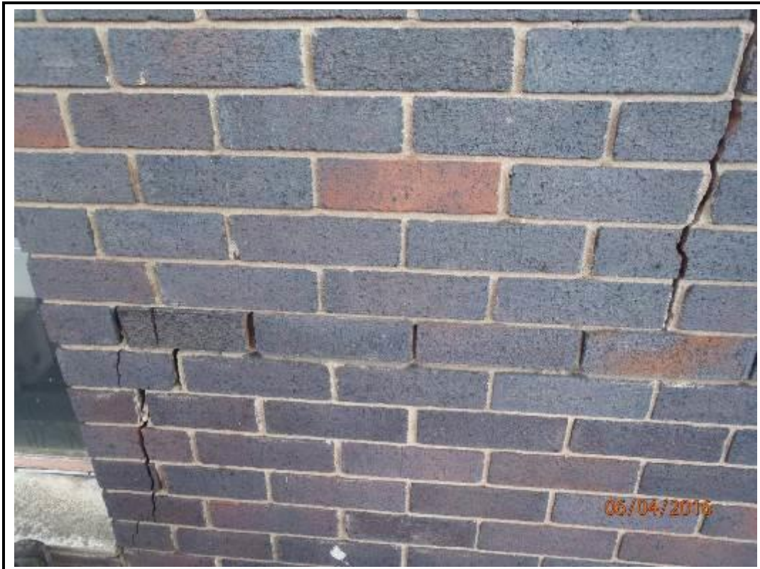
Photo 180. Drop 3 – West Elevation
