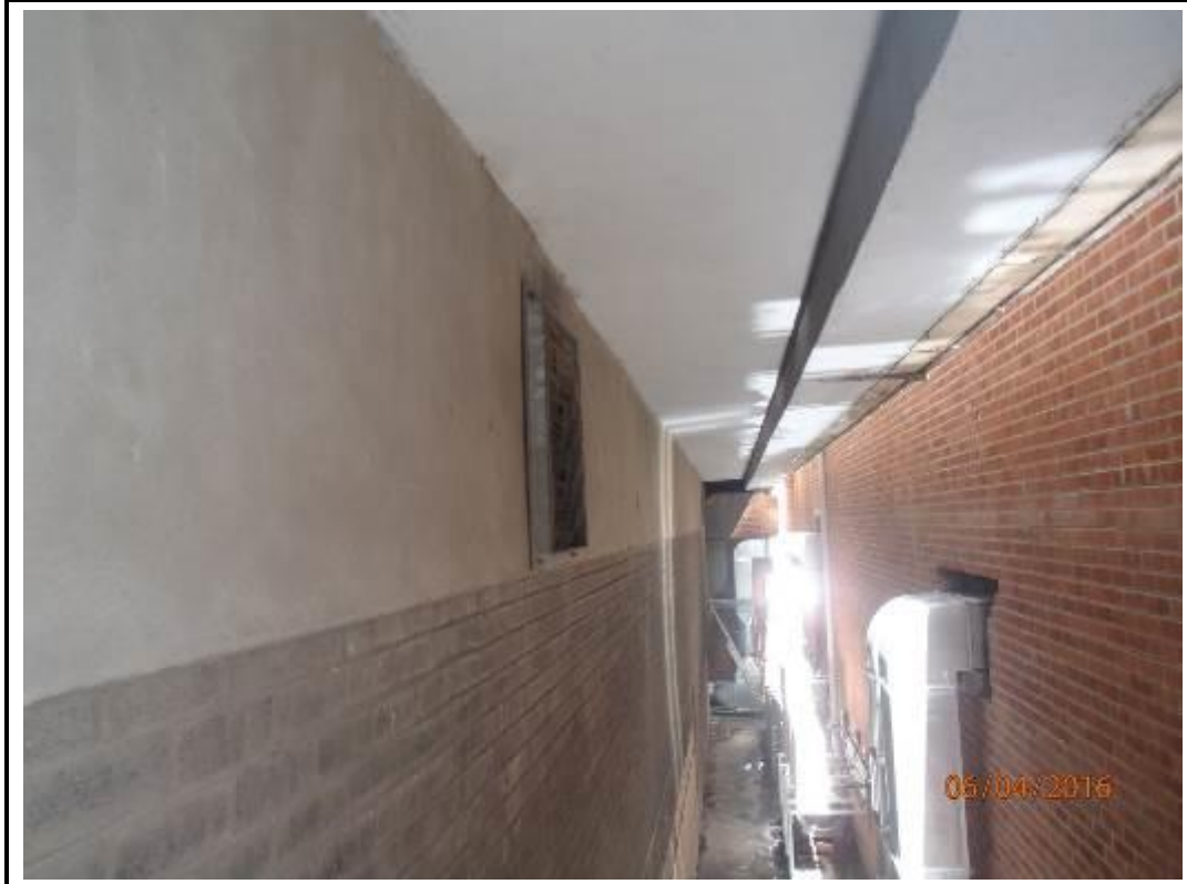
Photo 155. East Elevation – Brickwork Cladding Beneath Overhang
