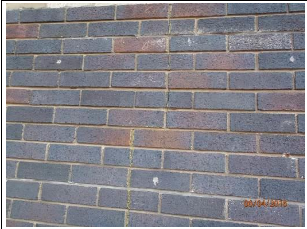
Photo 171. Drop 1 – West Elevation
