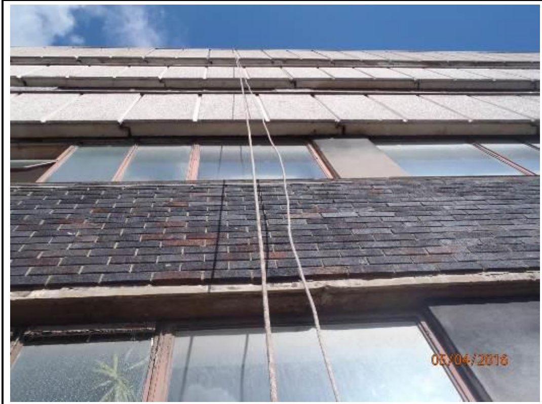
Photo 83. Drop 6 – South Elevation
