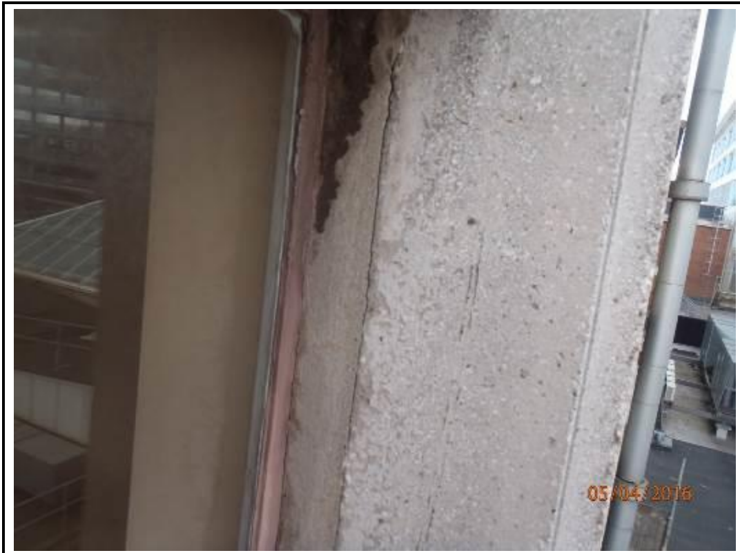
Photo 128. Drop 14 – South Elevation
