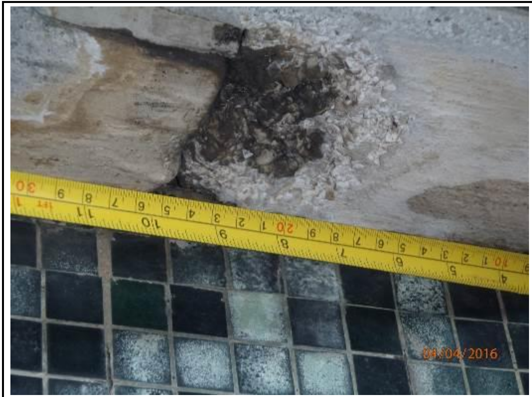
Photo 69. Drop 3 – South Elevation
