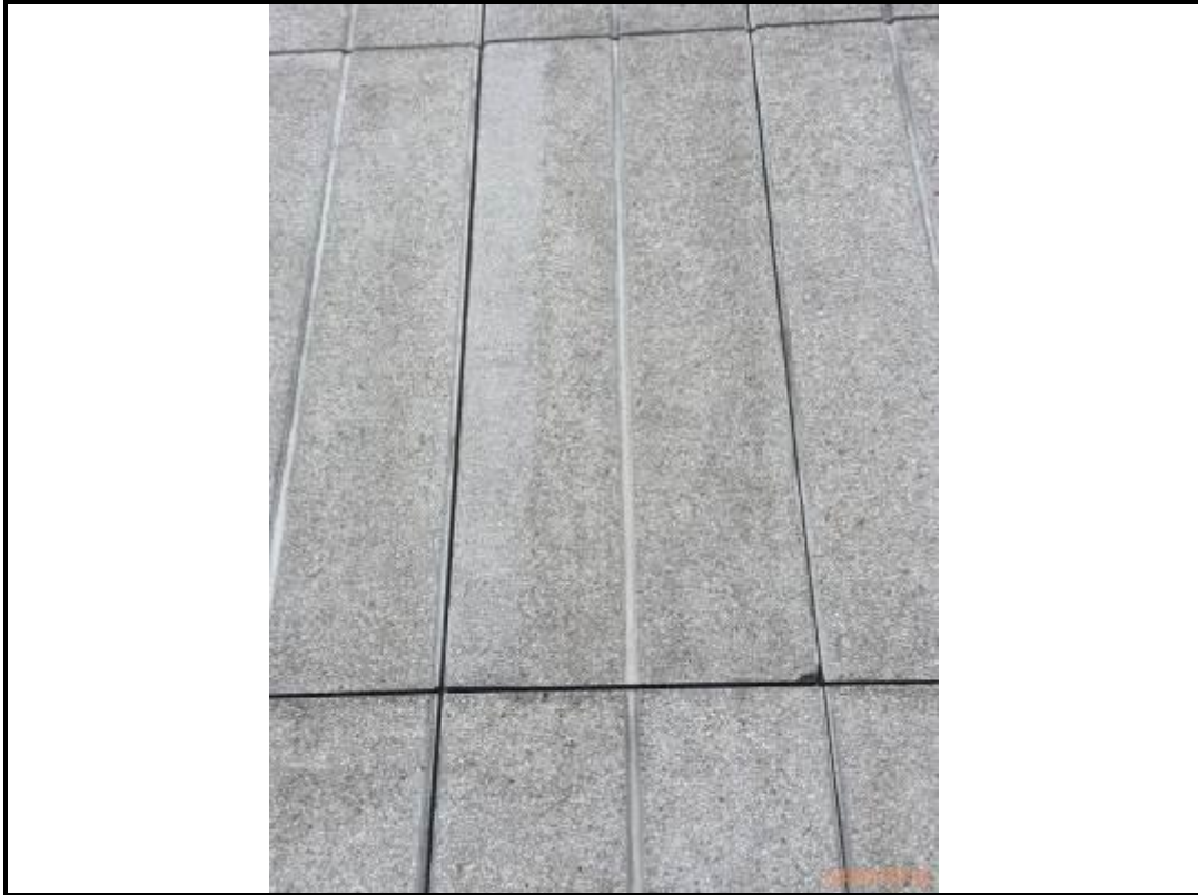
Photo 23. Drop 7 – East Elevation
