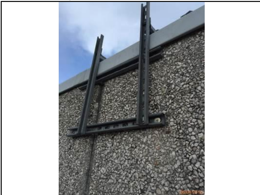
Photo 194. Drop 7 – West Elevation
