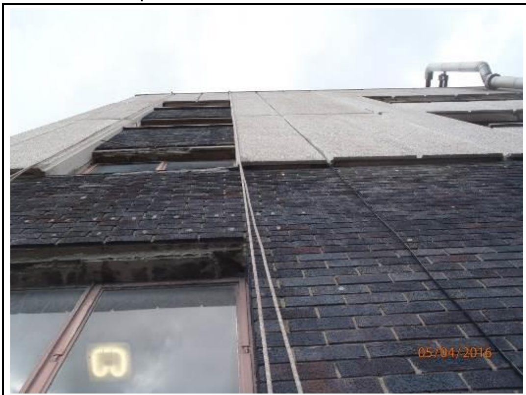
Photo 134. Drop 14 – South Elevation
