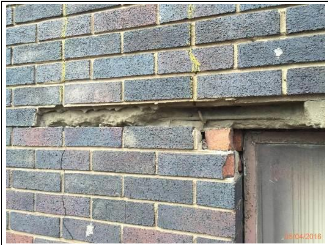
Photo 118. Drop 13 – South Elevation
