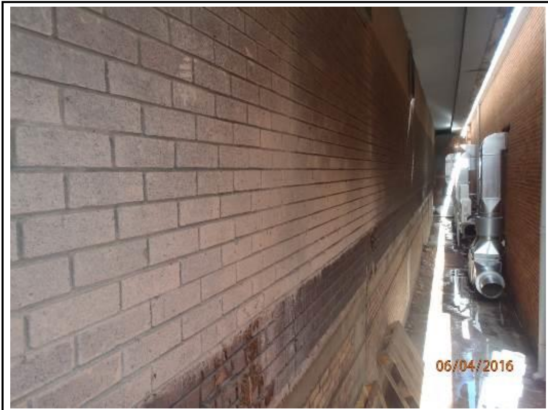
Photo 142. East Elevation – Brickwork Cladding Beneath Overhang
