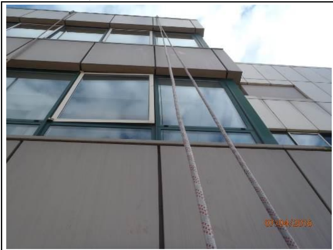
Photo 244. Drop 5 – North Elevation
