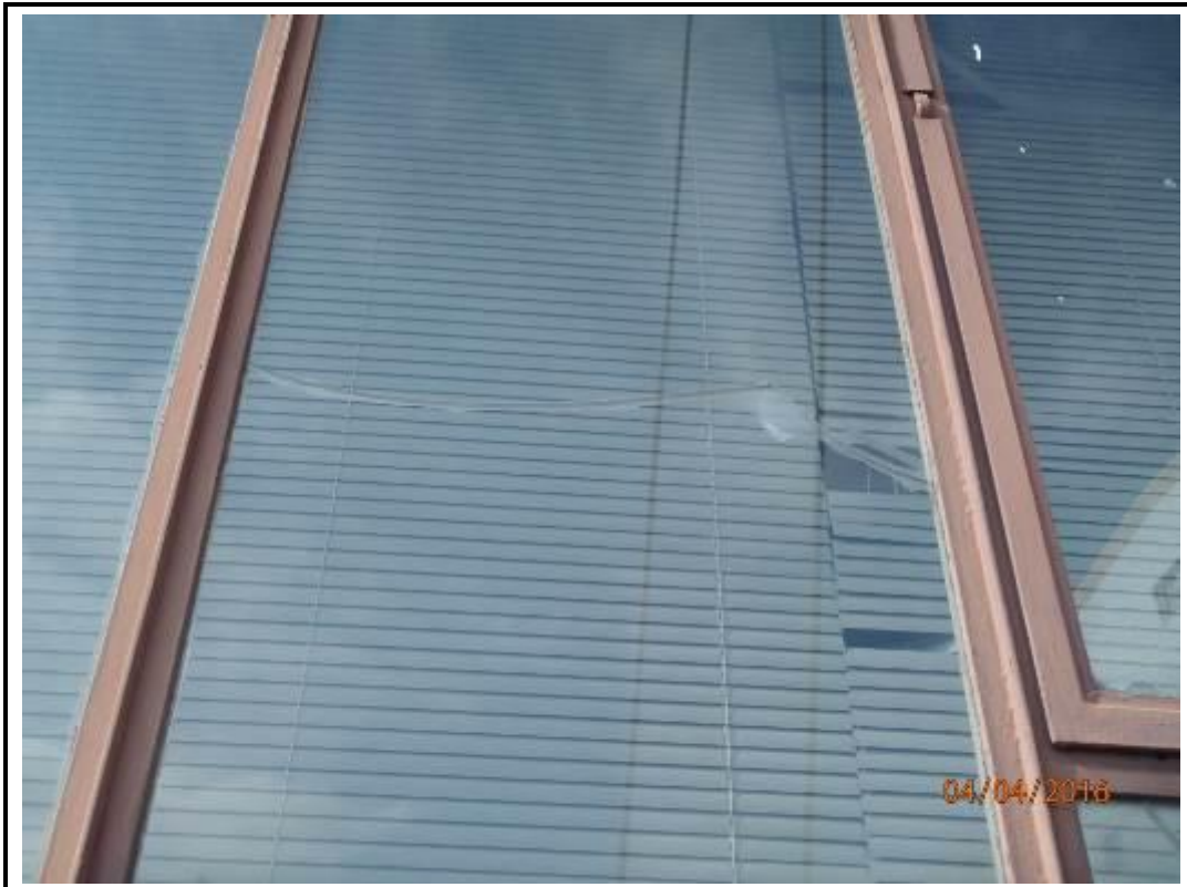
Photo 72. Drop 3 – South Elevation
