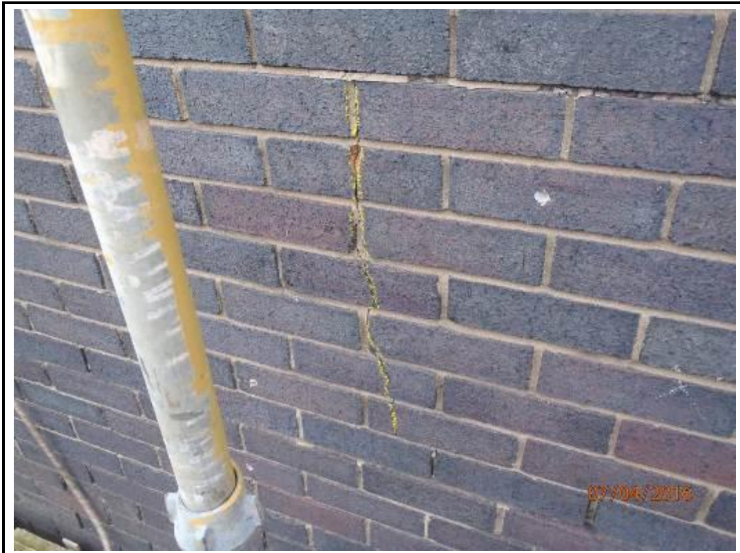
Photo 220. Drop 12 – West Elevation
