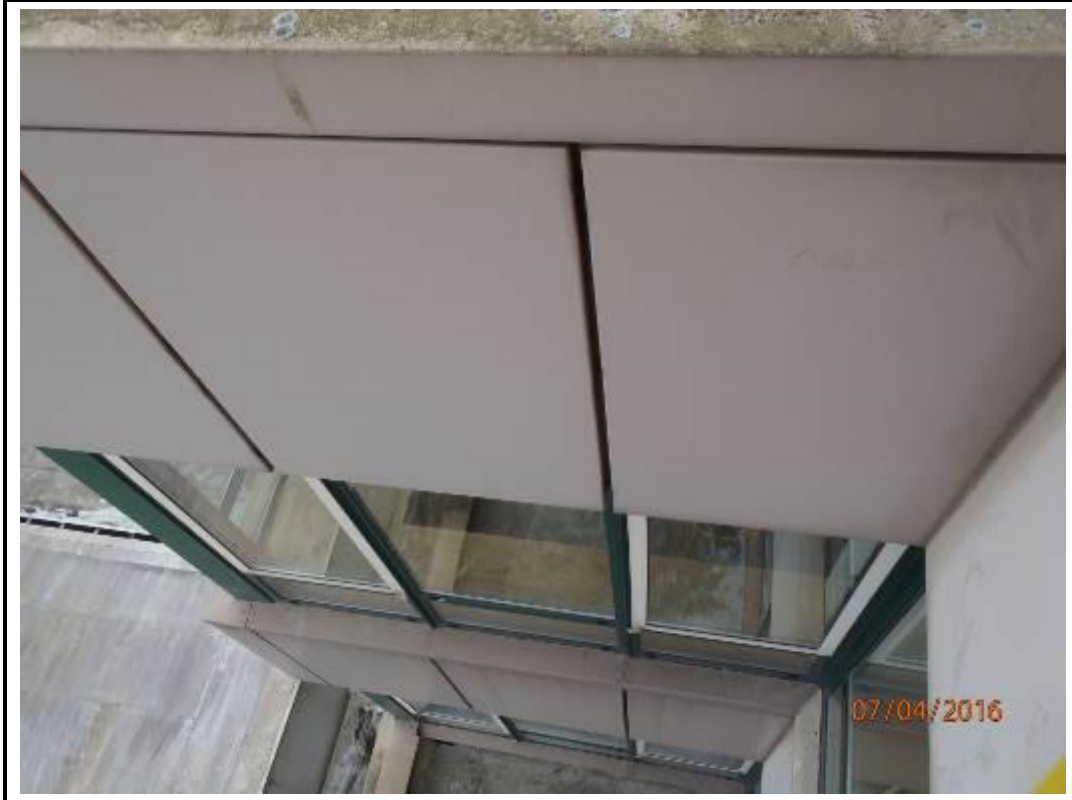
Photo 241. Drop 4 – North Elevation
