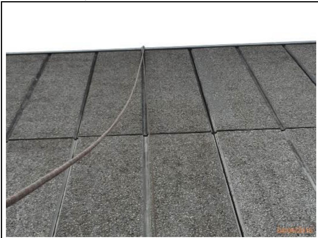
Photo 20. Drop 6 – East Elevation
