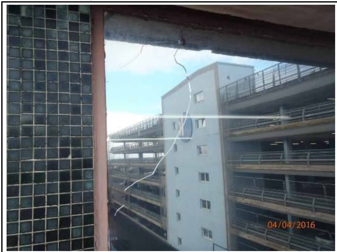
Photo 70. Drop 3 – South Elevation
