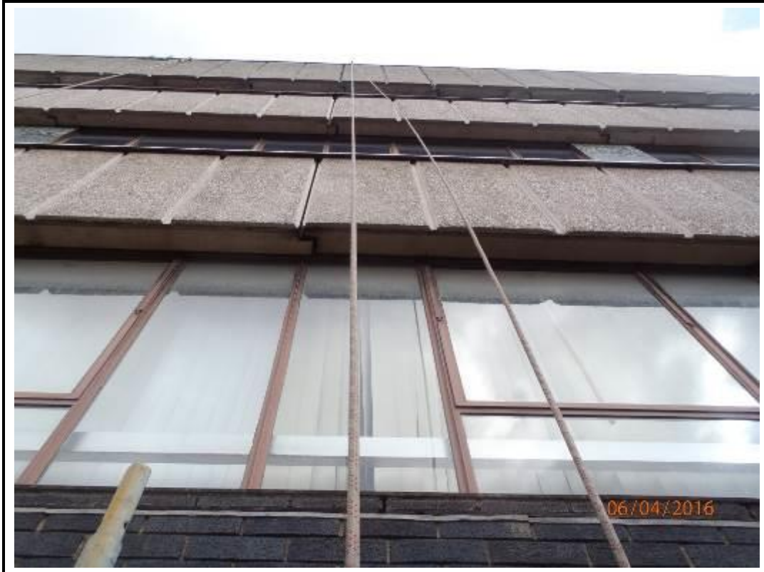
Photo 193. Drop 6 – West Elevation
