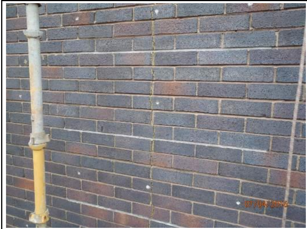
Photo 227. Drop 13 – West Elevation
