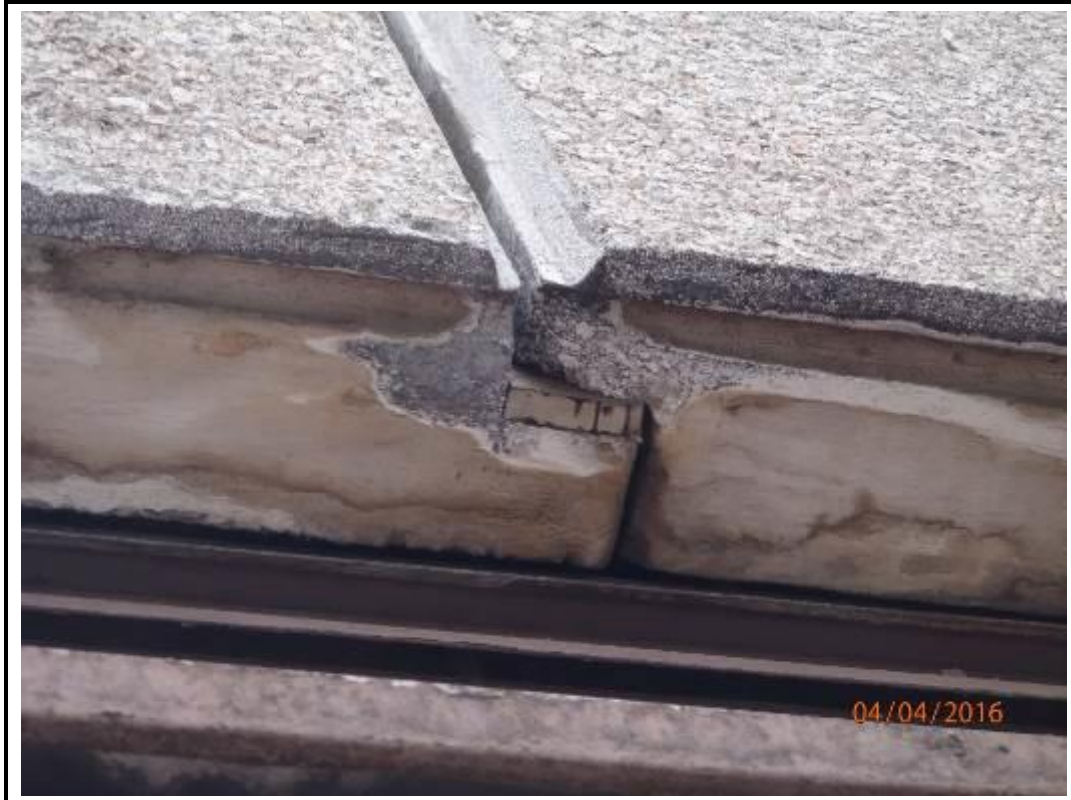
Photo 5. Drop 1 – East Elevation
