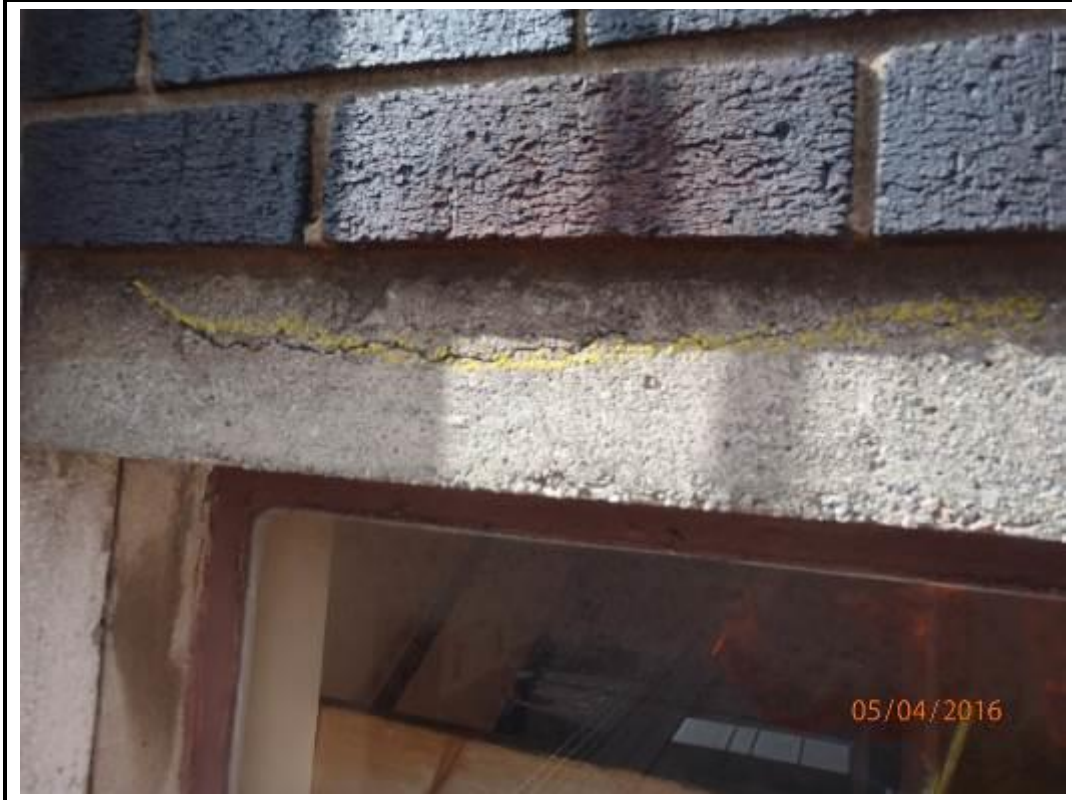
Photo 127. Drop 14 – South Elevation
