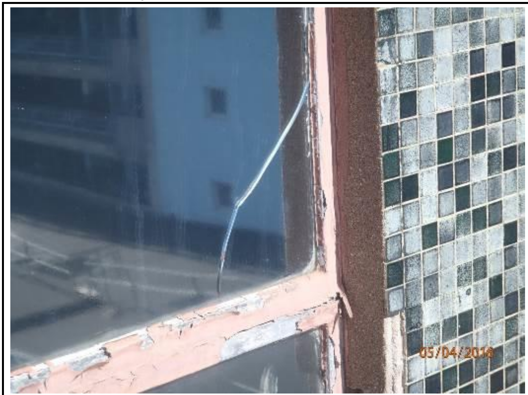
Photo 92. Drop 8 – South Elevation
