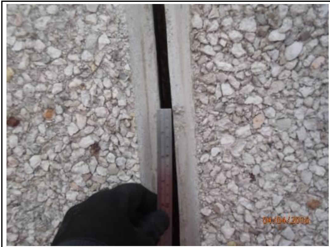
Photo 4. Drop 1 – East Elevation
