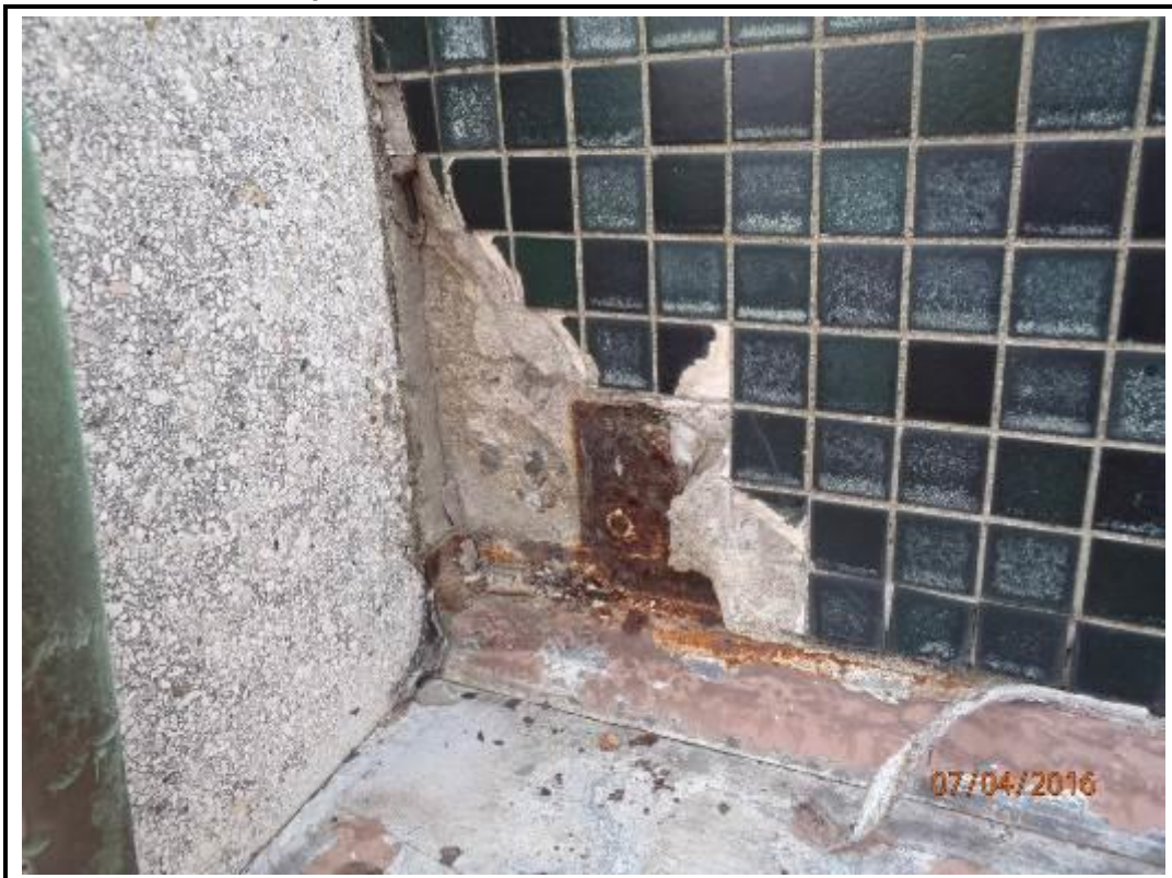
Photo 208. Drop 11 – West Elevation
