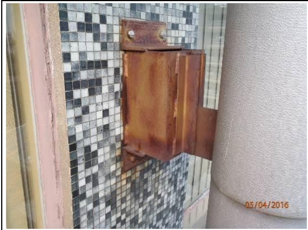
Photo 105. Drop 12 – South Elevation
