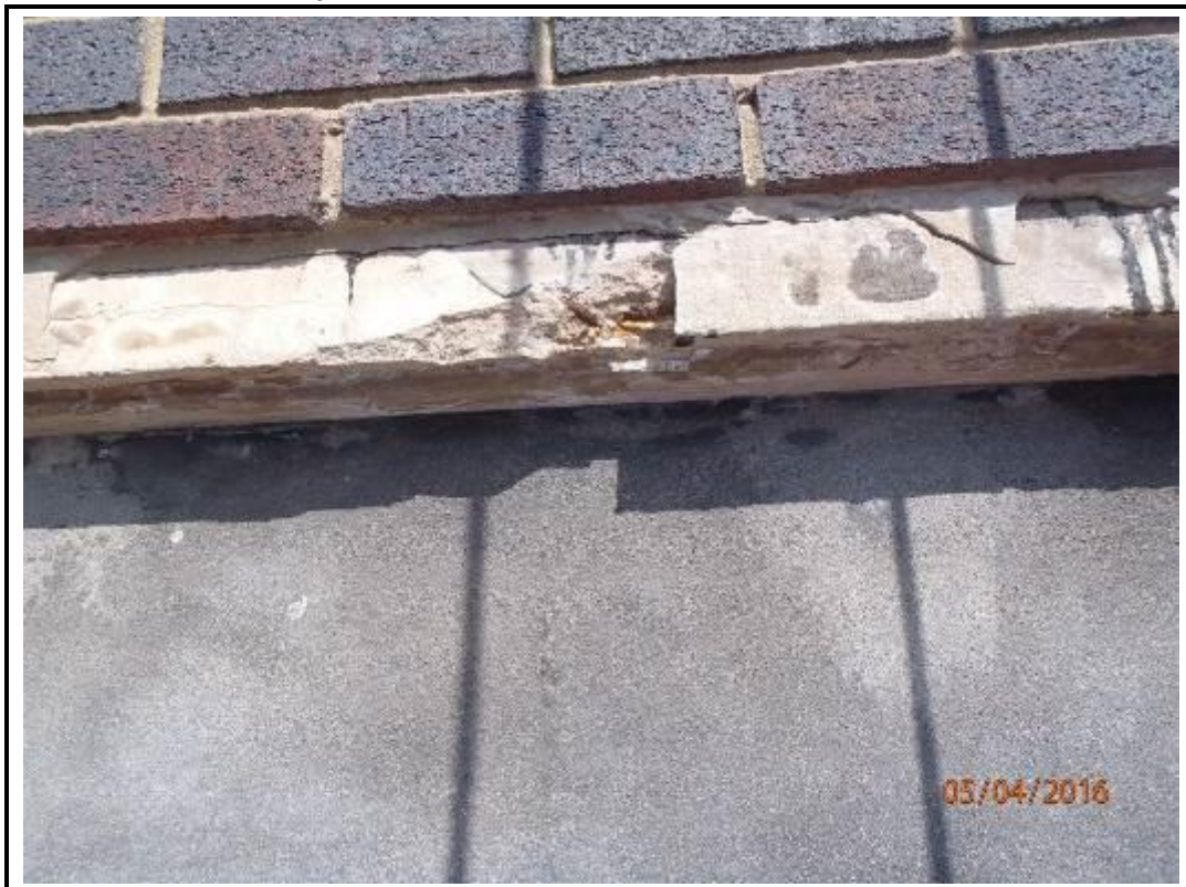
Photo 86. Drop 7 – South Elevation
