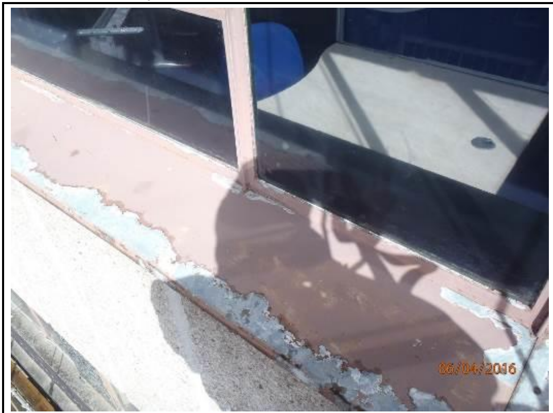
Photo 192. Drop 6 – West Elevation
