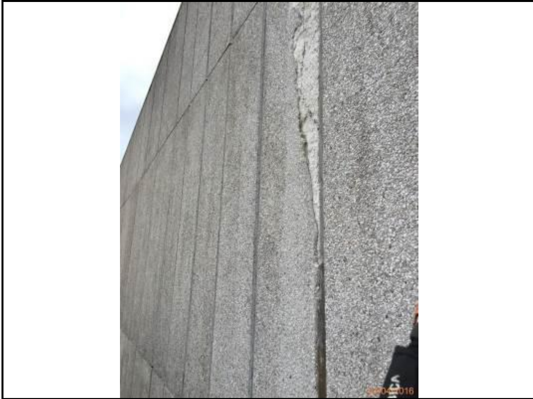
Photo 9. Drop 2 – East Elevation
