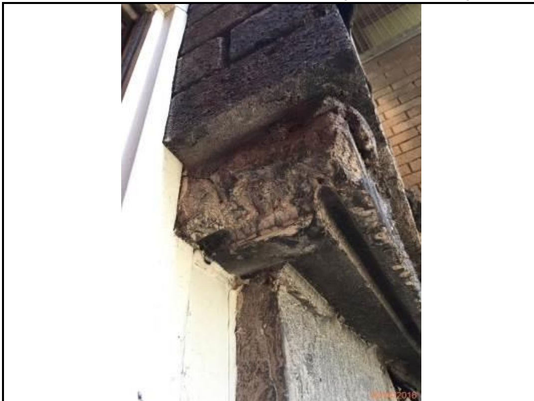
Photo 144. East Elevation – Brickwork Cladding Beneath Overhang
