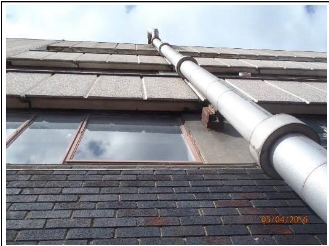
Photo 108. Drop 12 – South Elevation
