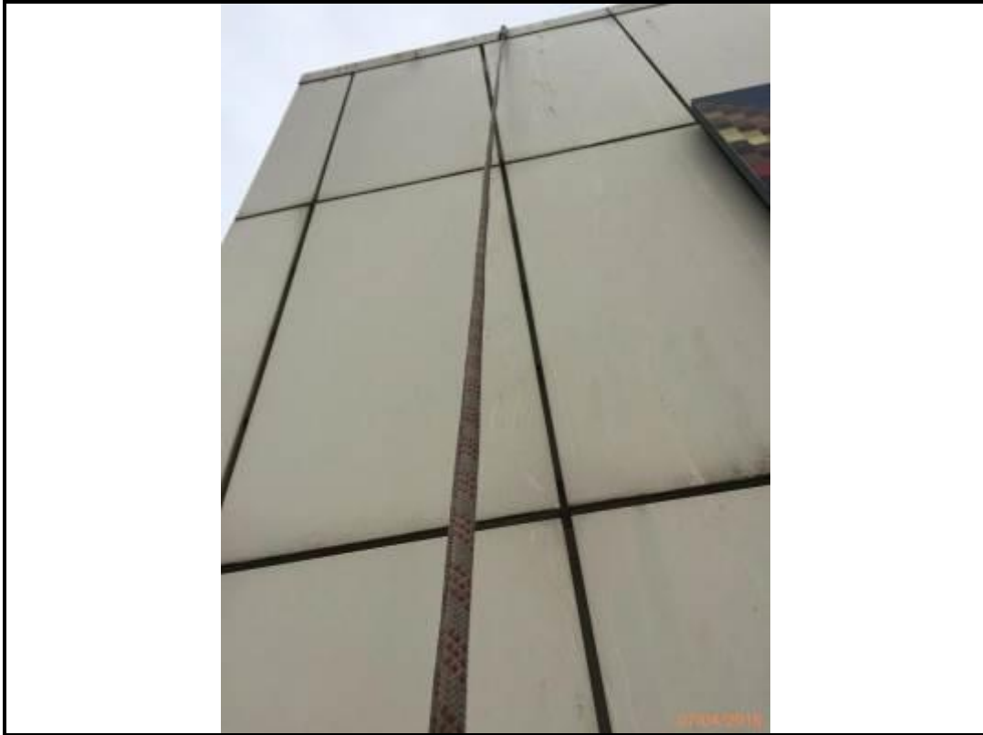
Photo 275. Drop 21 – North Elevation
