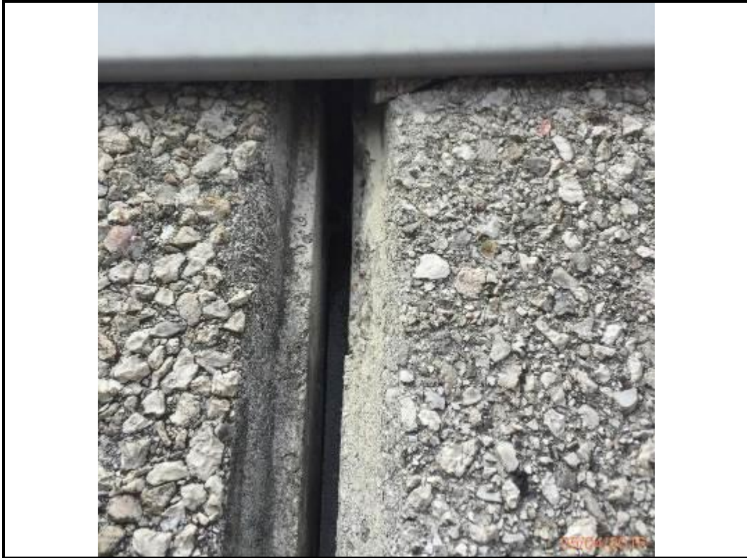
Photo 109. Drop 13 – South Elevation
