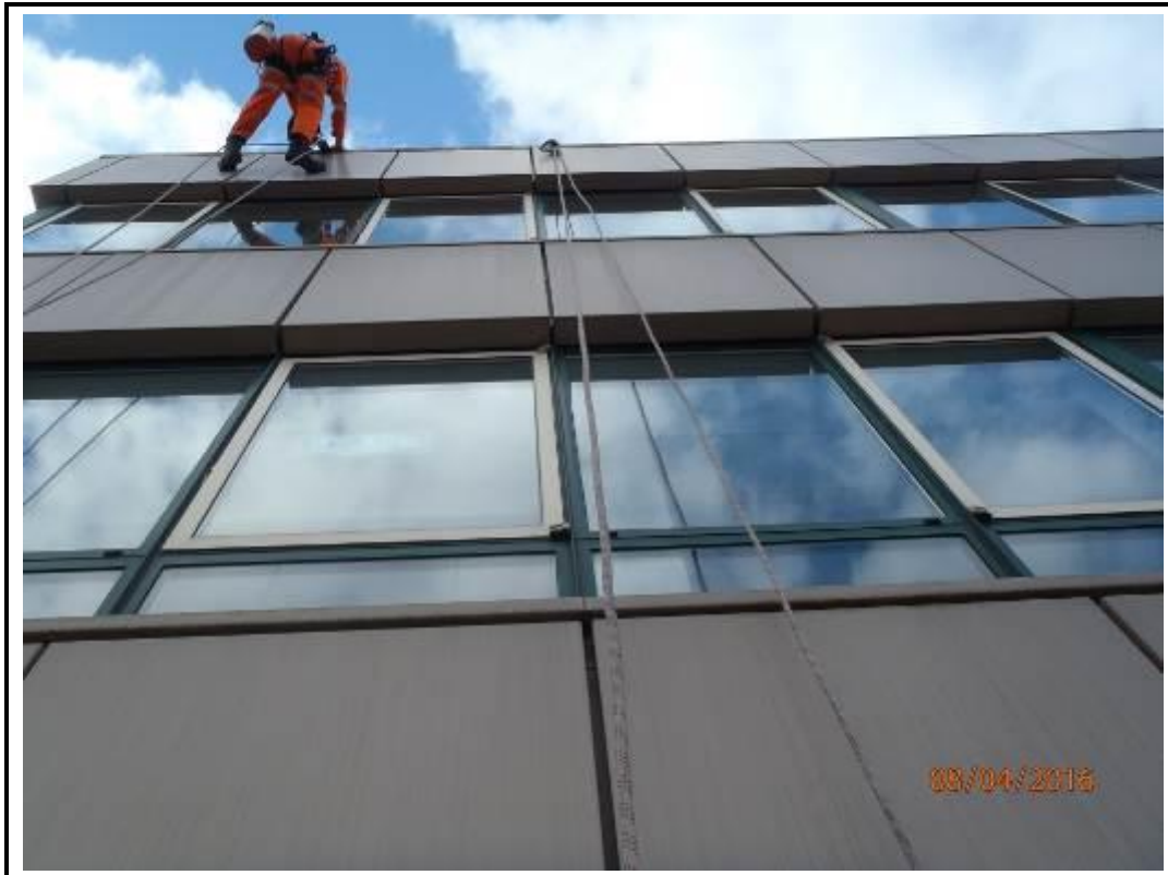
Photo 251. Drop 8 – North Elevation
