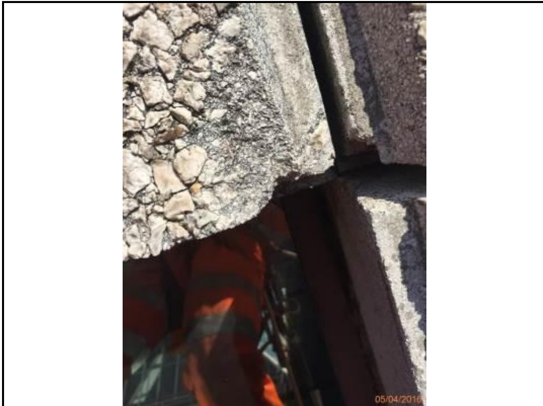
Photo 59. Drop 2 – South Elevation
