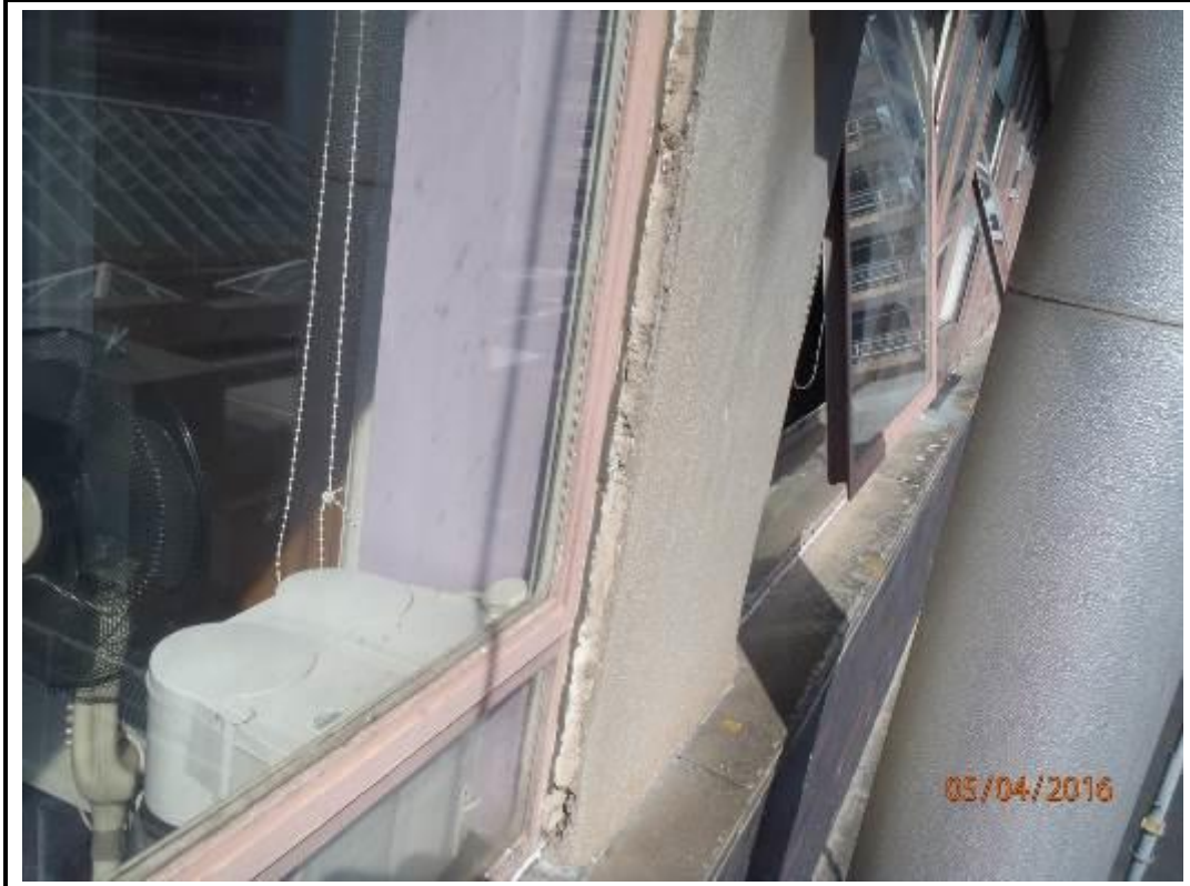
Photo 107. Drop 12 – South Elevation
