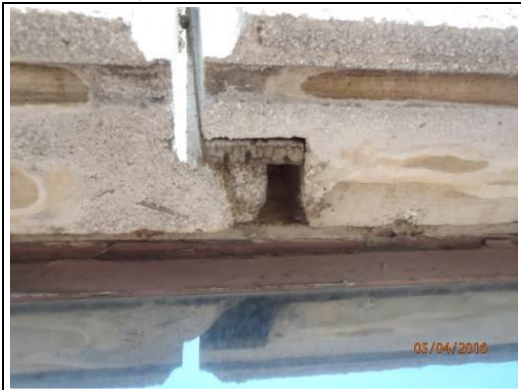
Photo 90. Drop 8 – South Elevation
