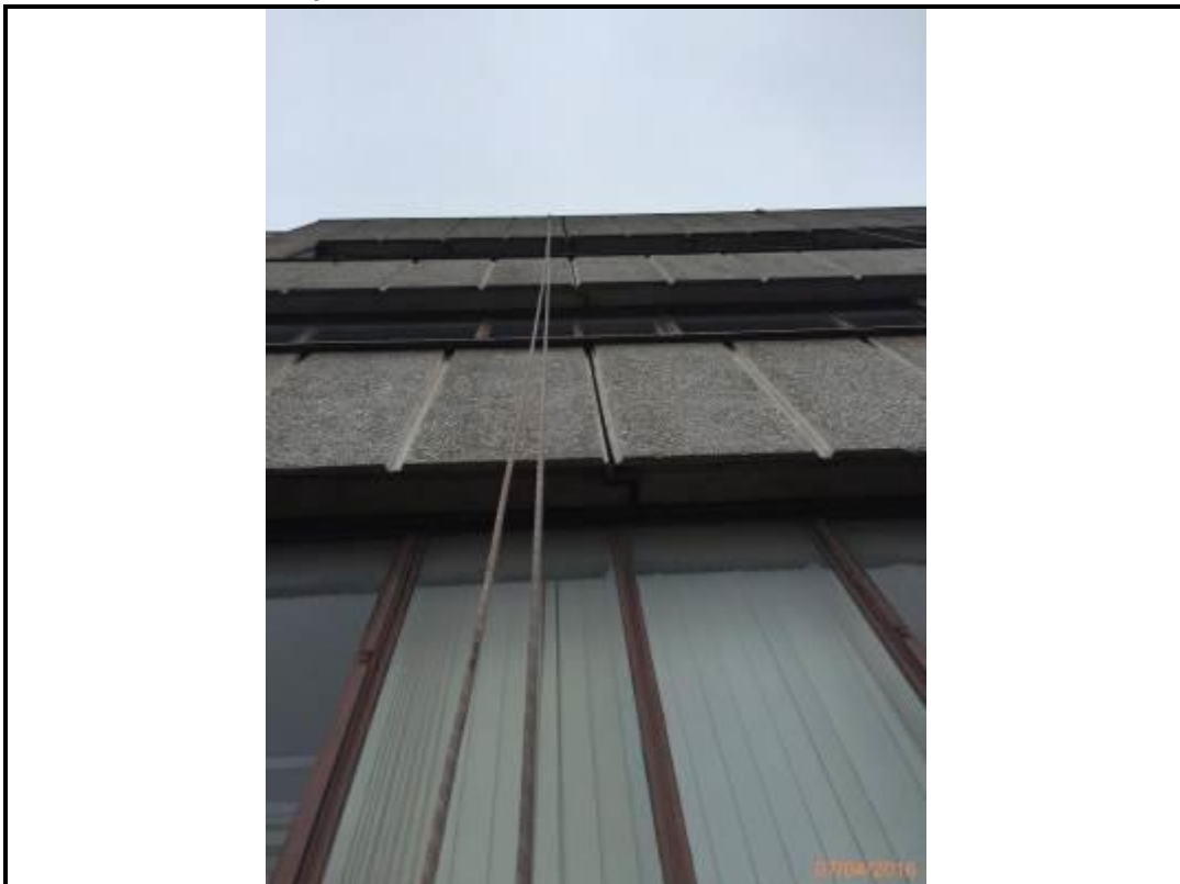
Photo 206. Drop 10 – West Elevation
