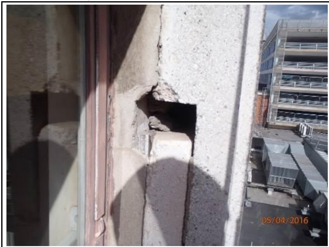
Photo 126. Drop 14 – South Elevation
