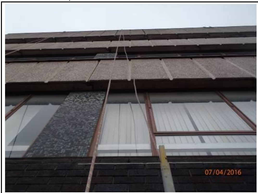
Photo 204. Drop 9 – West Elevation
