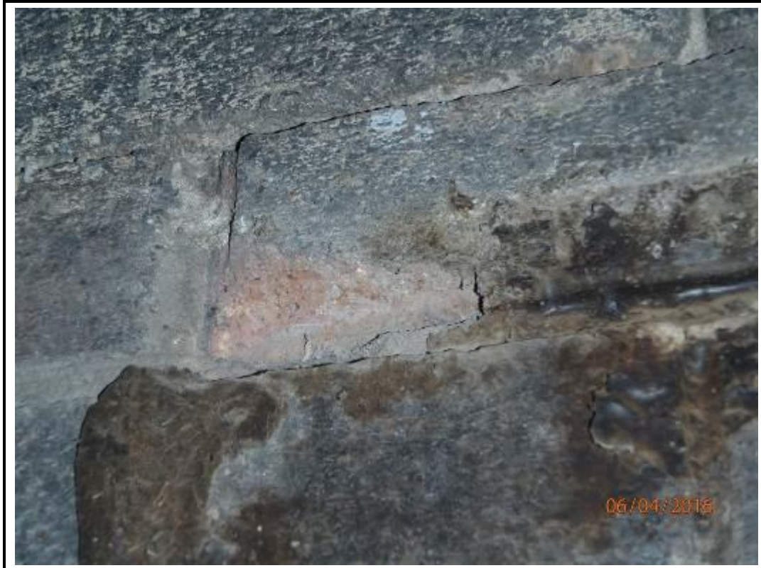
Photo 165. East Elevation – Brickwork Cladding Beneath Overhang
