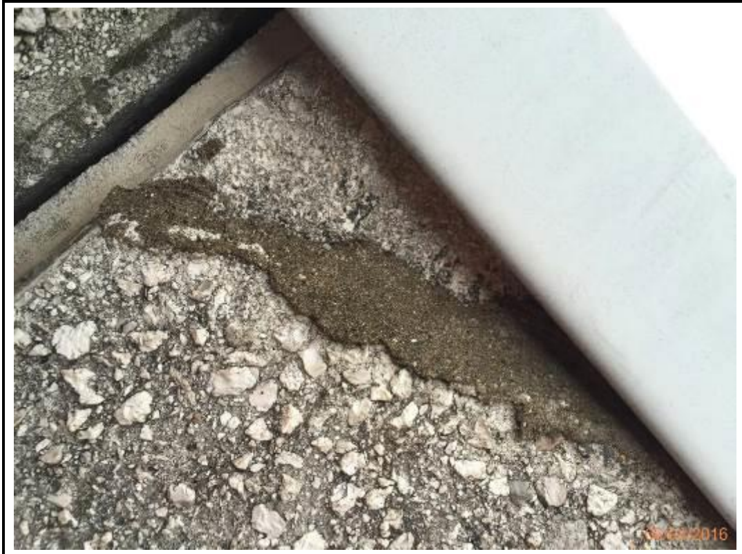
Photo 183. Drop 4 – West Elevation
