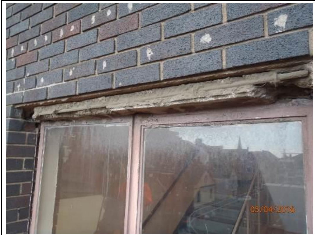
Photo 133. Drop 14 – South Elevation
