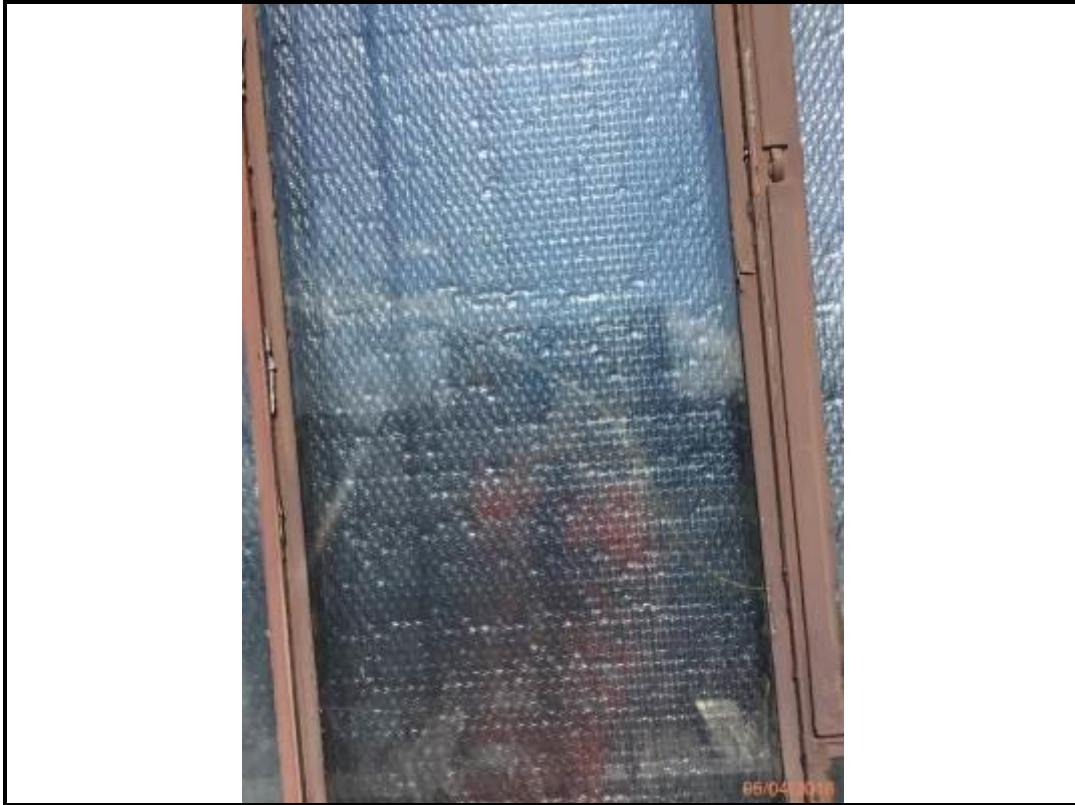
Photo 79. Drop 5 – South Elevation
