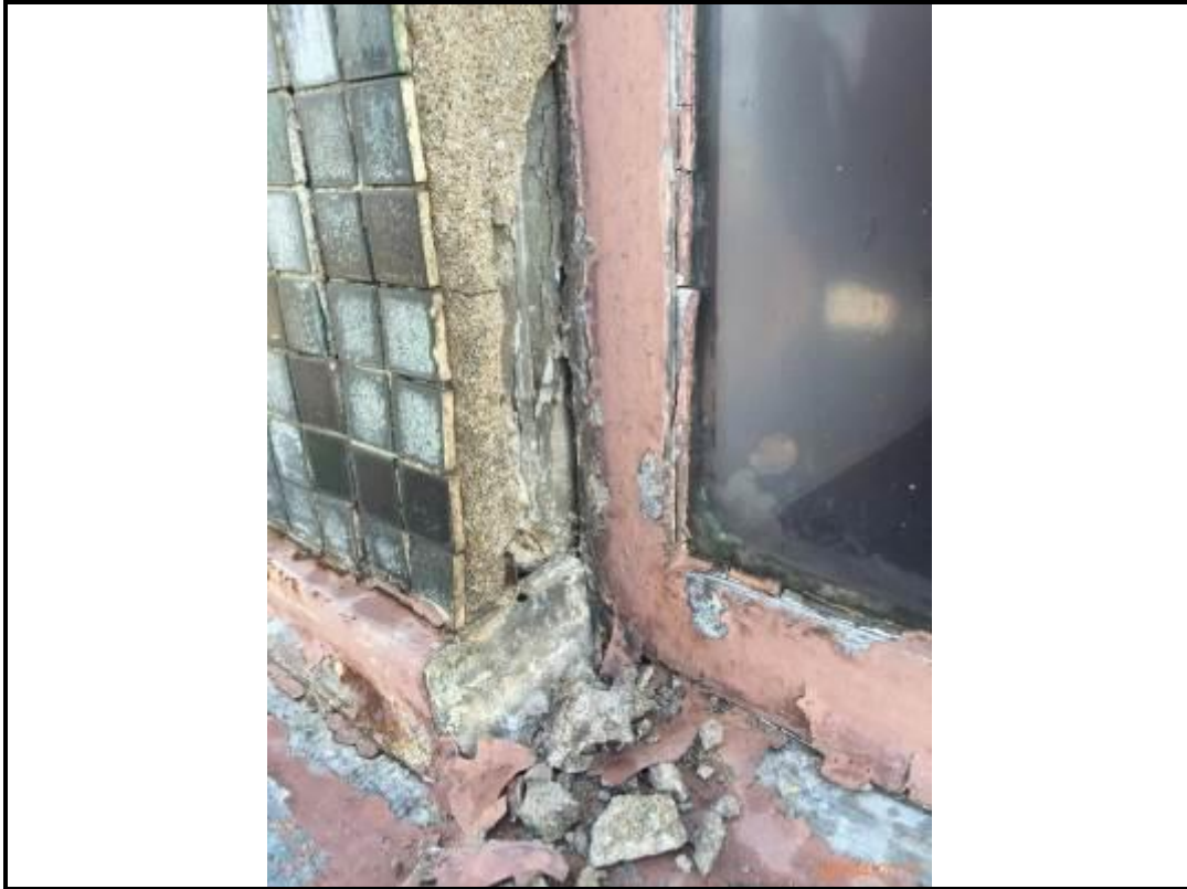
Photo 187. Drop 5 – West Elevation
