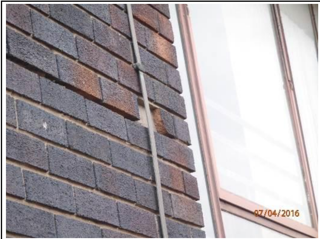
Photo 210. Drop 11 – West Elevation
