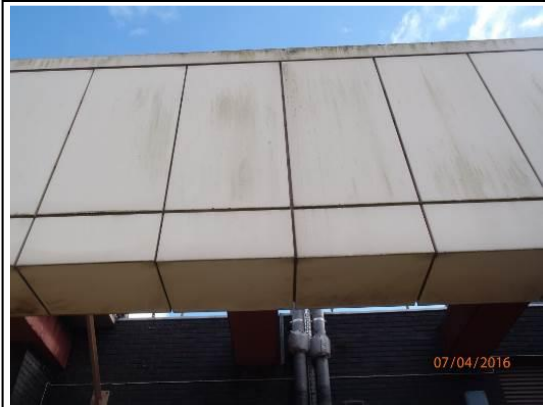
Photo 247. Drop 6 – North Elevation
