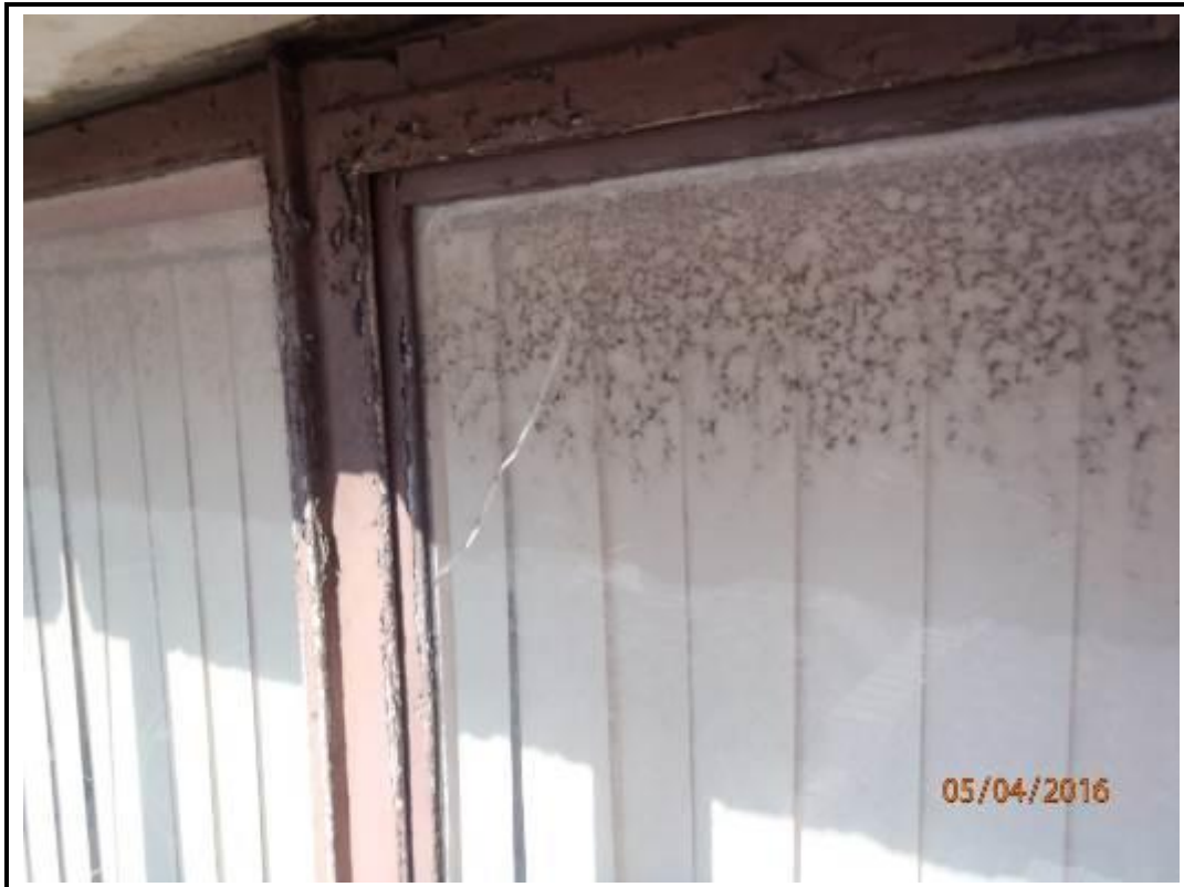
Photo 95. Drop 9 – South Elevation
