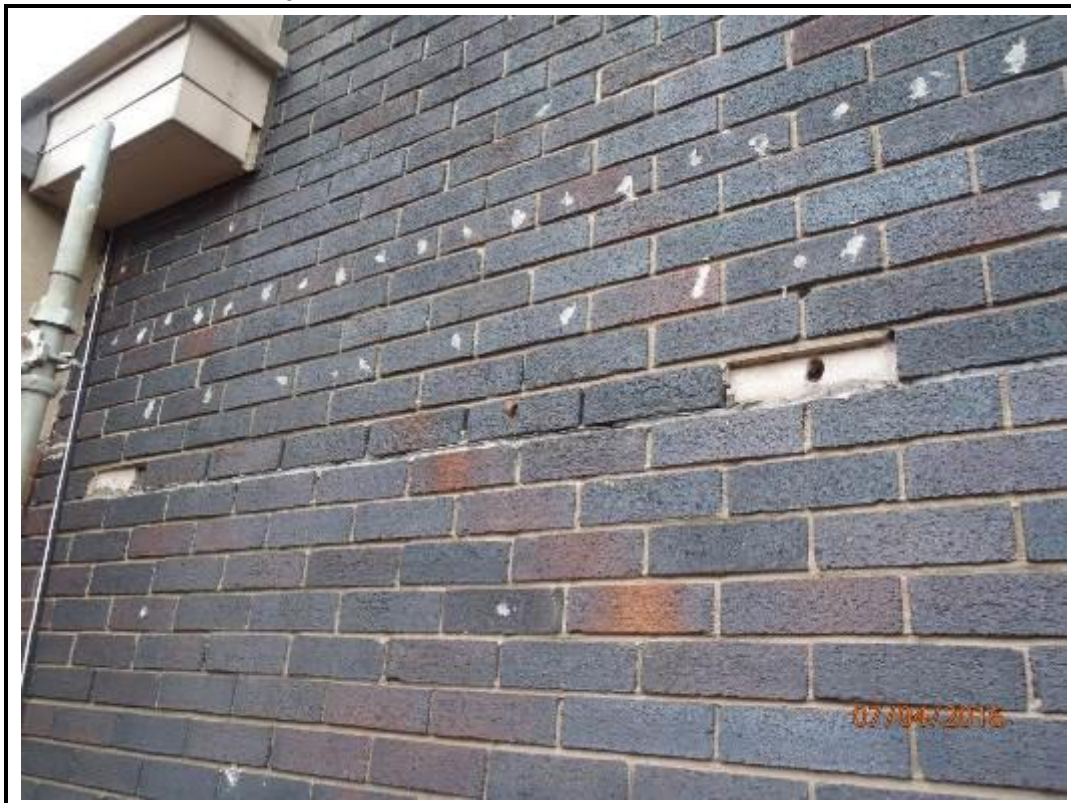
Photo 226. Drop 13 – West Elevation
