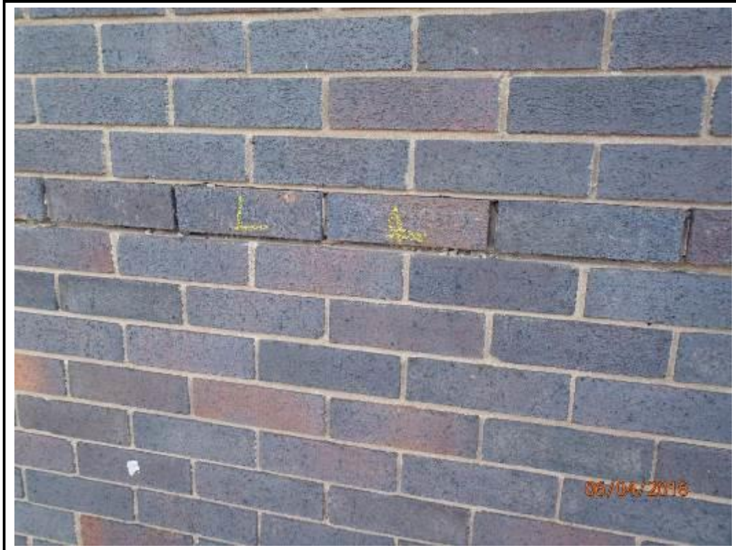
Photo 175. Drop 2 – West Elevation
