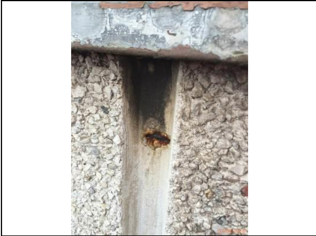
Photo 205. Drop 10 – West Elevation
