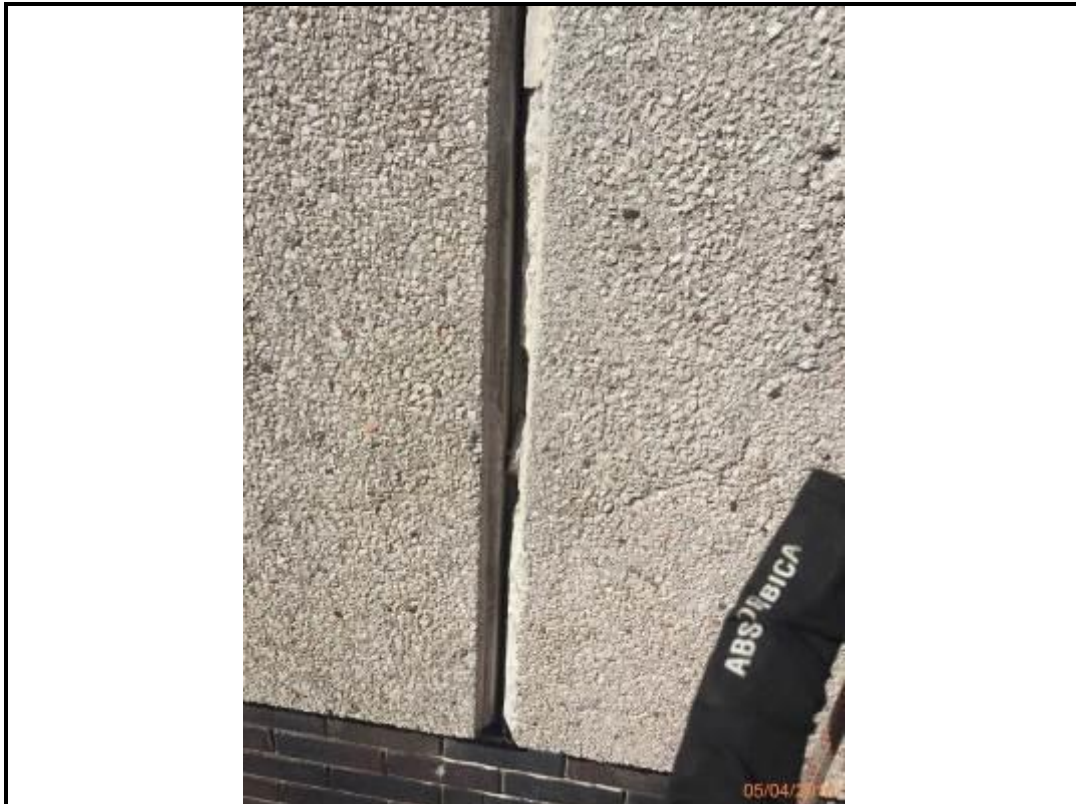
Photo 115. Drop 13 – South Elevation
