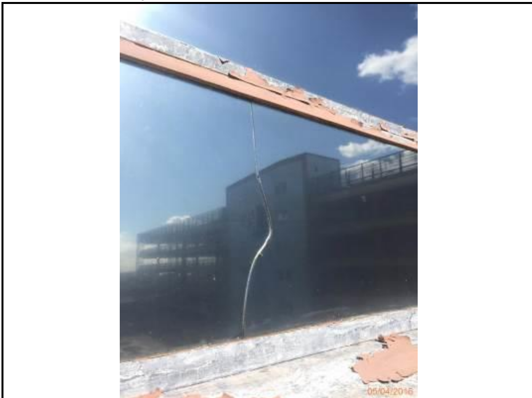
Photo 78. Drop 5 – South Elevation
