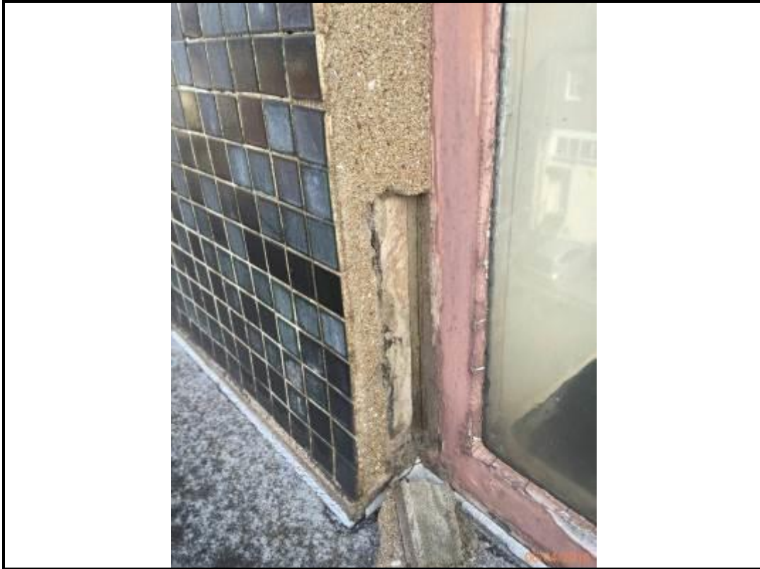
Photo 189. Drop 5 – West Elevation
