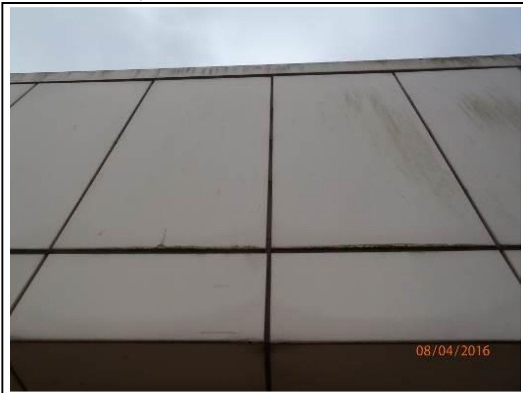
Photo 248. Drop 7 – North Elevation
