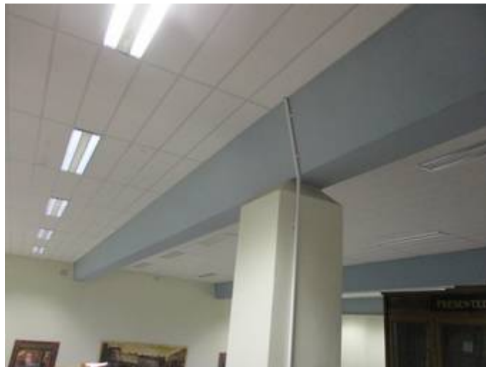
2 – Typical insitu cast concrete construction within the property.
