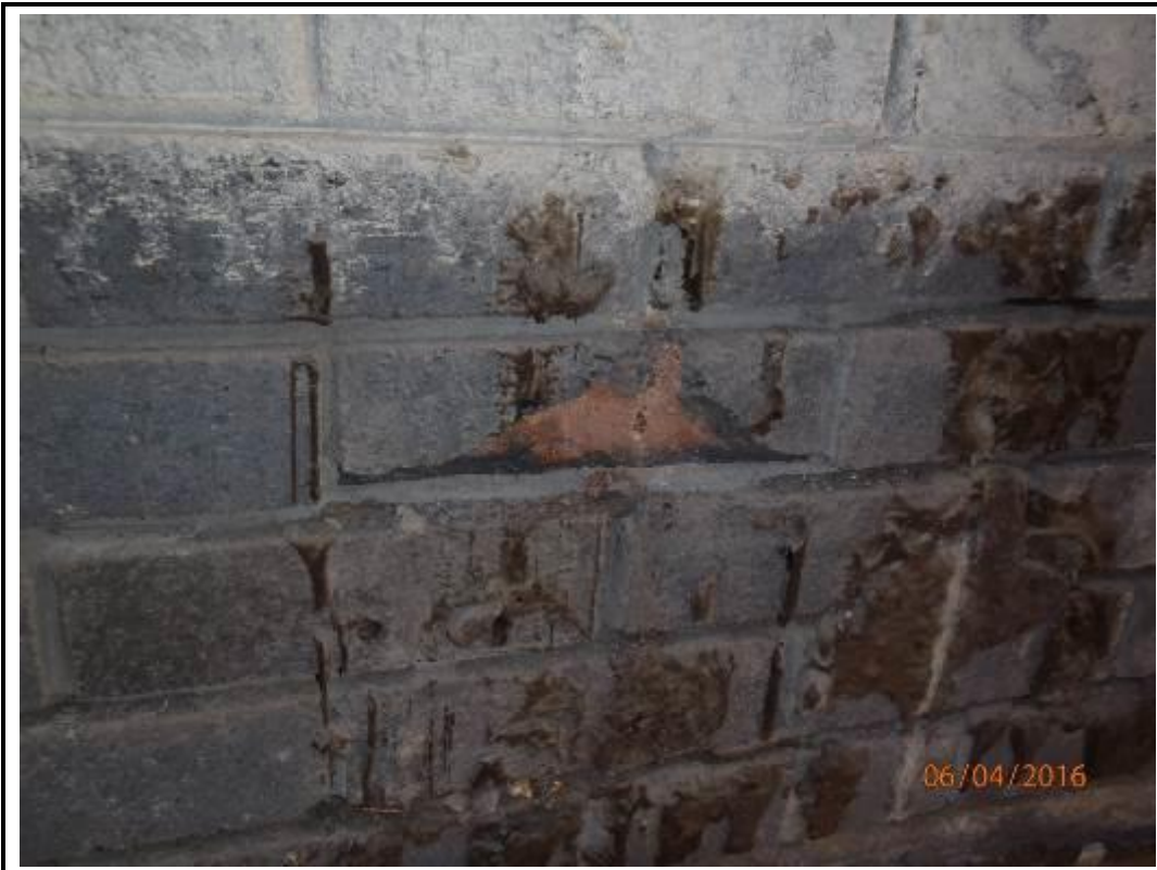
Photo 154. East Elevation – Brickwork Cladding Beneath Overhang
