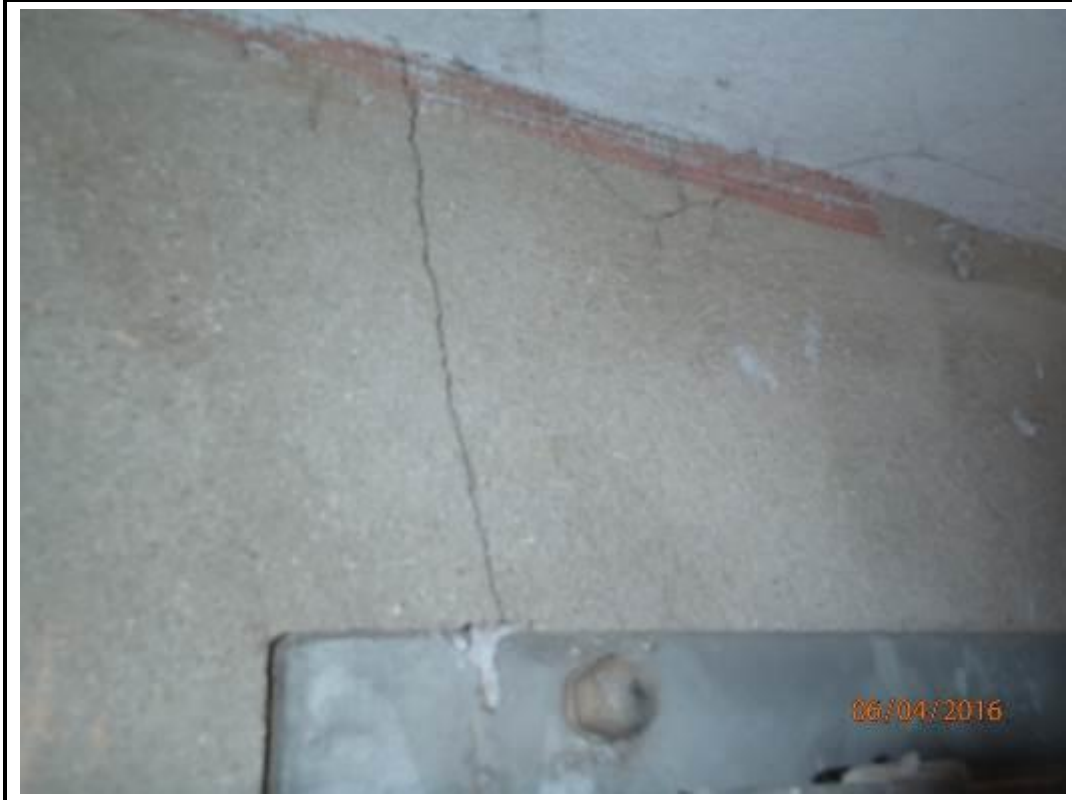
Photo 157. East Elevation – Brickwork Cladding Beneath Overhang
