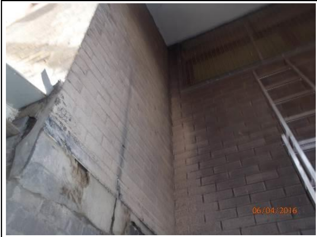
Photo 141. East Elevation – Brickwork Cladding Beneath Overhang
