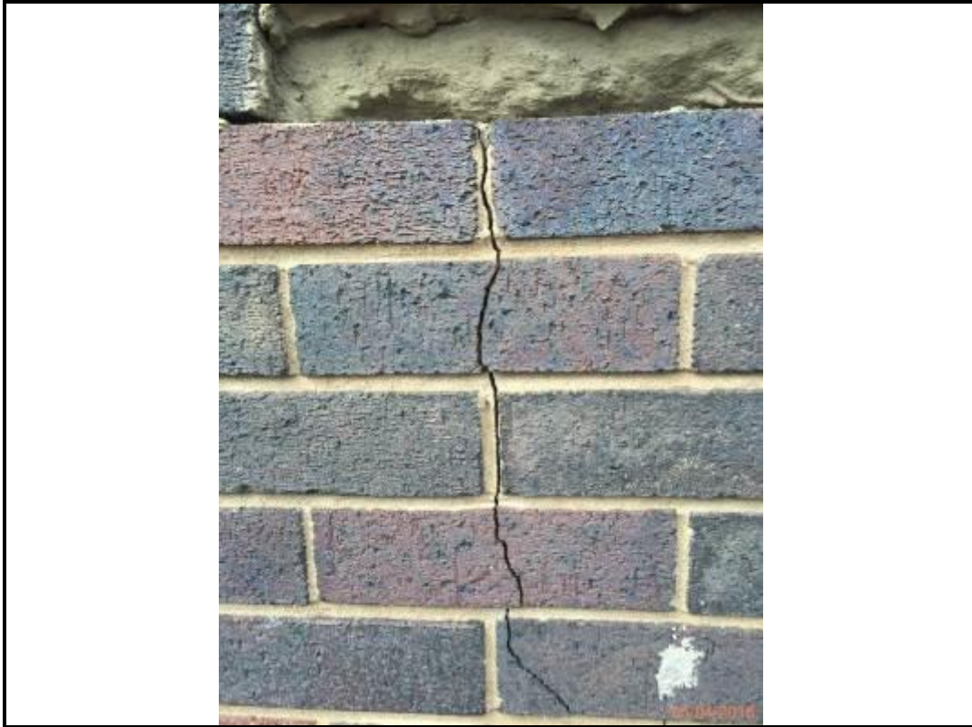
Photo 119. Drop 13 – South Elevation
