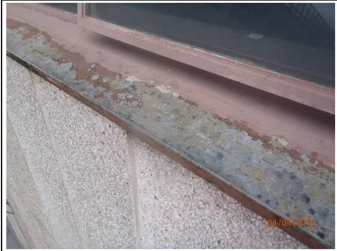
Photo 35. Drop 11 – East Elevation
