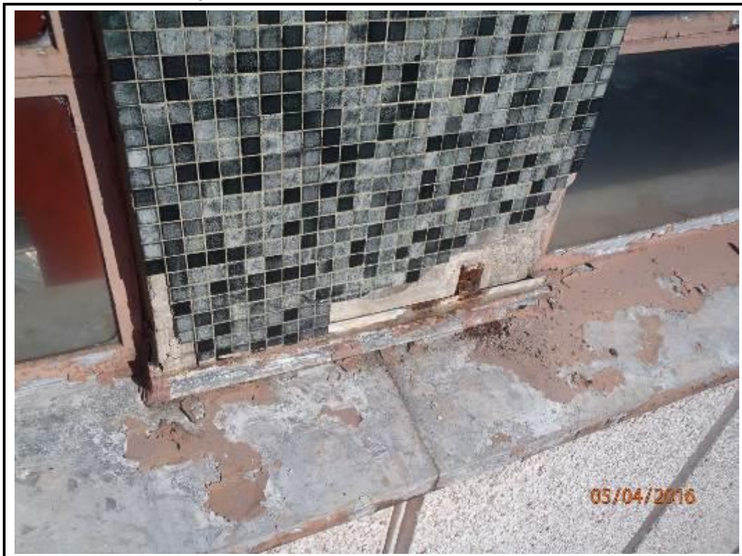
Photo 82. Drop 6 – South Elevation
