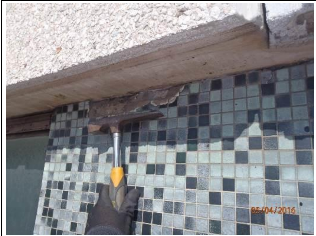
Photo 85. Drop 7 – South Elevation
