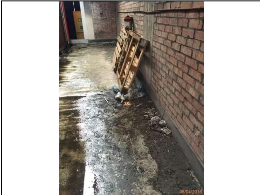
Photo 151. East Elevation – Brickwork Cladding Beneath Overhang
