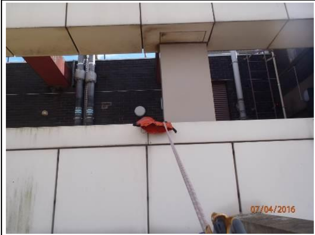
Photo 243. Drop 5 – North Elevation
