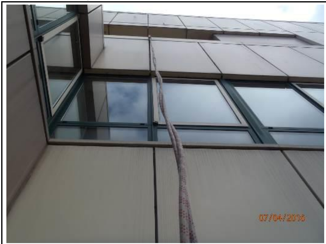
Photo 238. Drop 4 – North Elevation
