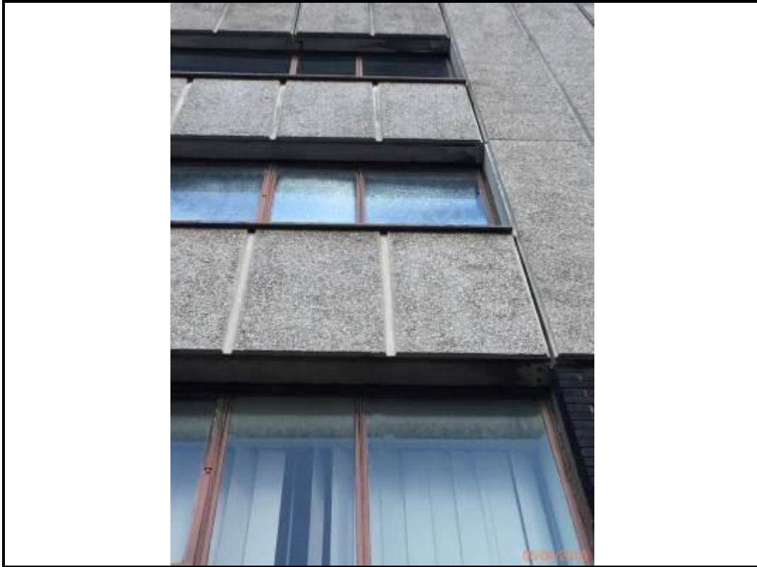
Photo 67. Drop 2 – South Elevation
