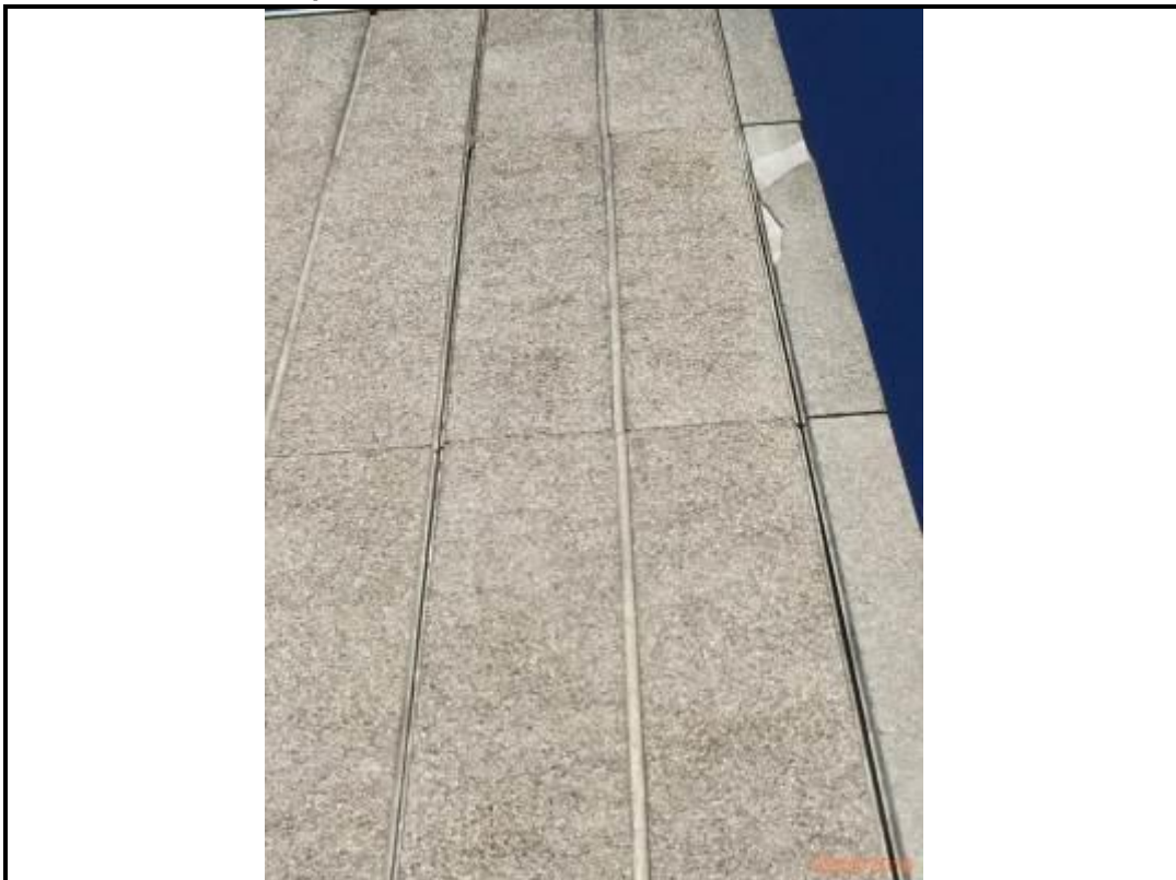
Photo 58. Drop 1 – South Elevation
