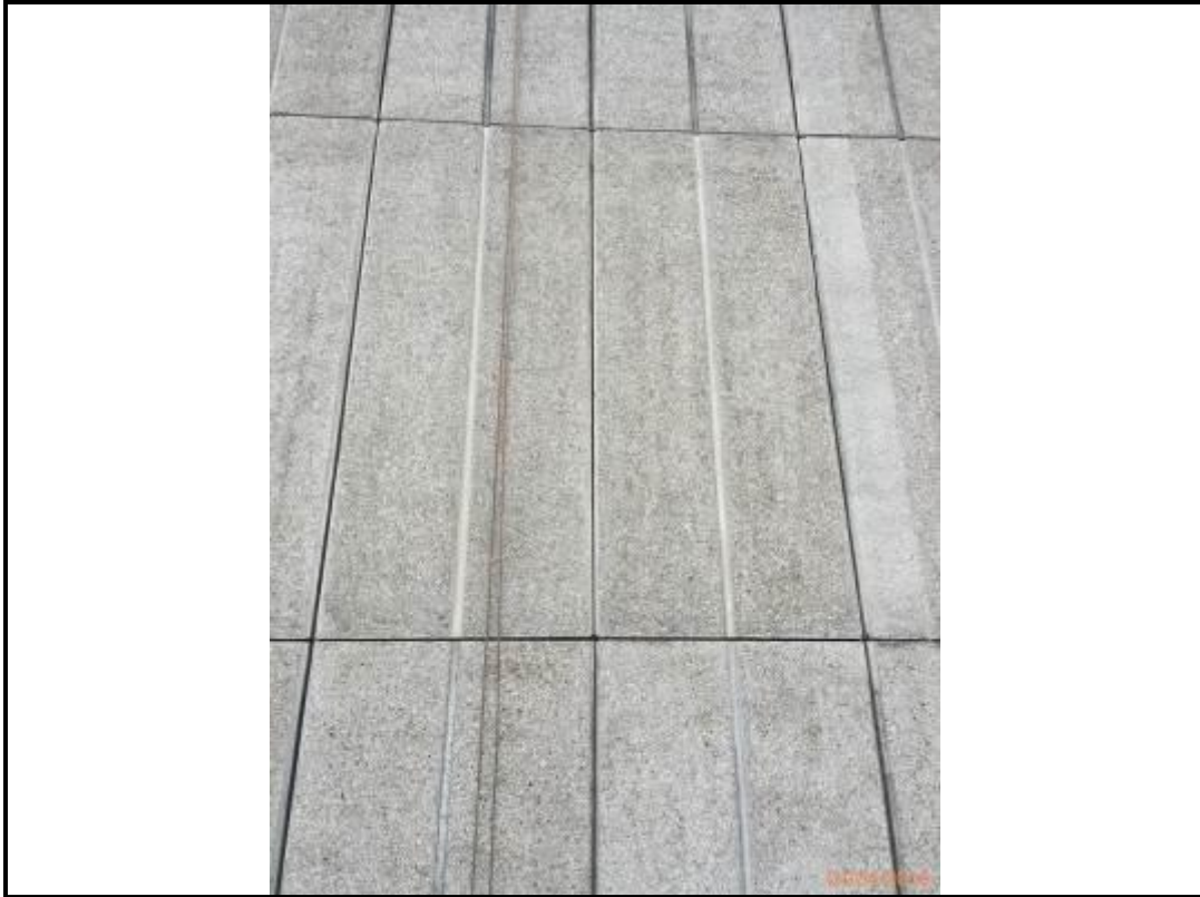
Photo 29. Drop 9 – East Elevation
