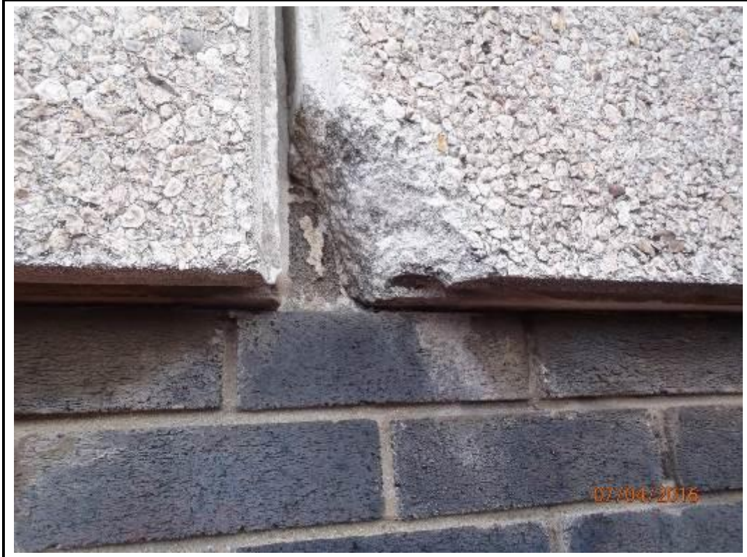
Photo 219. Drop 12 – West Elevation
