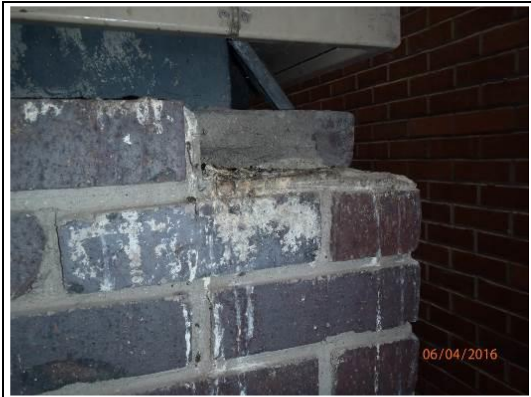
Photo 164. East Elevation – Brickwork Cladding Beneath Overhang
