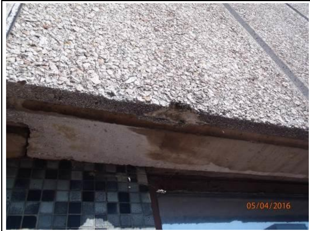
Photo 81. Drop 6 –South Elevation
