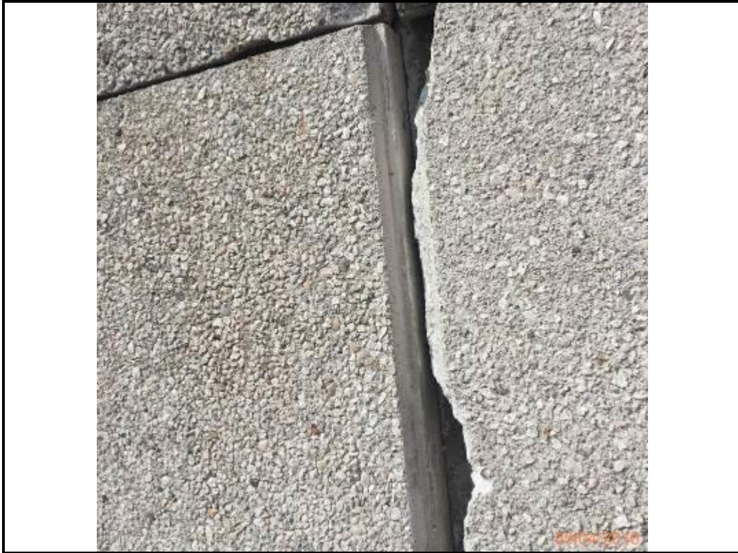
Photo 113. Drop 13 – South Elevation
