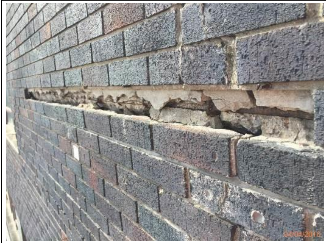
Photo 51. Drop 1 – South Elevation
