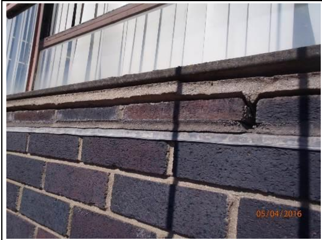
Photo 97. Drop 9 – South Elevation
