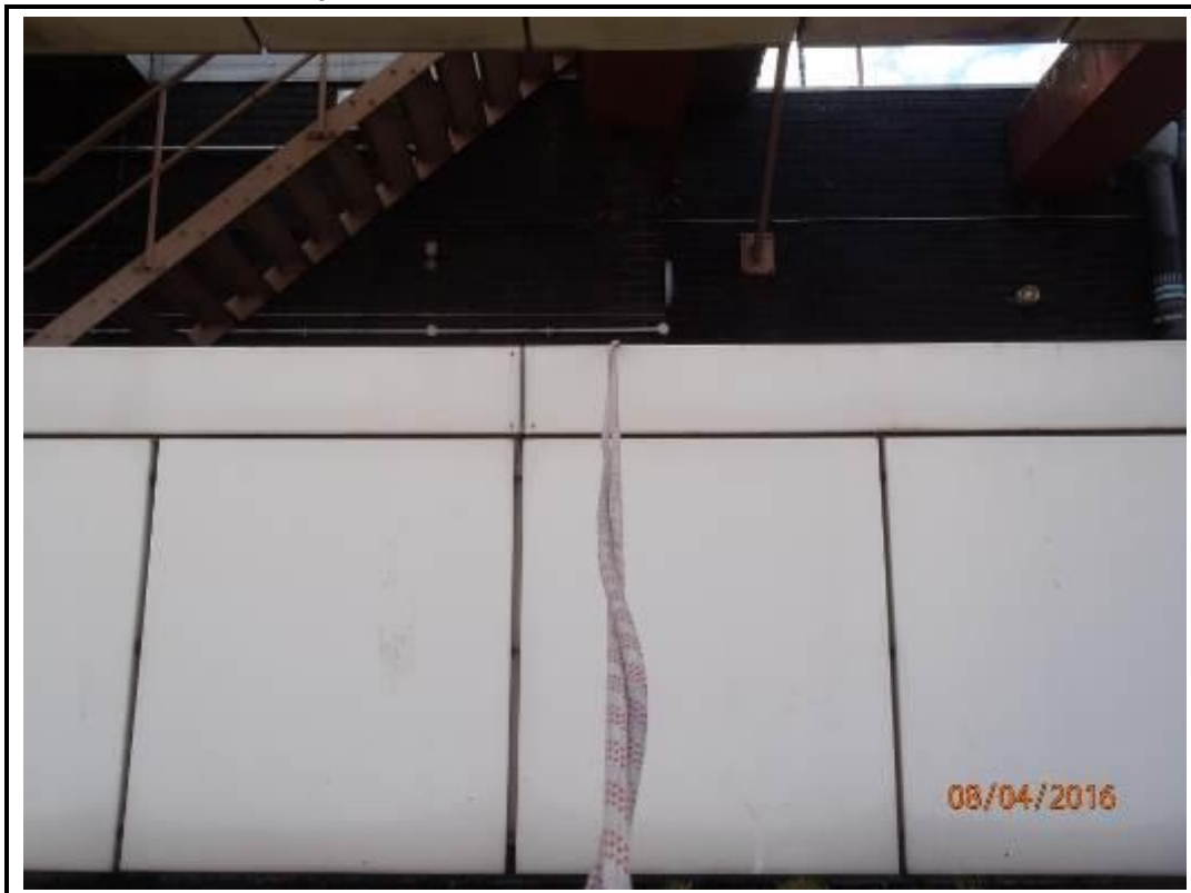
Photo 252. Drop 8 – North Elevation
