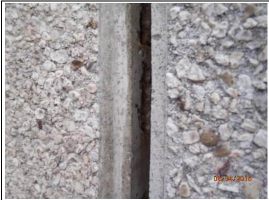
Photo 174. Drop 2 – West Elevation
