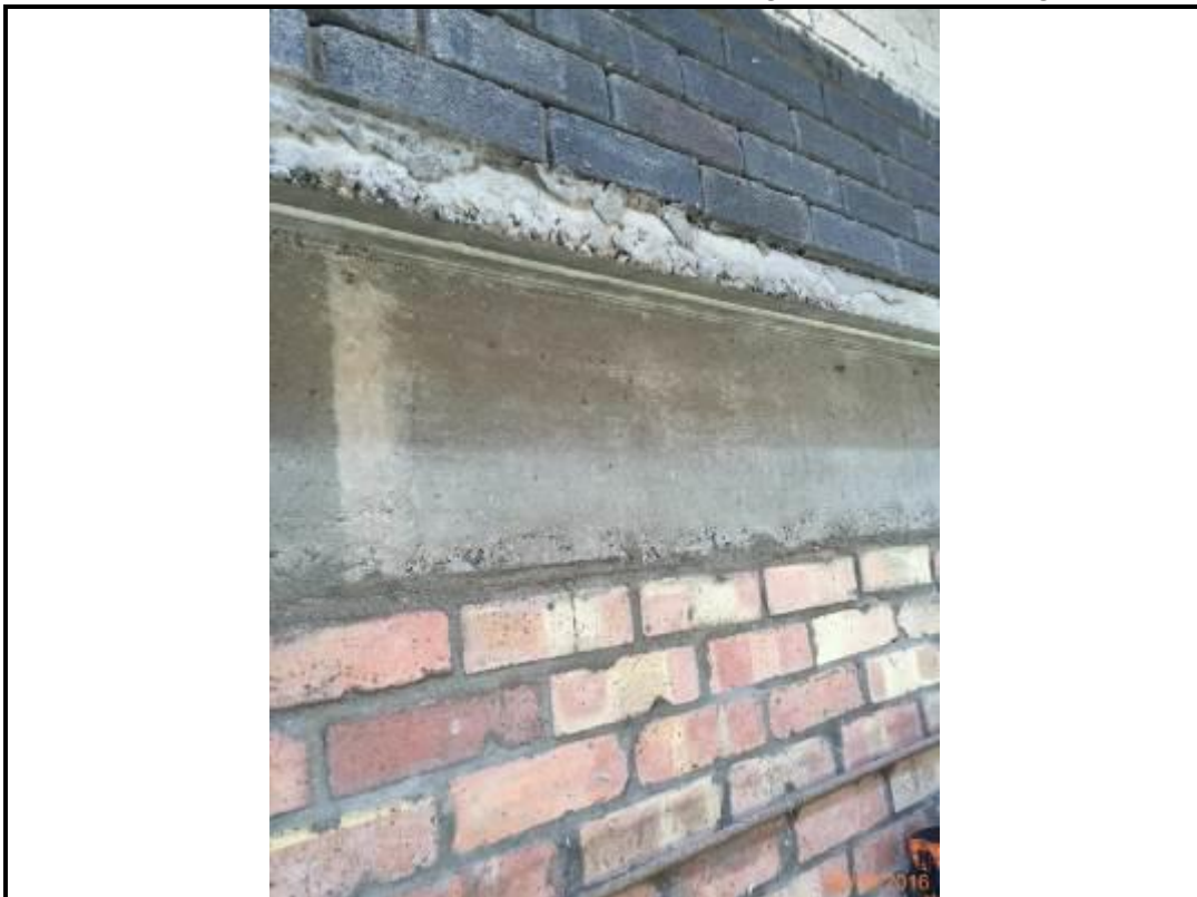
Photo 146. East Elevation – Brickwork Cladding Beneath Overhang
