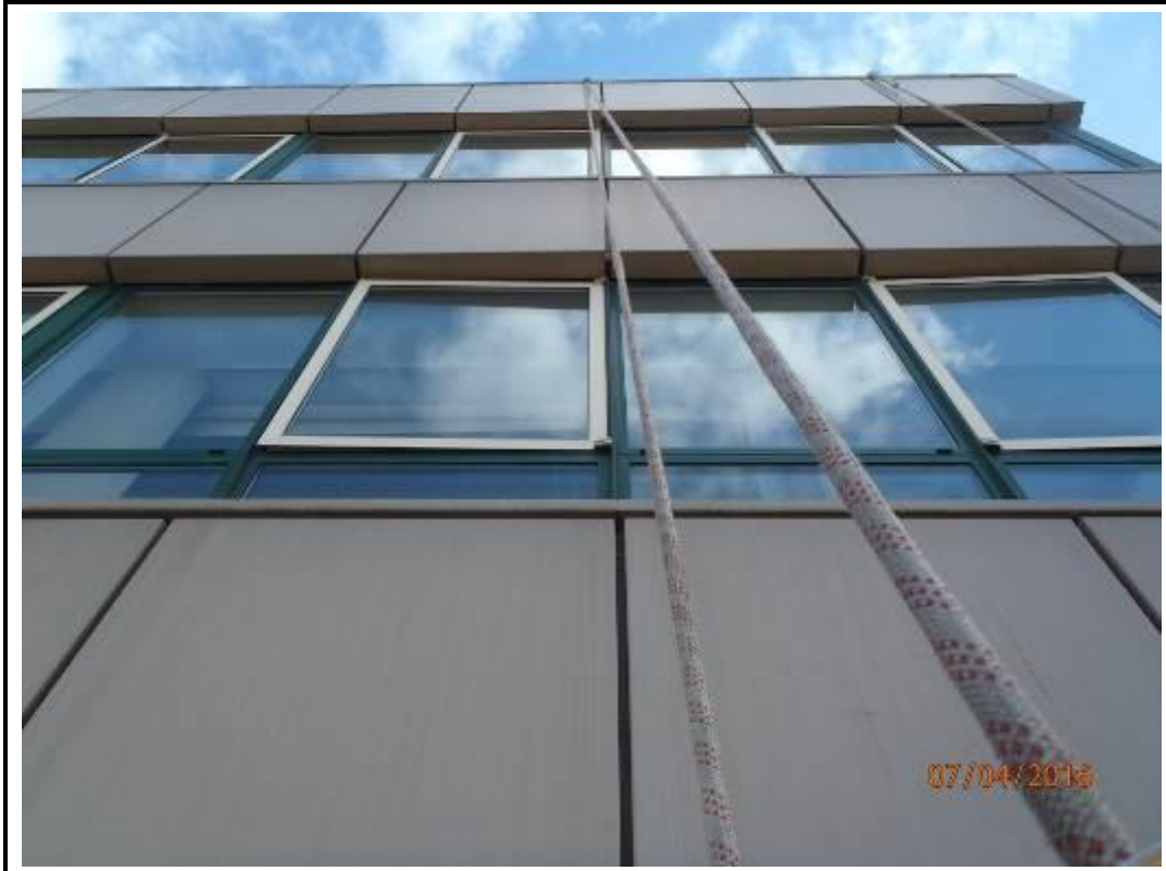
Photo 245. Drop 6 – North Elevation
