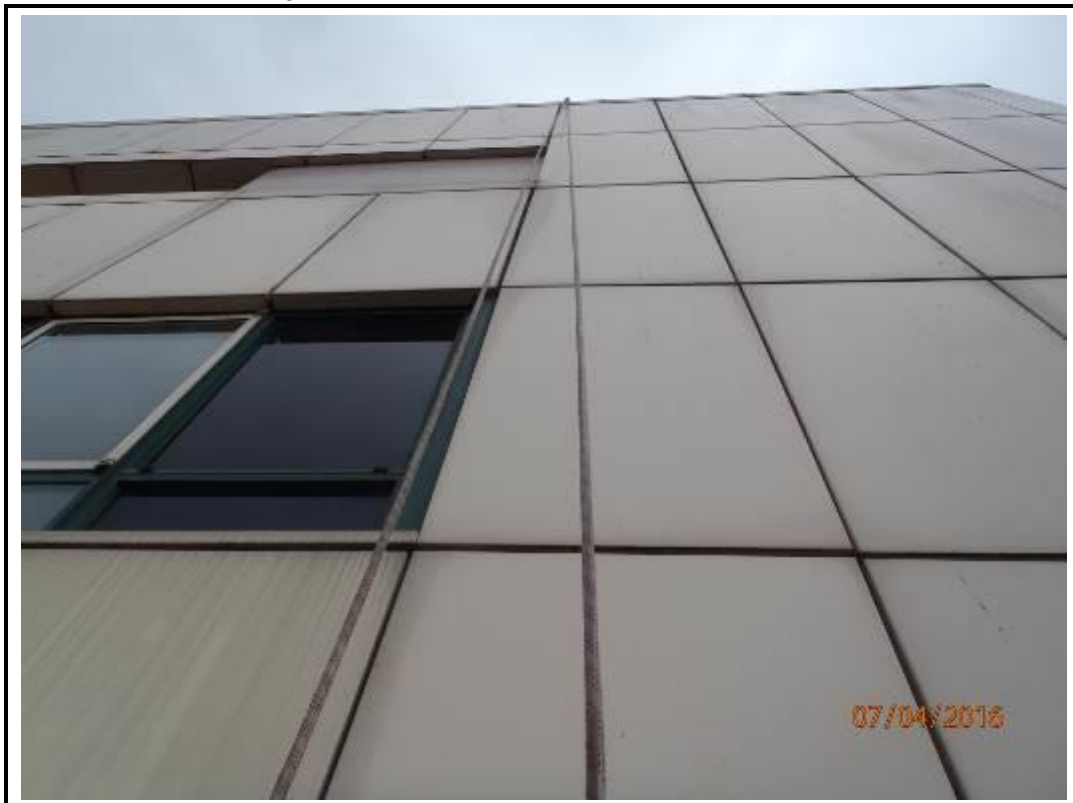
Photo 232. Drop 2 – North Elevation
