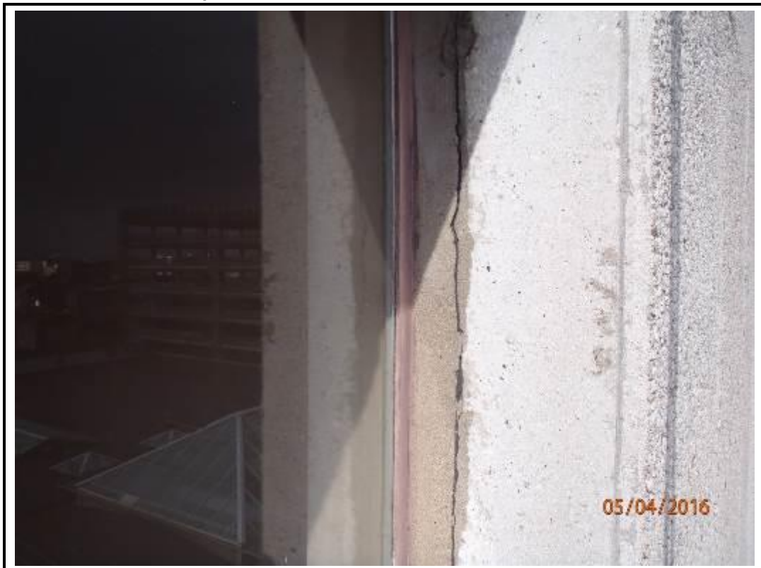
Photo 122. Drop 14 – South Elevation
