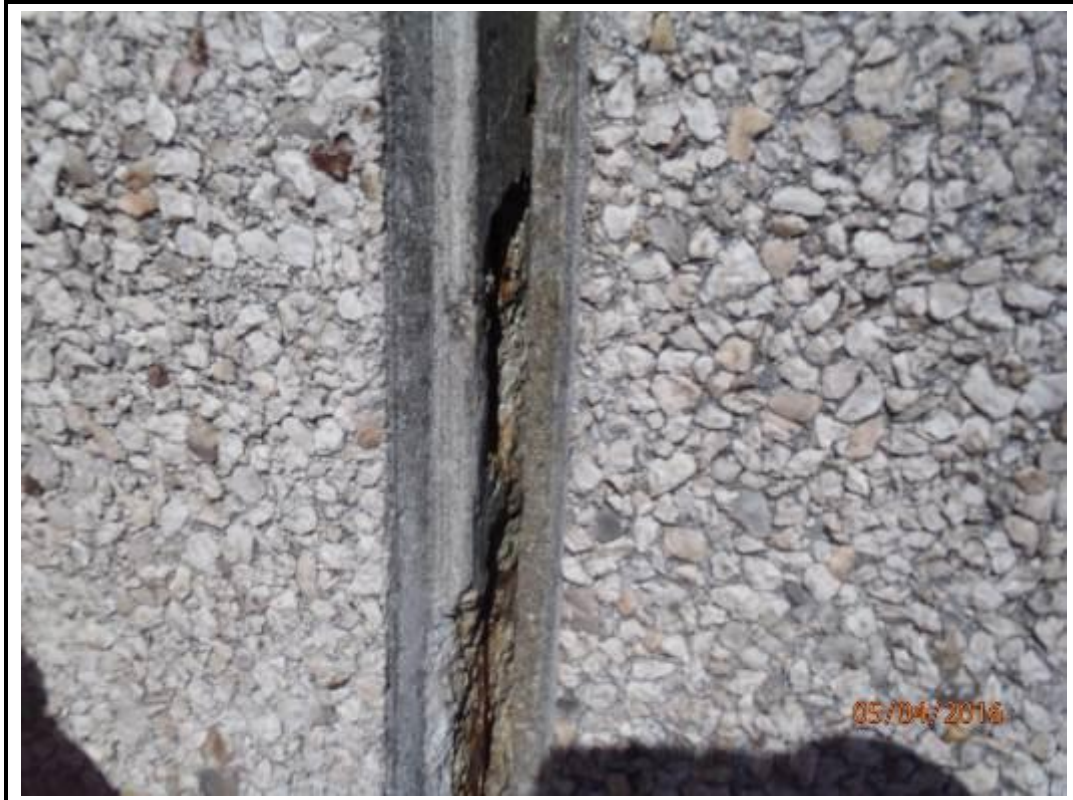
Photo 89. Drop 8 – South Elevation
