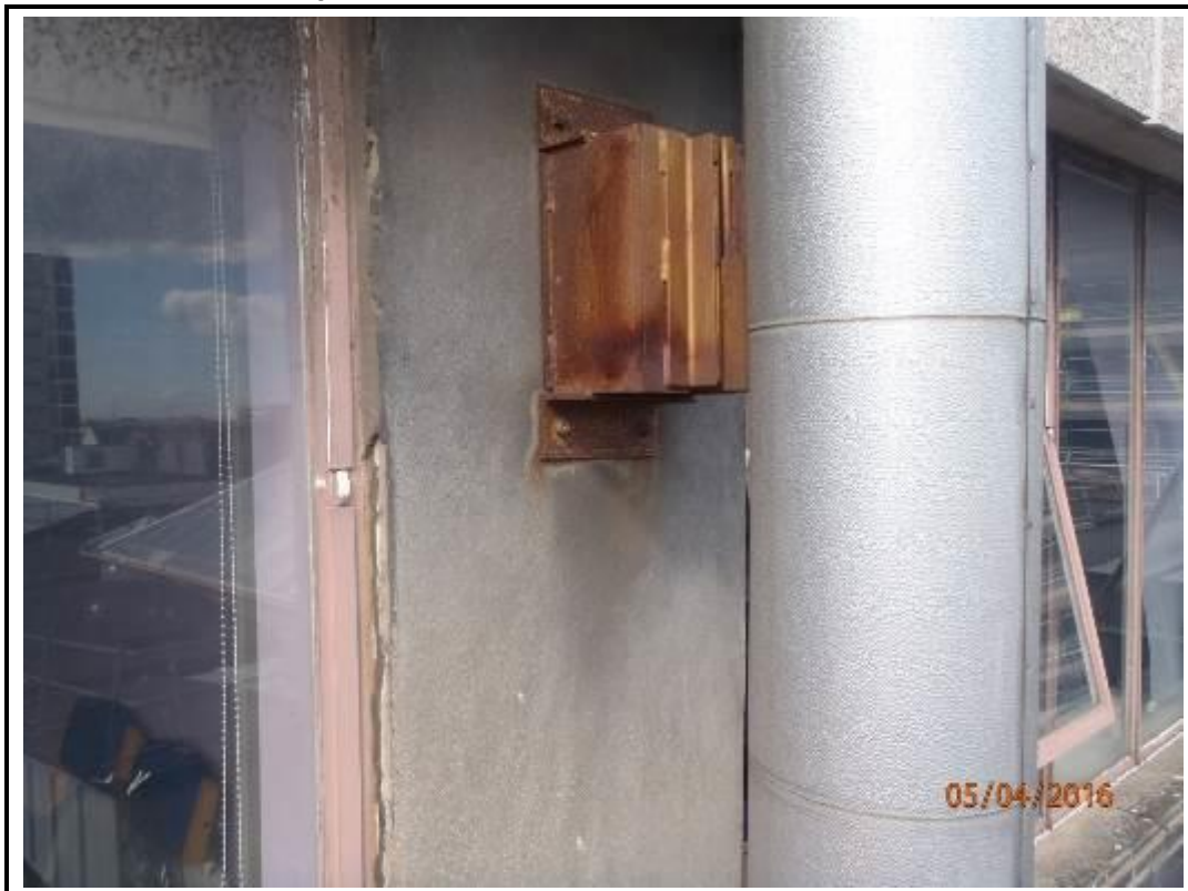
Photo 106. Drop 12 – South Elevation
