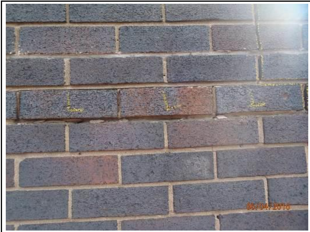
Photo 168. Drop 1 – West Elevation
