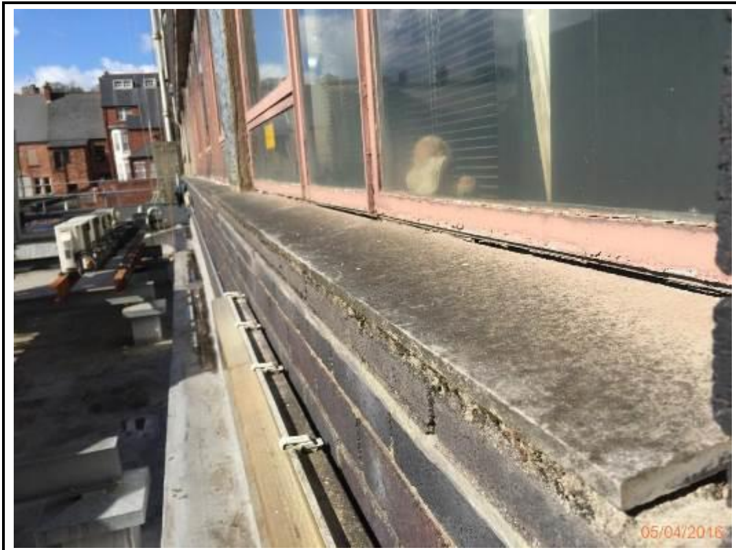
Photo 66. Drop 2 – South Elevation
