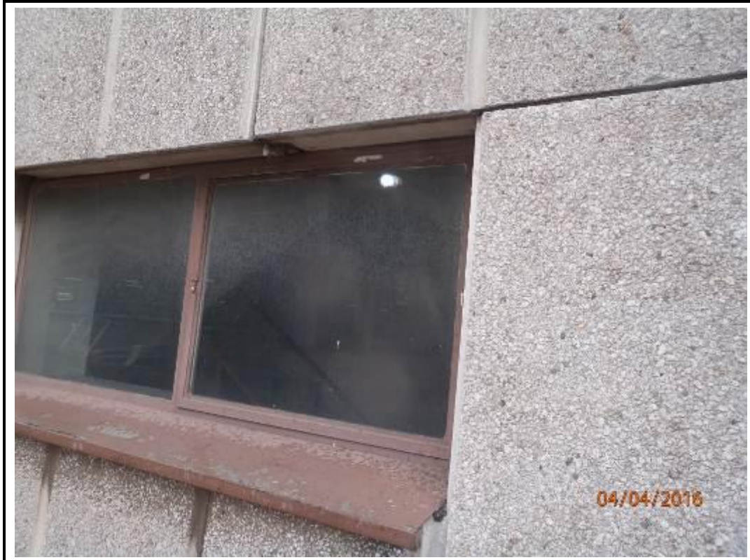
Photo 33. Drop 11 – East Elevation
