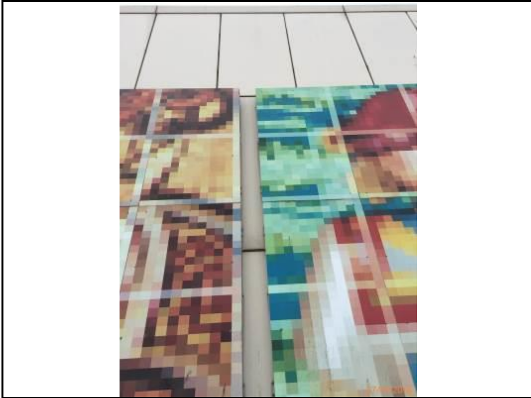
Photo 271. Drop 17 – North Elevation
