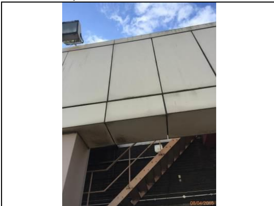
Photo 254. Drop 9 – North Elevation
