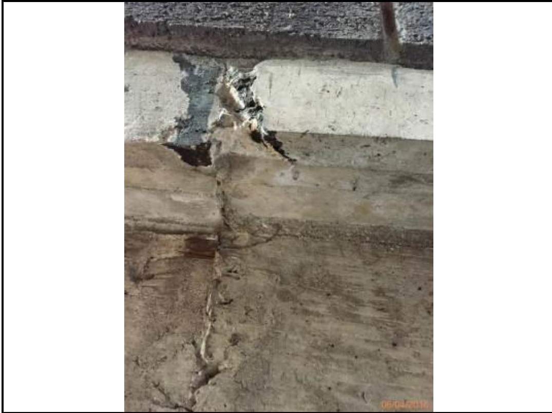
Photo 147. East Elevation – Brickwork Cladding Beneath Overhang
