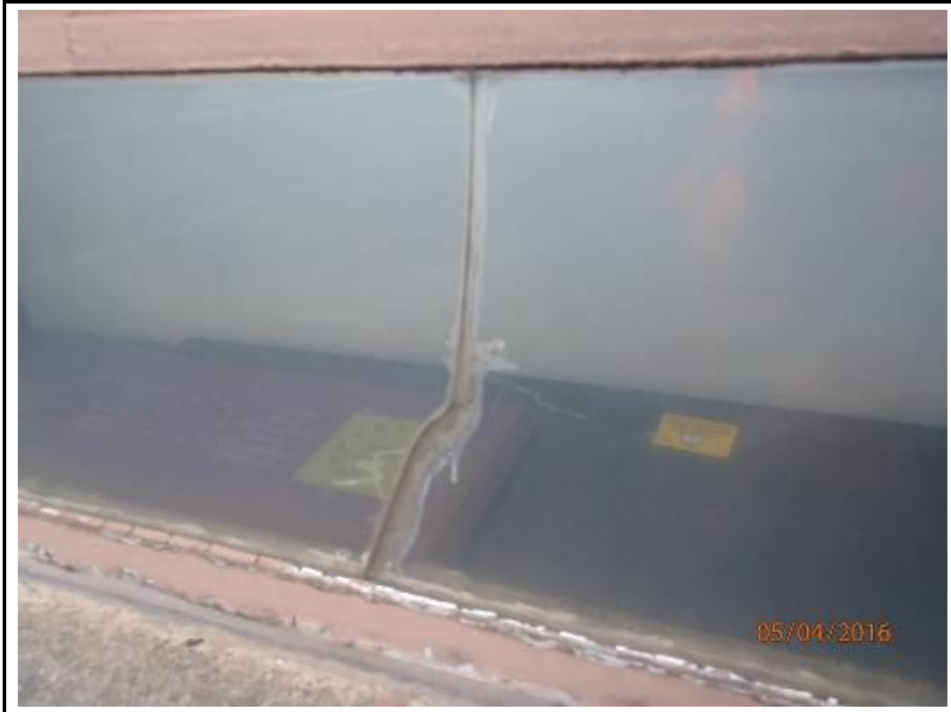
Photo 101. Drop 10 – South Elevation
