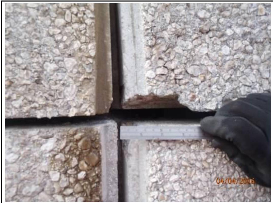
Photo 10. Drop 2 – East Elevation
