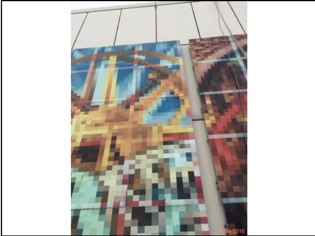
Photo 273. Drop 19 – North Elevation
