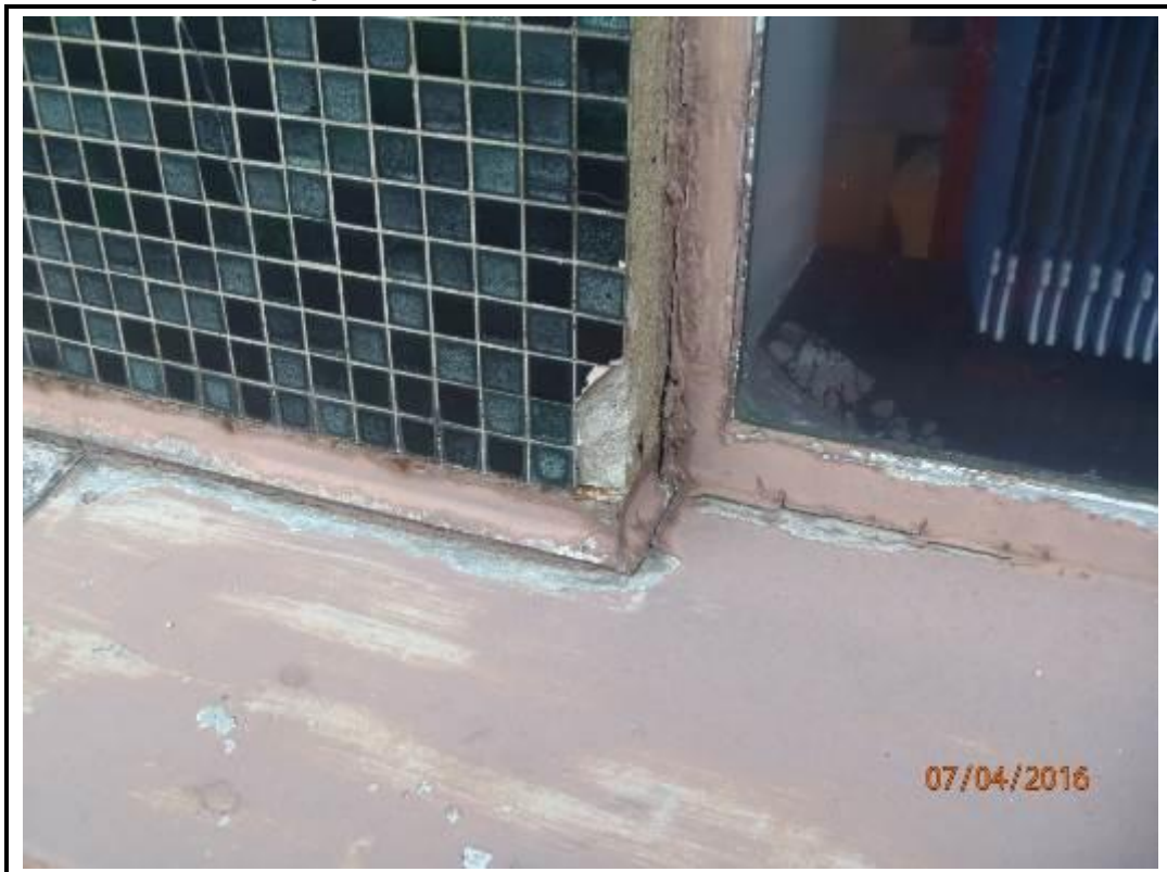
Photo 202. Drop 9 – West Elevation
