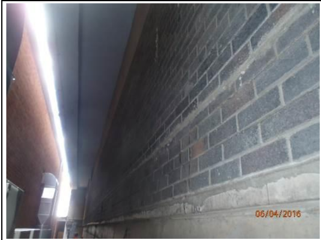
Photo 143. East Elevation – Brickwork Cladding Beneath Overhang
