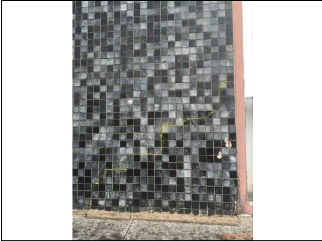
Photo 197. Drop 7 – West Elevation
