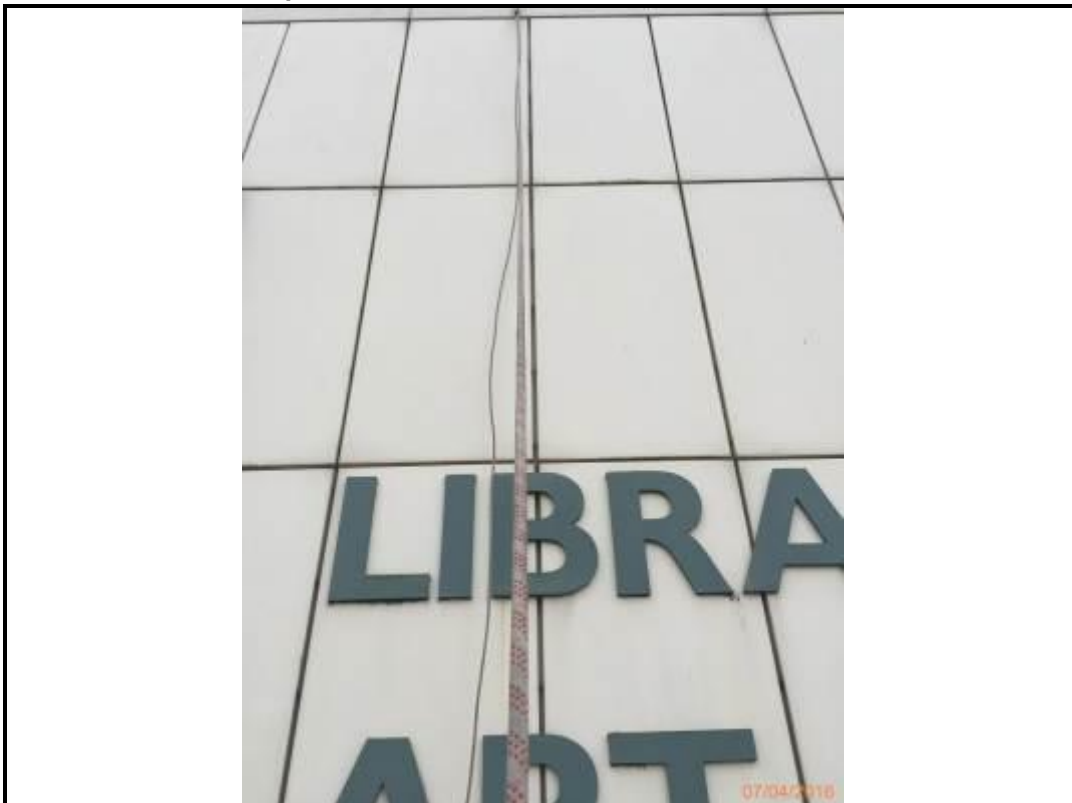
Photo 268. Drop 14 – North Elevation
