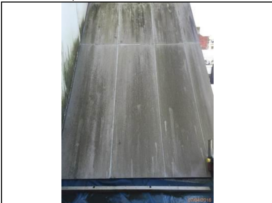
Photo 258. Drop 10 – North Elevation
