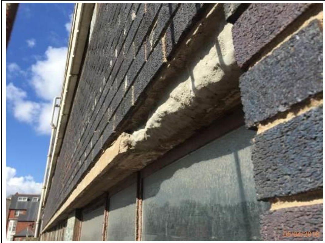
Photo 65. Drop 2 – South Elevation
