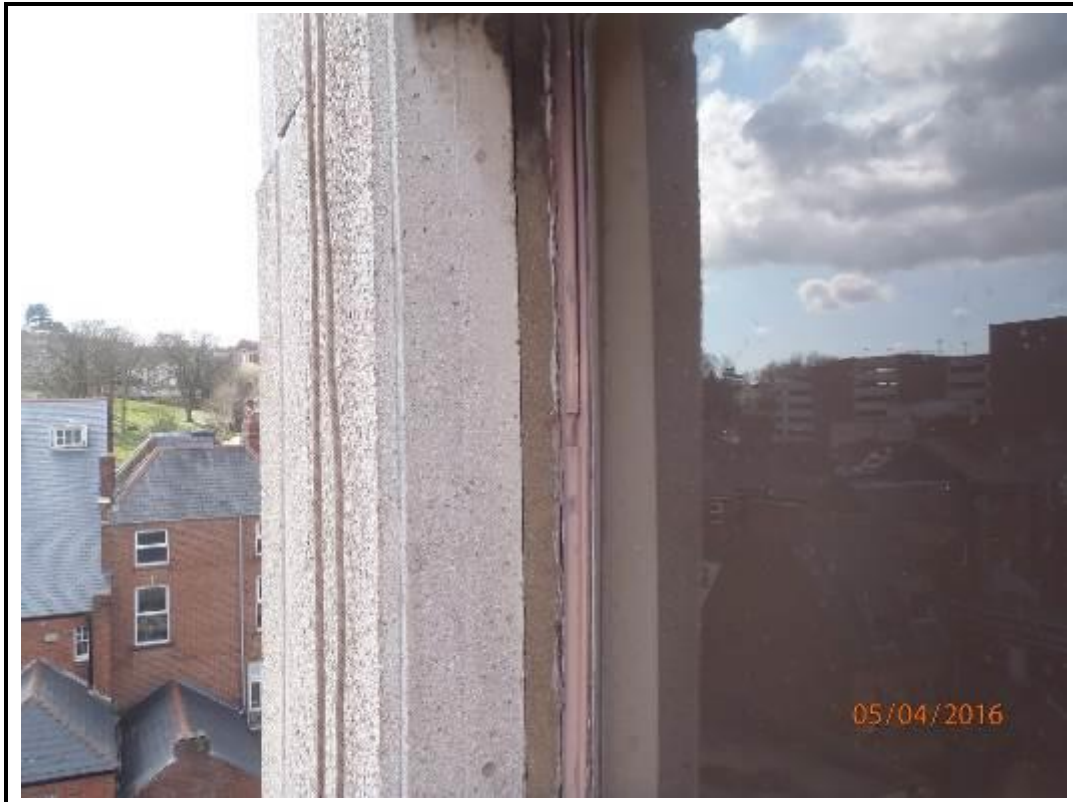
Photo 123. Drop 14 – South Elevation
