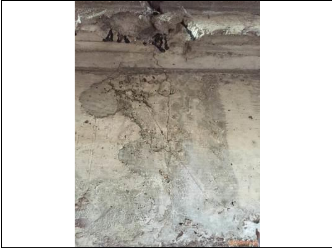
Photo 149. East Elevation – Brickwork Cladding Beneath Overhang
