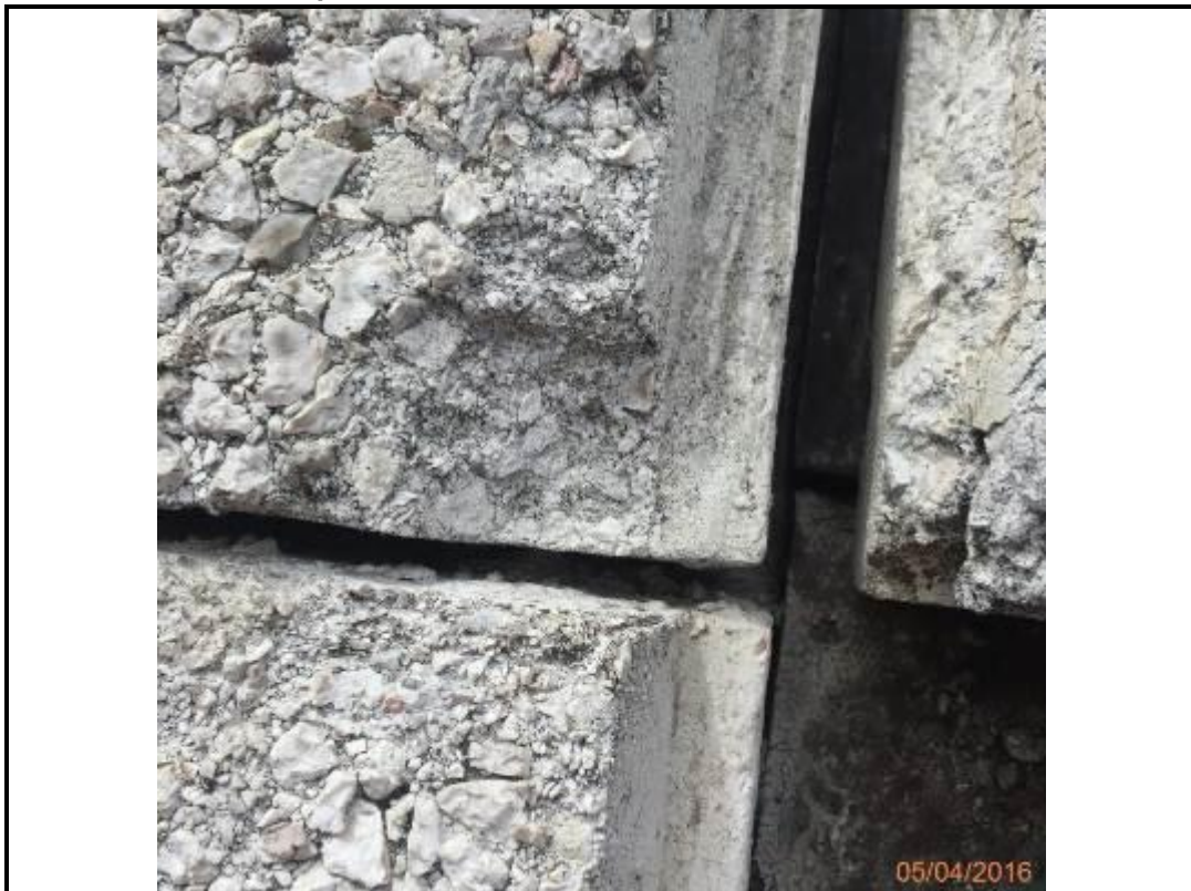
Photo 112. Drop 13 – South Elevation
