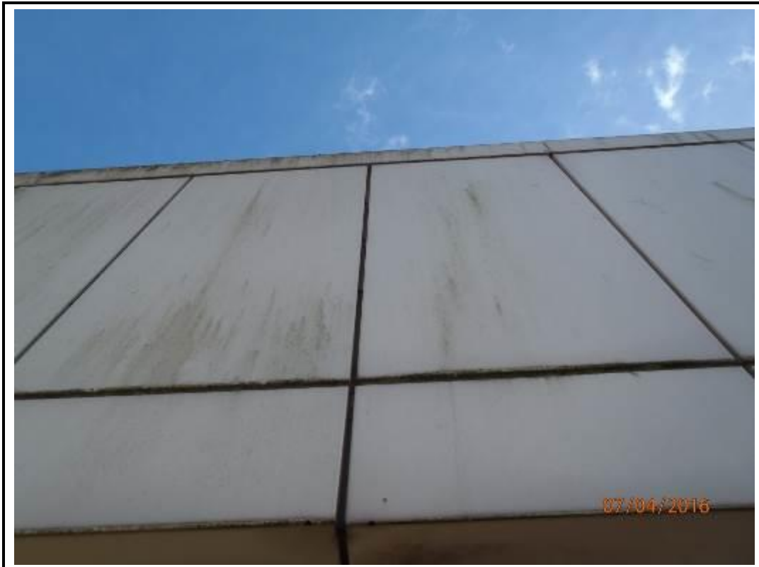
Photo 242. Drop 5 – North Elevation
