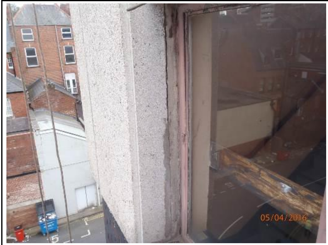
Photo 129. Drop 14 – South Elevation
