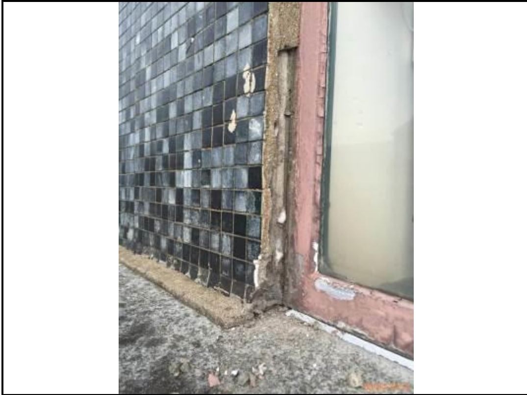
Photo 195. Drop 7 – West Elevation
