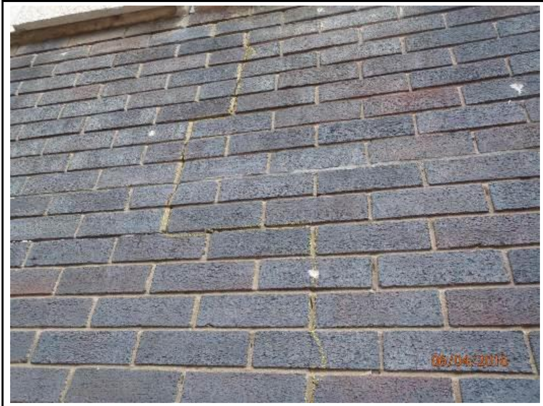
Photo 167. Drop 1 – West Elevation
