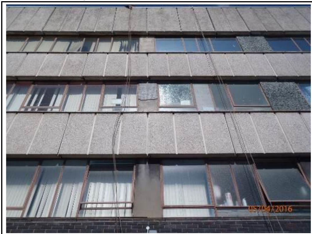
Photo 98. Drop 9 – South Elevation
