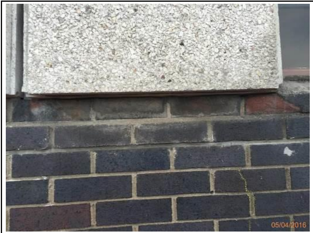
Photo 138. Drop 15 – South Elevation
