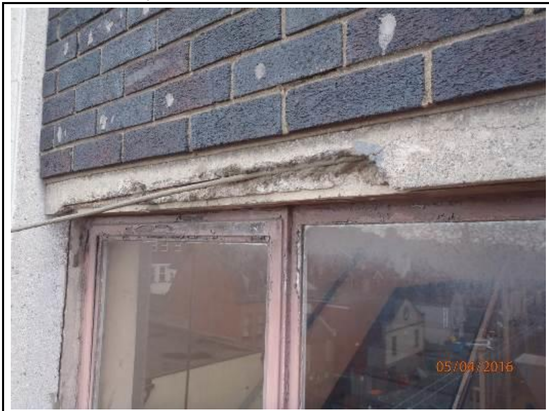
Photo 130. Drop 14 – South Elevation
