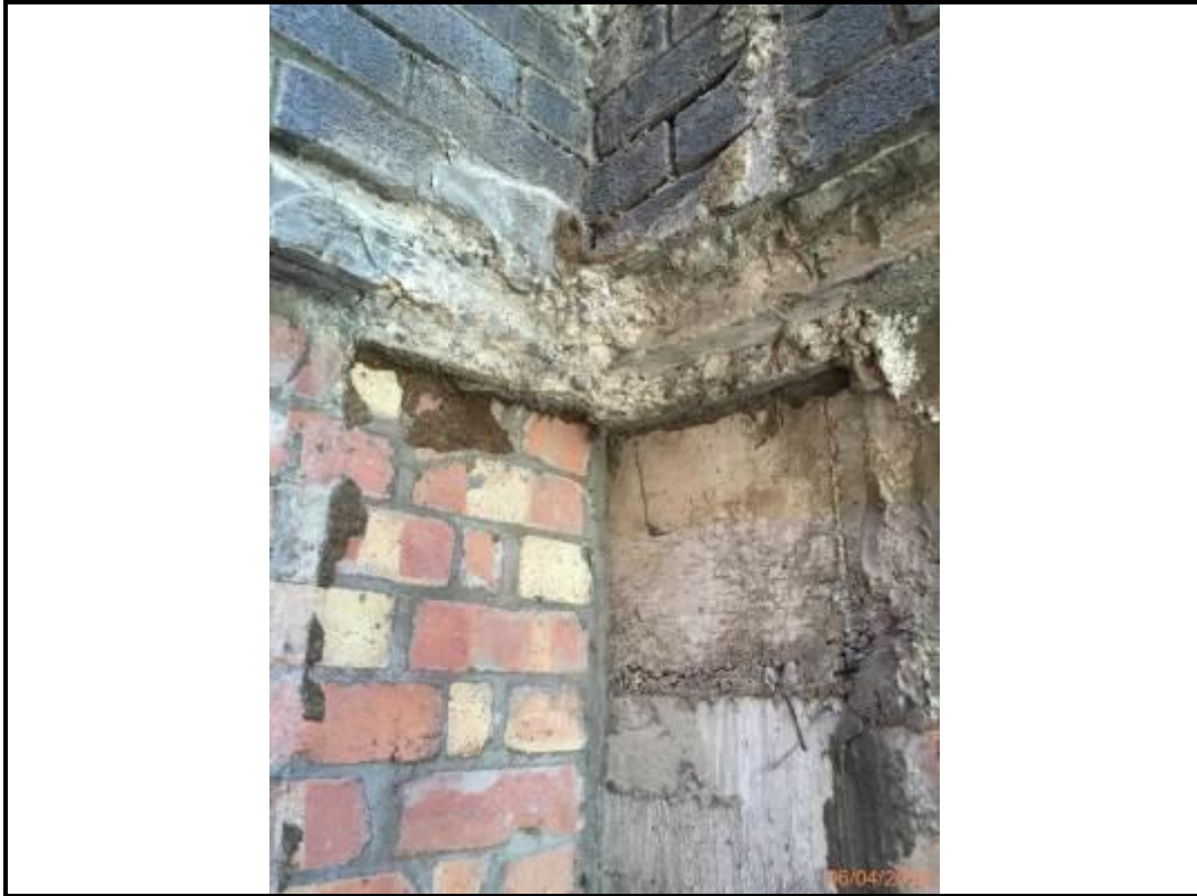
Photo 145. East Elevation – Brickwork Cladding Beneath Overhang
