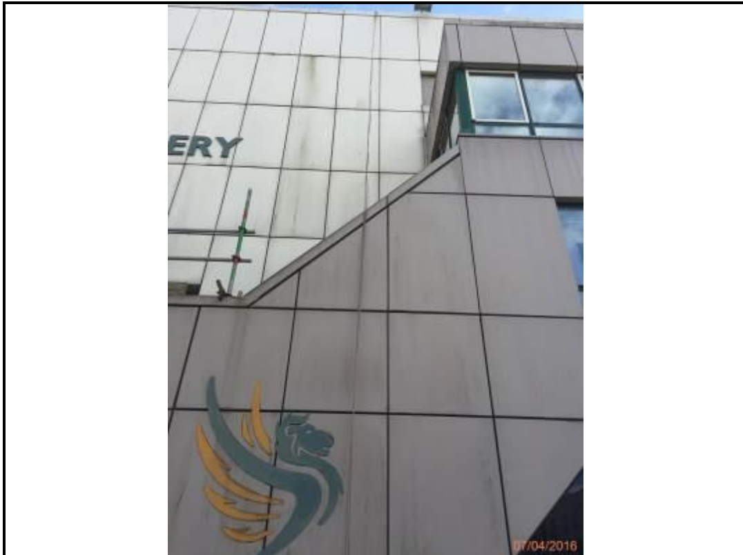
Photo 257. Drop 10 – North Elevation
