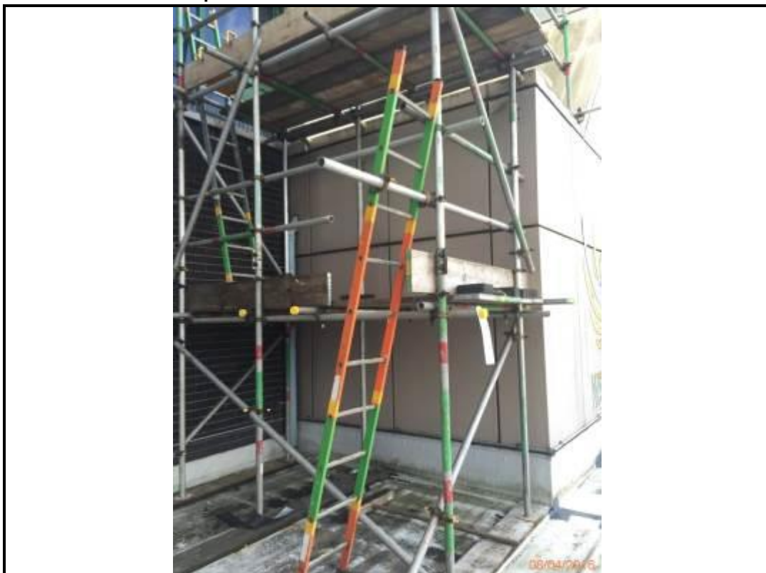
Photo 260. Drop 11 – North Elevation
