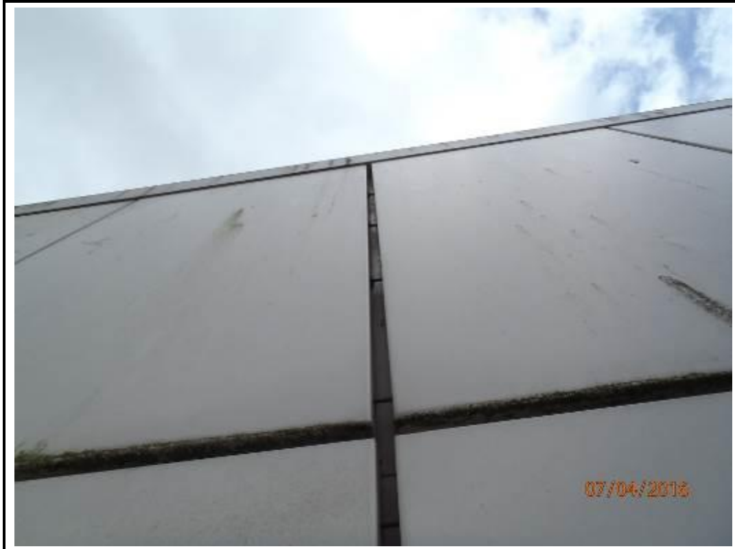
Photo 239. Drop 4 – North Elevation
