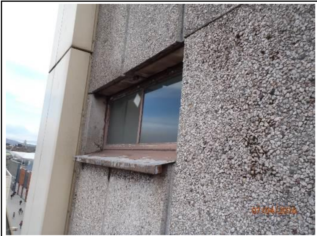
Photo 222. Drop 13 – West Elevation
