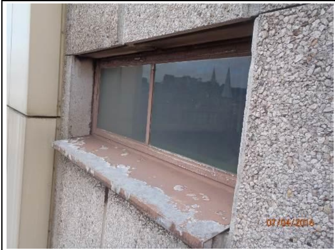
Photo 223. Drop 13 – West Elevation
