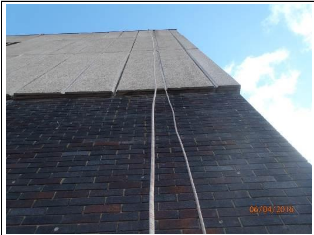
Photo 173. Drop 1 – West Elevation
