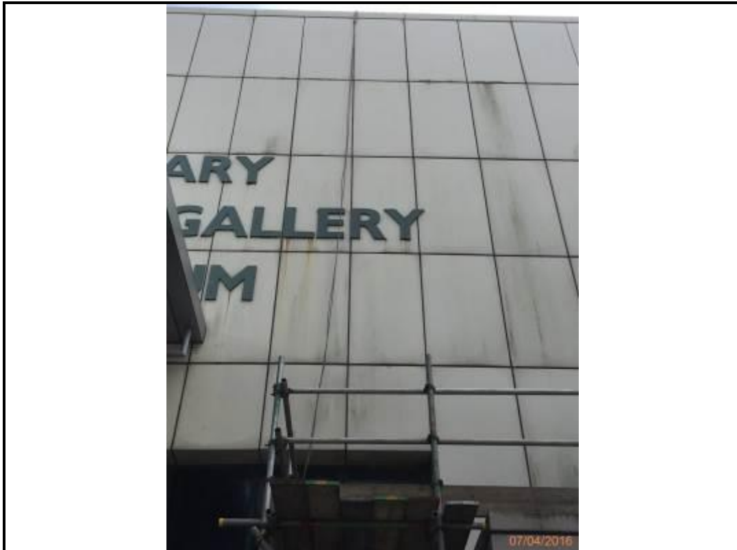
Photo 261. Drop 12 – North Elevation
