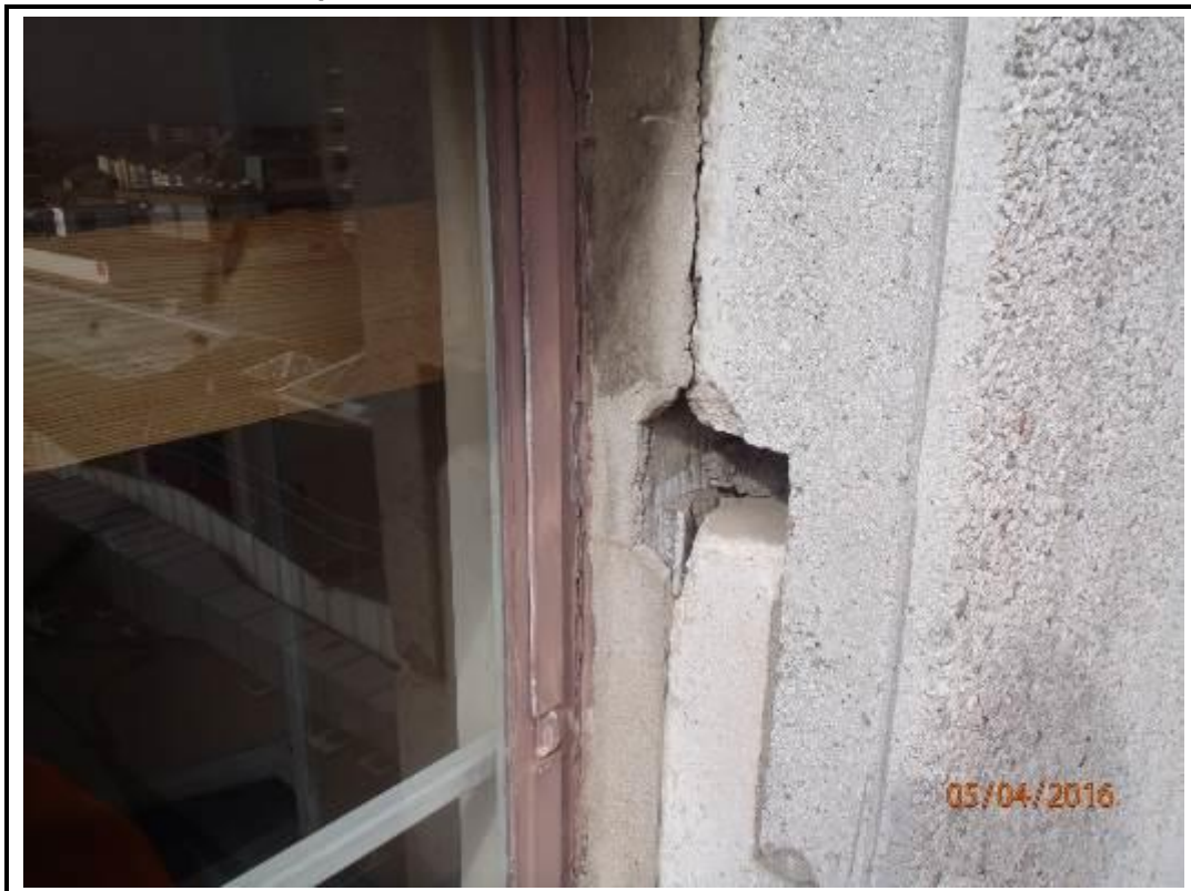
Photo 124. Drop 14 – South Elevation
