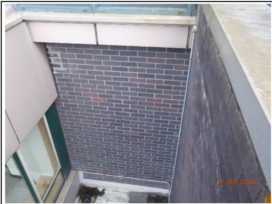
Photo 230. Drop 1 – North Elevation
