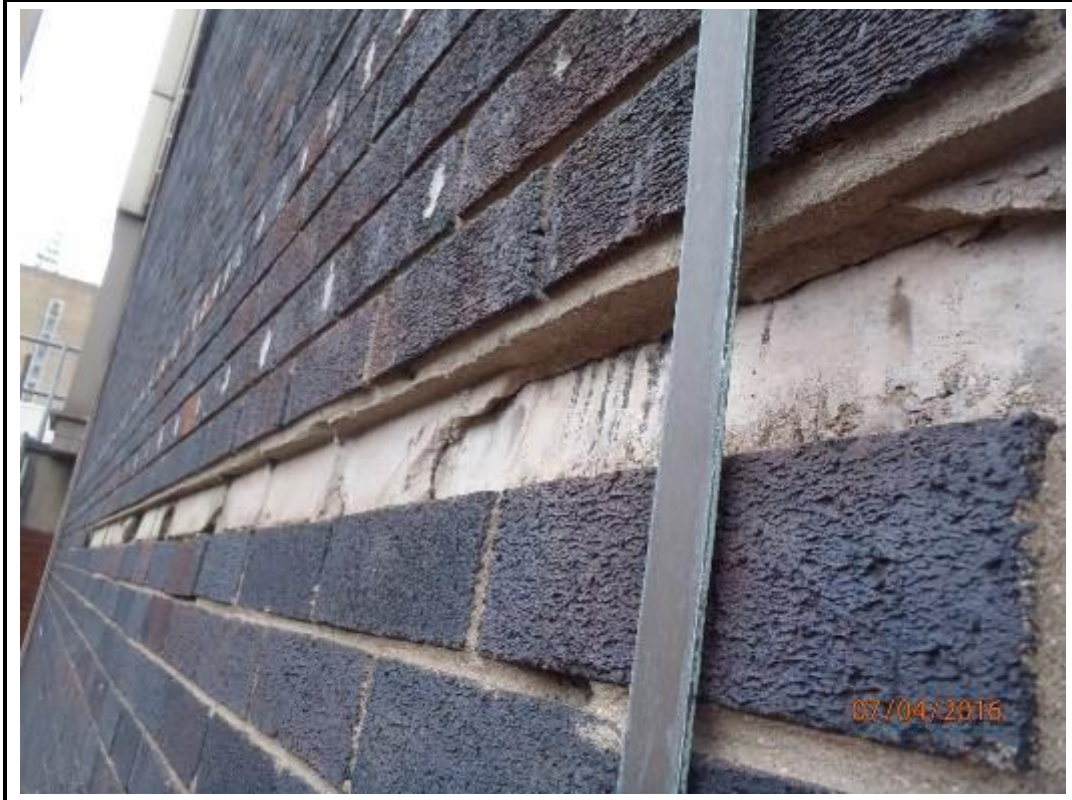
Photo 211. Drop 11 – West Elevation
