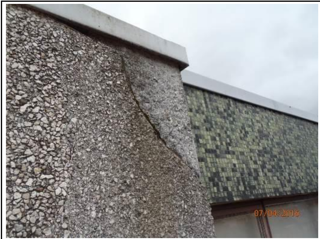
Photo 218. Drop 12 – West Elevation
