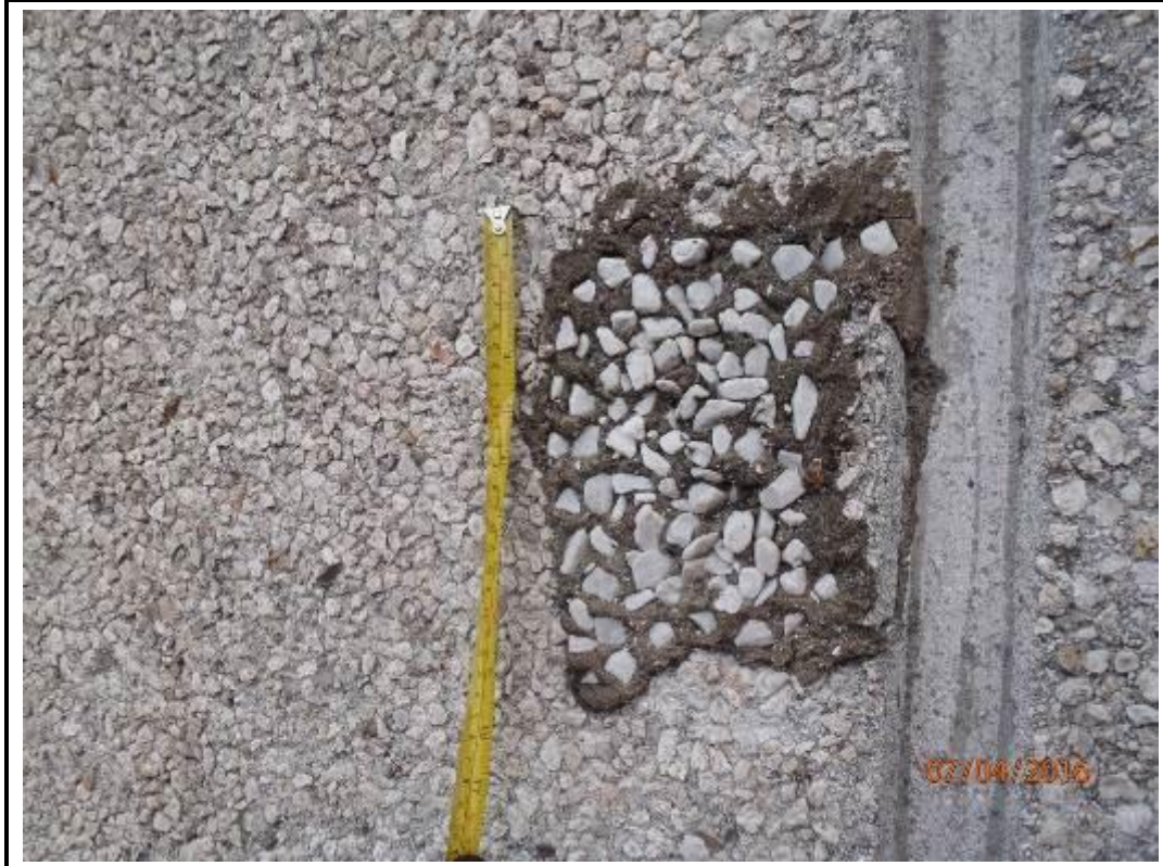
Photo 225. Drop 13 – West Elevation
