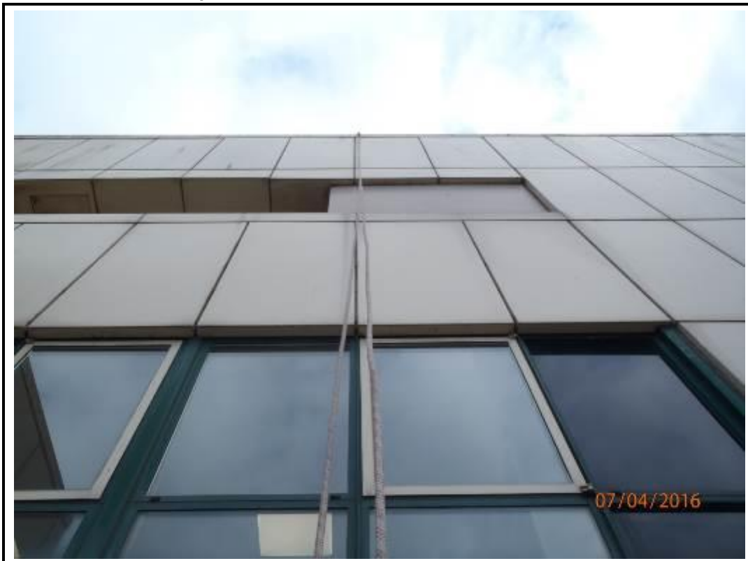
Photo 234. Drop 3 – North Elevation
