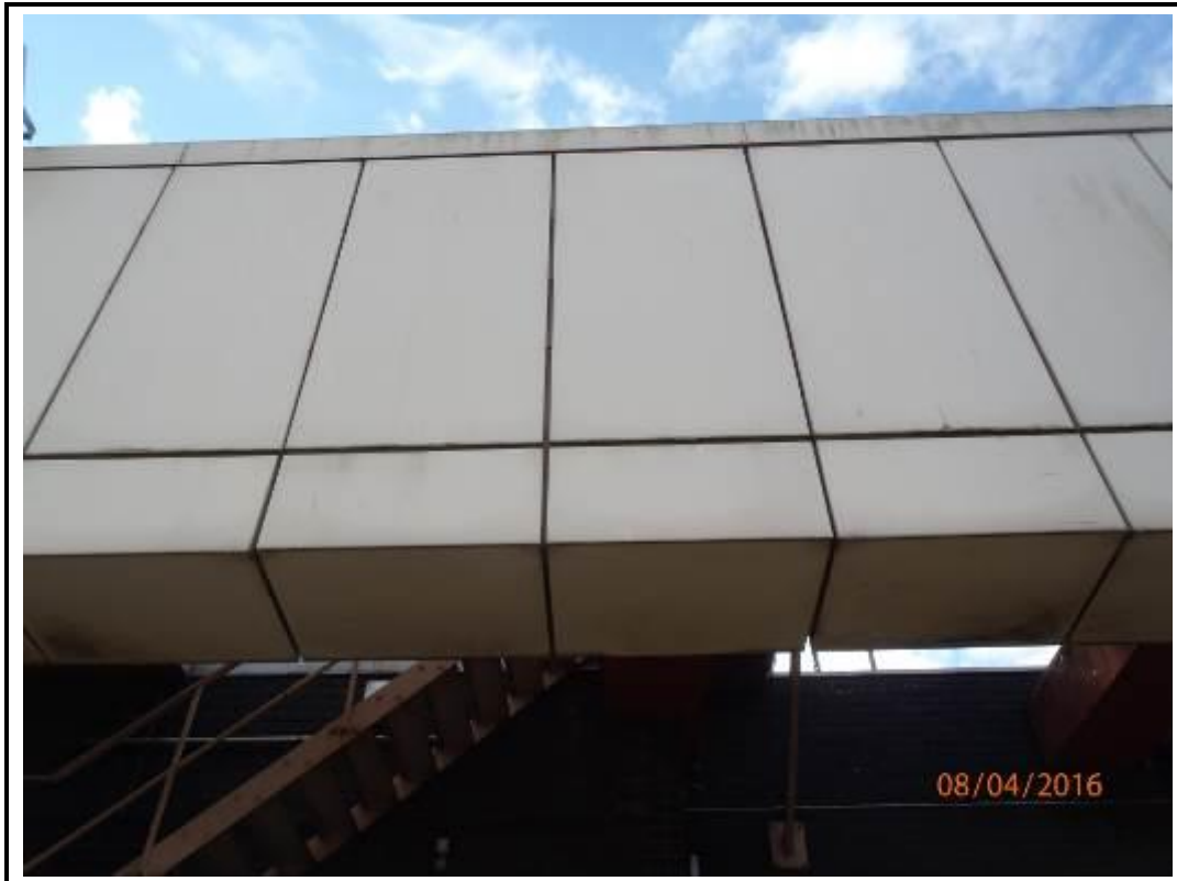
Photo 253. Drop 8 – North Elevation
