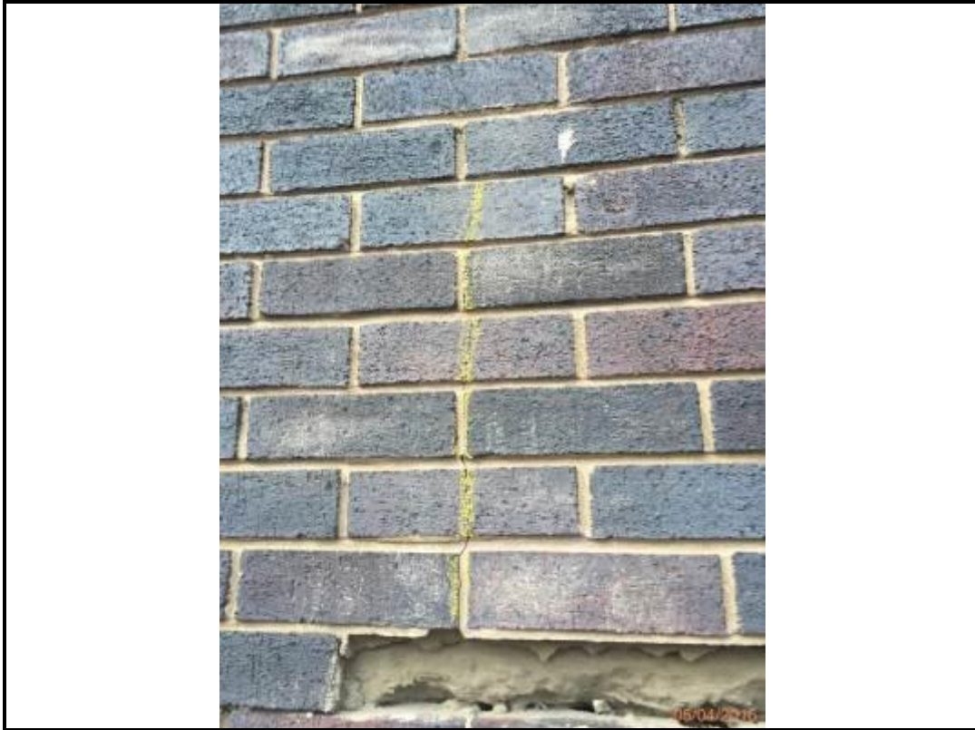
Photo 117. Drop 13 – South Elevation
