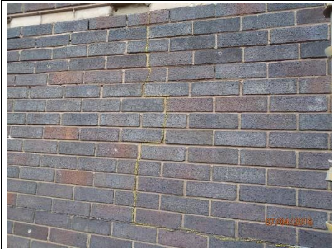
Photo 215. Drop 11 – West Elevation
