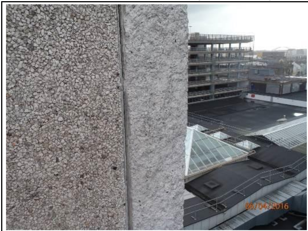
Photo 166. Drop 1 – West Elevation
