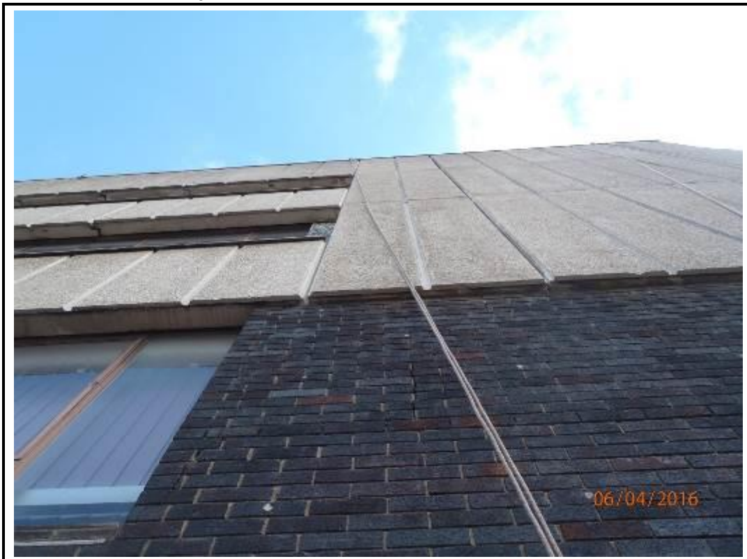
Photo 182. Drop 3 – West Elevation
