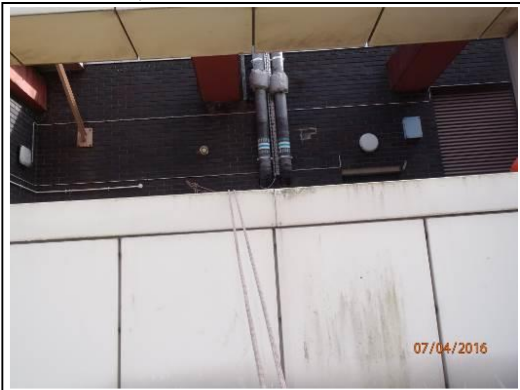
Photo 246. Drop 6 – North Elevation
