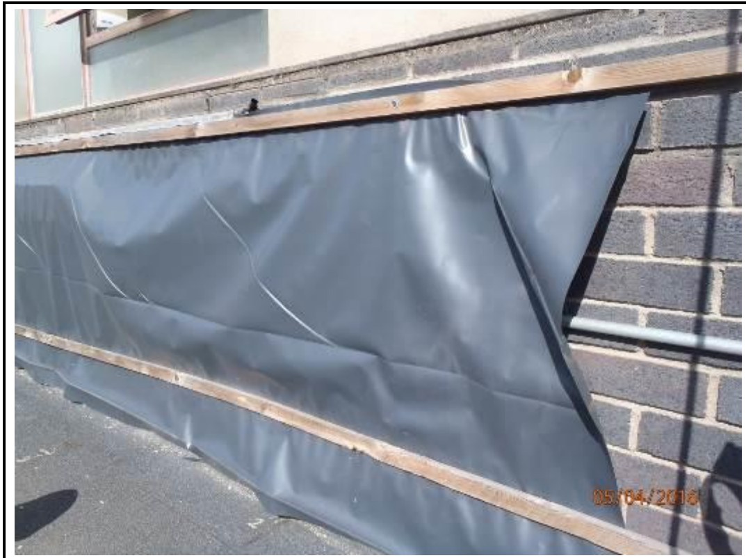
Photo 87. Drop 7 – South Elevation
