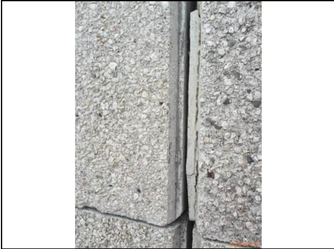
Photo 137. Drop 15 – South Elevation
