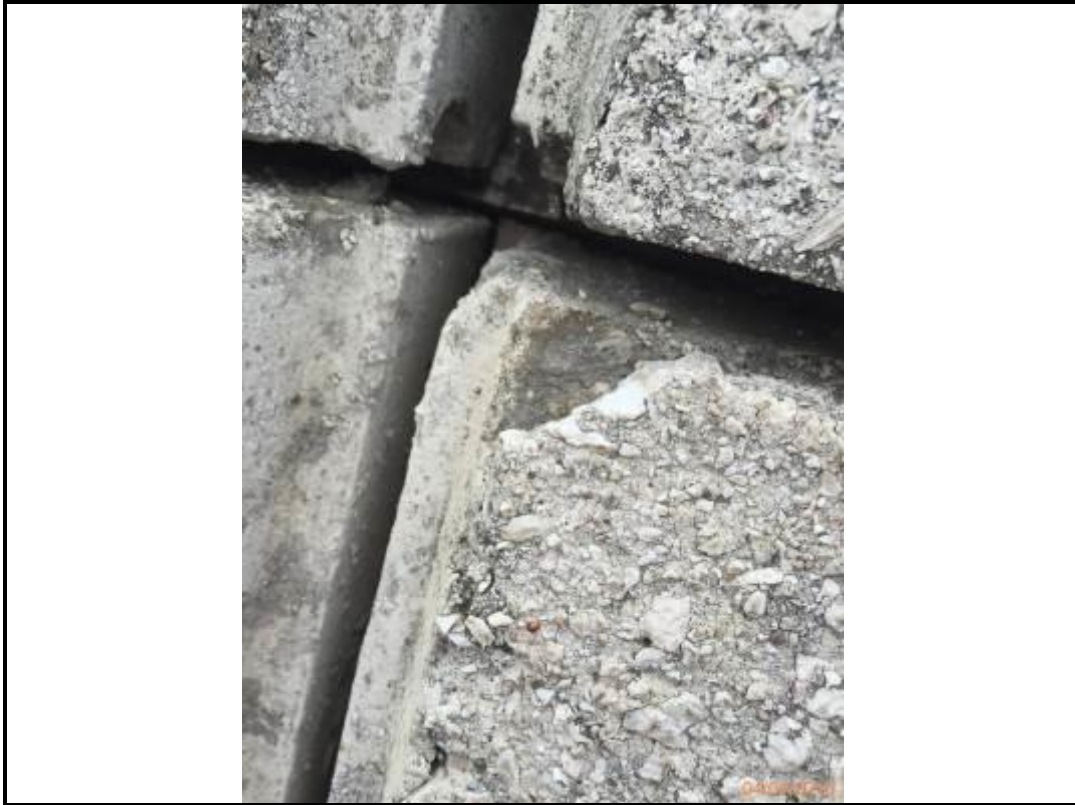
Photo 25. Drop 8 – East Elevation
