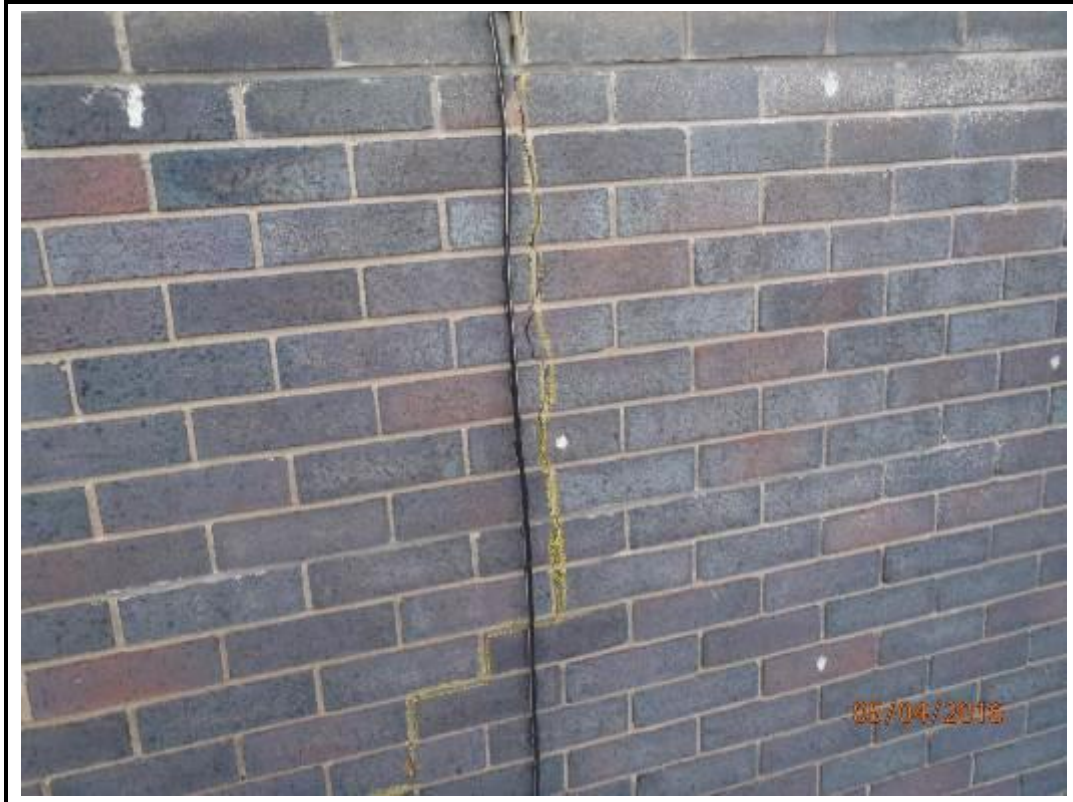
Photo 131. Drop 14 – South Elevation
