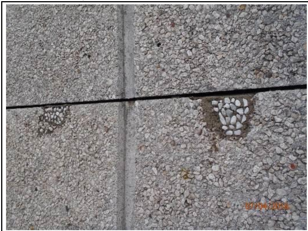
Photo 224. Drop 13 – West Elevation
