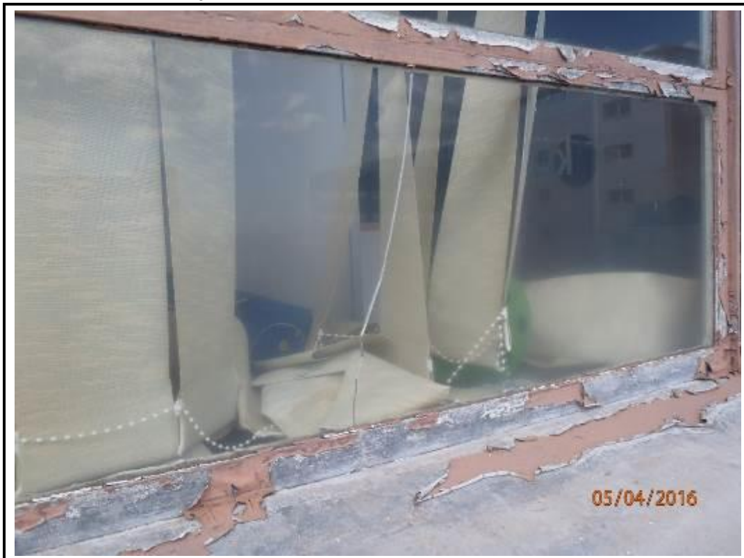
Photo 100. Drop 10 – South Elevation
