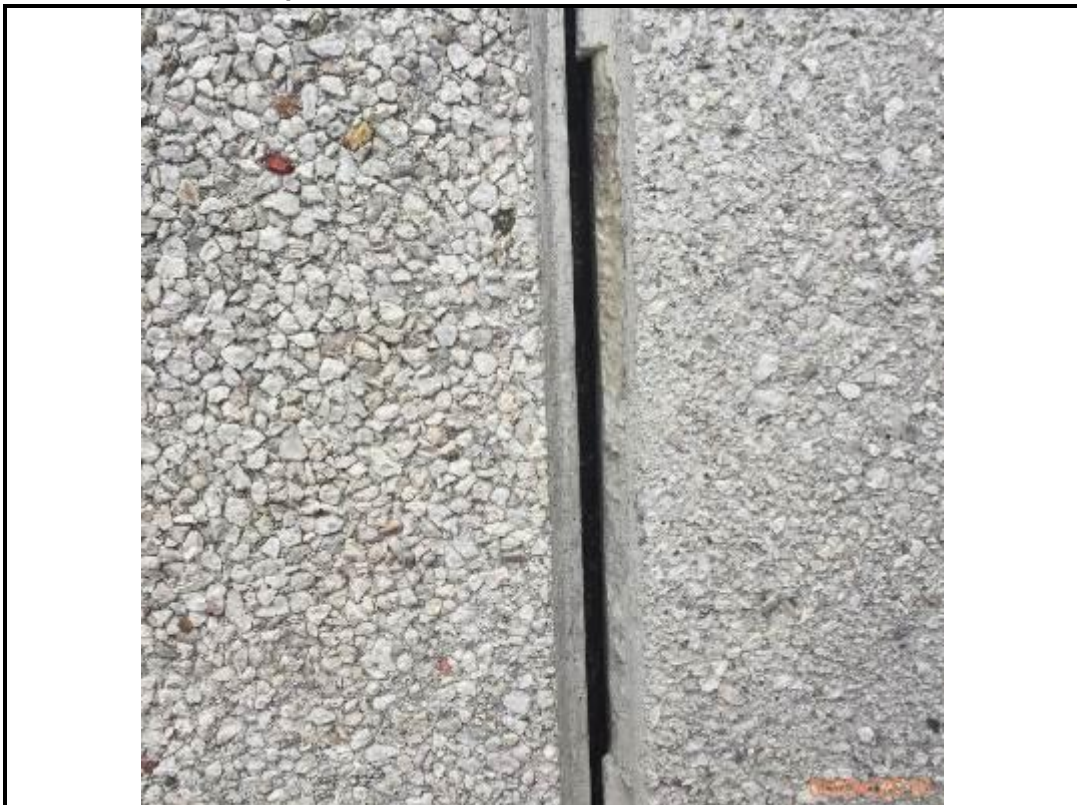
Photo 110. Drop 13 – South Elevation
