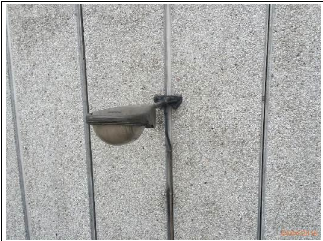
Photo 22. Drop 7 – East Elevation
