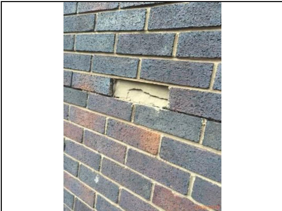
Photo 120. Drop 13 – South Elevation
