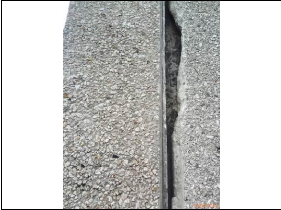
Photo 135. Drop 15 – South Elevation
