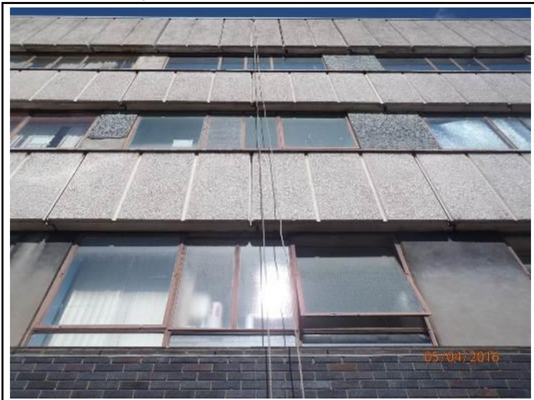
Photo 94. Drop 8 – South Elevation
