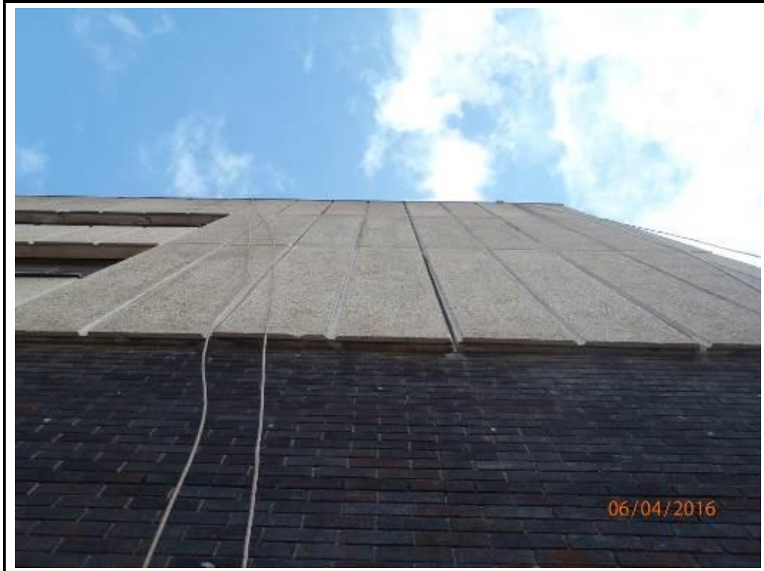
Photo 177. Drop 2 – West Elevation
