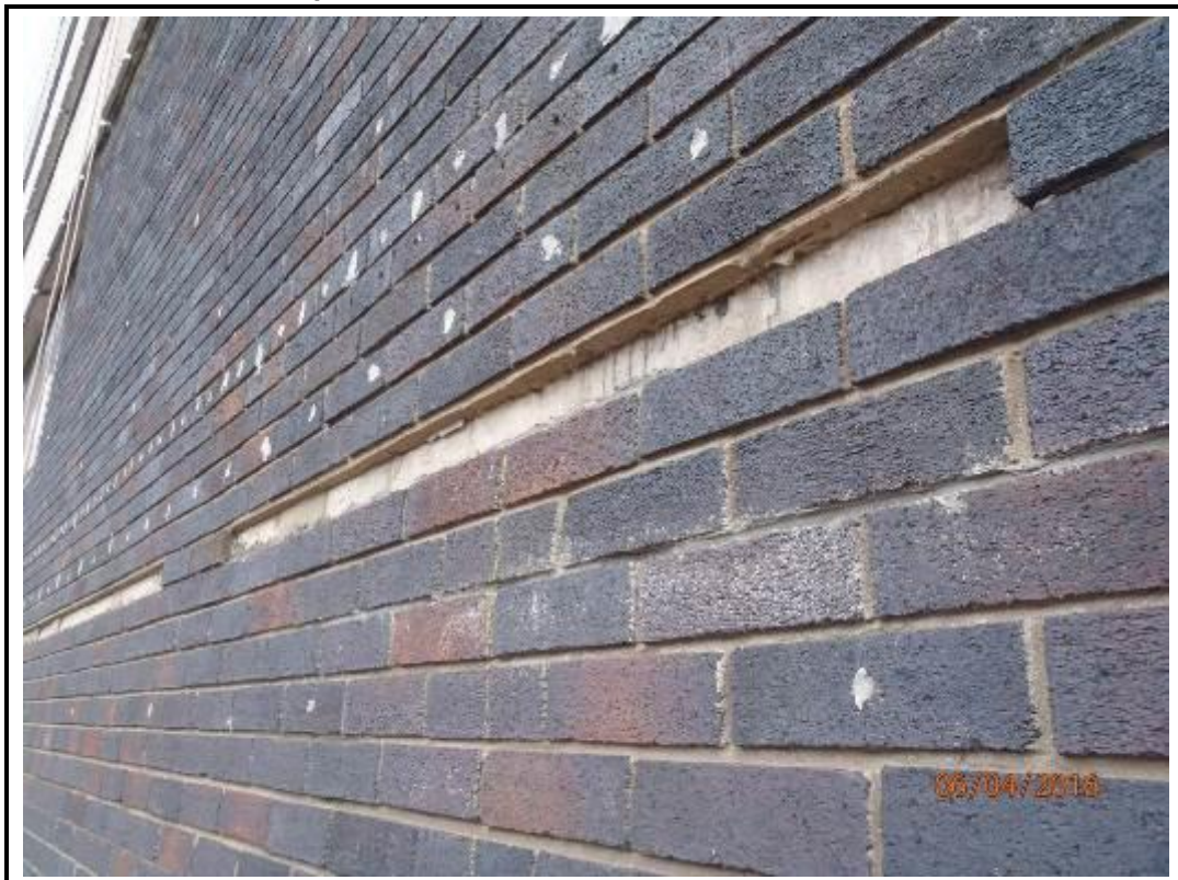
Photo 170. Drop 1 – West Elevation
