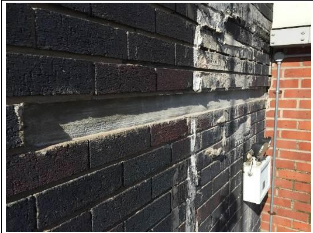
Photo 55. Drop 1 – South Elevation
