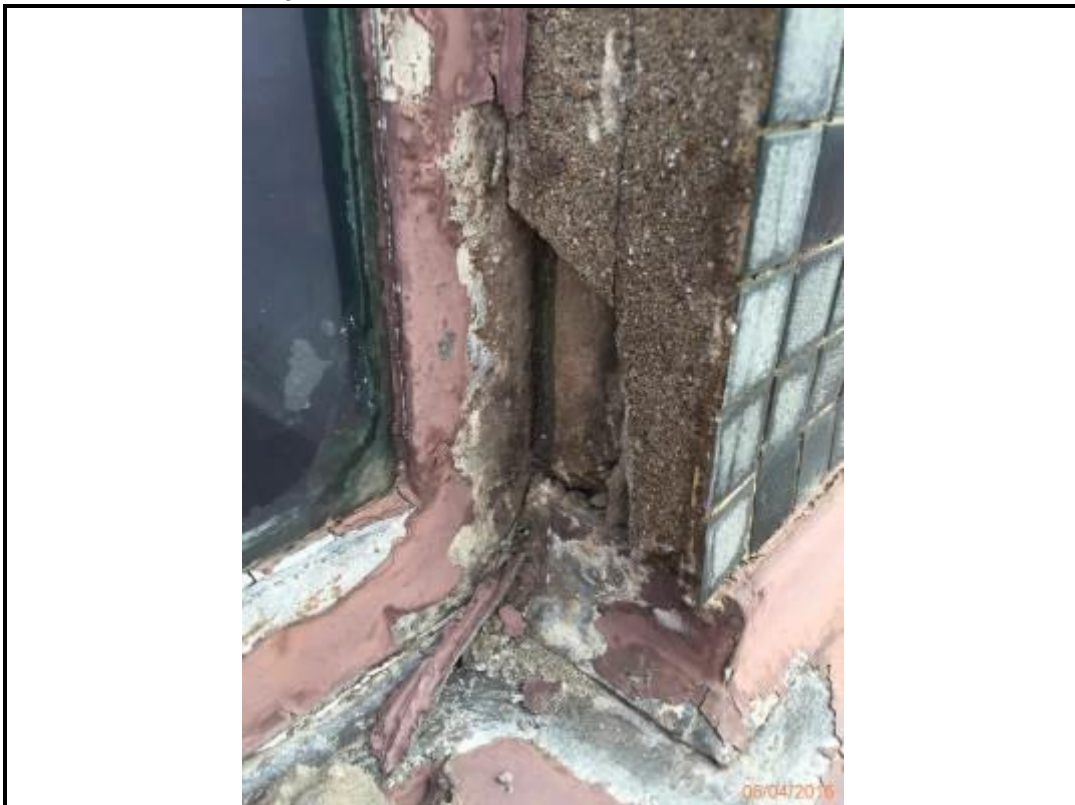
Photo 188. Drop 5 – West Elevation
