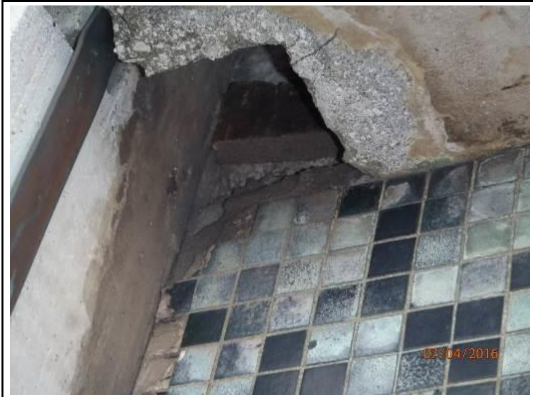
Photo 207. Drop 11 – West Elevation
