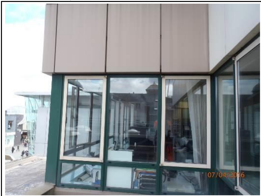
Photo 240. Drop 4 – North Elevation
