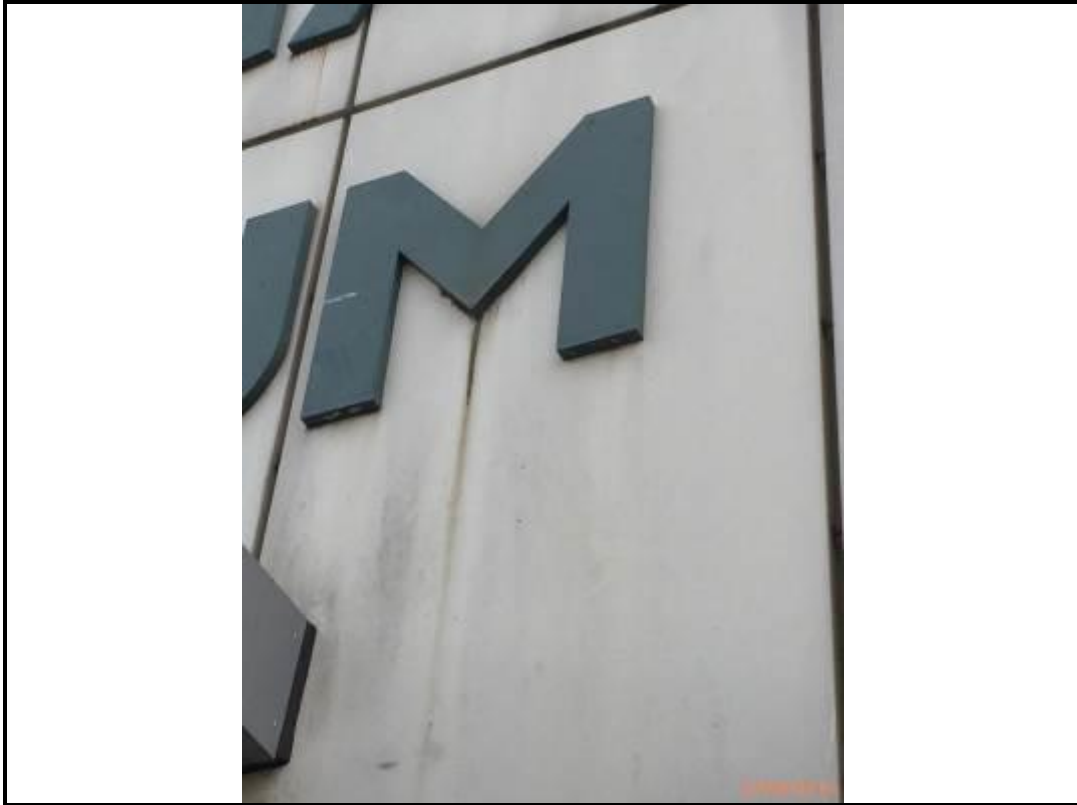
Photo 265. Drop 13 – North Elevation
