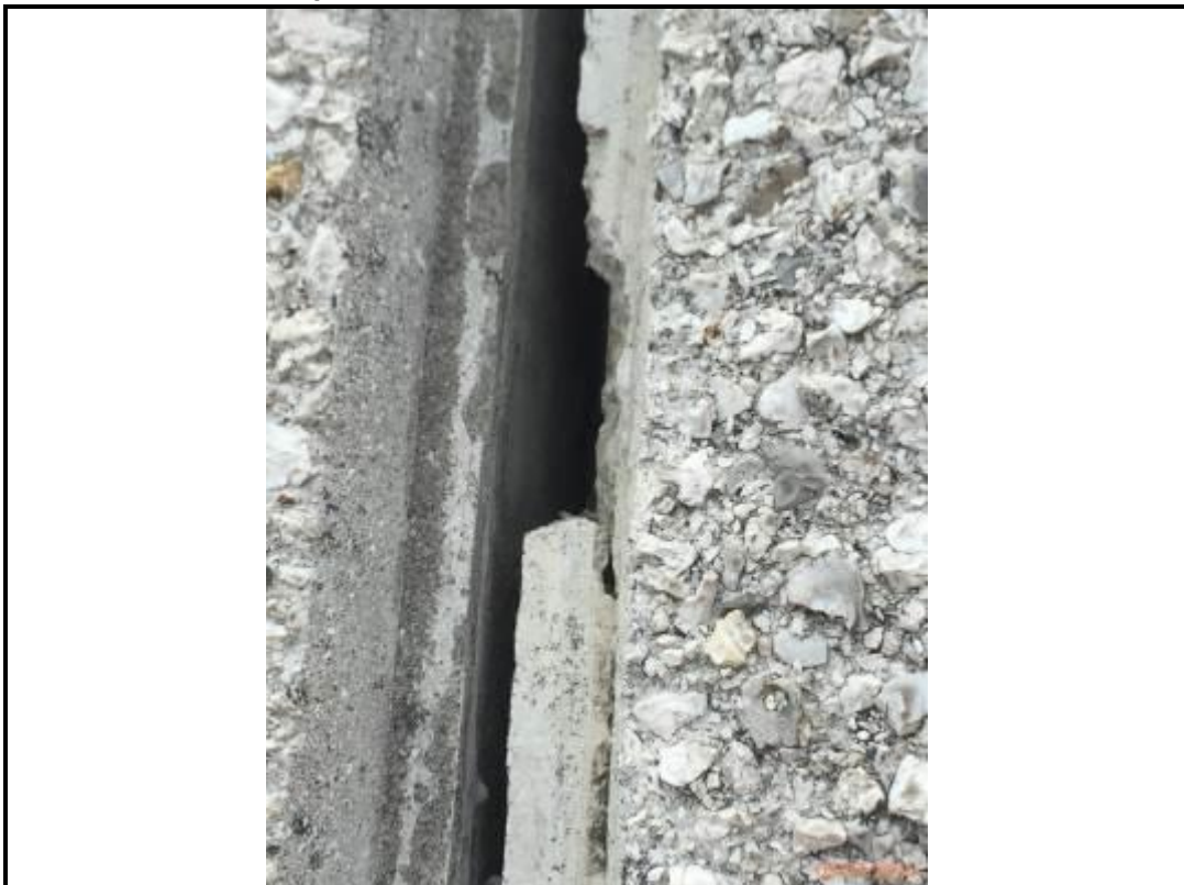
Photo 136. Drop 15 – South Elevation
