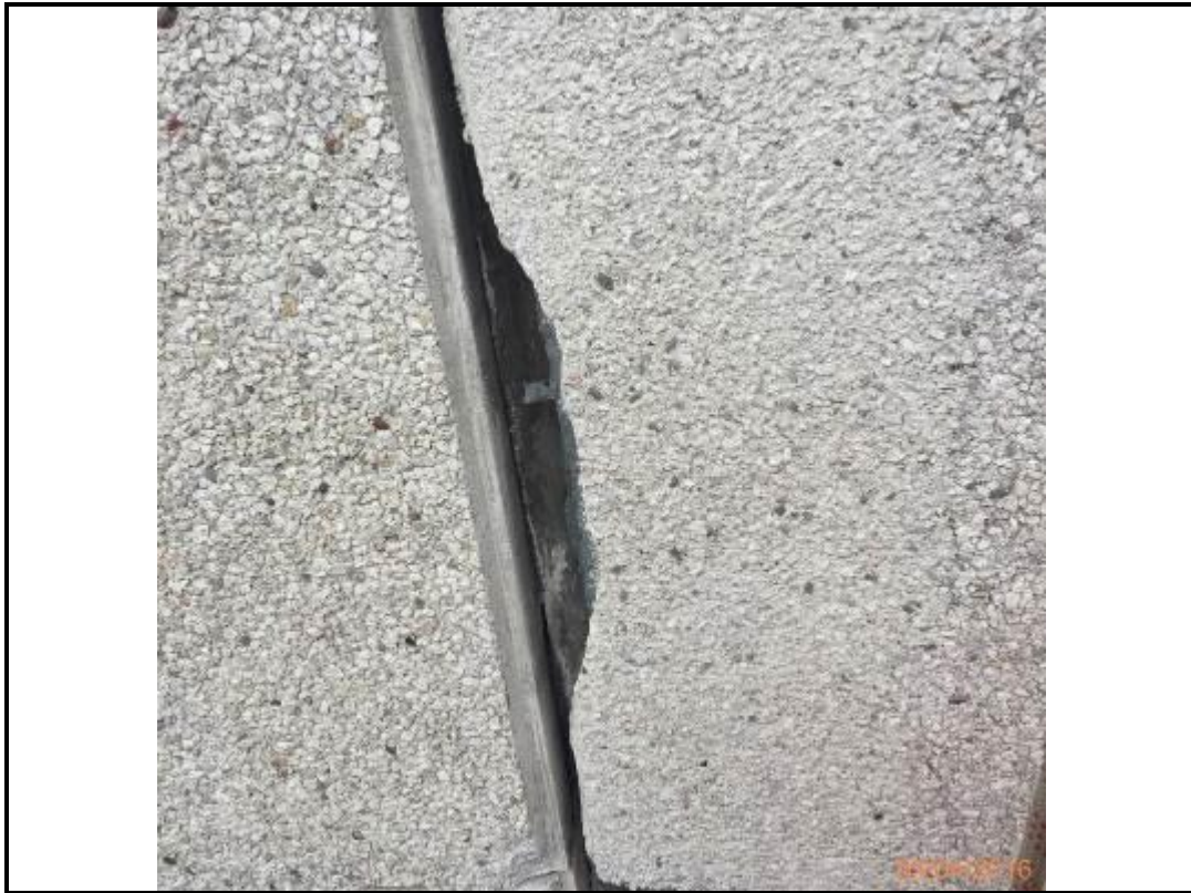
Photo 111. Drop 13 – South Elevation
