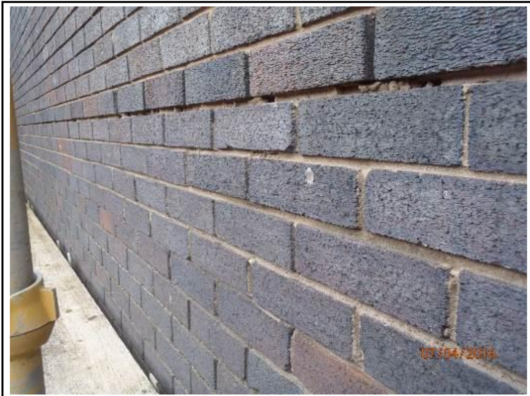
Photo 212. Drop 11 – West Elevation
