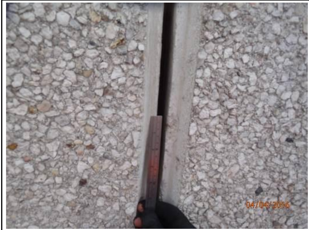
Photo 3. Drop 1 – East Elevation
