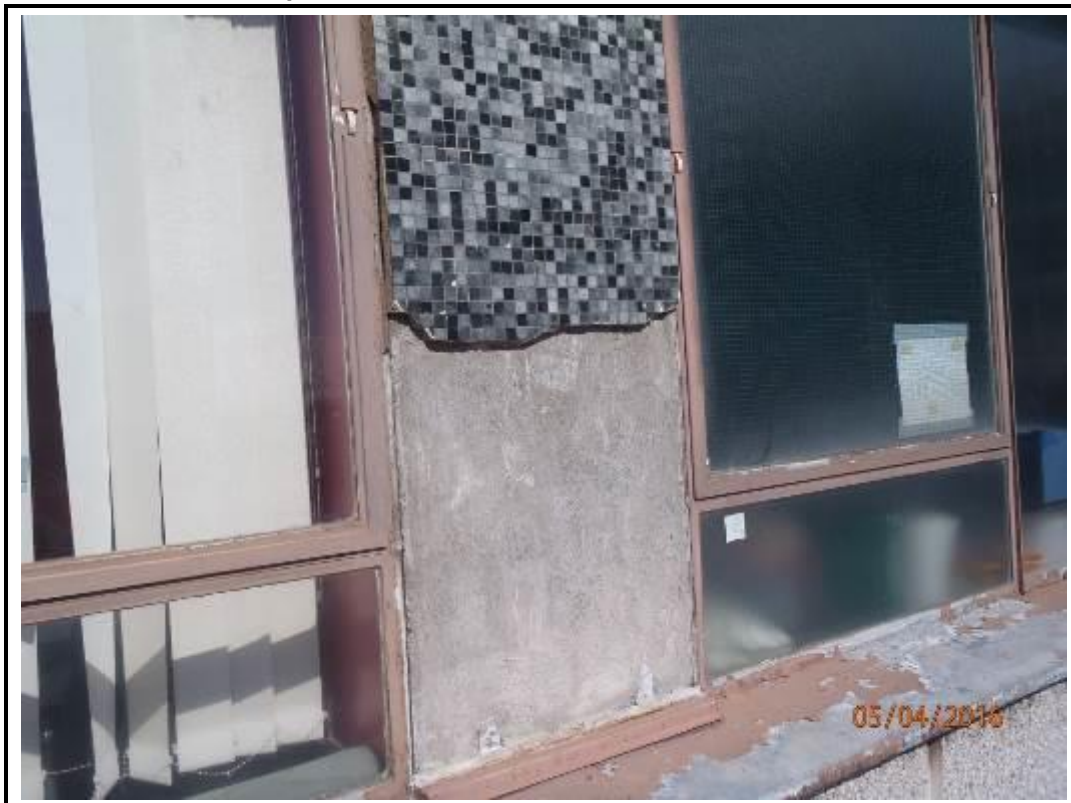
Photo 96. Drop 9 – South Elevation
