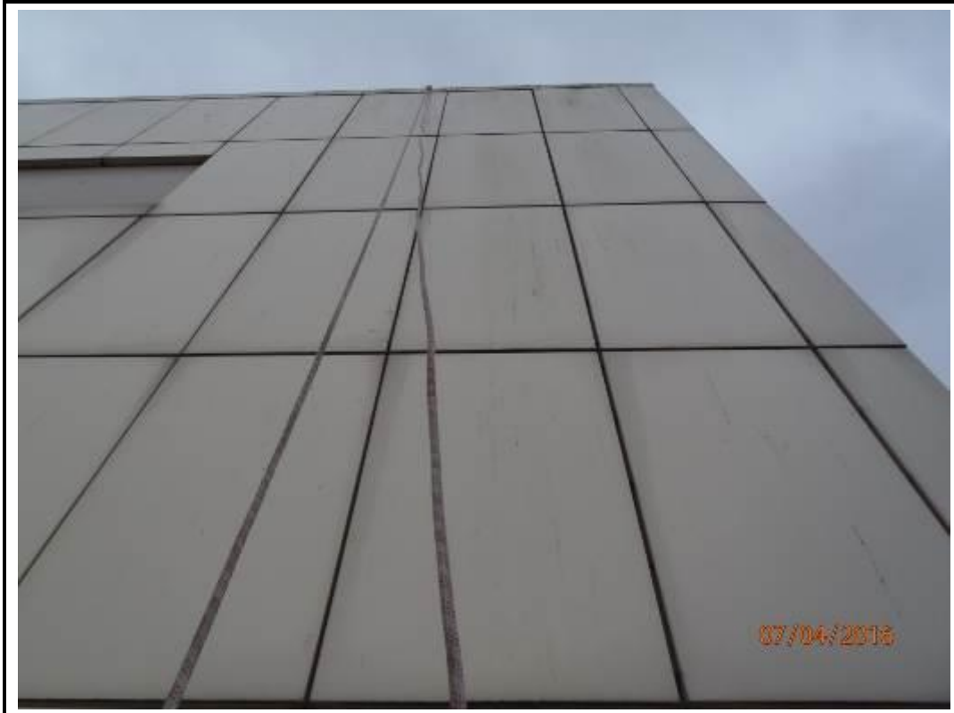
Photo 229. Drop 1 – North Elevation
