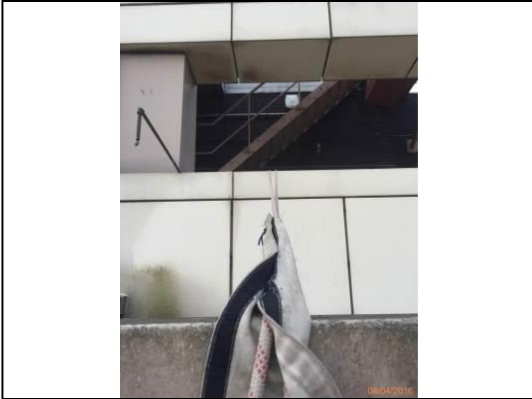
Photo 255. Drop 9 – North Elevation
