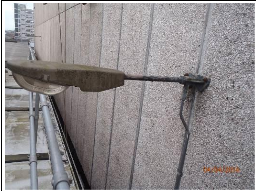
Photo 7. Drop 1 – East Elevation
