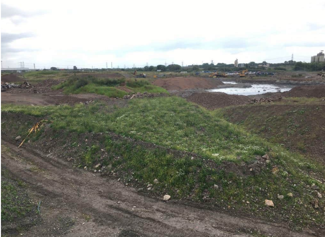
Photograph 4 (16/08/21) Northern boundary of 4g, in use as a stockpiling area for the concrete processing works.
