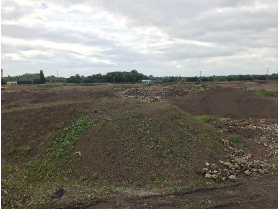
Photograph 5 (16/08/21) Central-western part of phase 4g, occupied by stockpiles of processed material.
