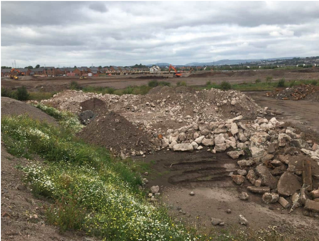
Photograph 1 (16/08/2021) Western boundary of Phase 4g, in use as a concrete stockpiling area.
