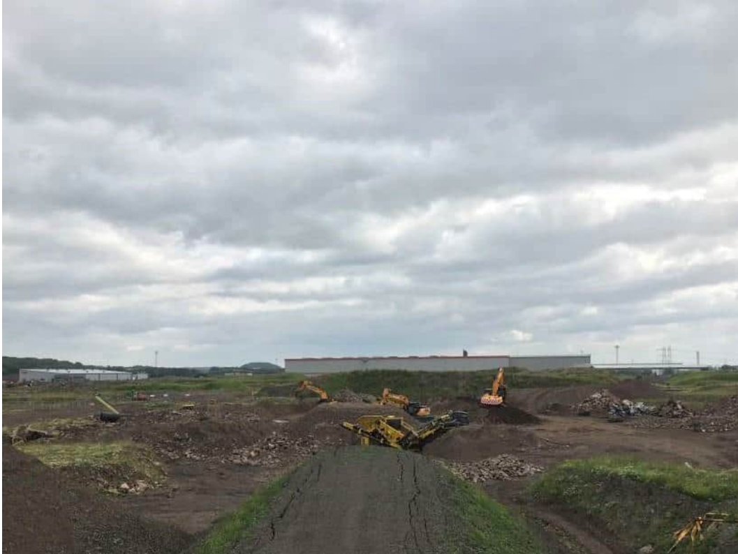
Photograph 3 (16/08/2021) Central part of 4g in use as a concrete screening and processing area.
