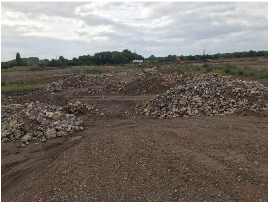
Photograph 6 (16/08/2021) Southern boundary of 4g, occupied by unprocessed concrete. In the south by a haul route and the west by surface water reen.
