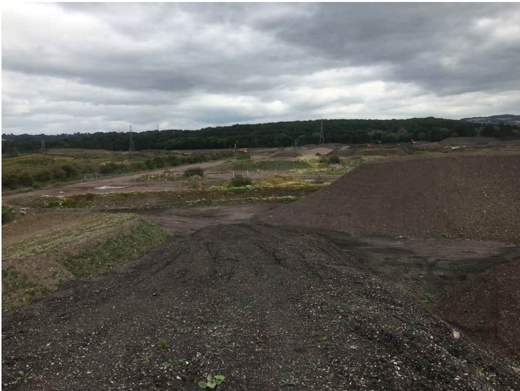
Photograph 2 (16/08/2021) North-west boundary of 4g occupied by stockpiles of fines produced from concrete processing. An east west trending reeN bounds the phase to the north.
