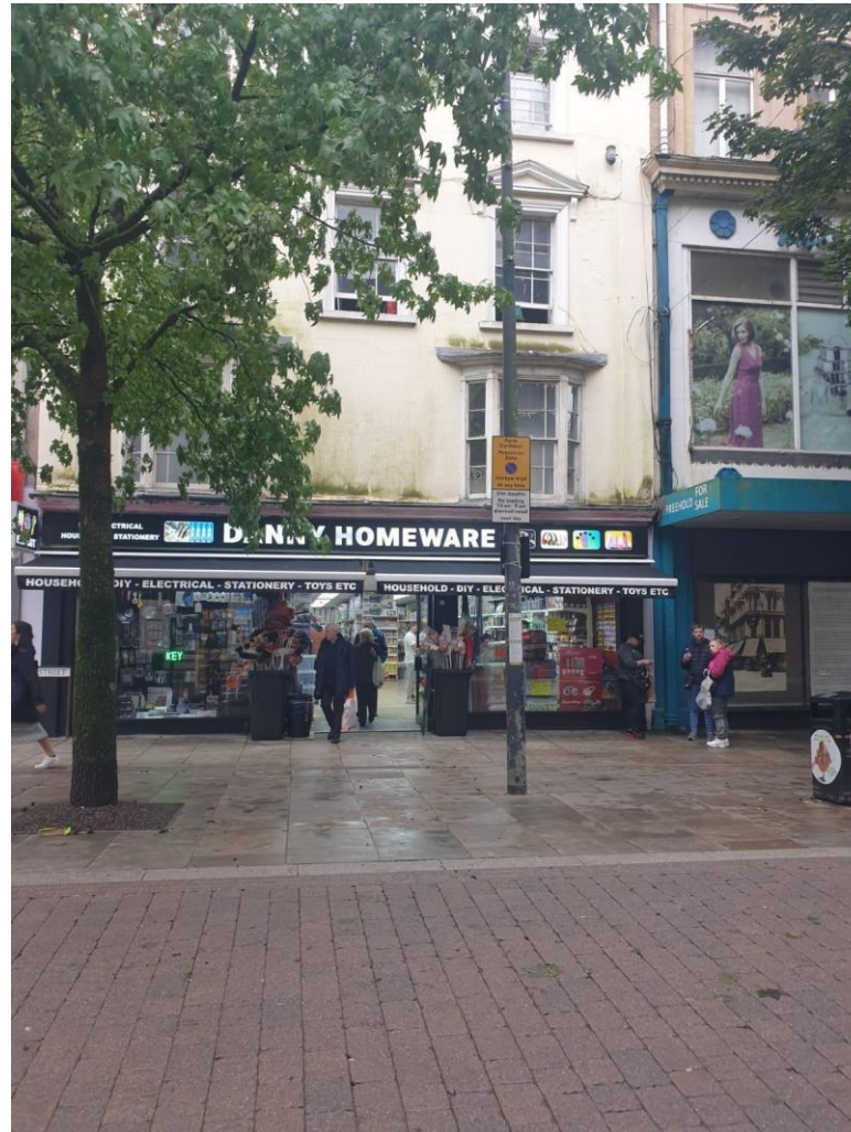
Fig 2: Showing Existing Street view from Commercial Street.
