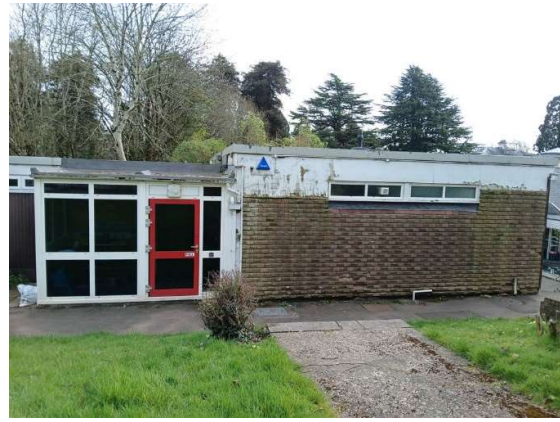
West Elevation (South end)
