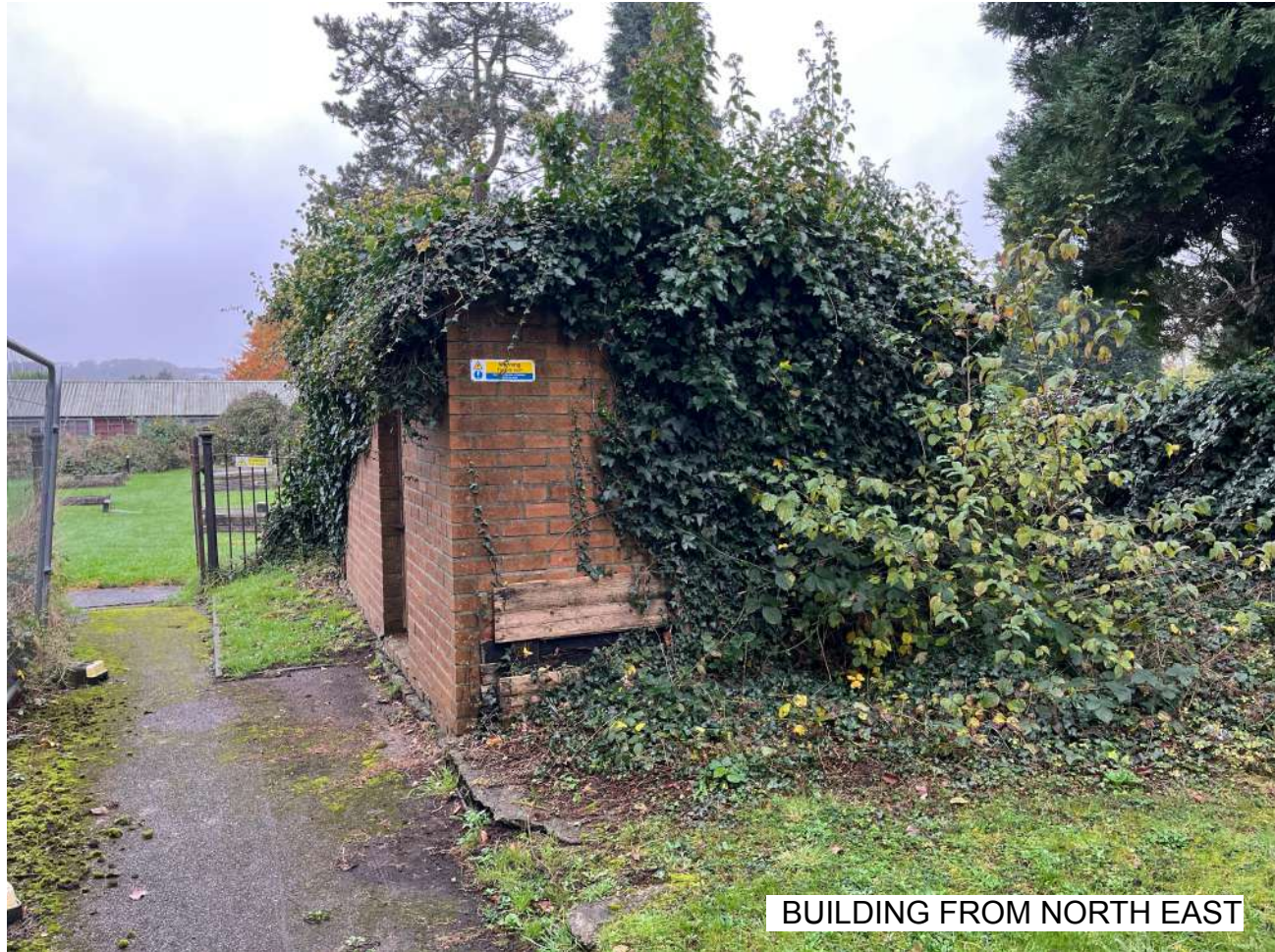
BUILDING FROM NORTH EAST
