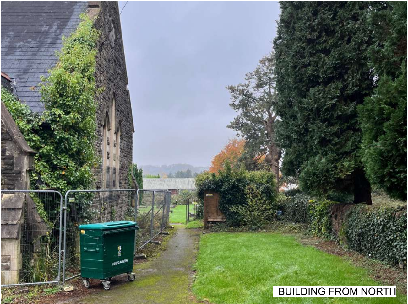
BUILDING FROM NORTH
