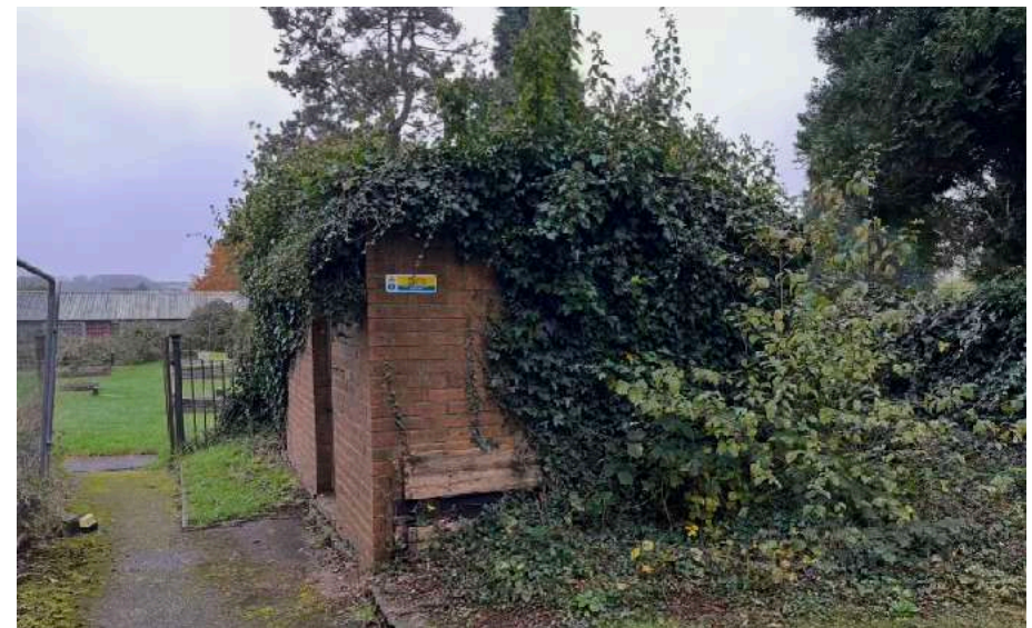
(Top) View of the gable end, from the southwest, showing the Church's main entrance. (Bottom) View of the outbuilding from the north.
