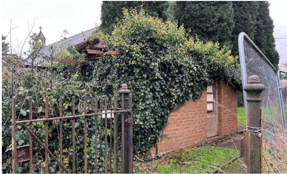
Existing outbuilding from the south
