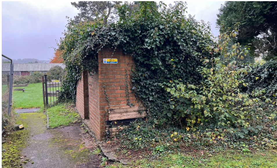
Existing outbuilding from the north, small dogwood sapling shown in foreground
