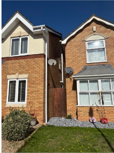
Fig. 2 Two stories close to landing windows in the area
