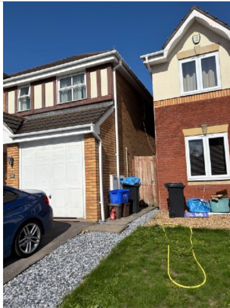
Fig. 3 Two stories close to landing windows in the area
