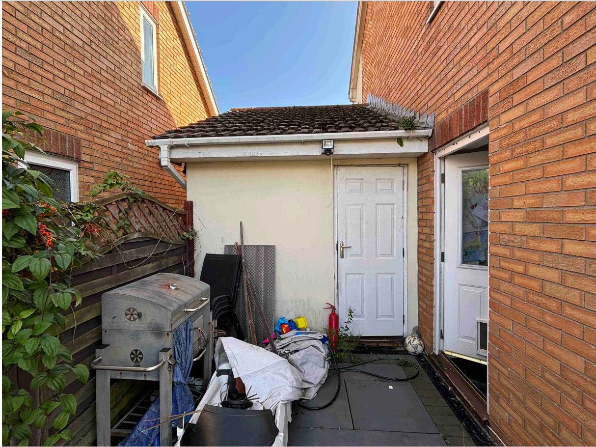
Fig. 5 Paved area of proposed extension
