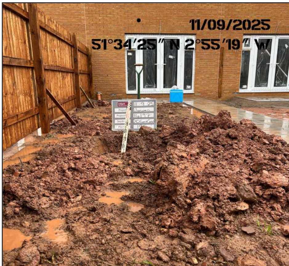
Plot 193 Soil Capping Depth Check
