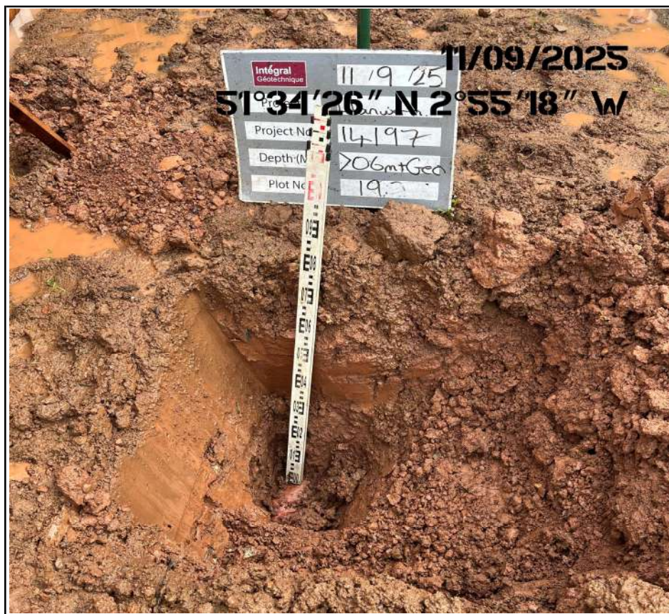
Plot 193 Trial Pit Excavation
