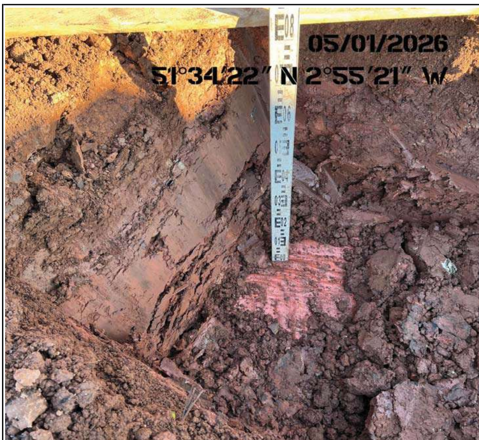
Plot 110 Membrane Placement
