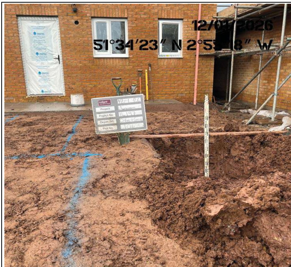
Plot 106 Soil capping Depth Check
