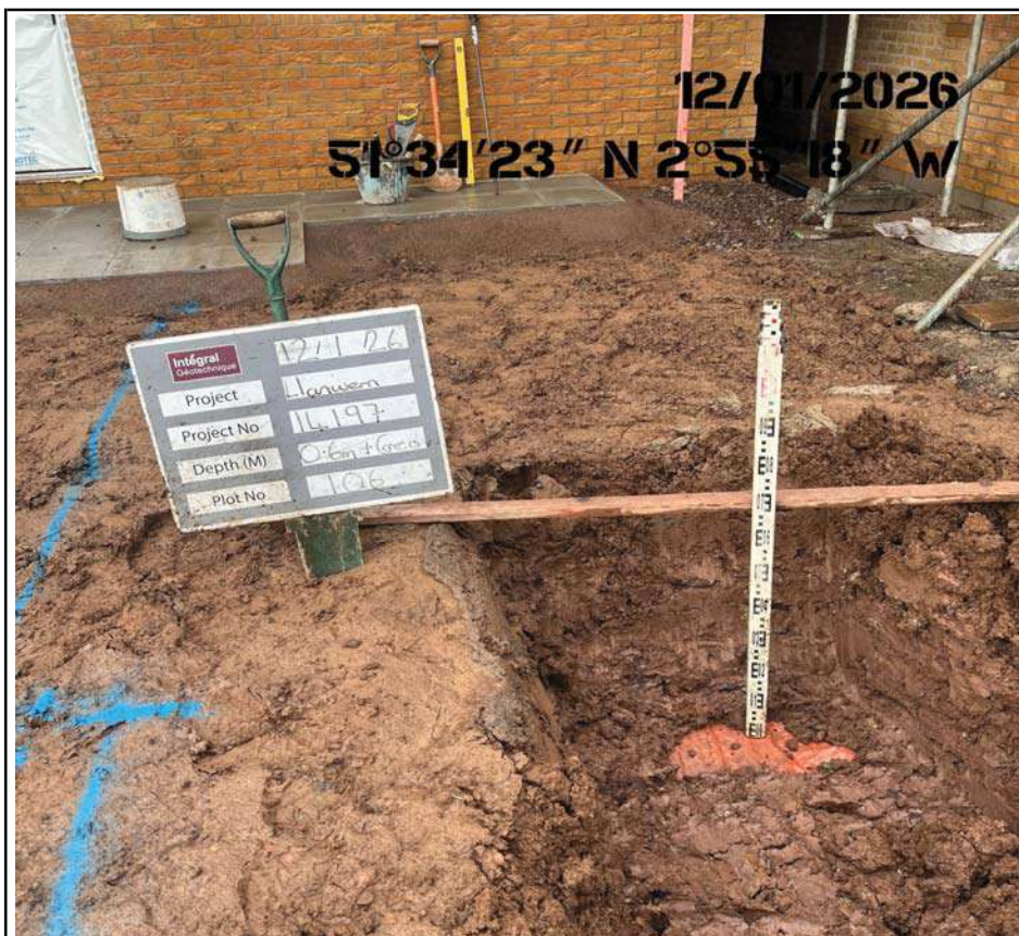
Plot 106 Trial Pit Excavation
