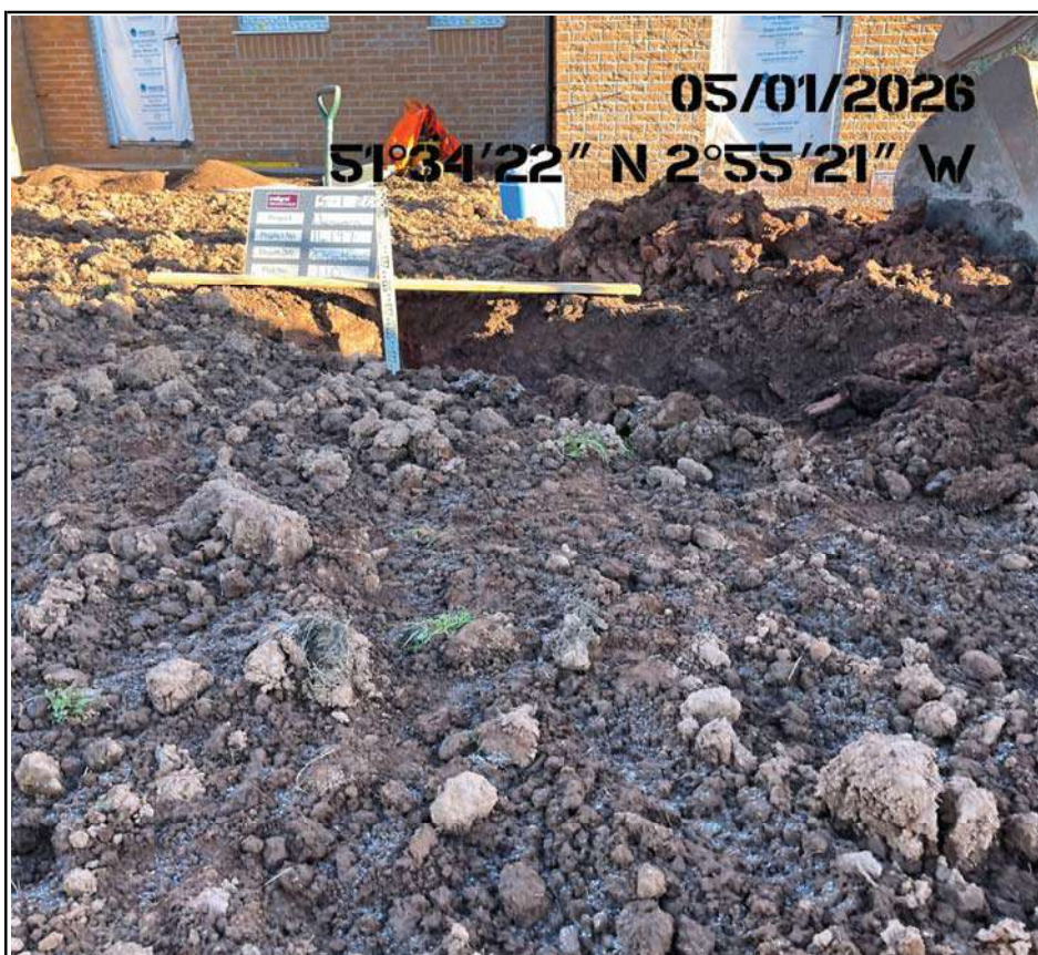
Plot 110 Soil Capping Depth Check
