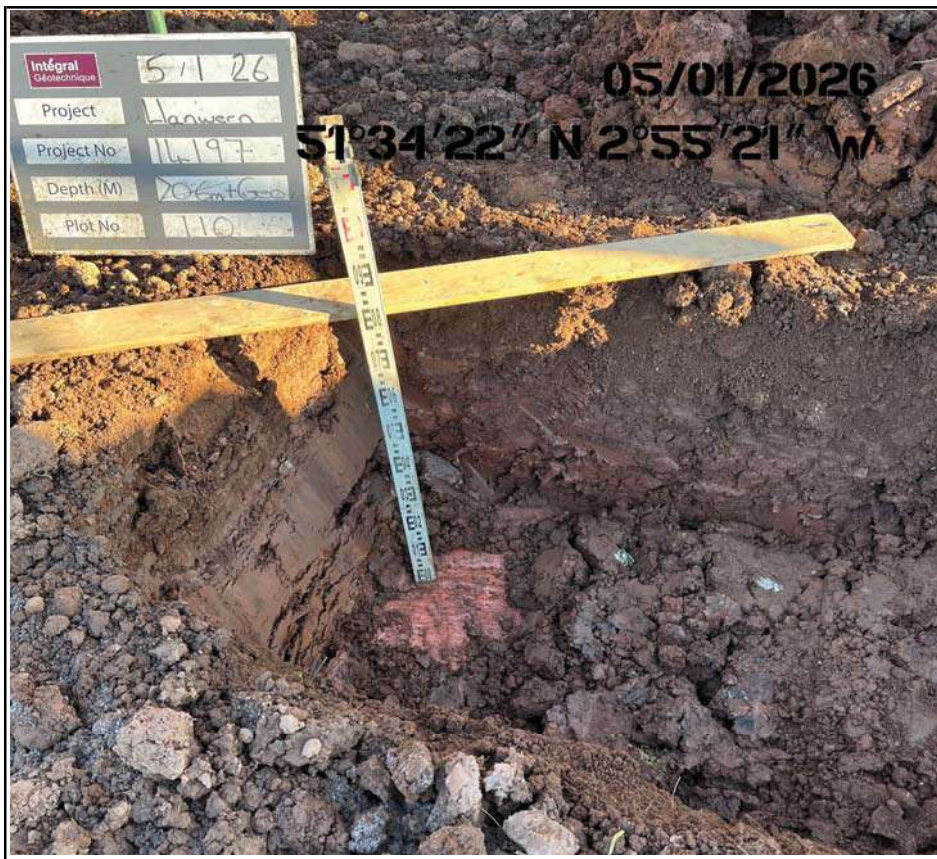
Plot 10 Trial Pit Excavation
