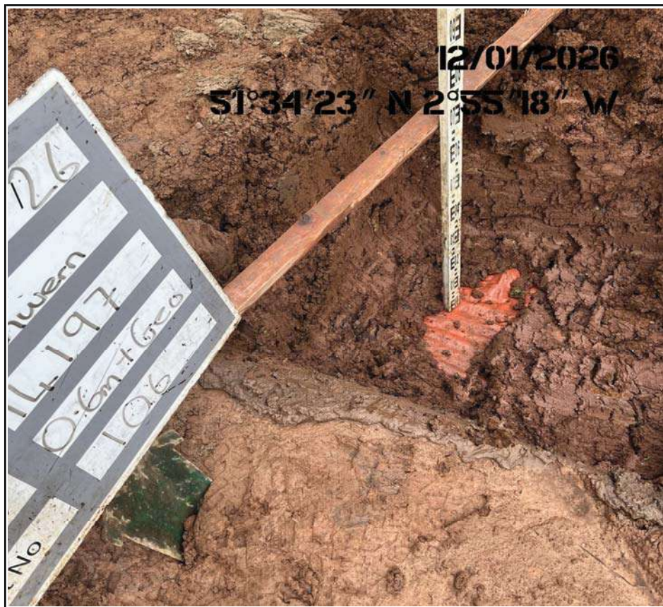
Plot 106 Membrane Placement
