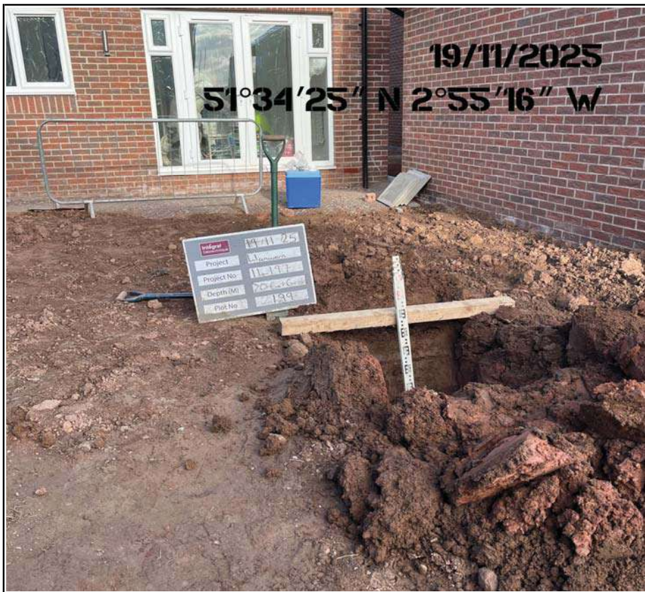
Plot 199 Soil Capping Depth Check
