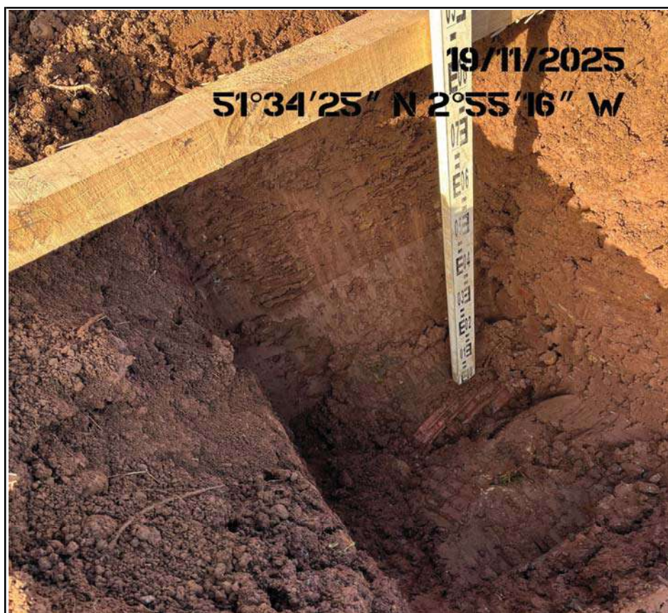
Plot 212 membrane Placement at Base of Capping Soils
