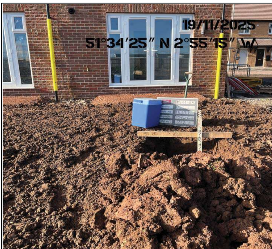
Plot 212 Soil Capping Depth Check
