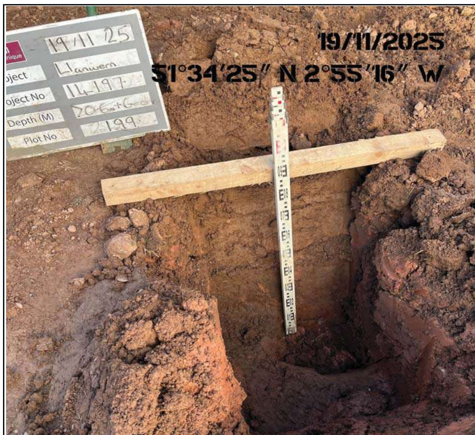
Plot 199 Trial Pit & Membrane Placement
